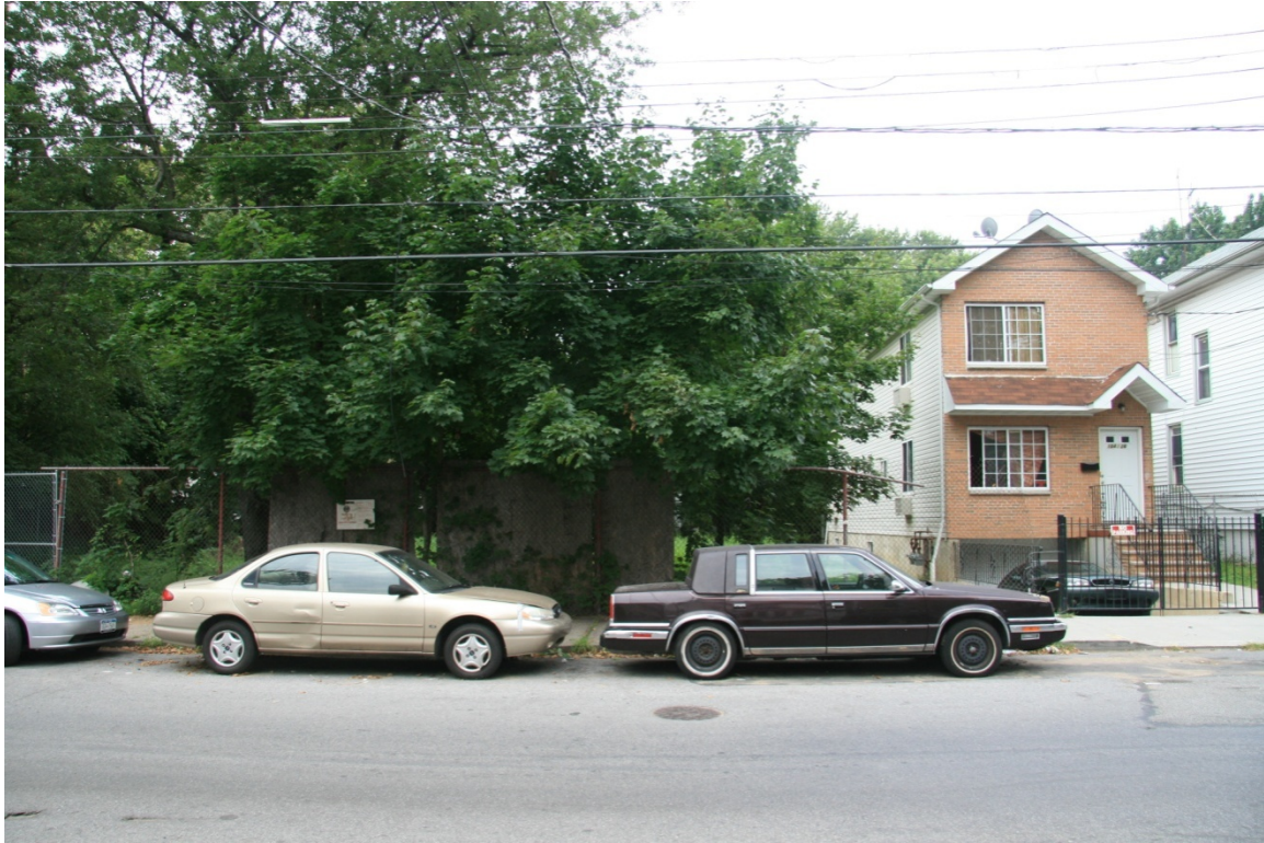
Image 22: Site prior to foundation installation
