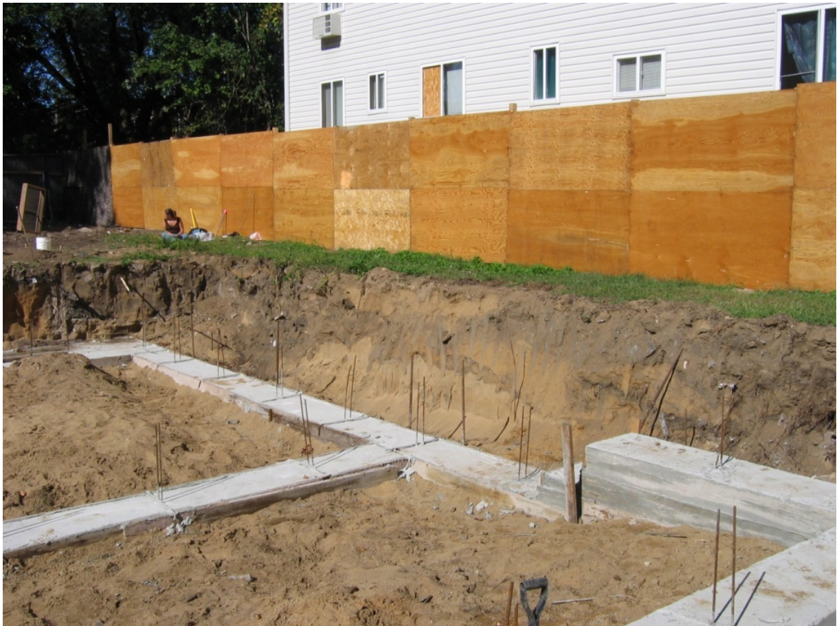
Figure 21: View of stratigraphic layers of the foundation trench
