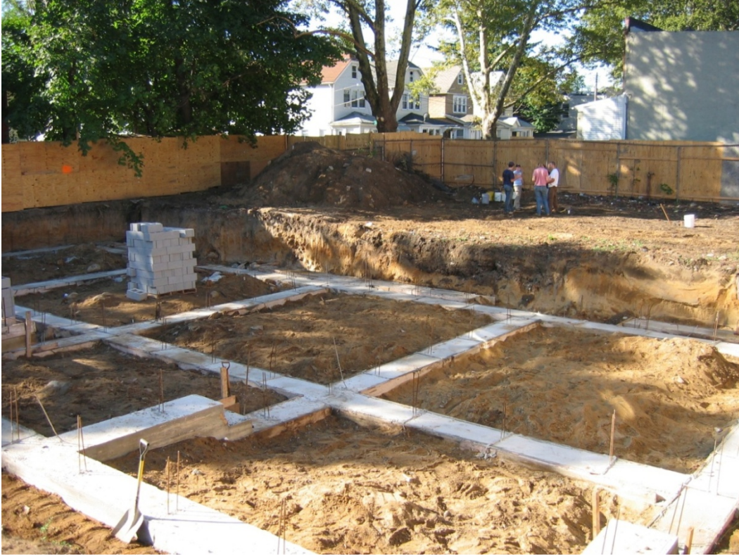
Image 27: new building foundation
