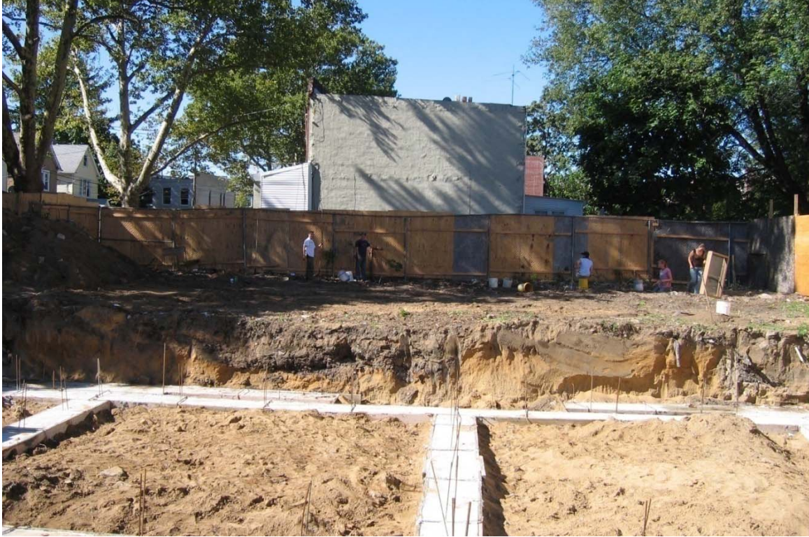
Figure 06: Foundation installed prior to excavation work commencing
