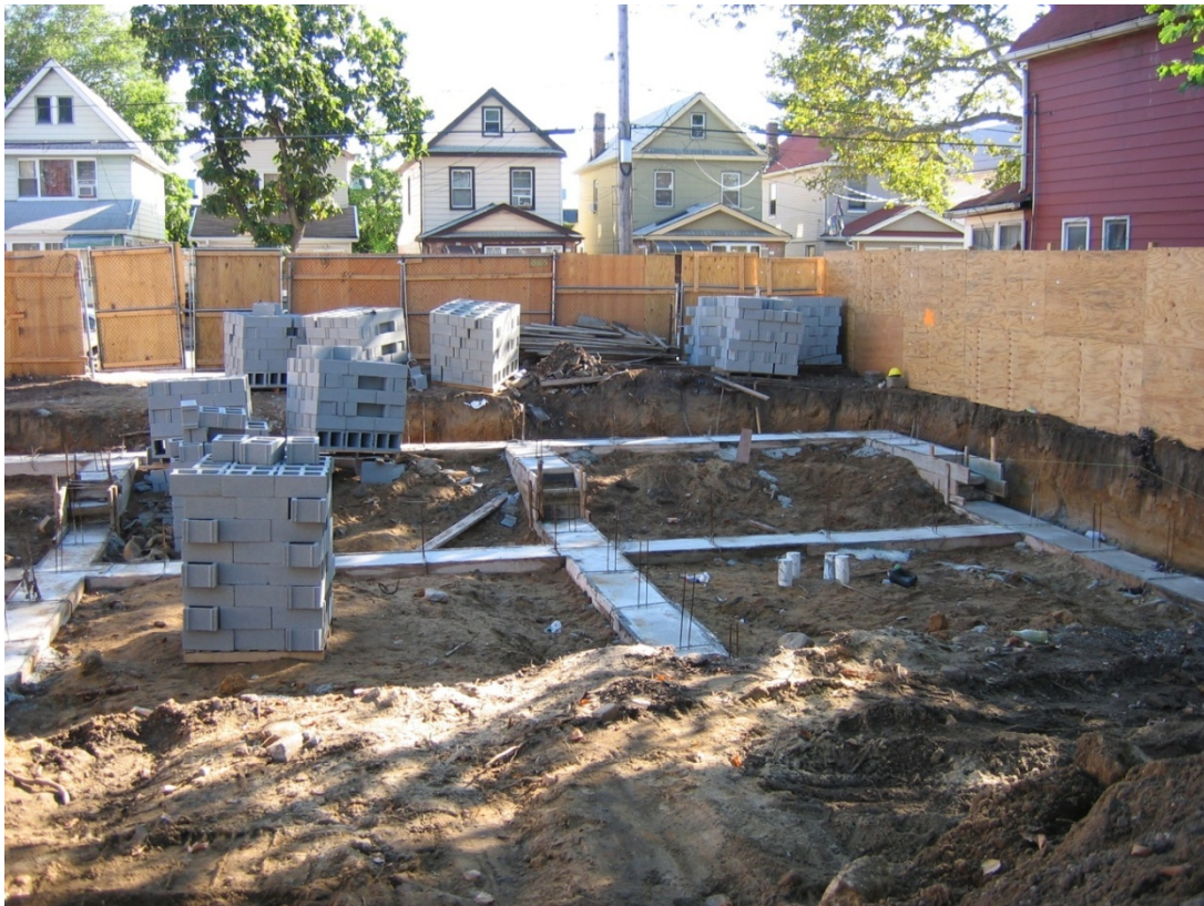
Image 28: new building foundation
