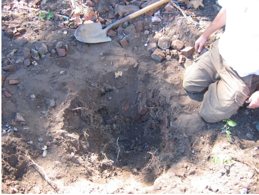
Figure 17: STP 18 – halted due to the abundance of construction debris within the STP
