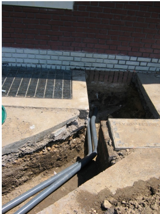
Image 51: House Electrical Line Excavation
