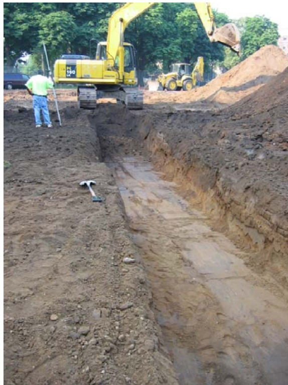
Image 16: Excavation for new drainage conduit
