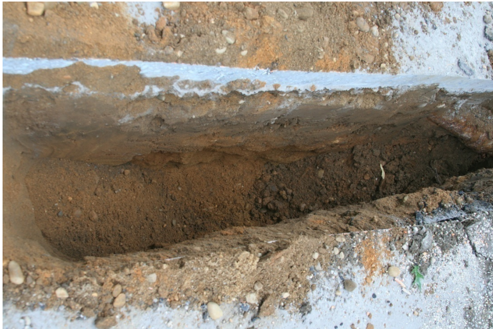
Image 15: Drain line excavation in progress
