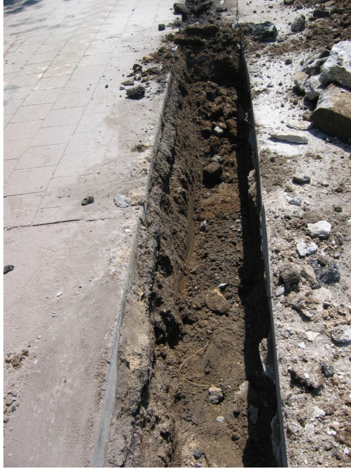
Image 14: Drain line excavation in progress
