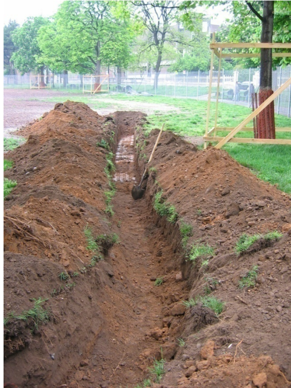
Image 08: Trenching for the new electrical line
