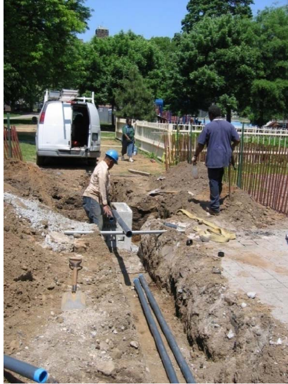
Image 09: Electrical trench installation – south of herb garden
