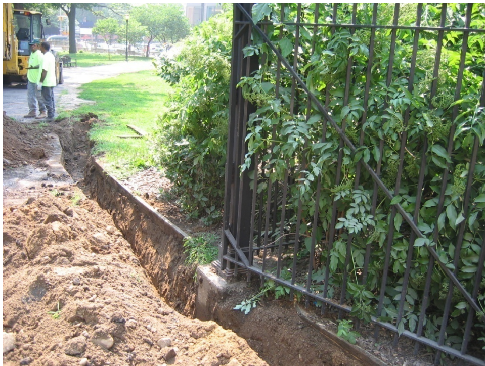
Image 49: House Electrical Line Excavation
