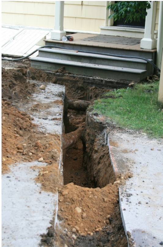
Image 50: House Electrical Line Excavation
