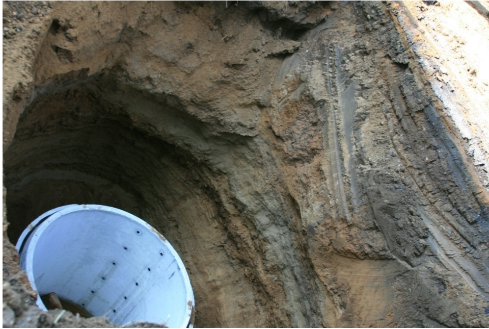
Image 11: Installation of holding tank as part of the pumping station
