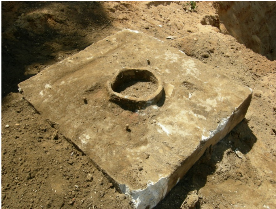
Image 37: Cast iron pipe protruding from concrete block
