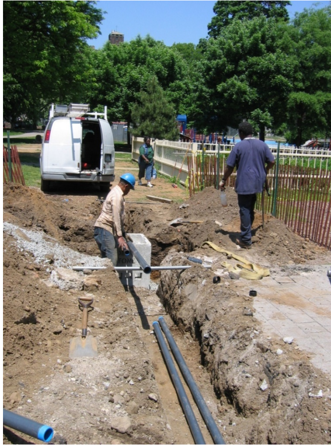
Image 52: House Electrical Line Excavation
