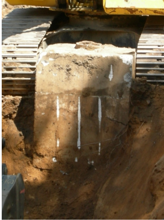
Image 38: Removal of cast iron pipe in concrete block
