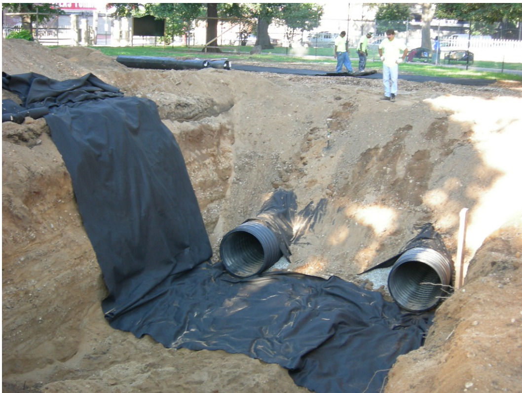
Image 34: Newly installed drainage conduits
