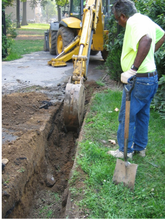
Image 28: Continuation of the electrical trench
