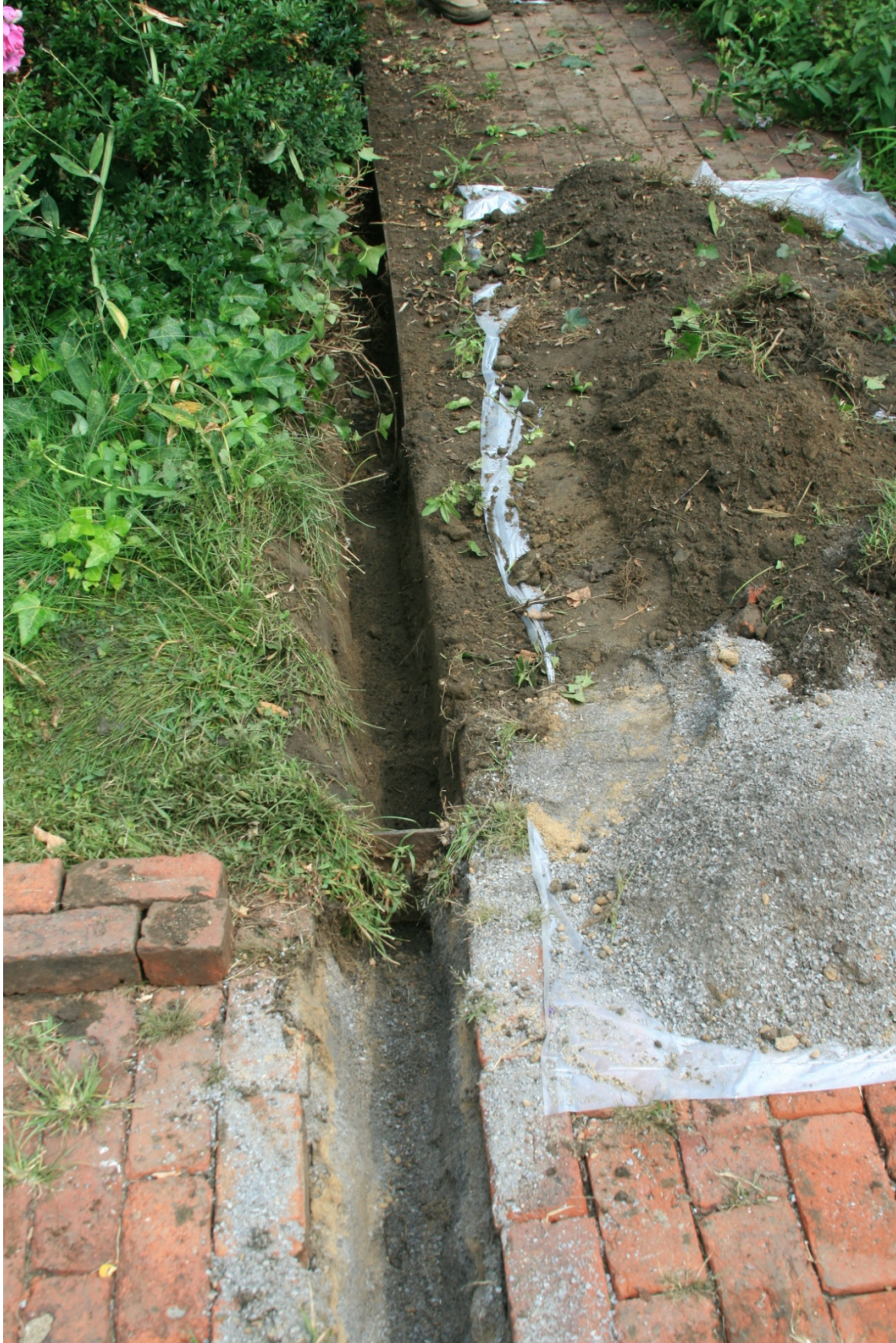
Figure 20: Area A – excavation for the new utility line
