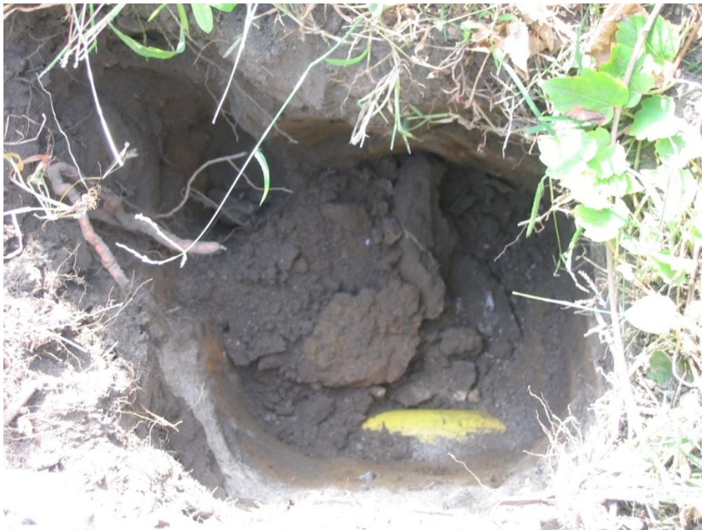
Figure 14: PVC gas line uncovered in Posthole #10
