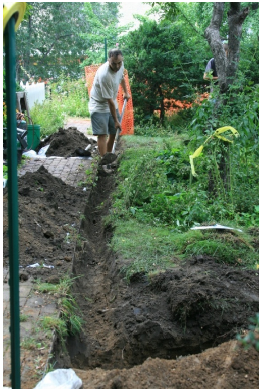
Figure 06: Area A excavation
