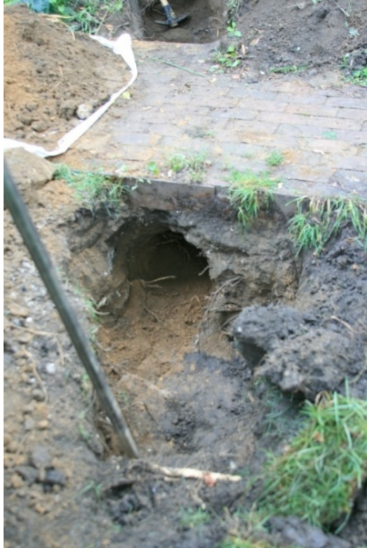
Figure 08: Tunneling underneath the brick path
