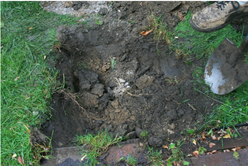
Figure 18: Area A – excavation for the new utility line
