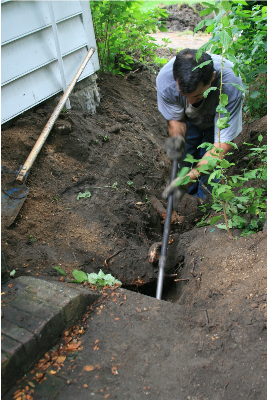
Figure 21: Area A – excavating underneath the brick pathway
