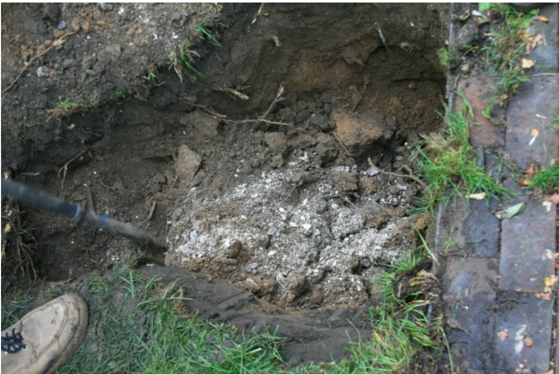
Figure 10: Catch basin excavation showing the ash lens
