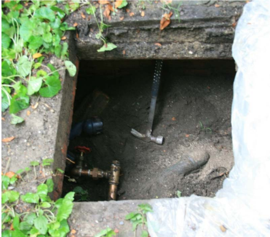
Figure 07: Water connection – concrete junction box
