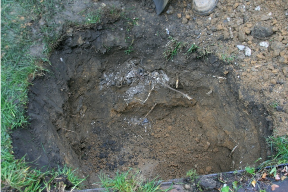
Figure 09: Catch basin excavation
