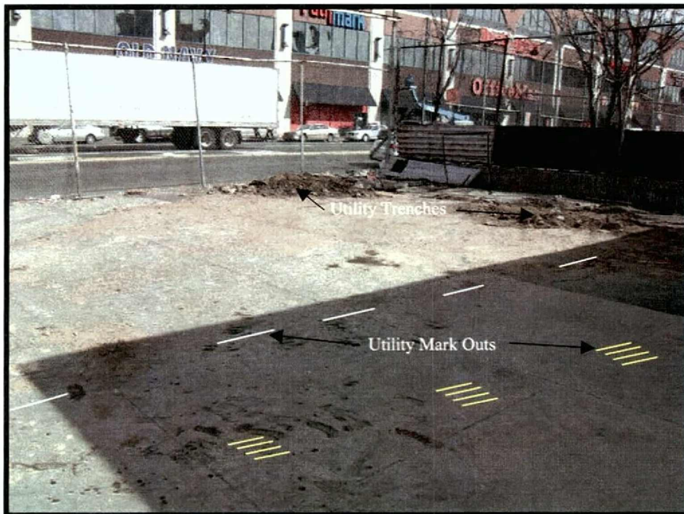
Photograph 4.7 Block 1119, Lot 1, Area A, view looking northeast. Note previous excavations to locate utility lines and white and yellow mark outs locating additional utilities.
