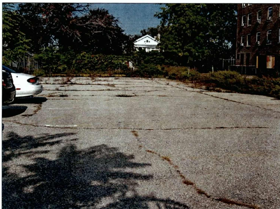
Cracked pavement in parking lot to the west of the Chait Building, looking north
