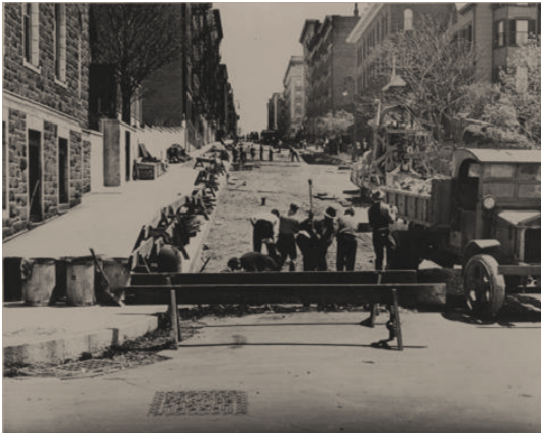
Image 08: WPA photo, circa 1936. Image taken from Riverside Drive facing east.
