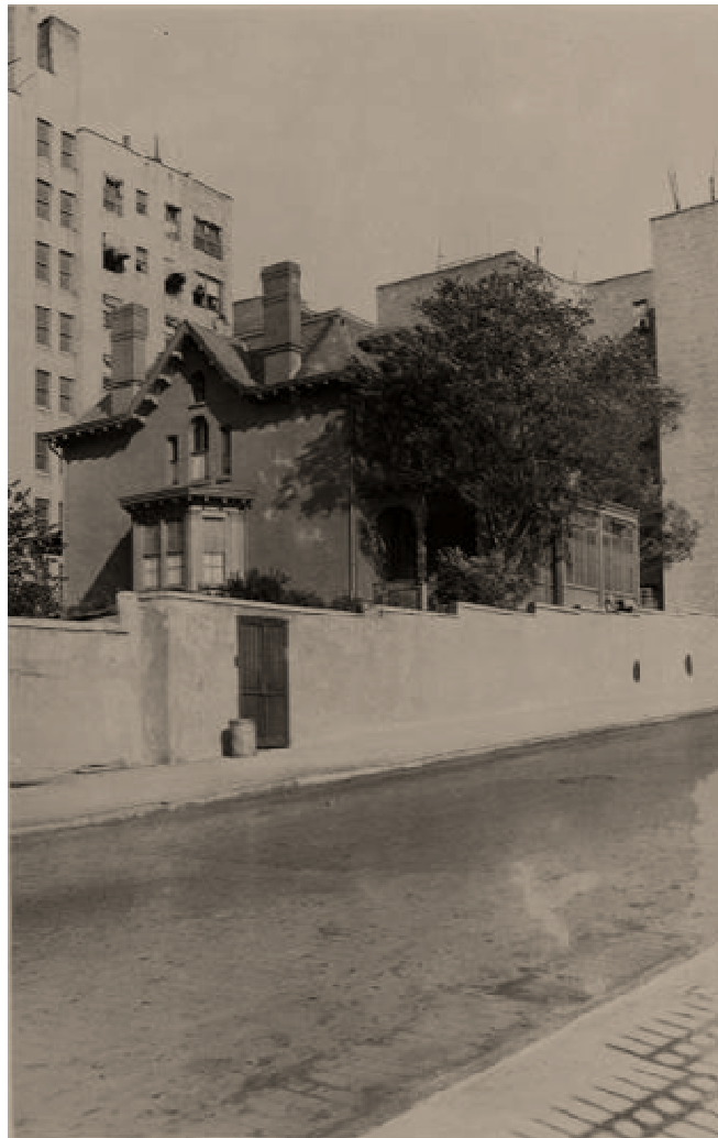
Image 07: 625-627 West 140 th Street September 1931 – depicting the Convent. Image taken facing northeast
