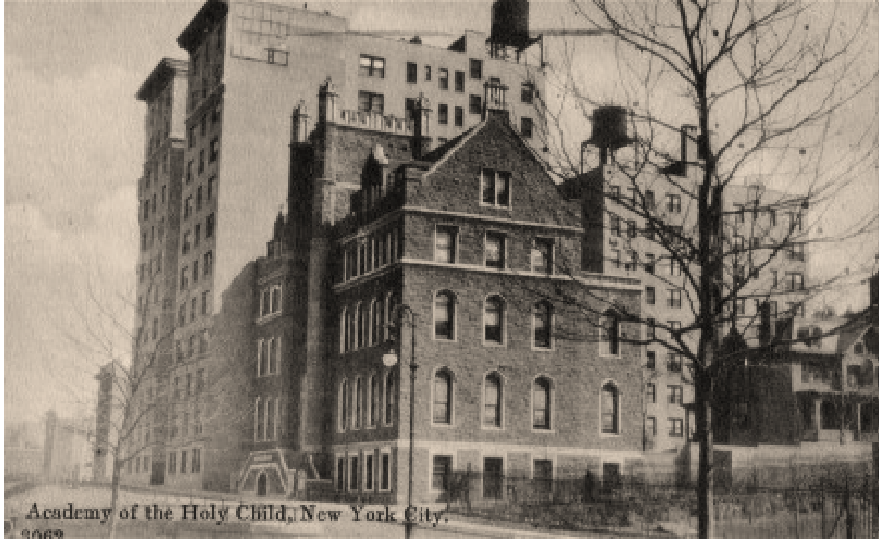
Image 06: A postcard image of St. Walburga's sent by a student to her family. Note the building in the right hand corner of the postcard – the Sister's Convent within the proposed project area. Image taken facing northeast.
