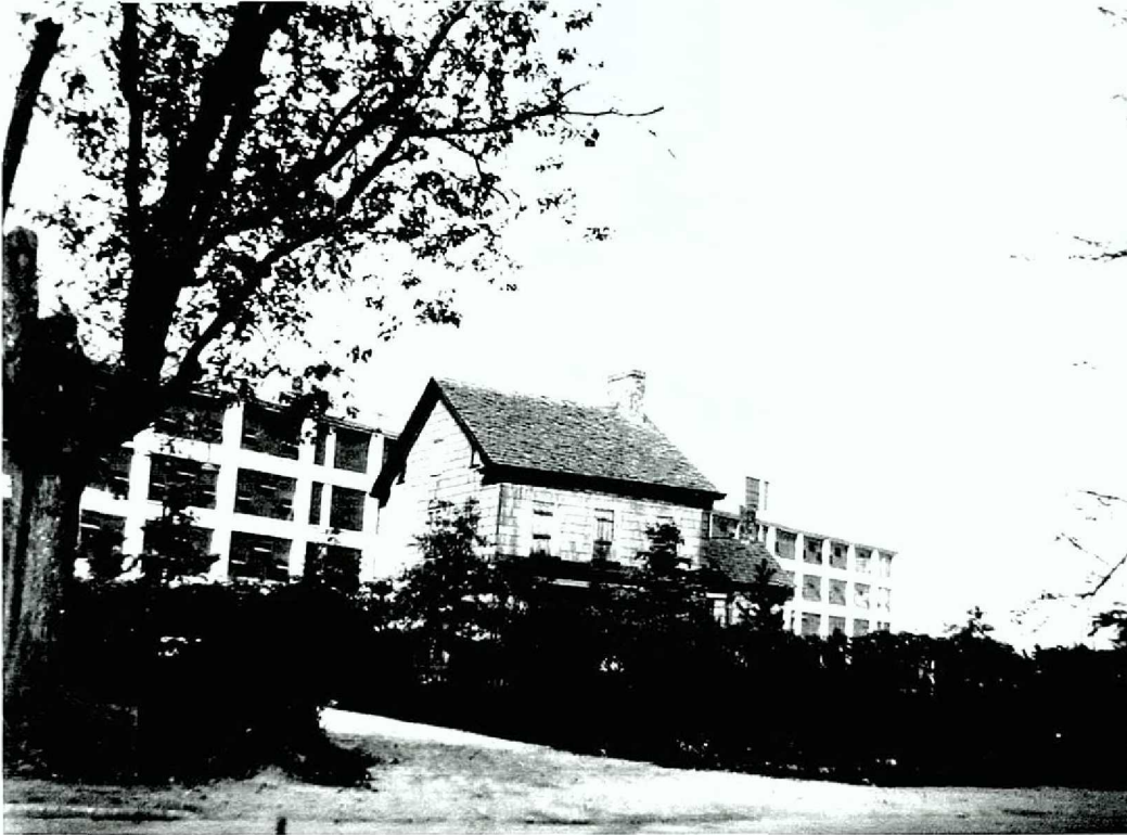
Photograph 17: Eugene L. Armbruster Photograph EA-QC-NT-318 (1922). Ludlow House (note driveway on left). View looking northeast from Corona Avenue.
