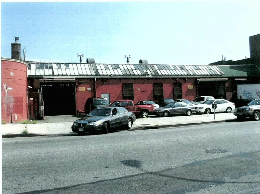
Photograph 4: Project site showing main warehouse building on Lot 86. View looking north from south side of Corona Avenue.
