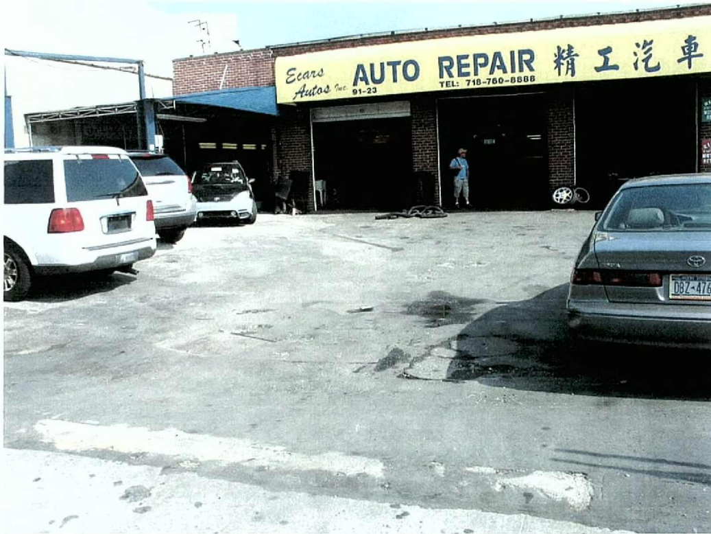
Photograph 11: Project site showing entrance to automobile repair shop building on Lot 110. View looking northwest from sidewalk along Corona Avenue.
