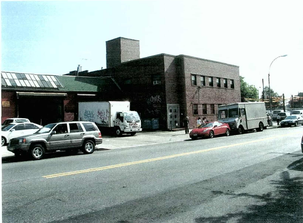
Photograph 8: Project site showing two-story factory building on eastern side of Lot 86. View looking northeast from south side of Corona Avenue.
