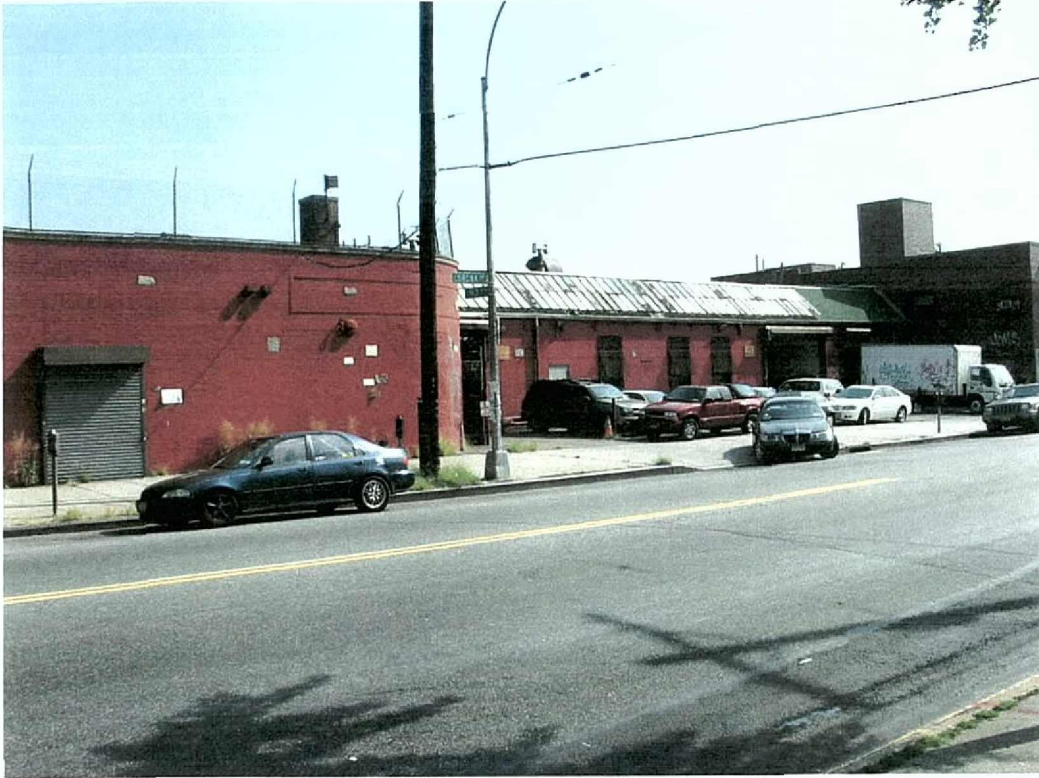
Photograph 3: Project site showing buildings on Lot 86 along north side of Corona Avenue. View looking northeast from south side of Corona Avenue.
