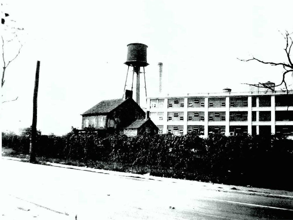
Photograph 18: Eugene L. Armbruster Photograph EA-QC-NT-321 (1922). Ludlow House. View looking northwest from Corona Avenue.
