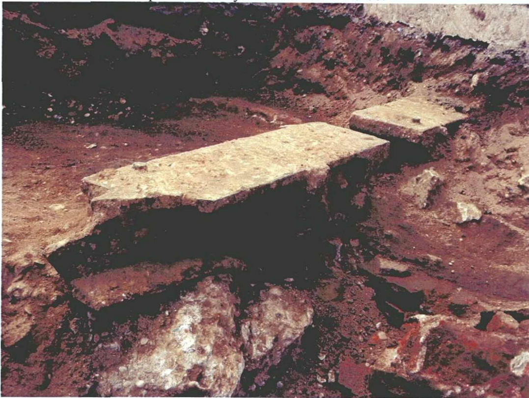
Photograph 14 - Side view close up of possible trolley line rail mount with gap for cable. Facing southwest, photo taken by Michael Audin 4-8-08.
