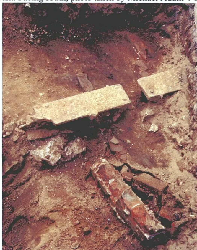
Photograph 12 - Overview of possible trolley line rail mount and brick lining for cable (oriented NW to SE). Facing south, photo taken by Michael Audin 4-8-08.
