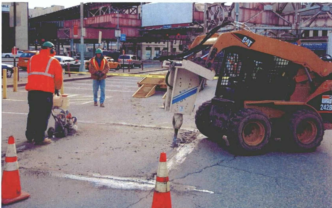
Photograph 2 - Equipment used for the test pit excavation. Facing east, photograph taken by Travis Andrews 4-8-08.
