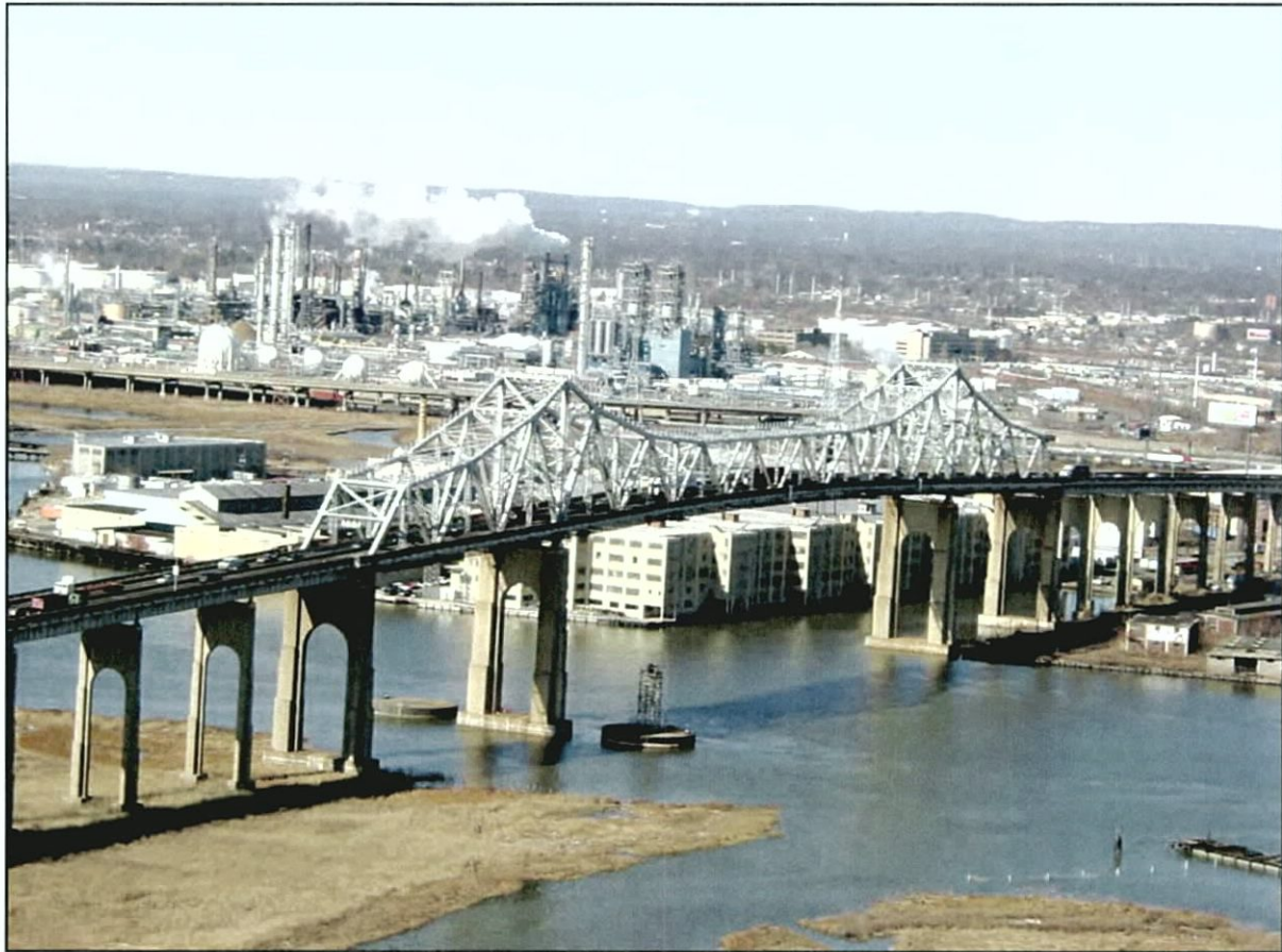
PHOTO 1: Aerial View of the Goethals Bridge Looking Southwest toward Elizabeth-Linden
