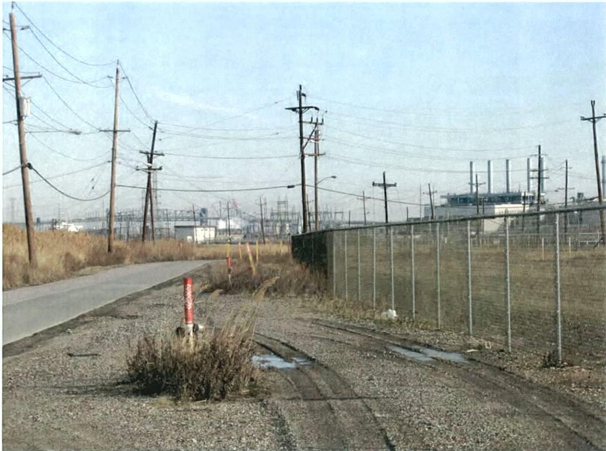
PHOTO 9: View North from Grasselli Road toward Linden Generating Station
