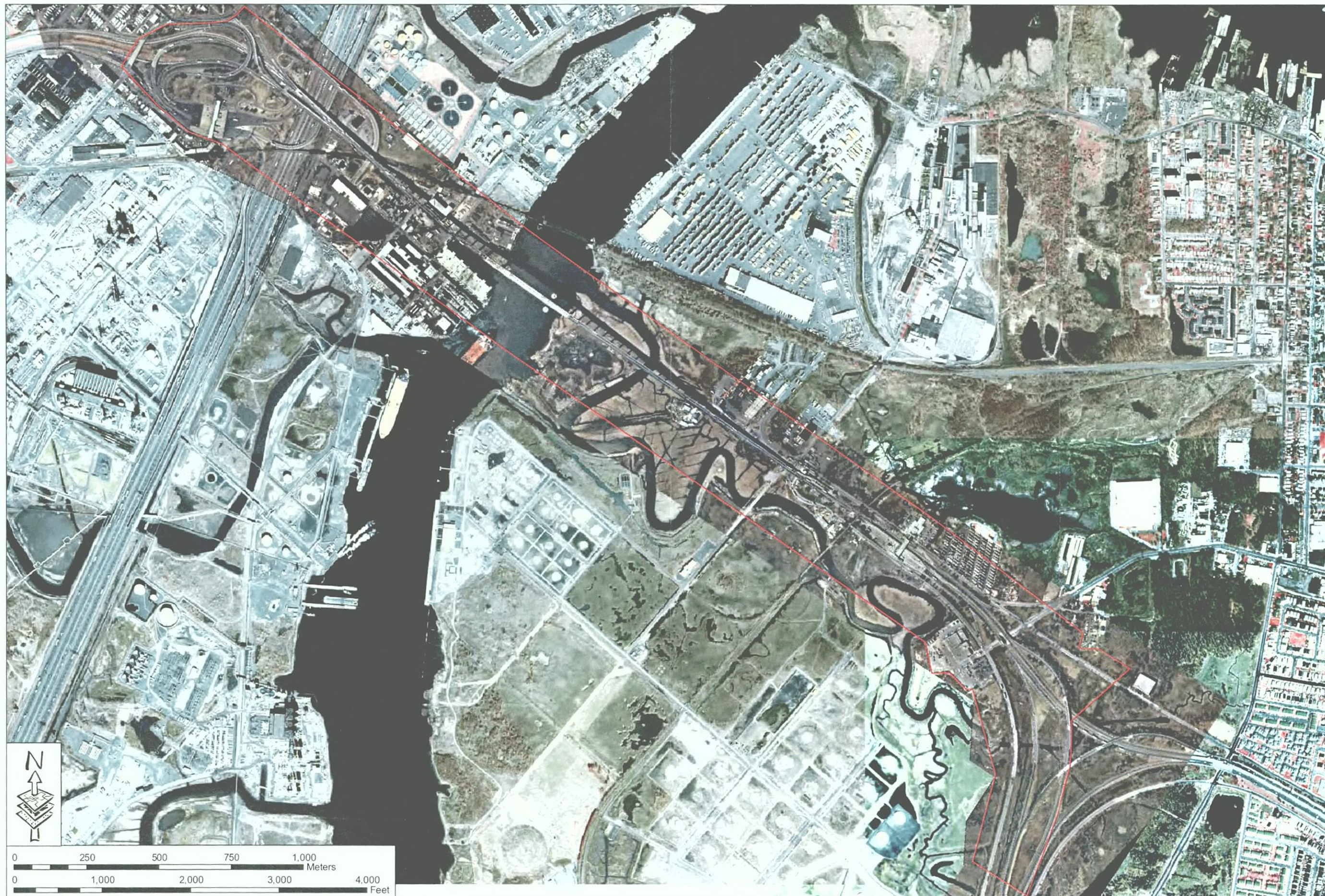
FIGURE 1: Aerial View of the Study Corridor
