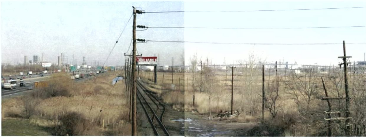
Photo 8: Panoramic View North of the NJ Turnpike and waterfront from Tremley Point Bridge
