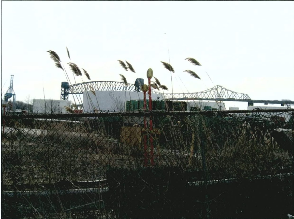
PHOTO 2: View Southeast from the Elizabeth River toward the Goethals Bridge and Arthur Kill Lift Bridge
