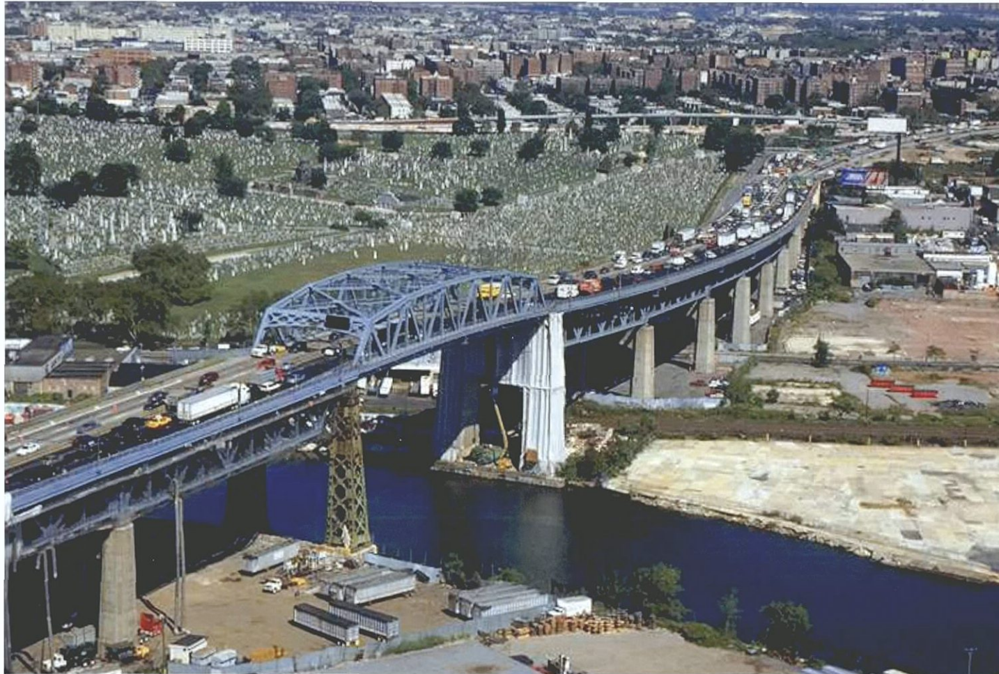
Figure IV-5: View of Main Span, Kosciuszko Bridge and Queens Approach, looking north (Calvary Cemetery and Sunnyside, Queens in background)
