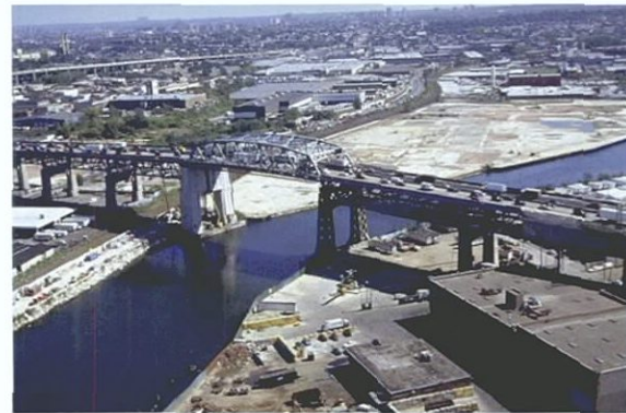
FIGURE 4: AERIAL VIEW OF THE MAIN SPAN ABOVE NEWTOWN CREEK LOOKING EAST
