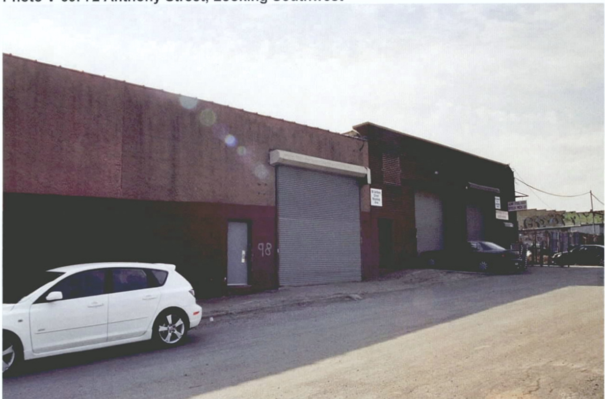
Photo V-60. 96-102 Anthony Street, Looking Southwest
