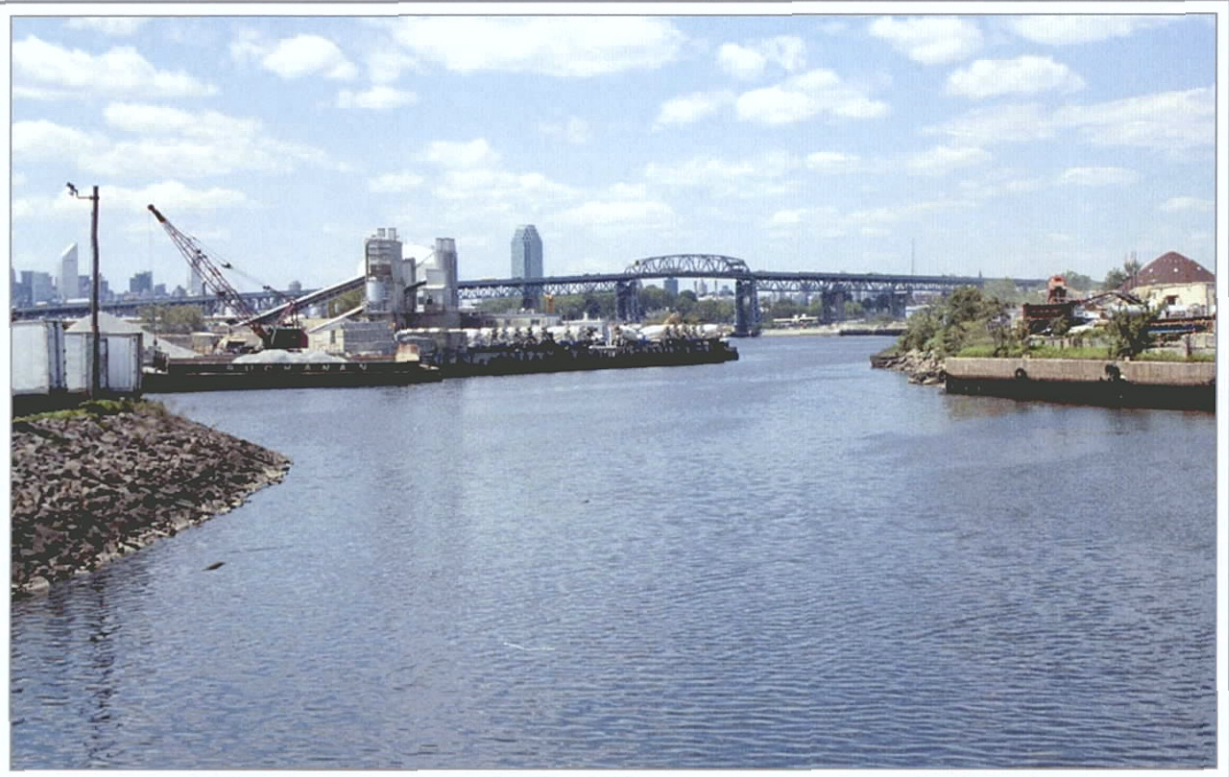
Photo V-15. Kosciuszko Bridge, looking northwest from Grand Street Bridge
