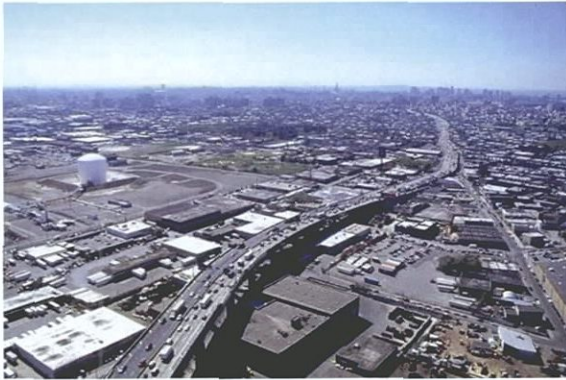
FIGURE 1: AERIAL VIEW OF THE BROOKLYN APPROACH LOOKING SOUTHWEST
