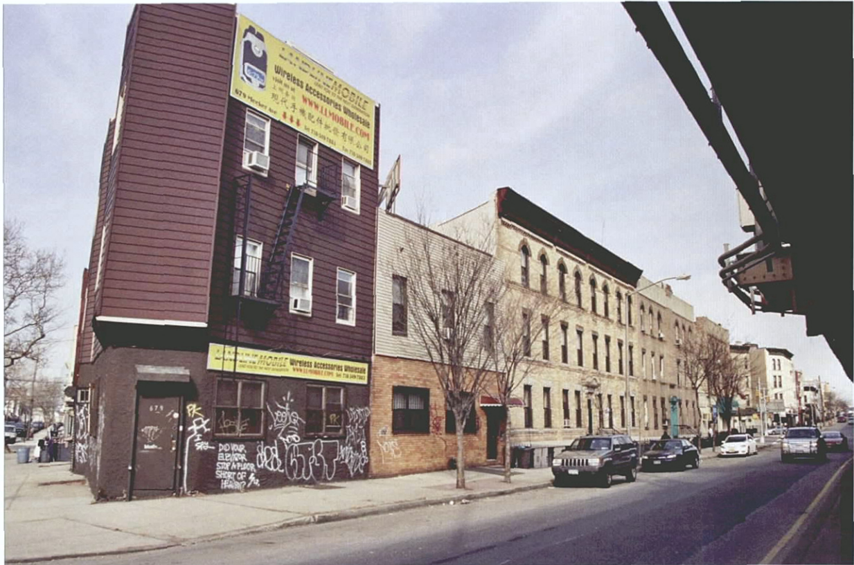
Photo V-28. 679, 685, 687, and 695 Meeker Avenue, Looking Northeast
