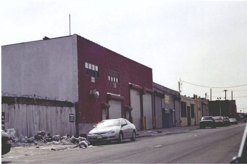
Photo V-38. 958-972 Meeker Avenue, Looking Southwest
