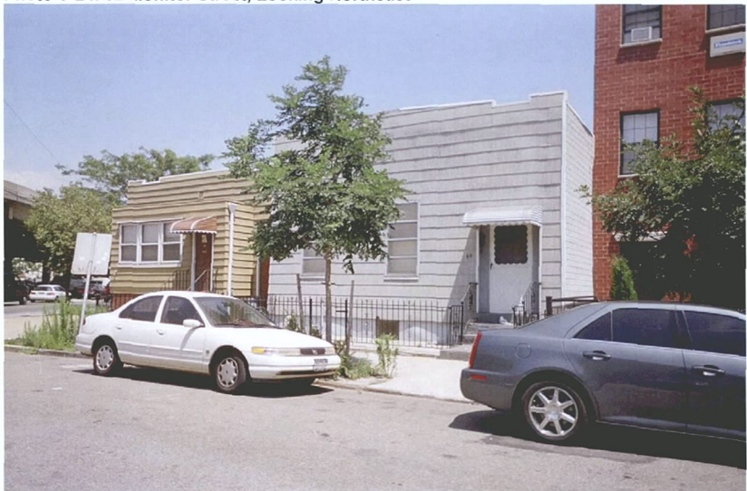
Photo V-25. 60 Monitor Street, Looking Northeast
