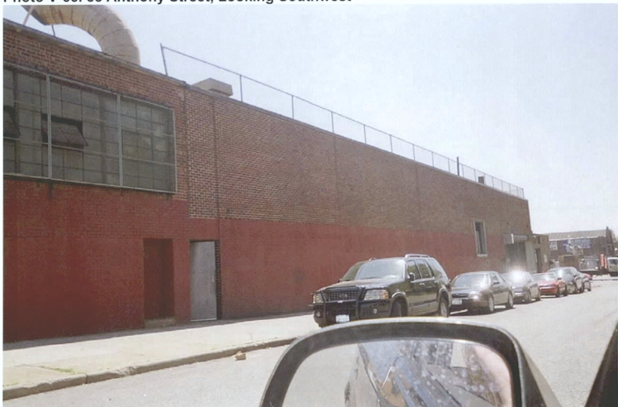
Photo V-56. 46-52 Anthony Street, Looking Southwest
