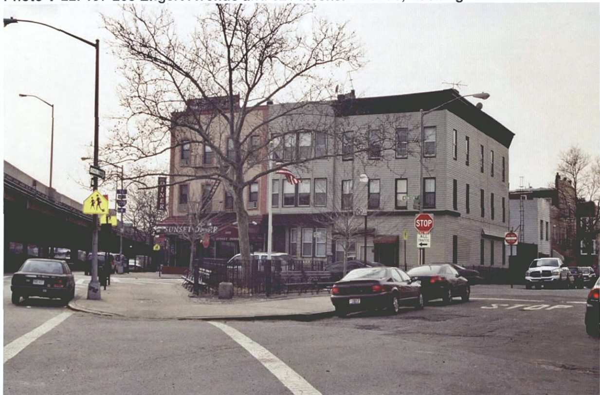
Photo V-23. 71-75 Monitor Street, Looking West
