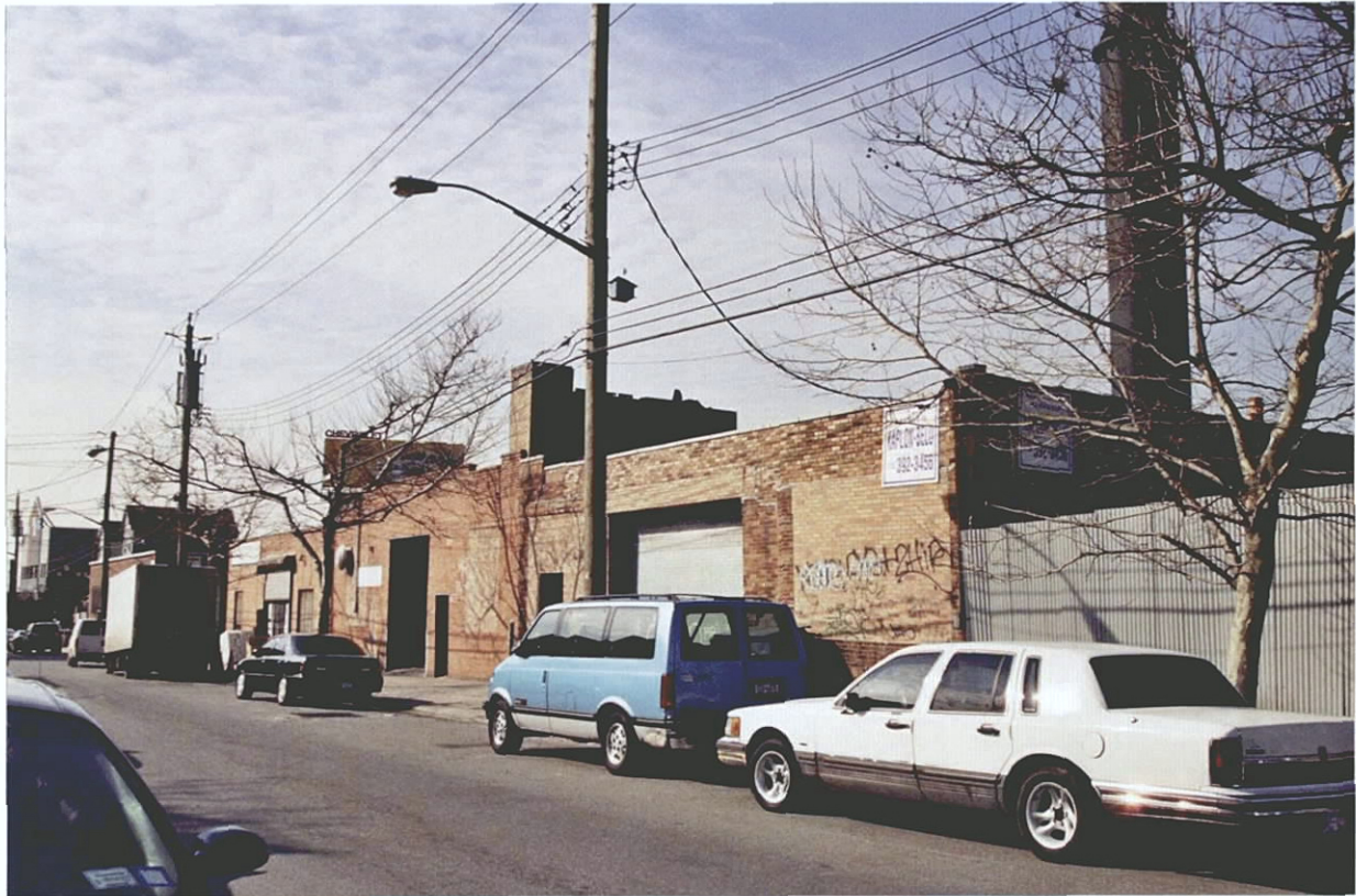
Photo V-95. 54-08, 54-14 and 54-18 43rd Street, Looking Southwest
