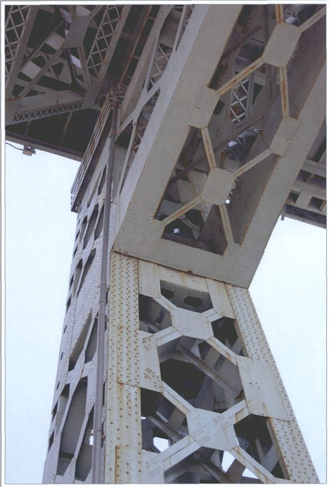
Photo 9: Detail of truss connection beneath Kosciuszko Bridge
