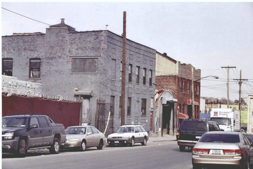
Photo V-34. 843-845, 855, and 857-869 Meeker Avenue, Looking Northeast
