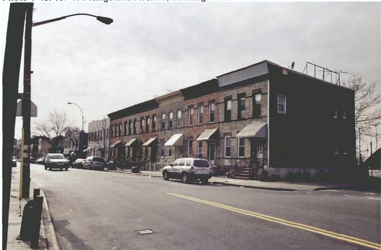
Photo V-46. 145-151 Kingsland Avenue, Looking South
