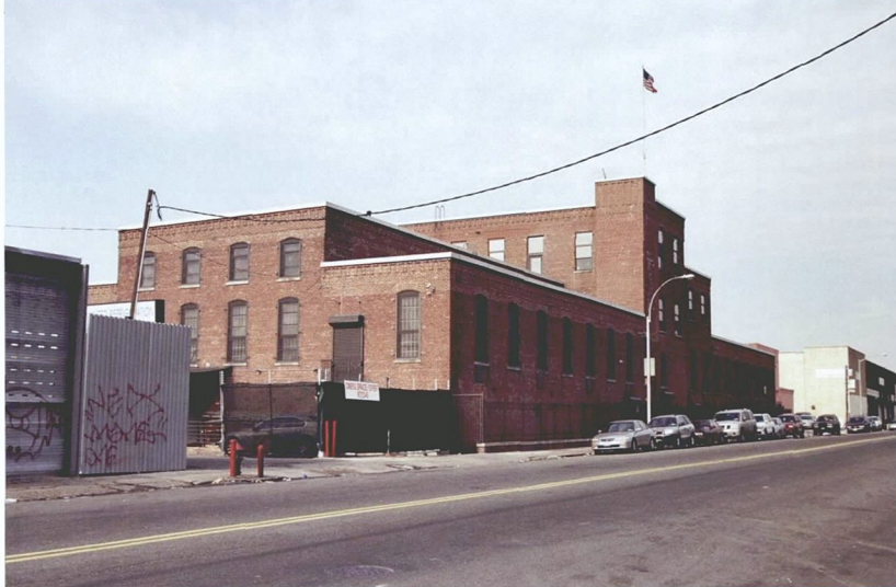
Photo V-82. 36-60 Review Avenue, Looking Northwest
