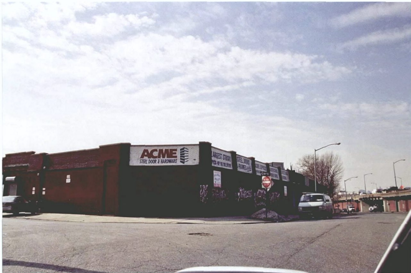
Photo V-65. 503-513 Porter Avenue, Looking Southwest Along Cherry Street
