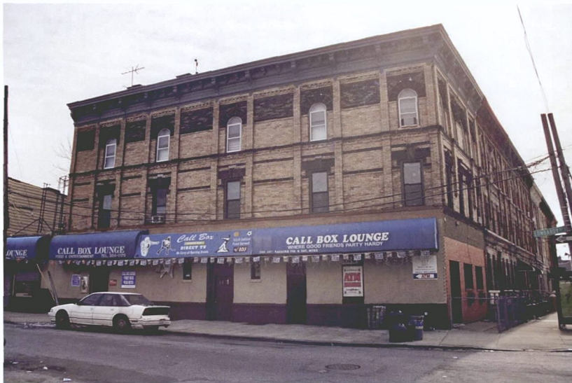
Photo V-47. 148 Kingsland Avenue, Looking South
