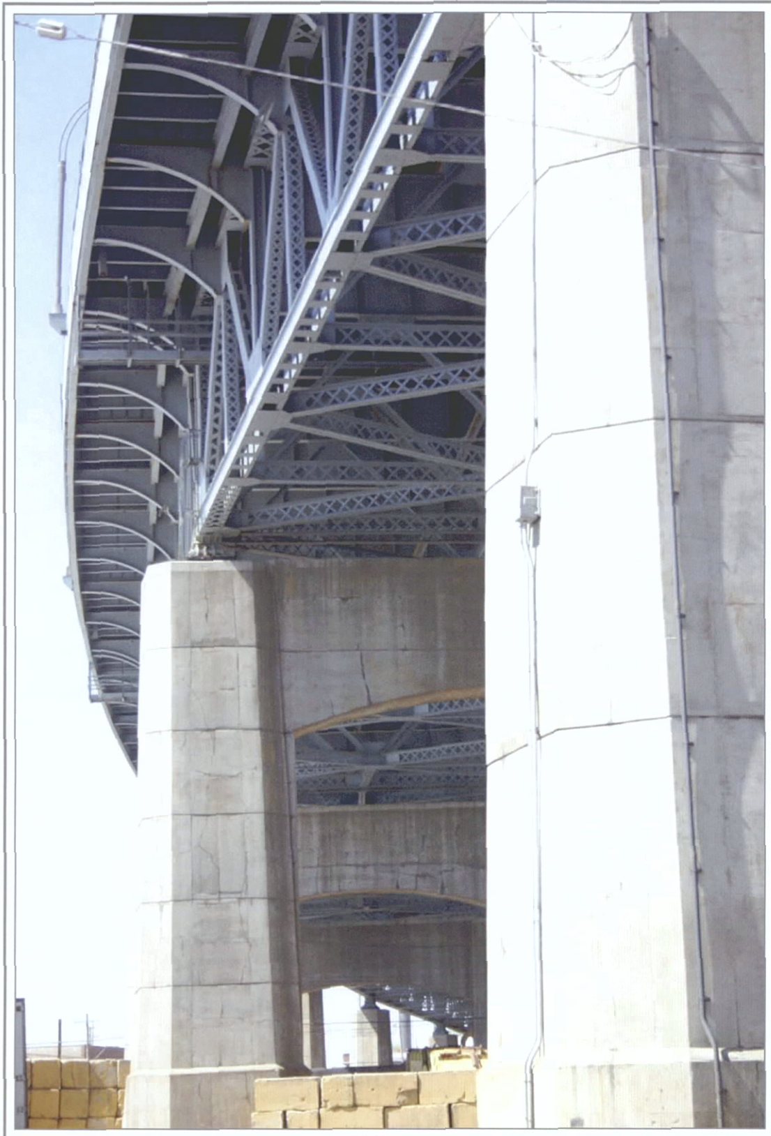
Photo V-17. Detail of concrete piers and substructure, looking southwest from Greenpoint, Brooklyn, New York
