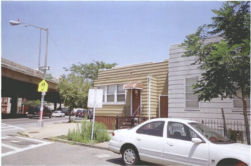
Photo V-24. 62 Monitor Street, Looking Northeast
