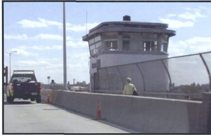
Image 16: Pulaski Bridge, Greenpoint, Brooklyn, New York Image Courtesy of EHT Tracerics, May 2006
