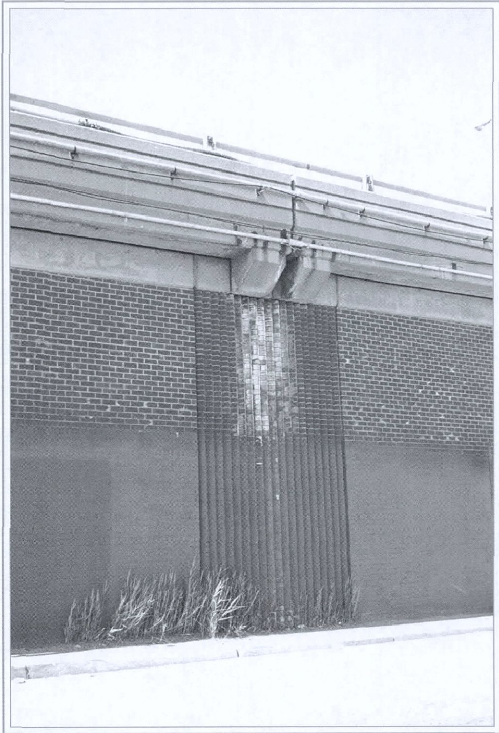
Photo 10: Detail of sawtooth brick elements on exterior of bridge abutments, on the Brooklyn side
