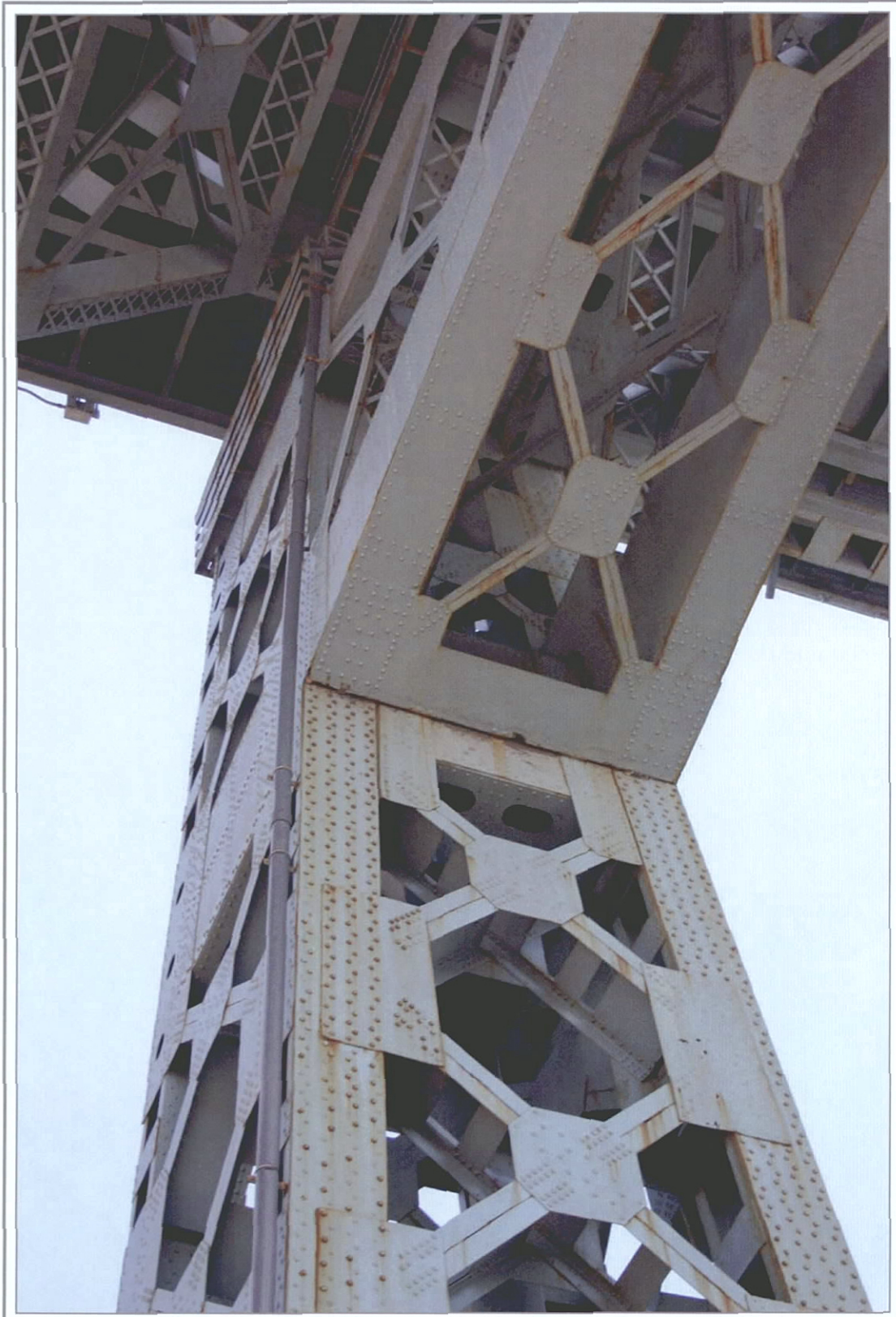
Photo V-20. Detail of truss connection beneath Kosciuszko Bridge
