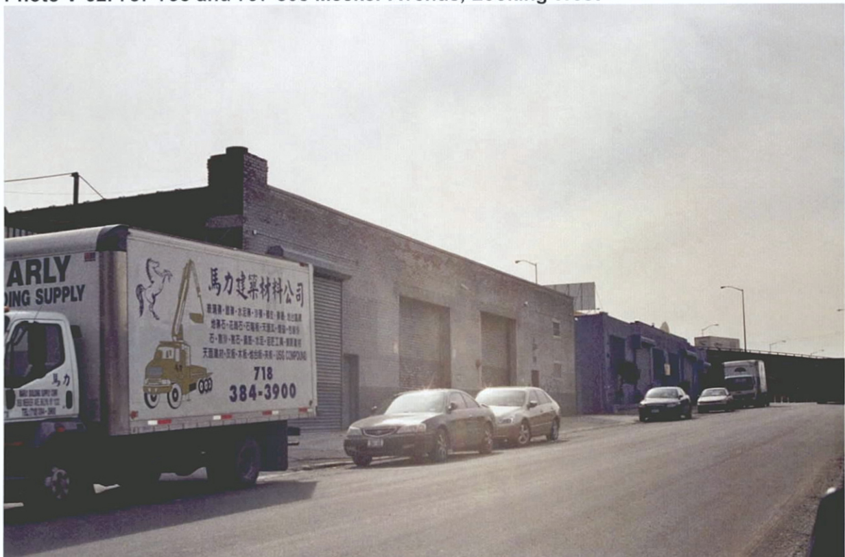
Photo V-33. 810-822 Meeker Avenue, Looking Southwest
