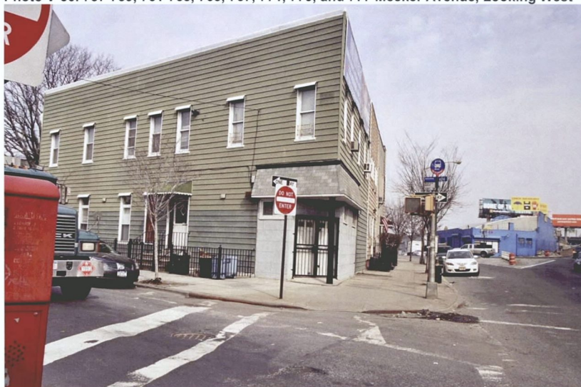
Photo V-31. 779 Meeker Avenue, Looking Northeast
