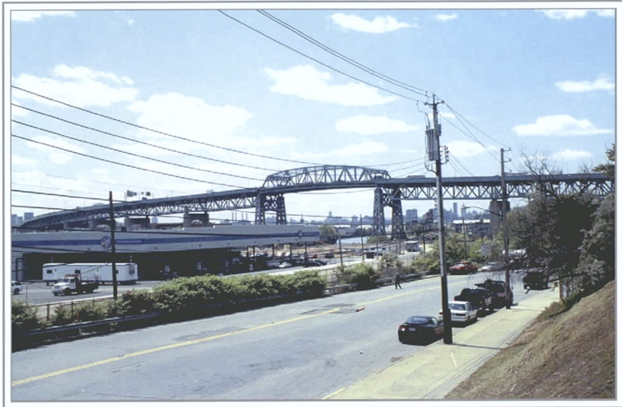
Kosciuszko Bridge, looking west from 56 th Road, Queens, New York
