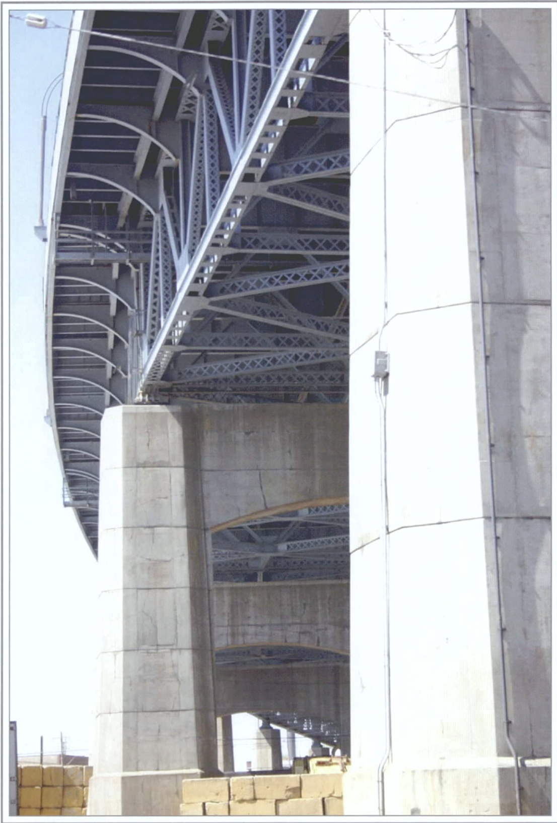
Detail of concrete piers and substructure, looking northeast from Greenpoint, Brooklyn, New York
