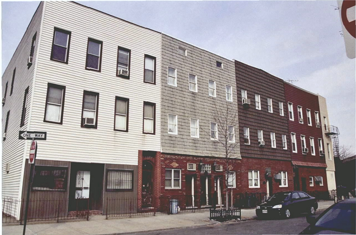
Photo V-22. 197-203 Engert Avenue and 621 Meeker Avenue, Looking North
