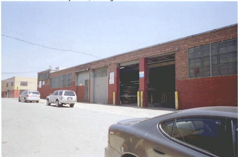
Photo V-58. 54-70 Anthony Street, Looking Southwest
