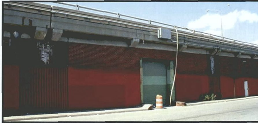
Image 3: Detail of bridge abutments and storage spaces, Image courtesy of EHT Tracerics, May 2006
