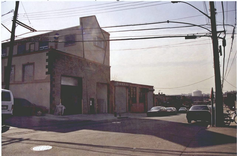
Photo V-90. 55-01 and 55-05 43rd Street, Looking Southeast
