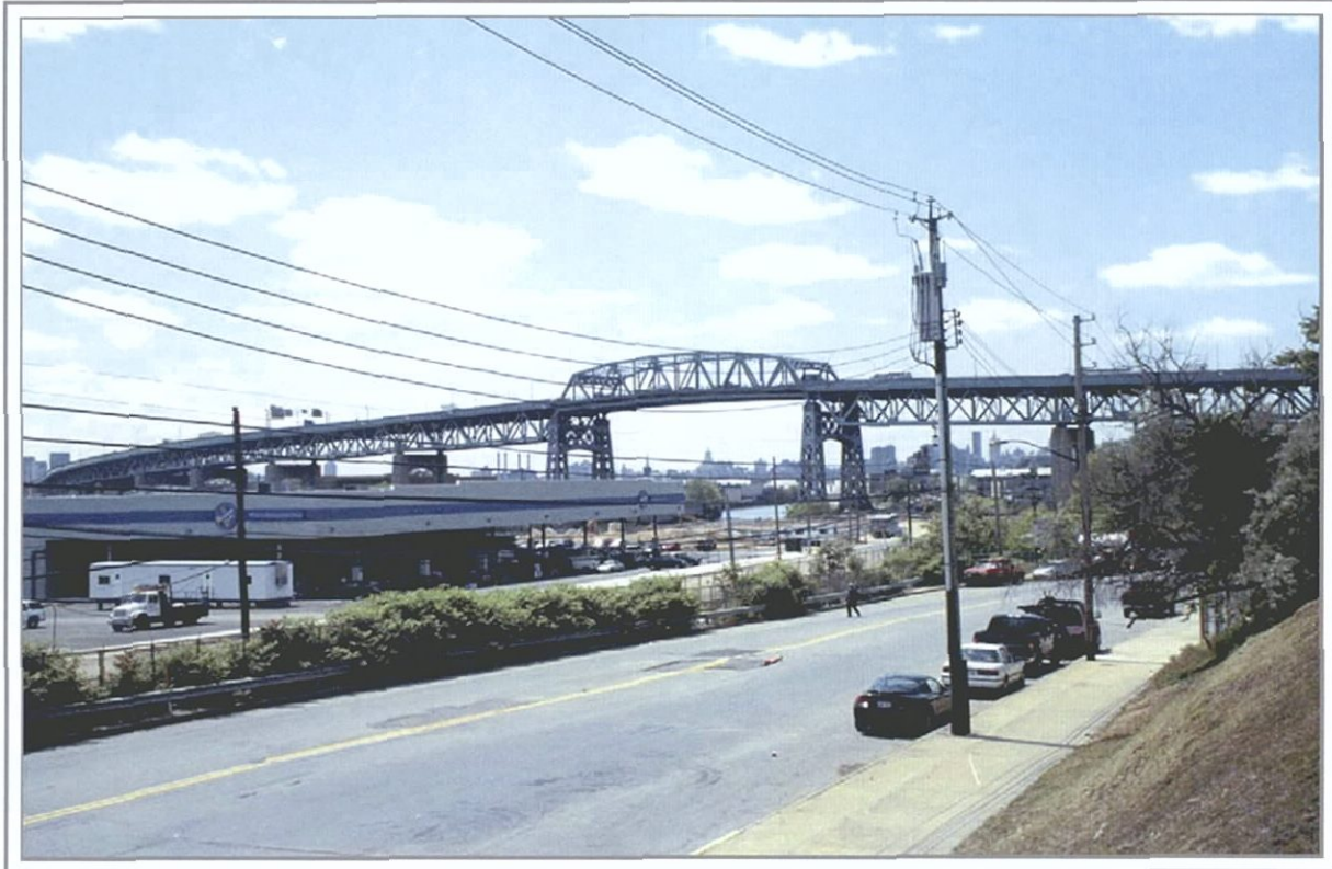
Photo 3: Kosciuszko Bridge, looking west from 56 th Road, Queens, New York
