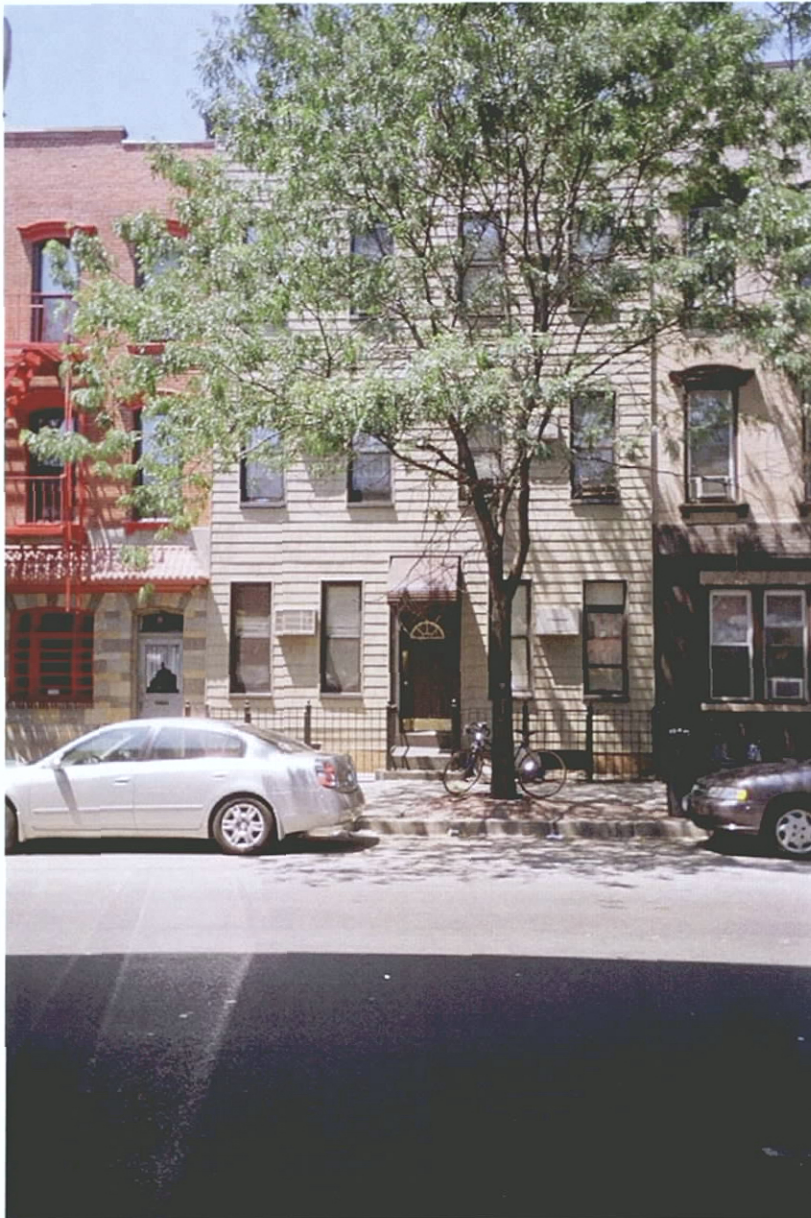
Photo V-26. 583 Meeker Avenue, Looking Northwest
