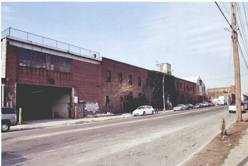
Photo V-81. 38-98 Review Avenue, Looking Southwest
