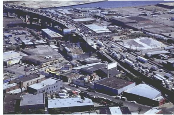
FIGURE 2: AERIAL VIEW OF THE BROOKLYN APPROACH AND WESTBOUND EXIT RAMP
