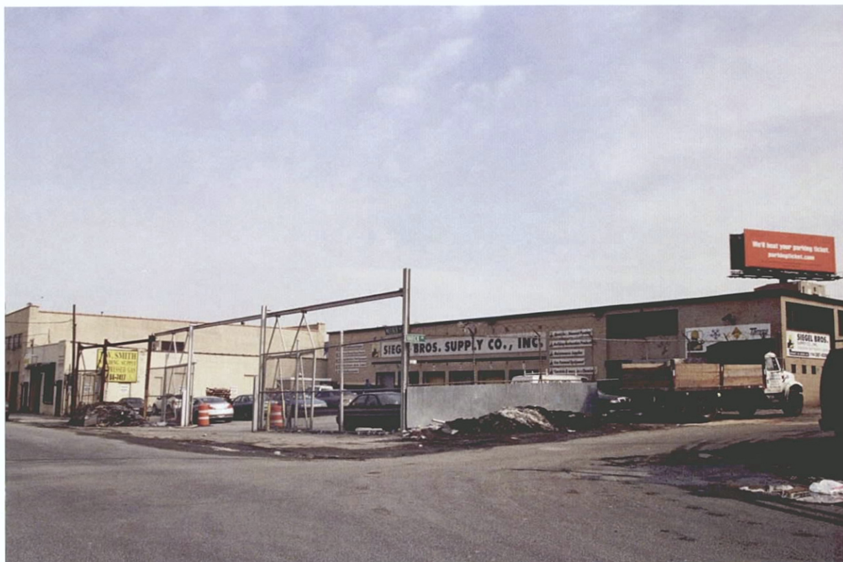
Photo V-36. 890-892 Meeker Avenue, Looking Southeast
