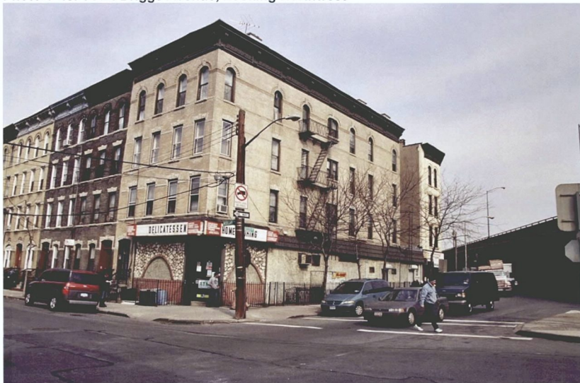
Photo V-44. 4 Driggs Avenue, Looking Northeast
