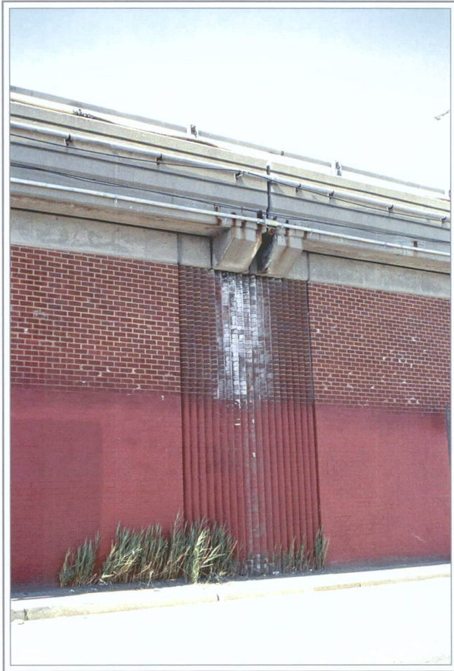
Detail of sawtooth brick elements on exterior of bridge abutments, on the Brooklyn side
