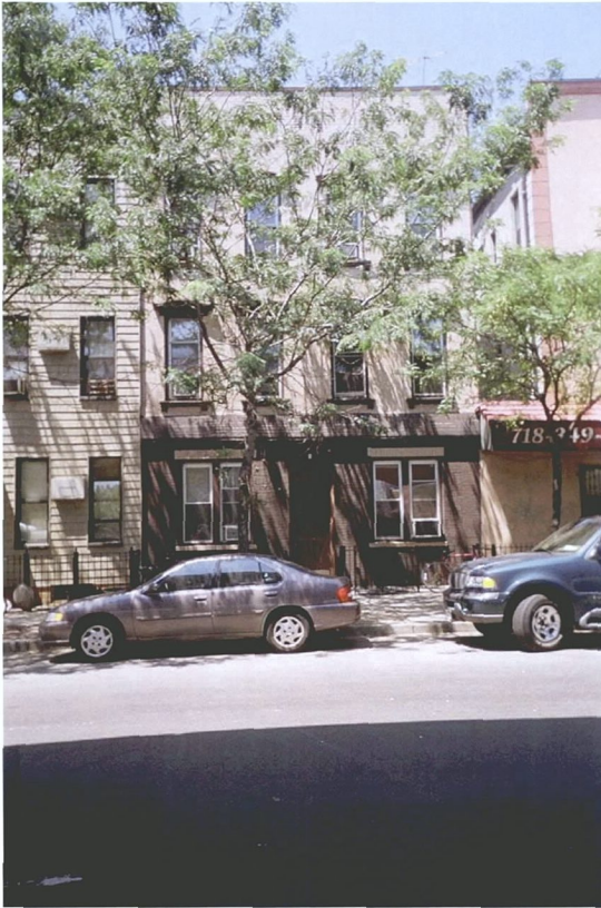
Photo V-27. 585 Meeker Avenue, Looking Northwest
