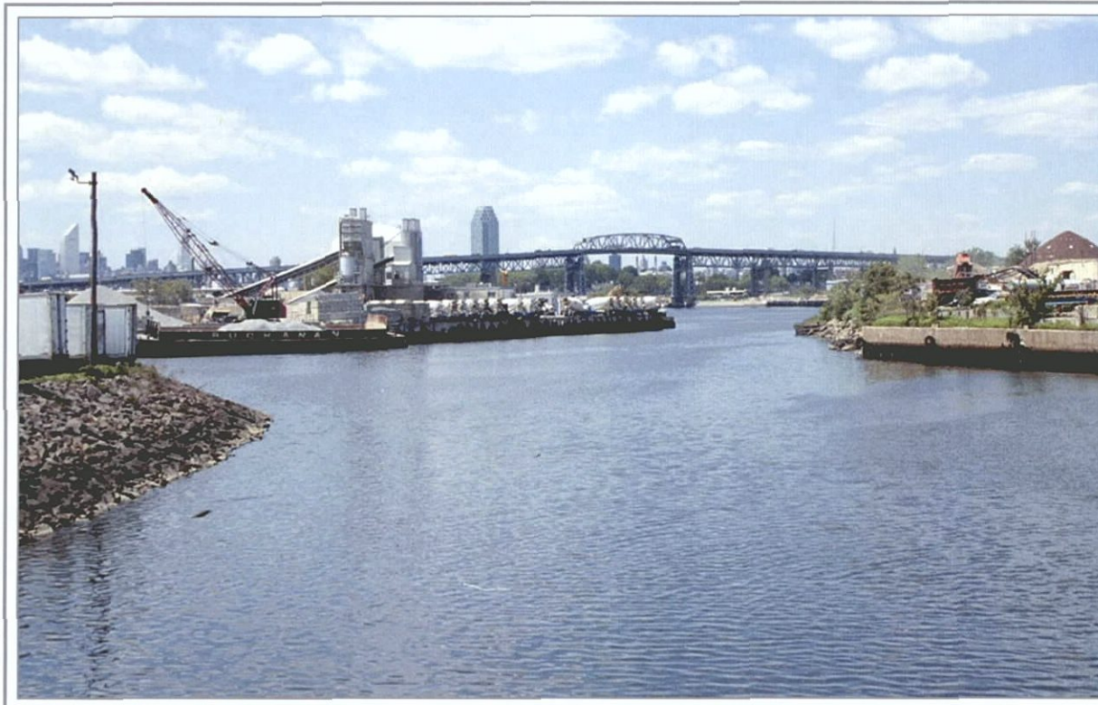
Photo 4: Kosciuszko Bridge, looking northwest from Grand Street Bridge
