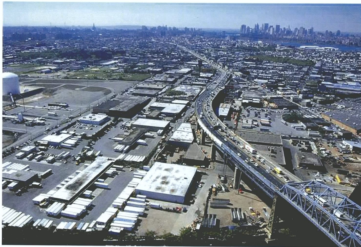
Figure IV-4: View of the Brooklyn Approach and the BQE, looking Southwest (Downtown Brooklyn and Lower Mahattan in background)
