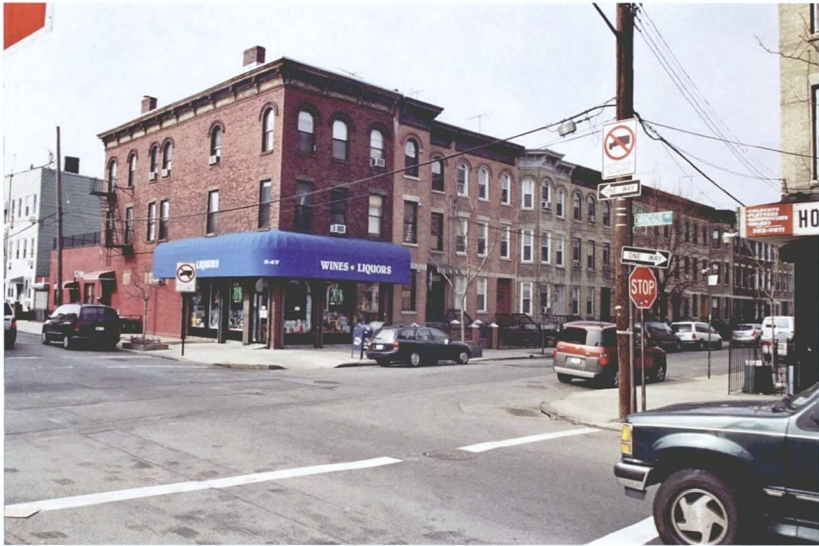
Photo V-43. 14-24 Driggs Avenue, Looking Northwest
