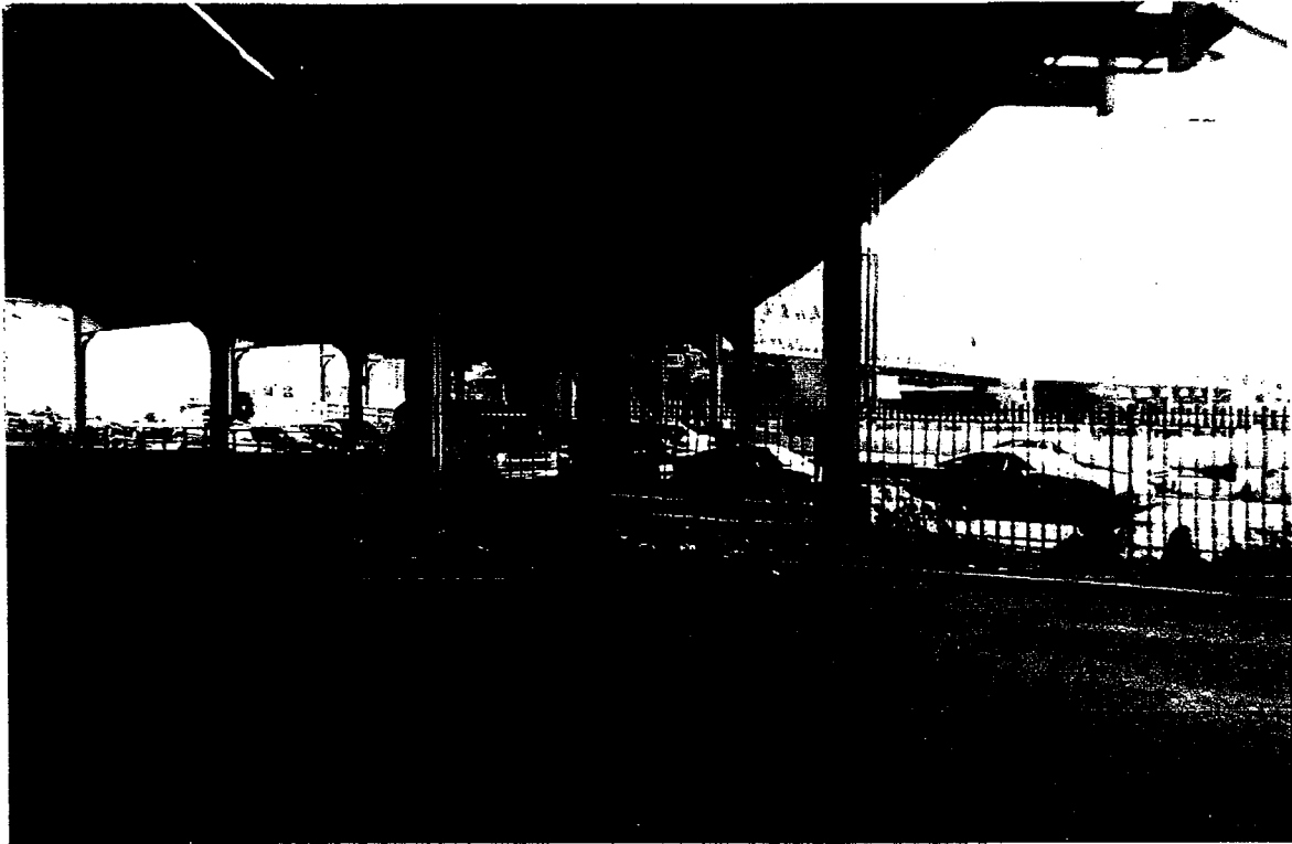
Photograph A. Beneath the Willis Avenue Bridge from First Avenue. (Facing northwest.)
