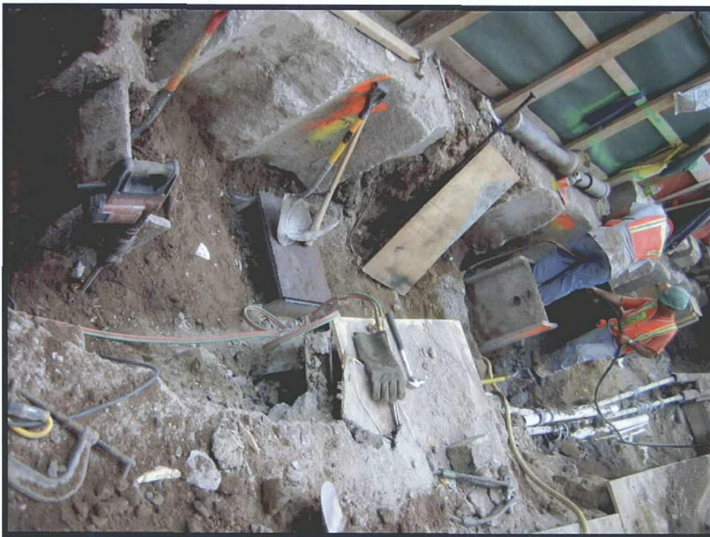
Photograph 5.2 North side of Dey Street, looking northeast.
