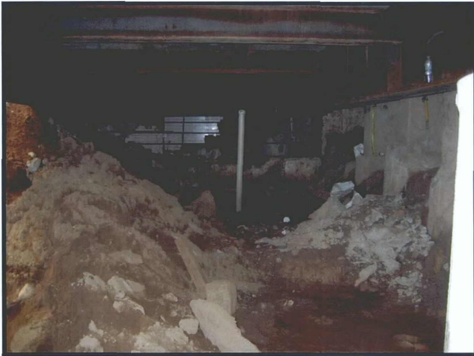
Photograph 5.21 Remnants of a former subway station and deconstructed token booth.
