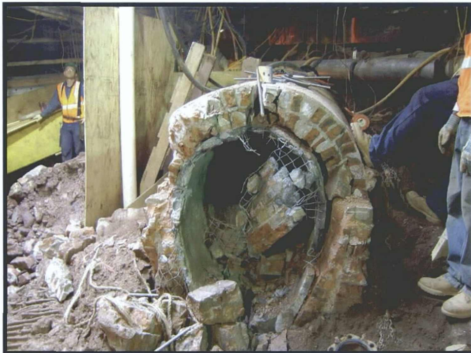
Photograph 5.13 Modern brick sewer line, looking west.
