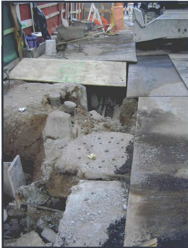
Photograph 5.4 Trench DB-7N, utility access manhole, looking east.
