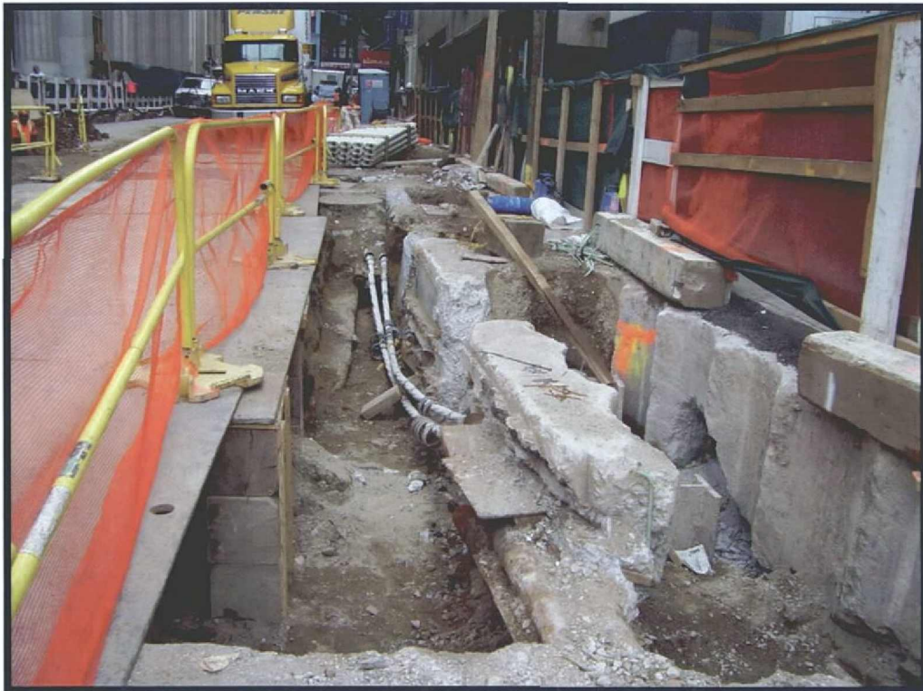
Photograph 5.5 South side of Dey Street, Trenches DB-2S to DB-8S, looking east.
