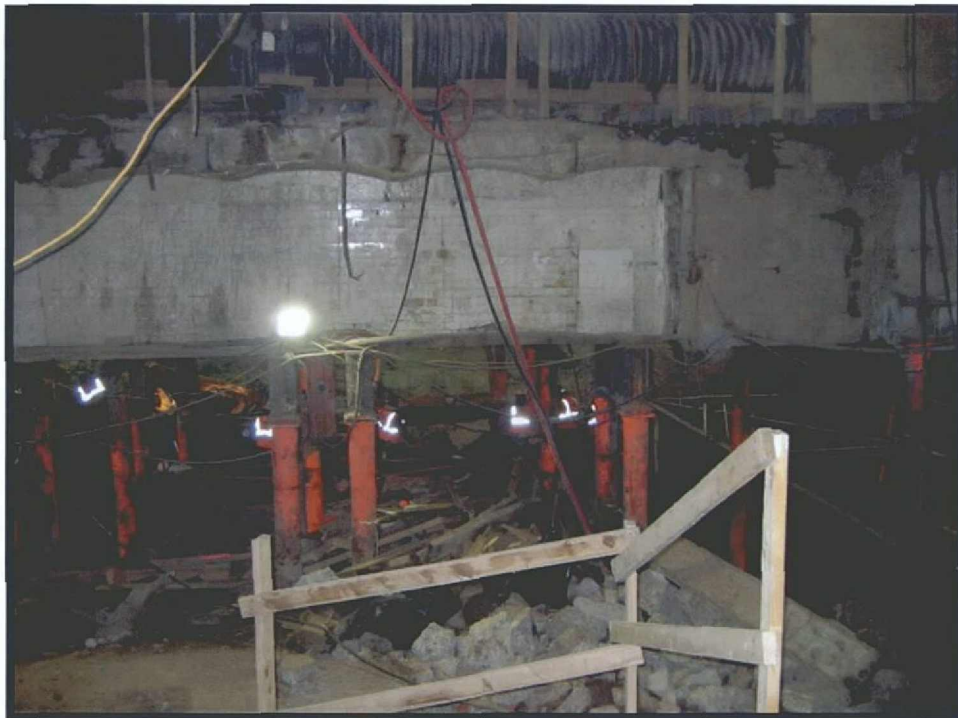
Photograph 5.20 Remnants of a former subway station wall.
