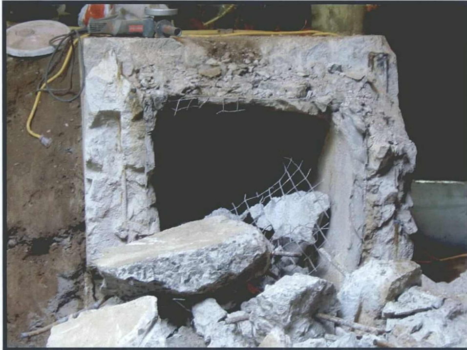
Photograph 5.14 Modern concrete sewer line, looking east.
