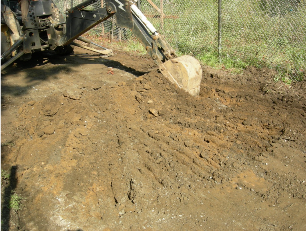
Image 15: Excavation for new path
