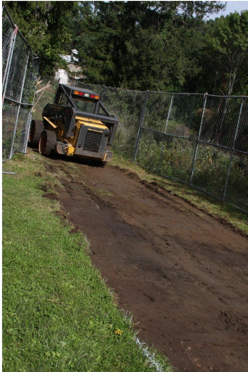
Image 05: Excavation of top soil – looking towards Carriage House
