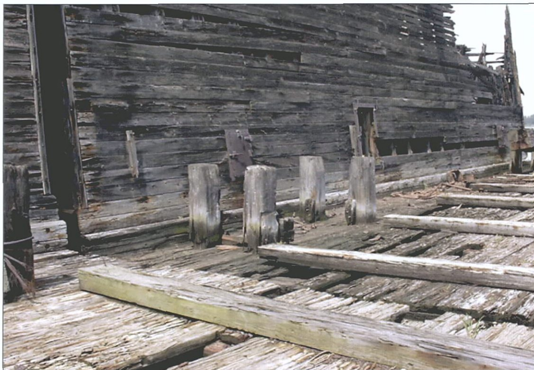
Figure 5-134. Port wing showing hatch locations. View to the northwest (port).
