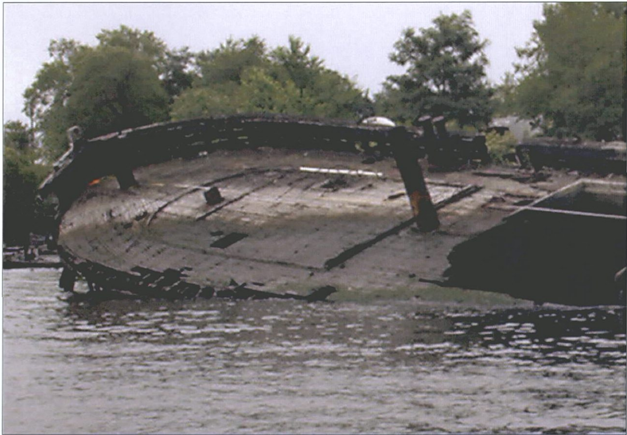
Figure 7-70. Forward third of Fish Hawk , including pilothouse, looking south. Note king plank and sisters along centerline.
