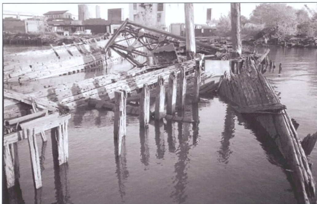
Figure 6-102. Heavily deteriorated bow section. View to the south (forward).
