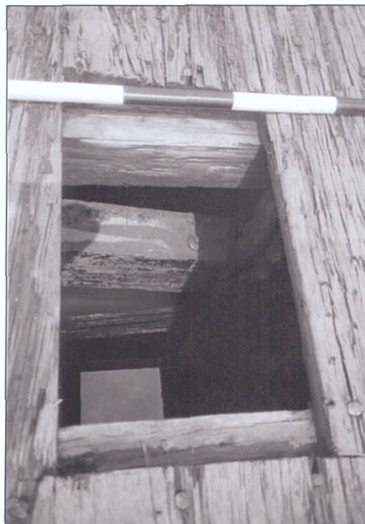
Figure 5-91. Access hatch detail.
