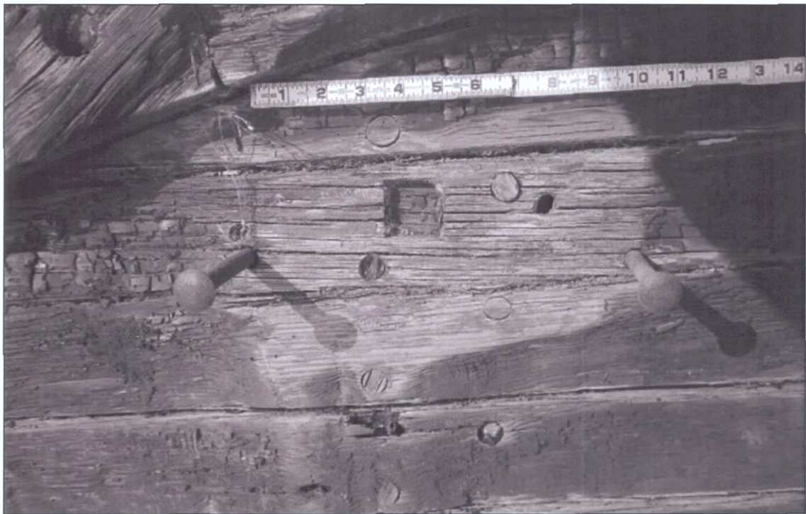
Figure 7-75. Photo of fastener pattern on main deck and quarterdeck planking.
