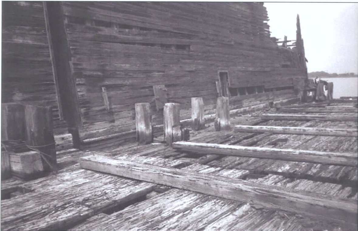
Figure 5-67. Port aft bitt. View to the north.
