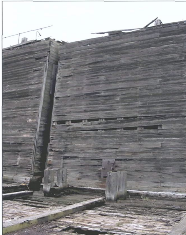
Figure 5-120. Port wing aft. Note chine logs at base and differing size planking, especially larger scantling planks at top. View to the southwest (port).
