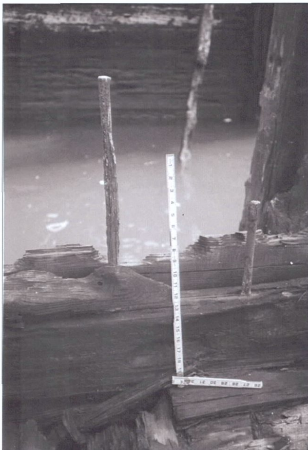
Figure 5-175. One-inch drift pins in outer hull timbers.
