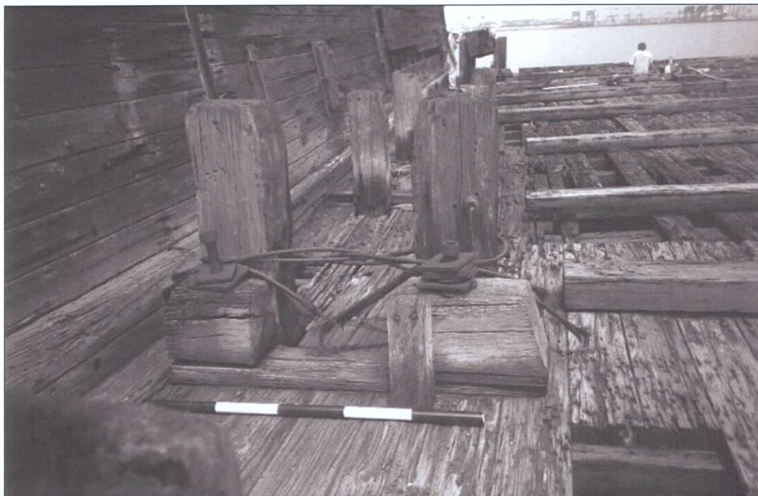
Figure 5-68. Bitt cradle. View to the north (forward).
