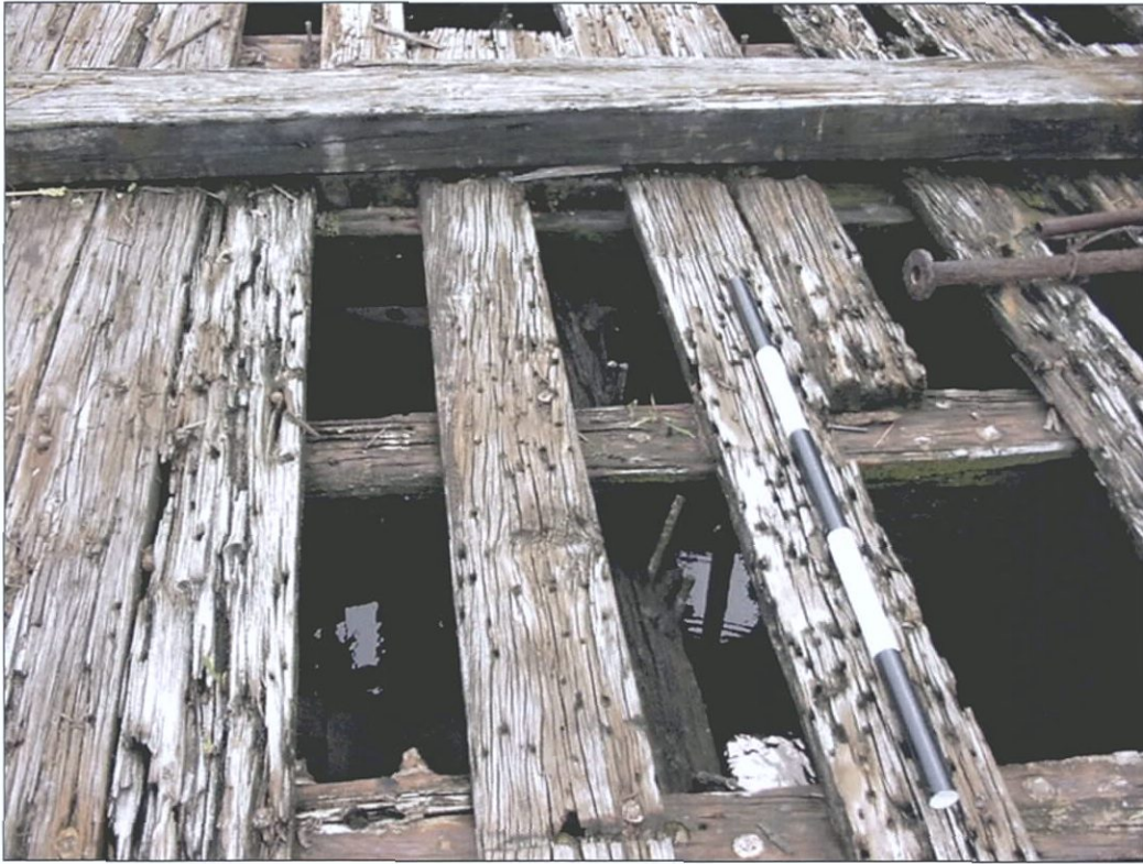
Figure 5-76. Deck plank. Port side, view to the south (aft).
