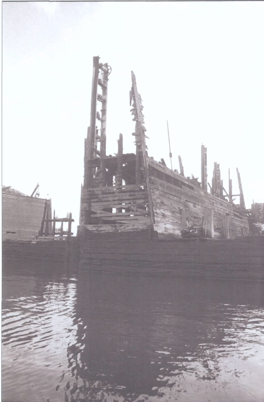
Figure 5-23. Main deck starboard side. View to the south.
