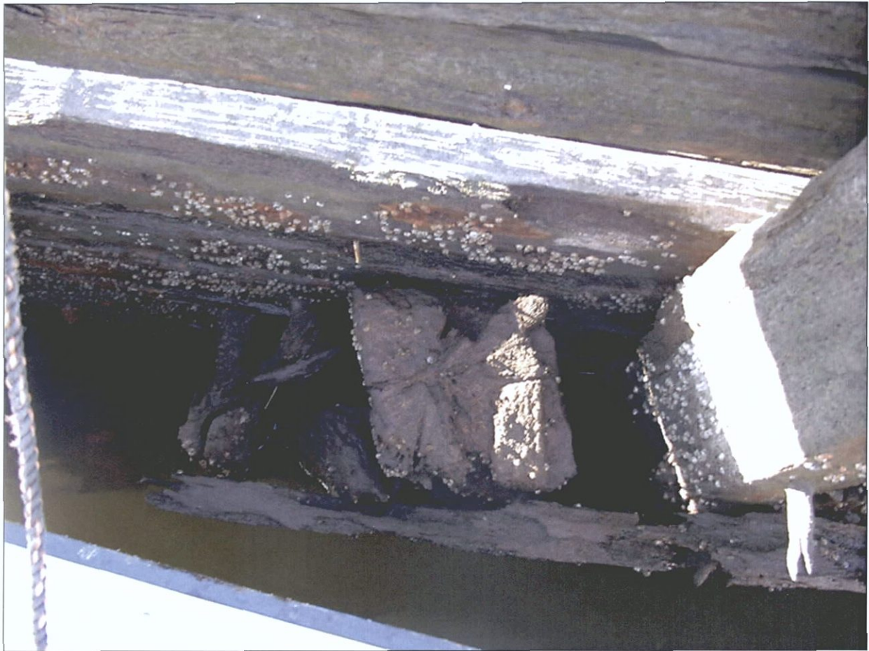
Figure 6-107. Port side forward, cant frame detail.
