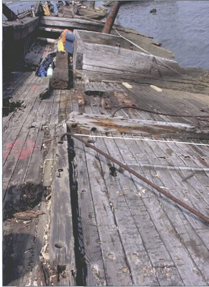
Figure 7-71. View aft (north), showing deck planking.
