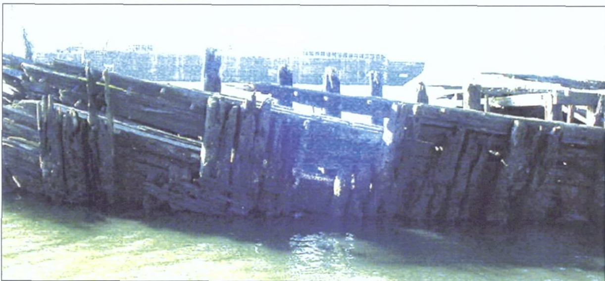
Figure 6-106. Port side, forward, framing (colors exaggerated to enhance definition). View to the southwest.
