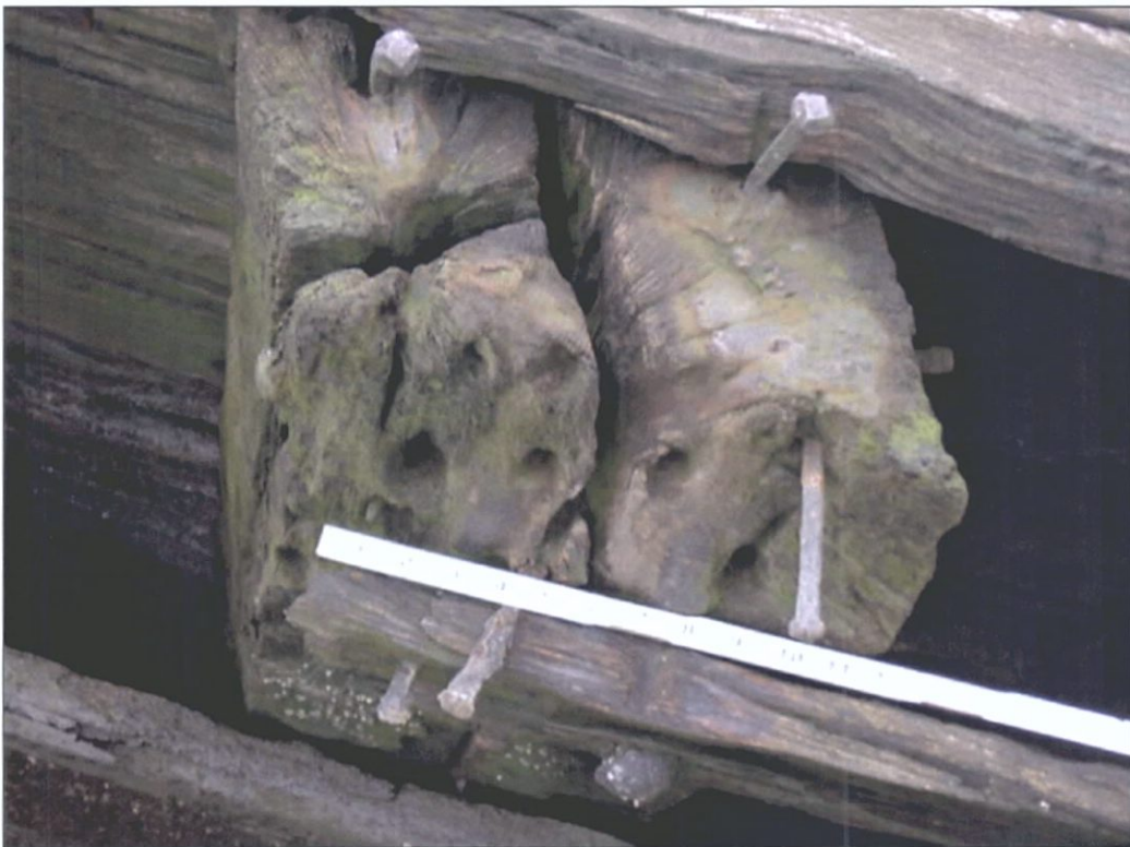
Figure 7-54. Close-up of the fifth canted frame.
