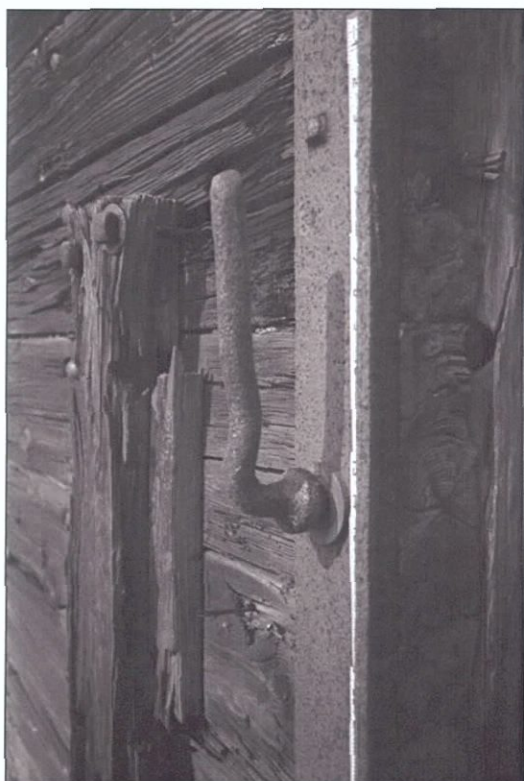
Figure 5-139. Hatch dog detail. Port wing, view to the southwest (aft).
