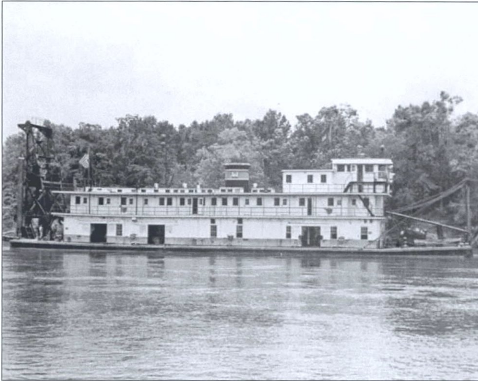
Figure 4-14. Dredge William T. Guthrie at work on the Apalachicola River, circa 1900 (photo courtesy of the Florida Photographic Collection).
