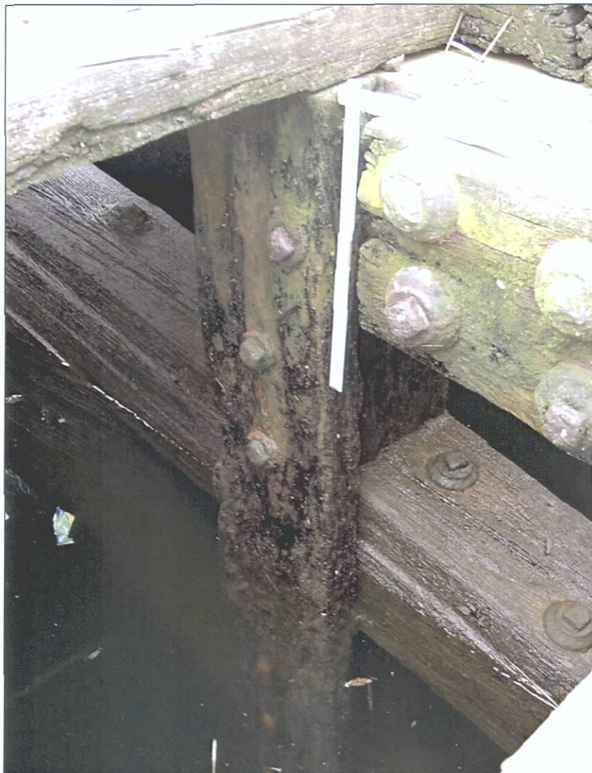
Figure 5-58. Main 16-inch laminated arched truss (T1). View toward southeast (aft starboard corner).
