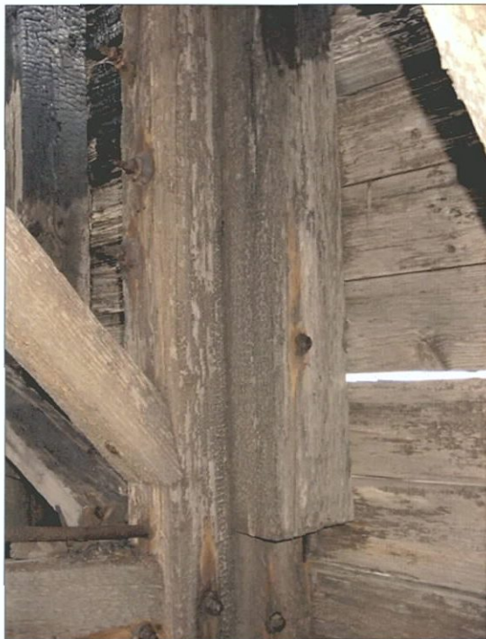
Figure 5-114. Mortise and tenon joint, outer wall, port wing. View to the southwest (aft).
