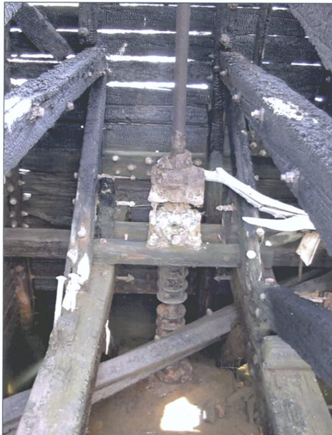
Figure 5-153. Impeller drive shaft.
