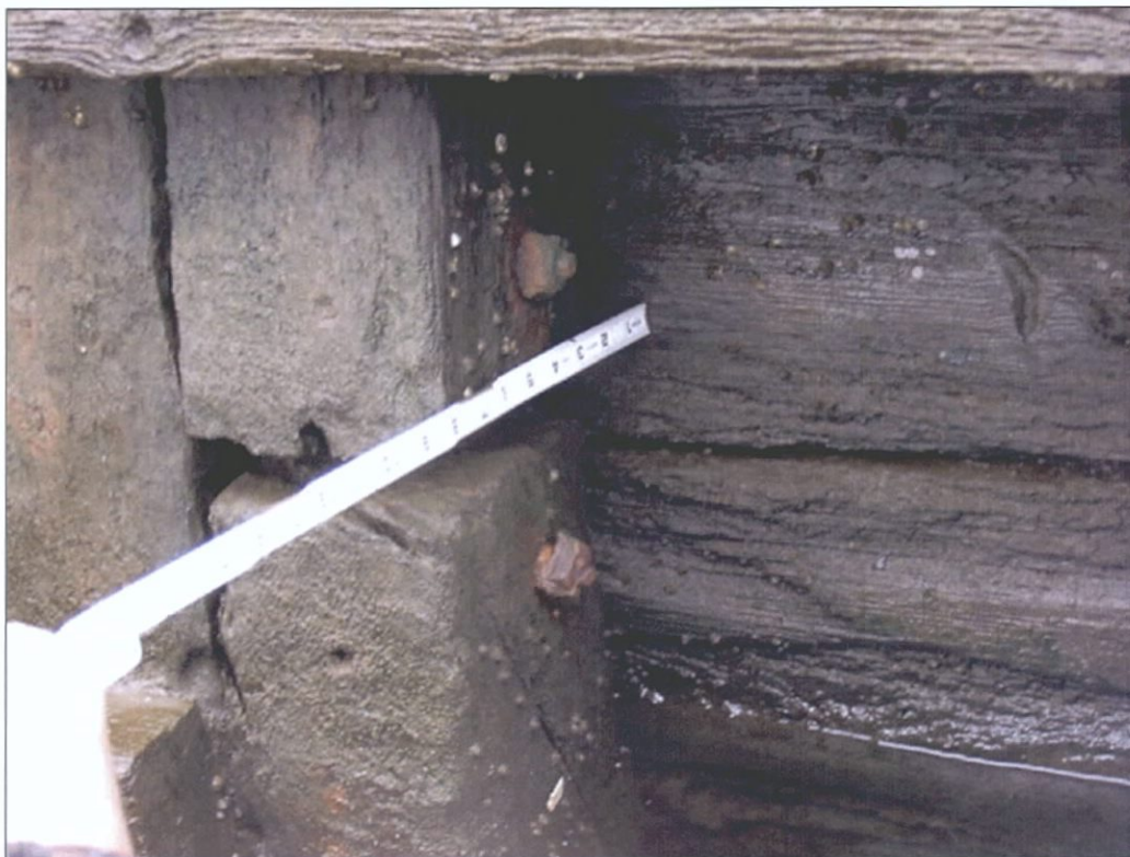
Figure 7-51. Close-up of exposed framing in Figure 7-49. Starboard side, looking east.
