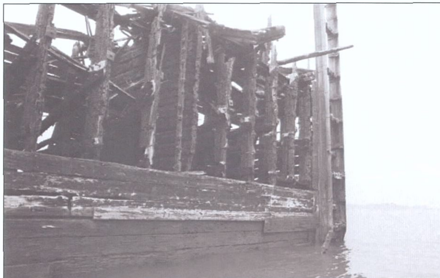
Figure 5-165. Starboard forward spud. View to the north (forward).
