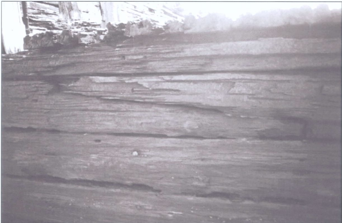
Figure 5-31. Outer hull plank with scarph joint. Forward (north) end of vessel, view to the south.
