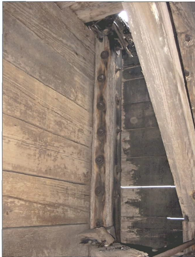
Figure 5-48. Intersection of bulkhead and outer hull in port wing. View to the northwest (port forward).
