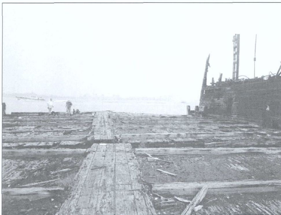
Figure 5-79. Keel block stringers (fore and aft). Also note bilge block stringers (athwartships). View to the north (forward).
