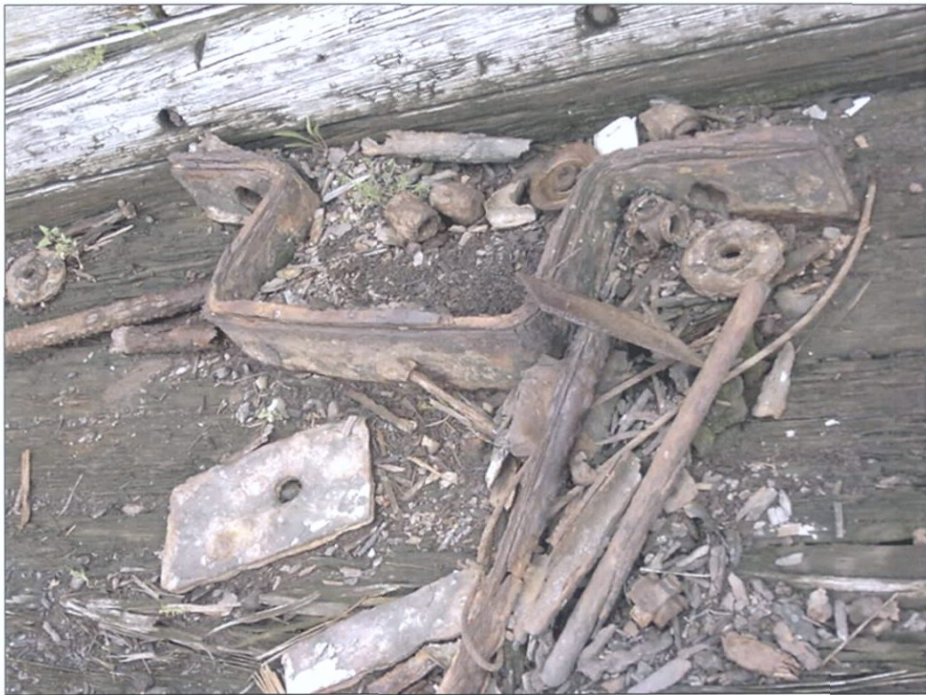
Figure 5-182. Pile of debris including coupling cinch plate, various pipes, and flanges relating to the railing. The piece of iron with the hole in it is a temporary tie down welded to the side of the vessel being repaired.
