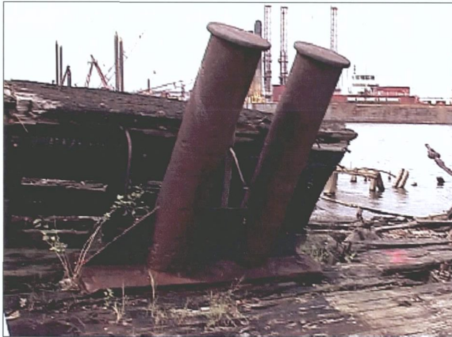
Figure 7-86. View of starboard bulwarks and bollard, looking southwest.
