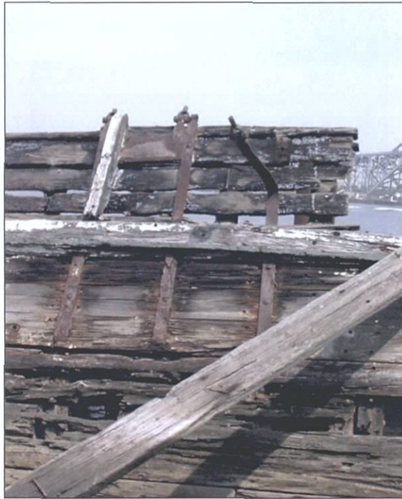
Figure 7-88. Detail of starboard chain plates.
