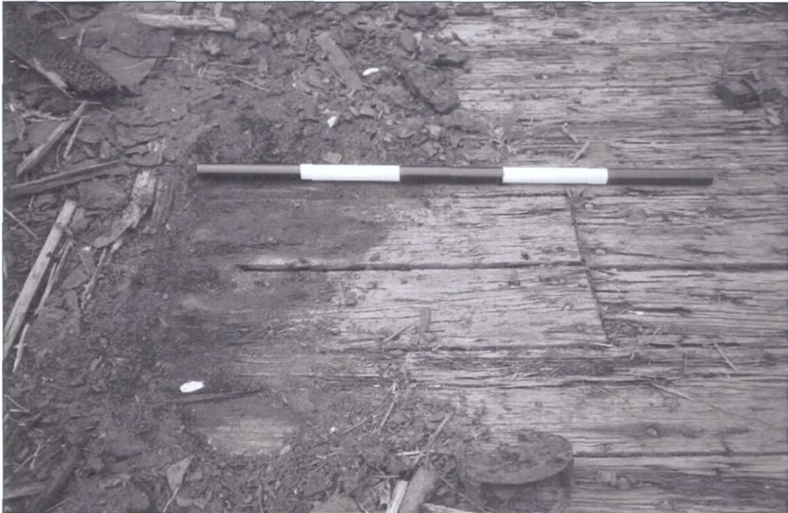
Figure 5-171. Small section of replaced deck plank on main deck. Note different fasteners on patch.
