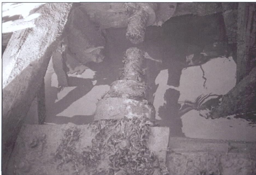
Figure 4-44. Remains of port pivot shaft. The shaft extends through the hull at center of photo. Companion shaft on the starboard side of the vessel terminates in the gear seen in Figures 4-40 and 4-45. View to the southwest (starboard).
