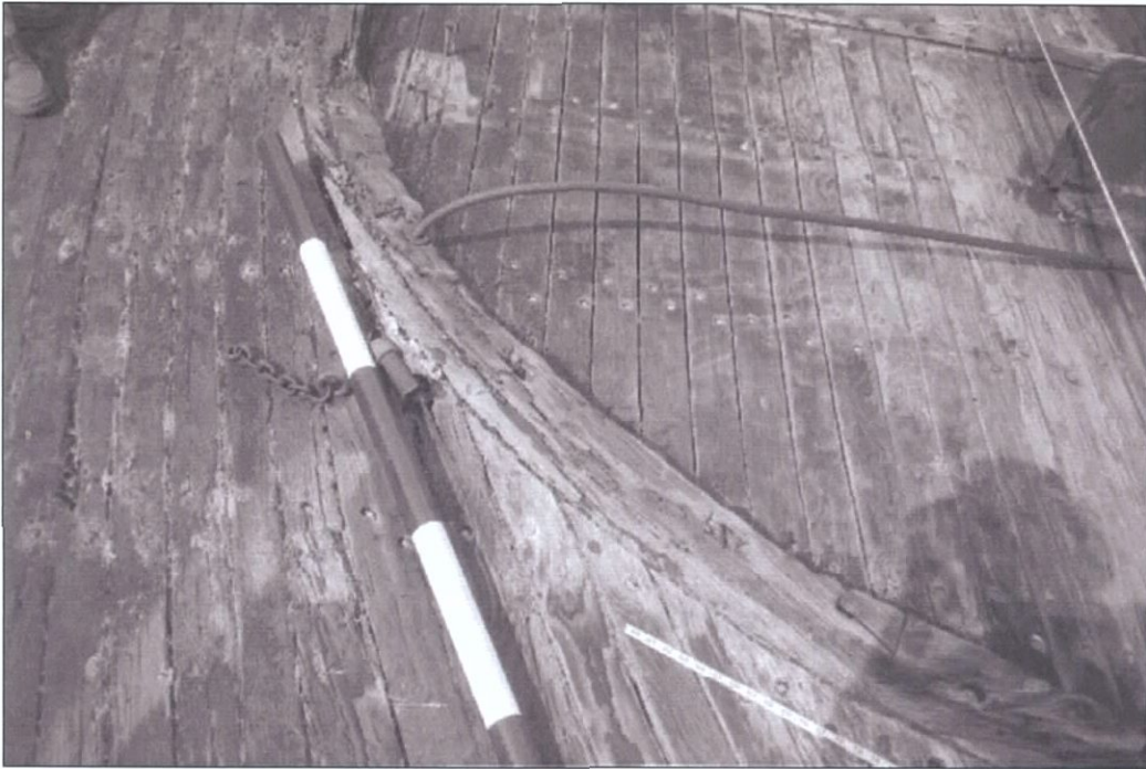
Figure 7-100. Forward end of pilothouse base. Note cut timbers.
