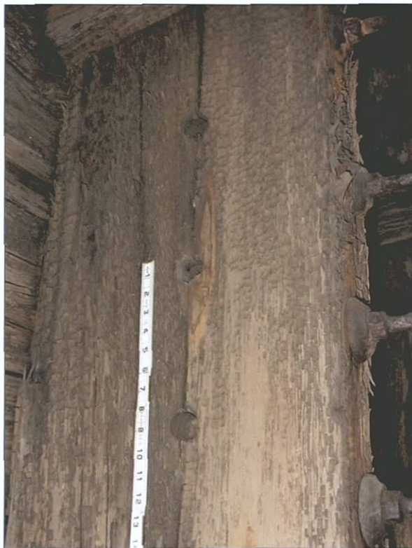
Figure 5-96. Outer wing frame detail, port wing. View to the northwest (port).
