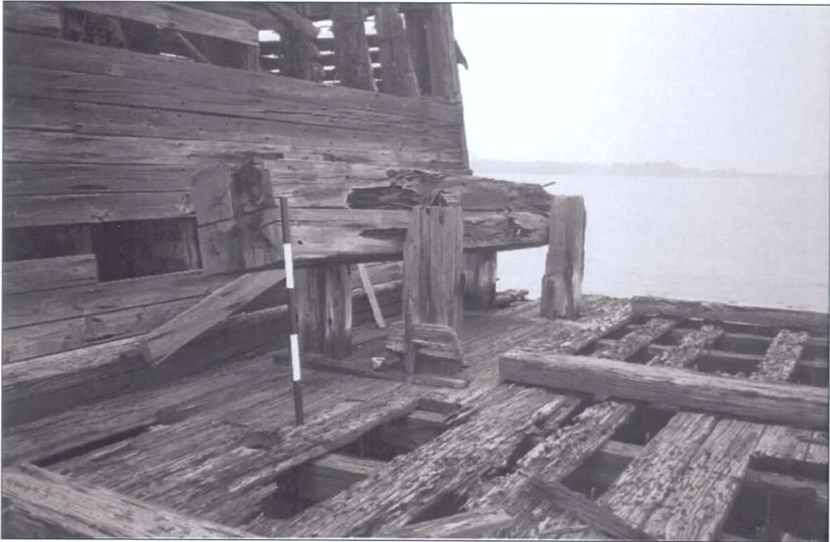
Figure 5-66. Port forward bitt. View to the north.
