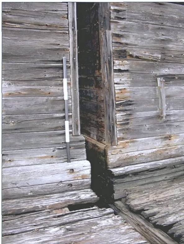
Figure 5-129. Port wing, aft inner corner, showing half round corner post. View to the west (port).
