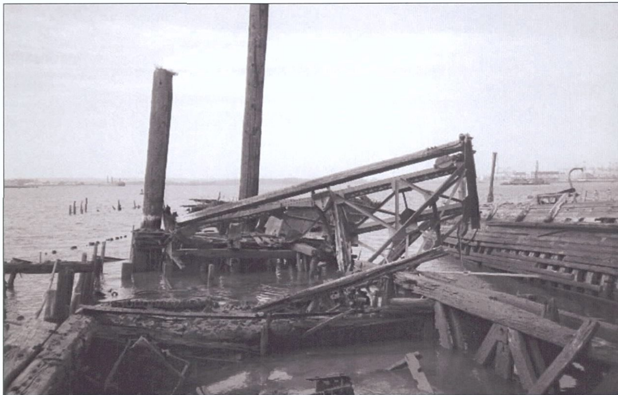
Figure 4-62. Aft end of V36, showing collapsed A-frame and spud poles. View to the north.
