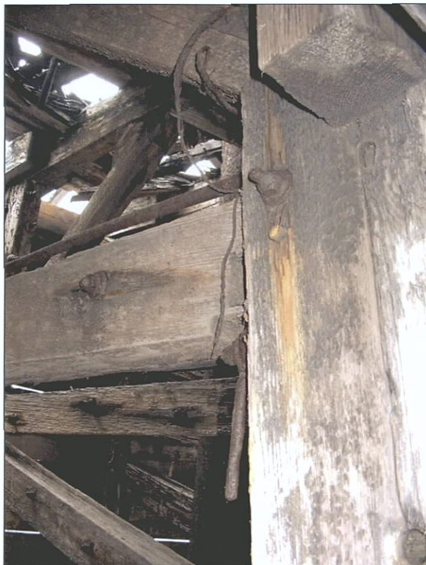
Figure 5-111. Opposite side of joint in Figure 5-110. Note iron fastener. View to the northwest (forward).
