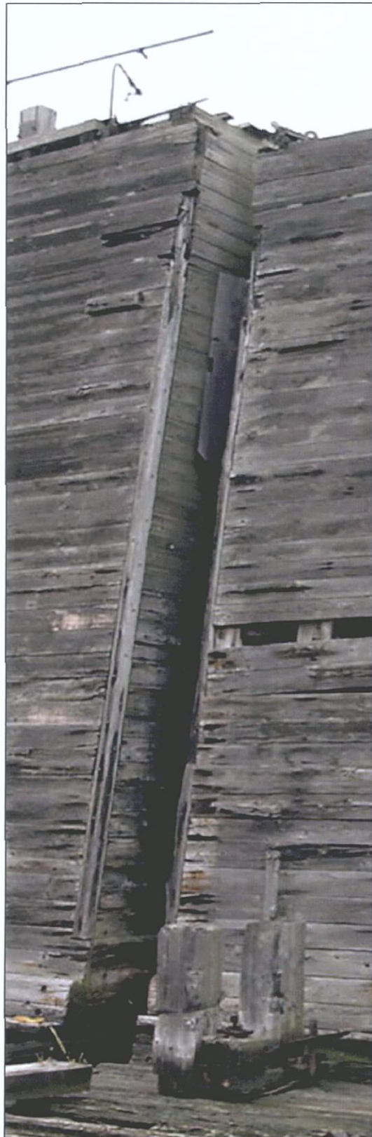
Figure 5-132. Port wing aft corner showing vertical half round.
