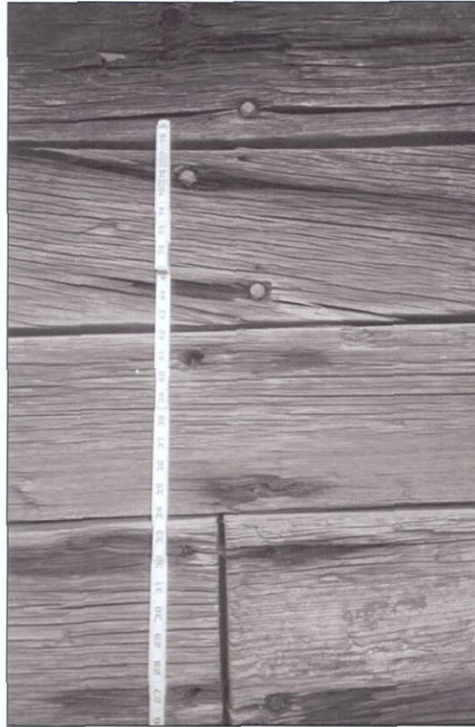
Figure 5-125. Port wing planking showing pattern of spikes. View to the west (port).
