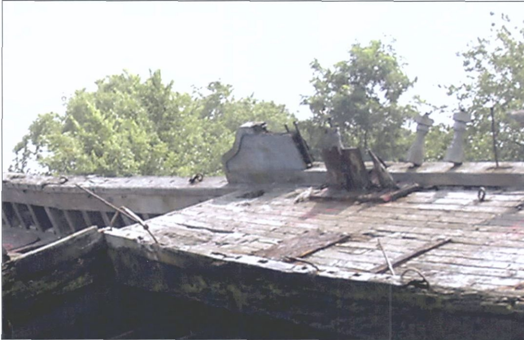
Figure 7-78. Detail of Figure 7-77 showing extension of main deck bulwark cap into the quarterdeck as the covering board. View to the southwest.
