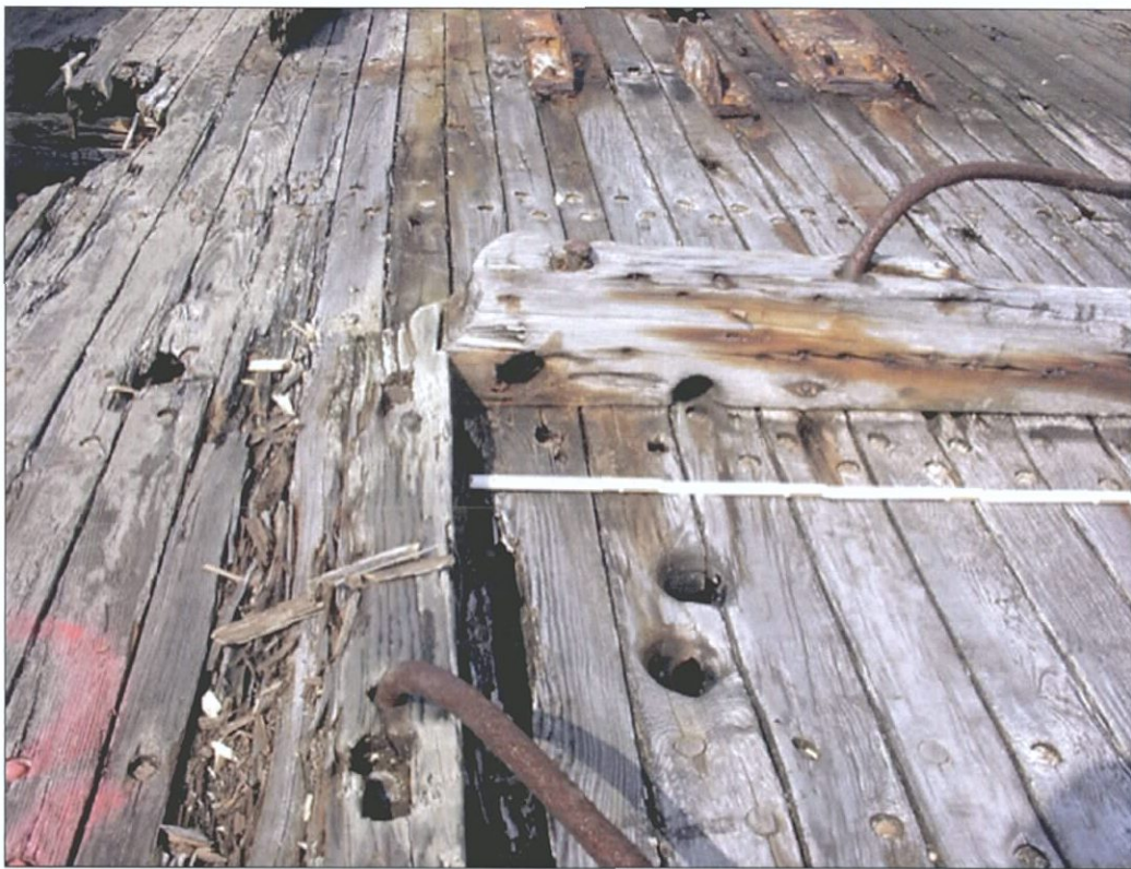
Figure 7-101. Aft end of pilothouse. View to the north.
