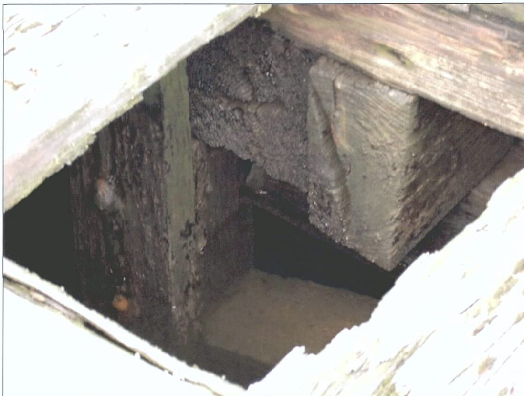
Figure 5-75. View of bitt structure at deck beam 6. View toward northwest (forward port). Note stringer to right of vertical stanchion, chock to right of stringer, and transverse support below stringer and chock.
