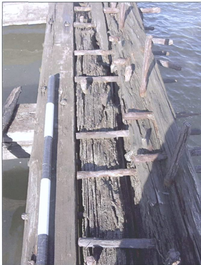
Figure 6-94. Port side view aft (north) showing three-timber waterway of cargo deck. Note pattern of fasteners.
