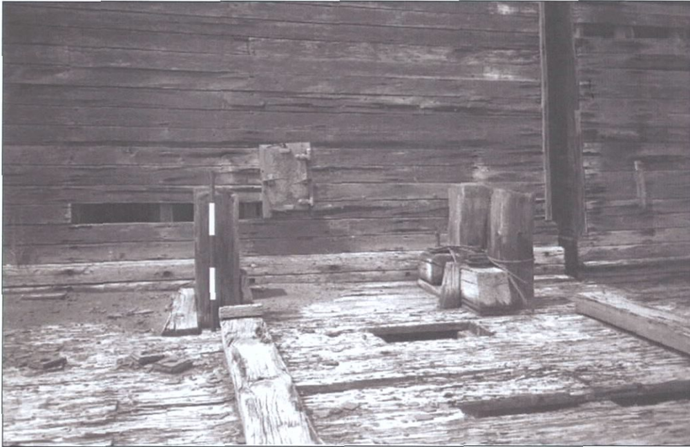
Figure 5-90. Forward looking port (west). Note access hole right of center.
