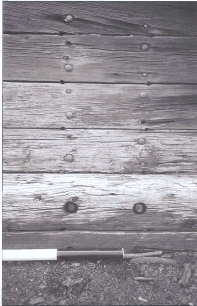
Figure 5-174. Port wing chine logs and outer planking. Note countersunk bolts and carriage bolts. View to the west (port).
