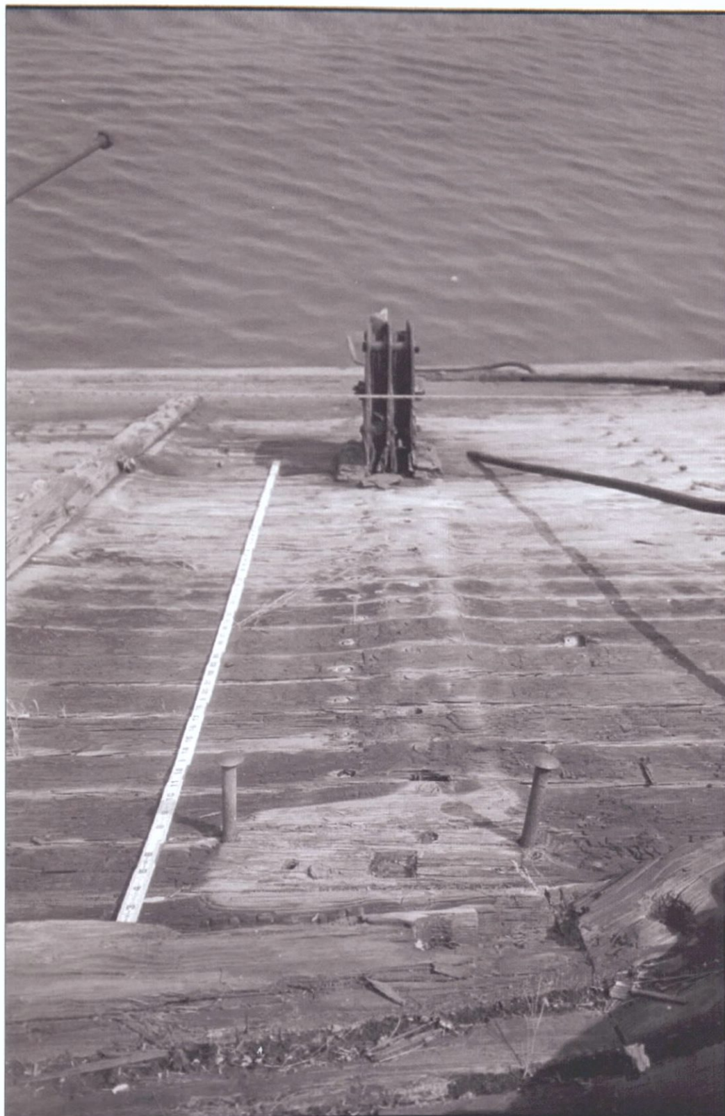
Figure 7-83. Forward section of pilothouse showing remains of steering gear. View to the east (starboard). Note mounting pad for pulley in foreground.
