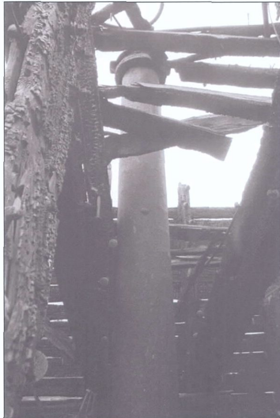
Figure 5-157. Vertical discharge pipe. Starboard wing, view to the east (starboard).
