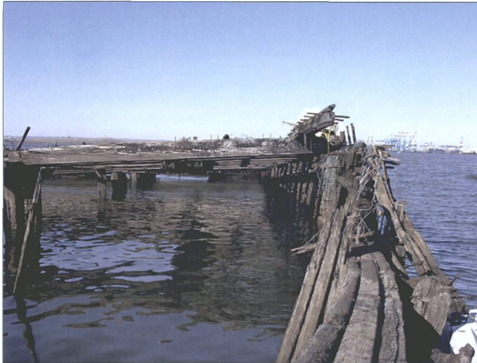
Figure 6-81. Bow looking aft (north) showing composite mold and bilge ceiling.
