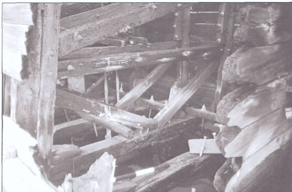
Figure 5-100. Wing truss at main deck level. Starboard wing. View to the northeast.
