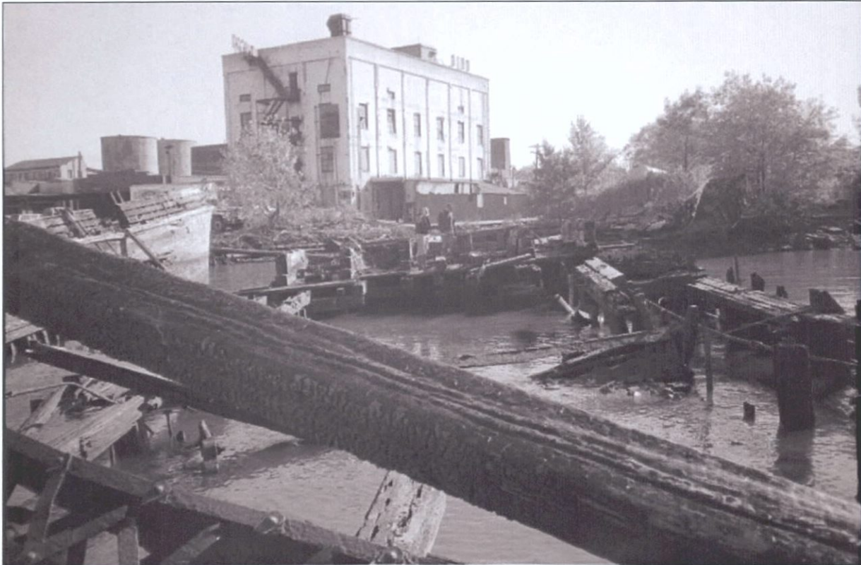
Figure 4-26. V36 main deck. View to the south (forward). Note collapsed A-frame in foreground.
