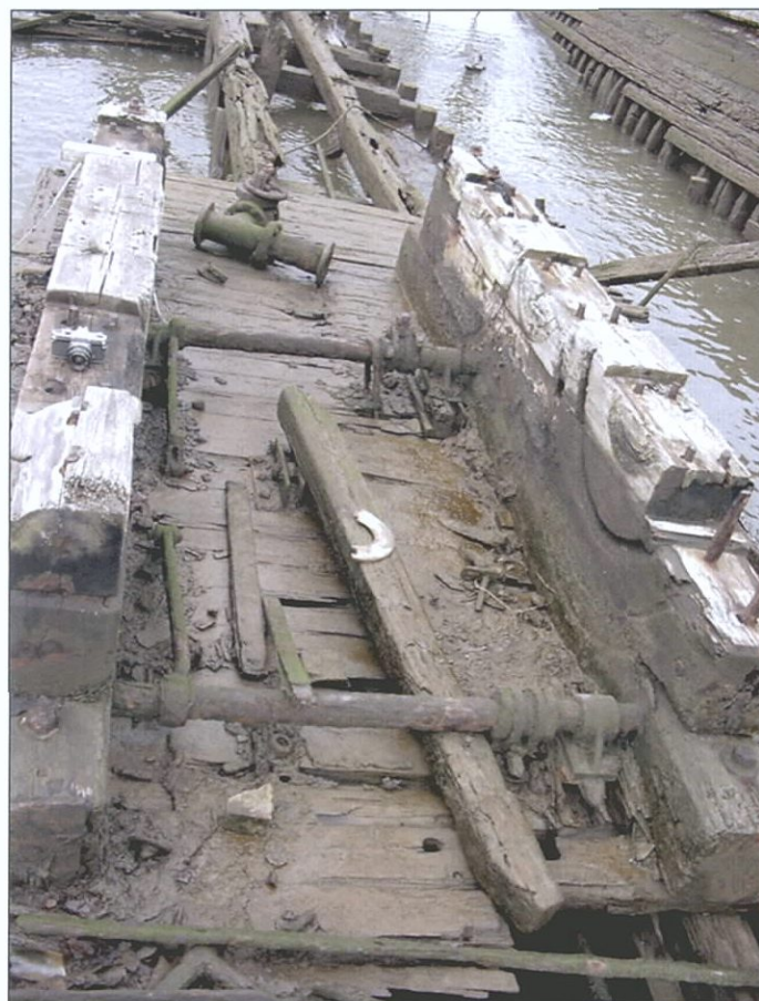
Figure 4-55. Port-most machinery mounts on main deck. View to the north (aft).
