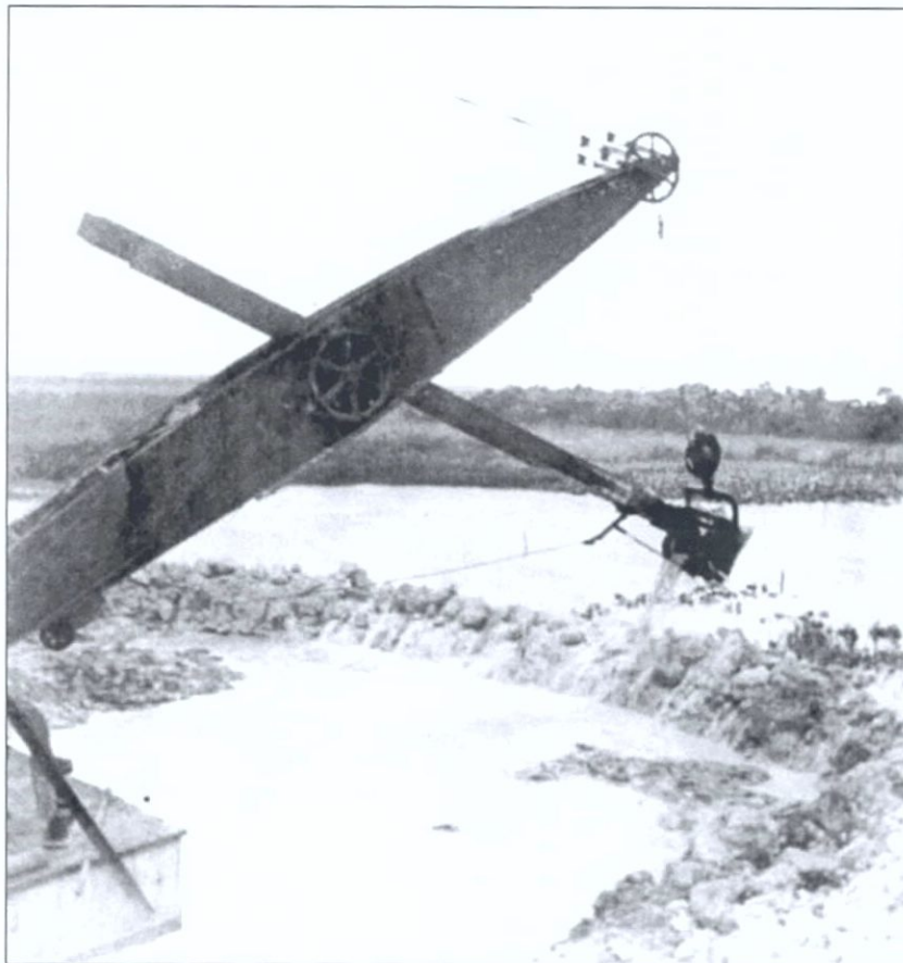
Figure 4-04. Close-up of bucket dredge Miami at work on the Miami River, circa 1910 (photo courtesy of the Florida Photographic Collection).
