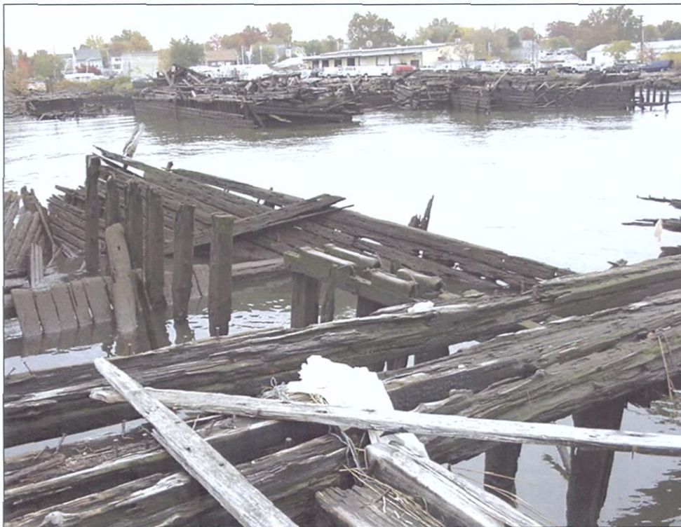
Figure 6-97. View starboard forward (southwest) showing centerline stanchion and portion of stringers.
