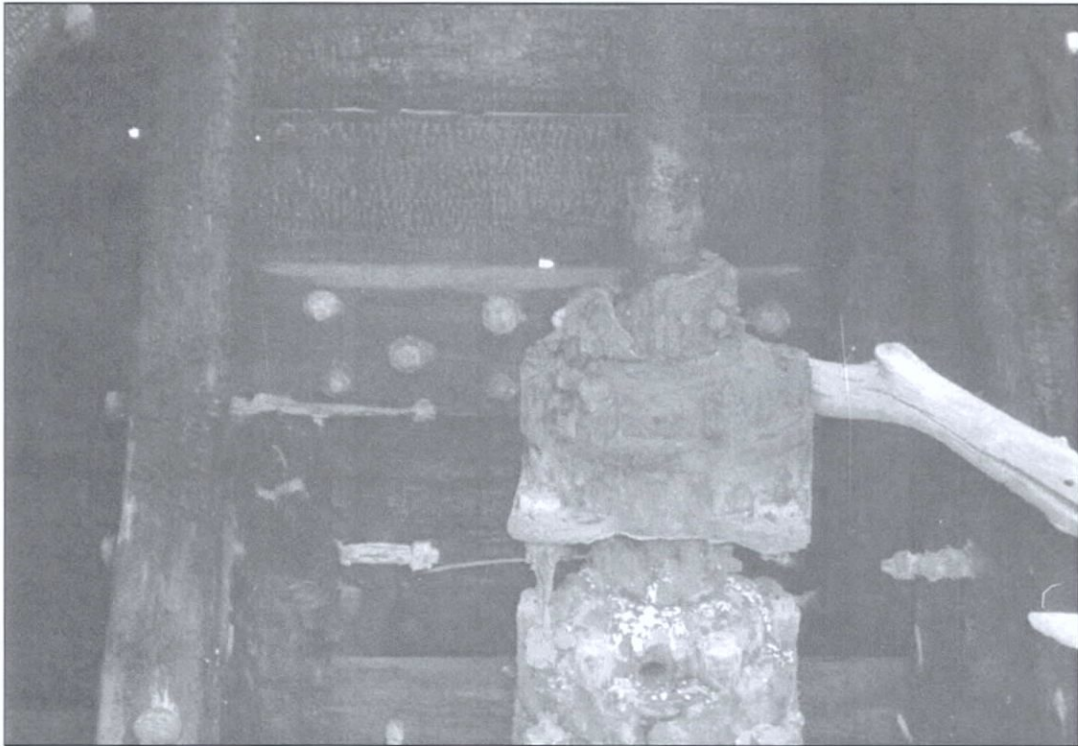
Figure 5-34. View of chock reinforced butt joint. View to the east (starboard).
