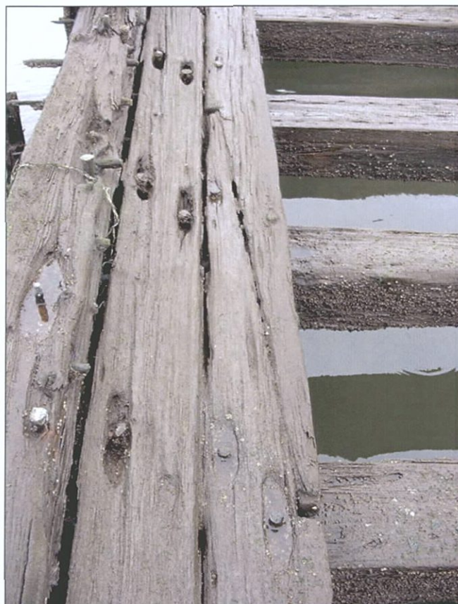
Figure 6-96. Port side looking forward (south) showing scarph joint.
