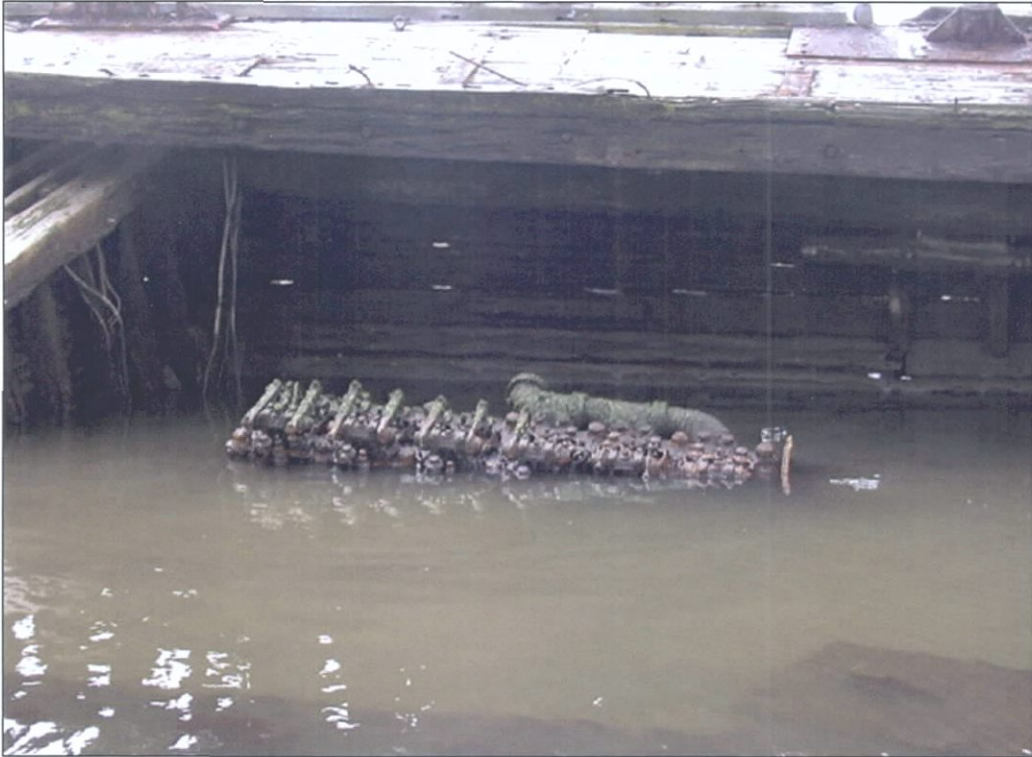
Figure 7-68. Single 6-cylinder diesel engine in engine room. Note aft bulkhead on left. Looking starboard (west).
