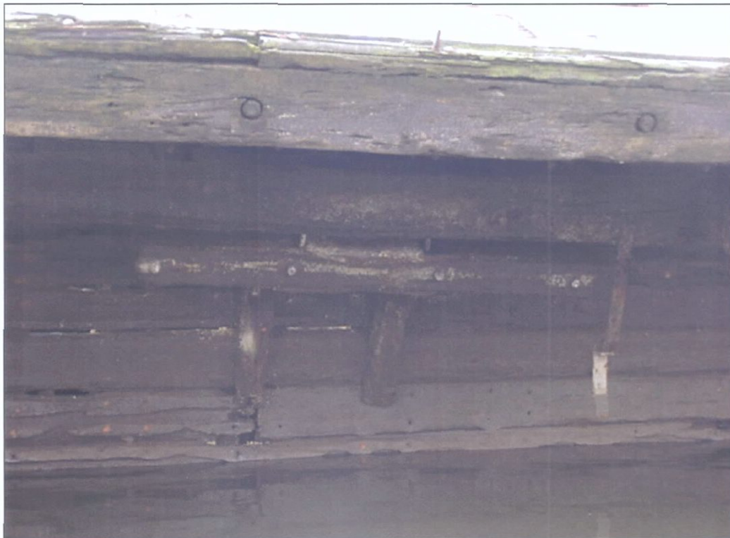
Figure 7-63. Photo of seine boat davit anchor structure, located below the quarterdeck.
