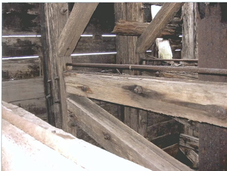
Figure 5-112. View of horizontal truss beam tie rod and joint, outer wall of starboard wing. This joint is directly opposite that shown in Figures 5-109 and Figure 5-110. View to the northwest (forward).
