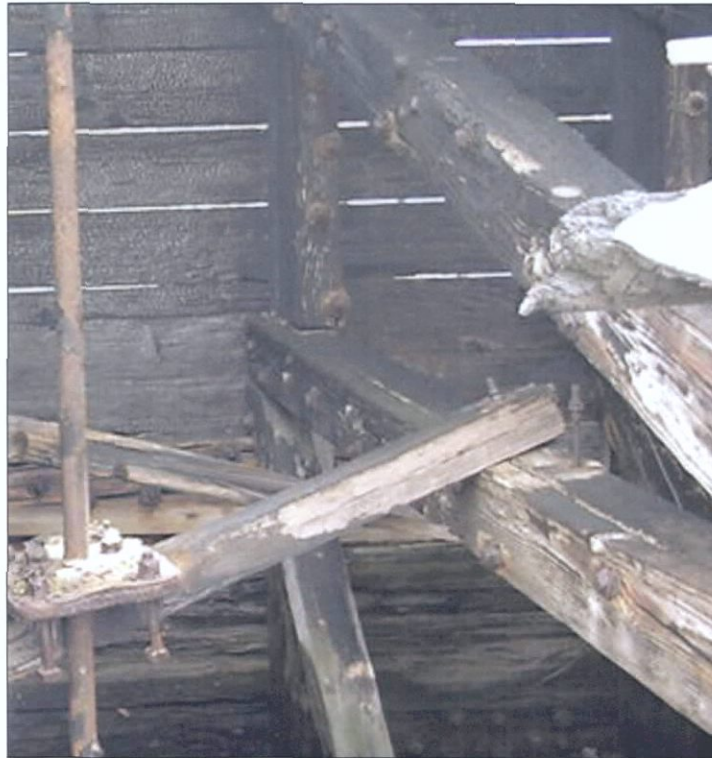
Figure 5-109. Starboard wing outer wall, view to the east. Note joint against outer hull, at center of photo.
