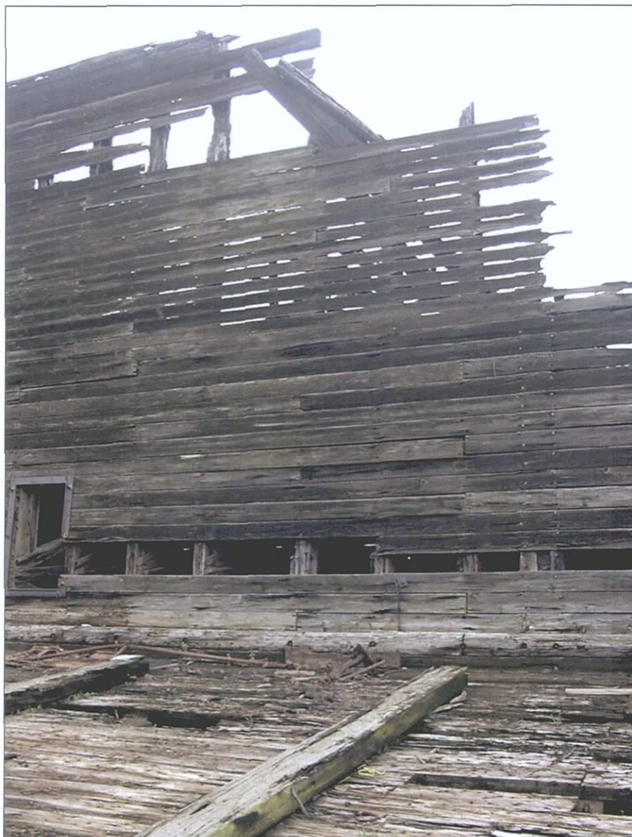
Figure 5-118. Port wing showing inner wing wall planking. Note change in dimension toward top. View to the west (port).
