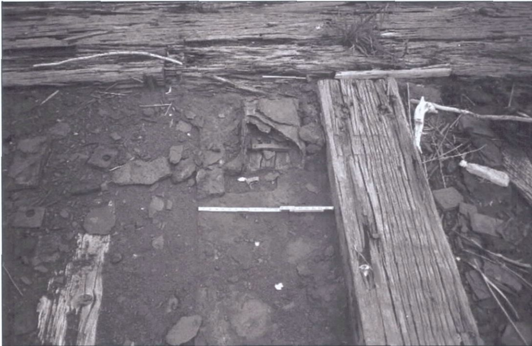
Figure 5-84. Deck drain. View to the east (starboard).
