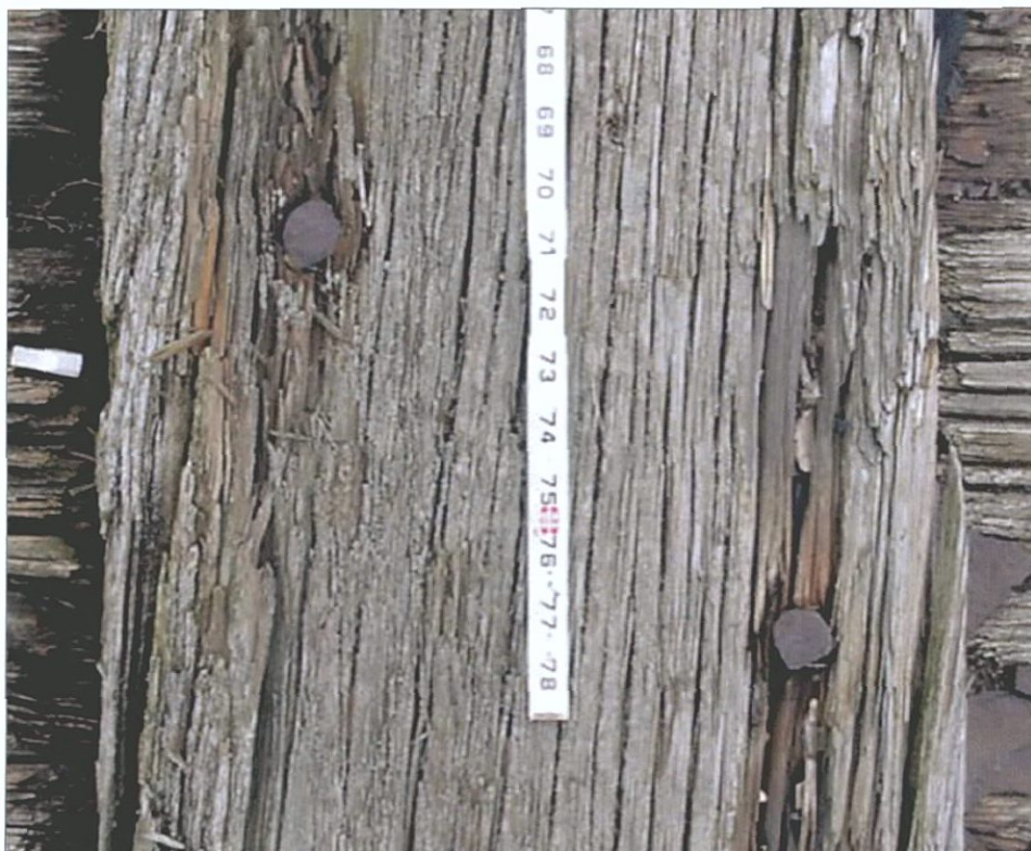
Figure 5-83. Bilge block stringer fastener pattern detail.
