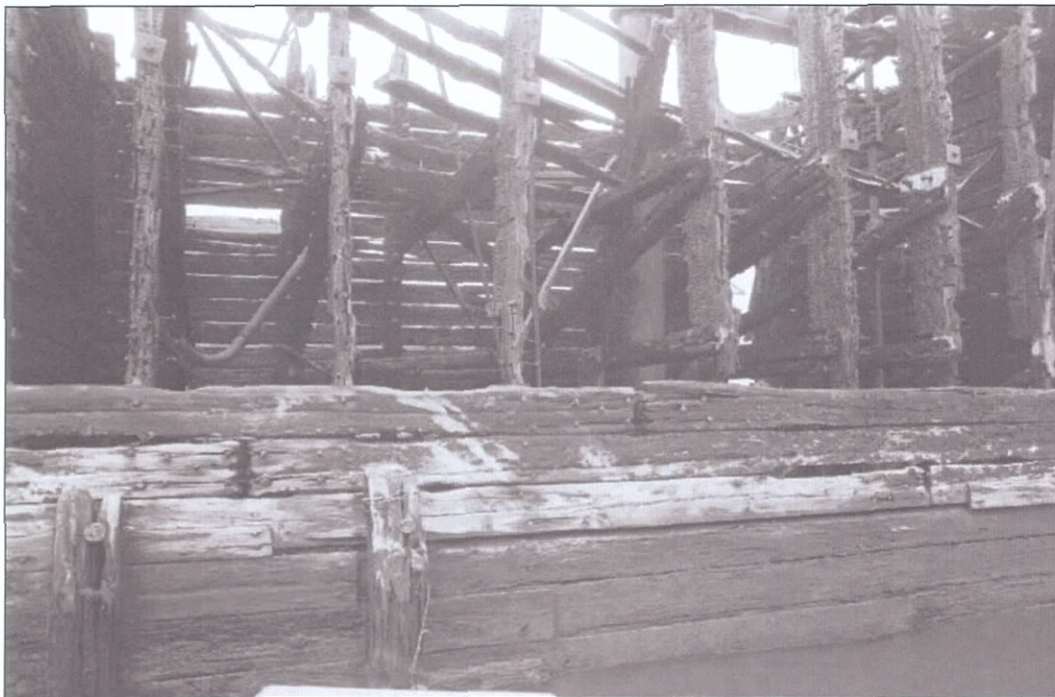
Figure 5-45. View starboard wing showing placement of watertight bulkheads, noted at opposite ends of photograph. View to the west.
