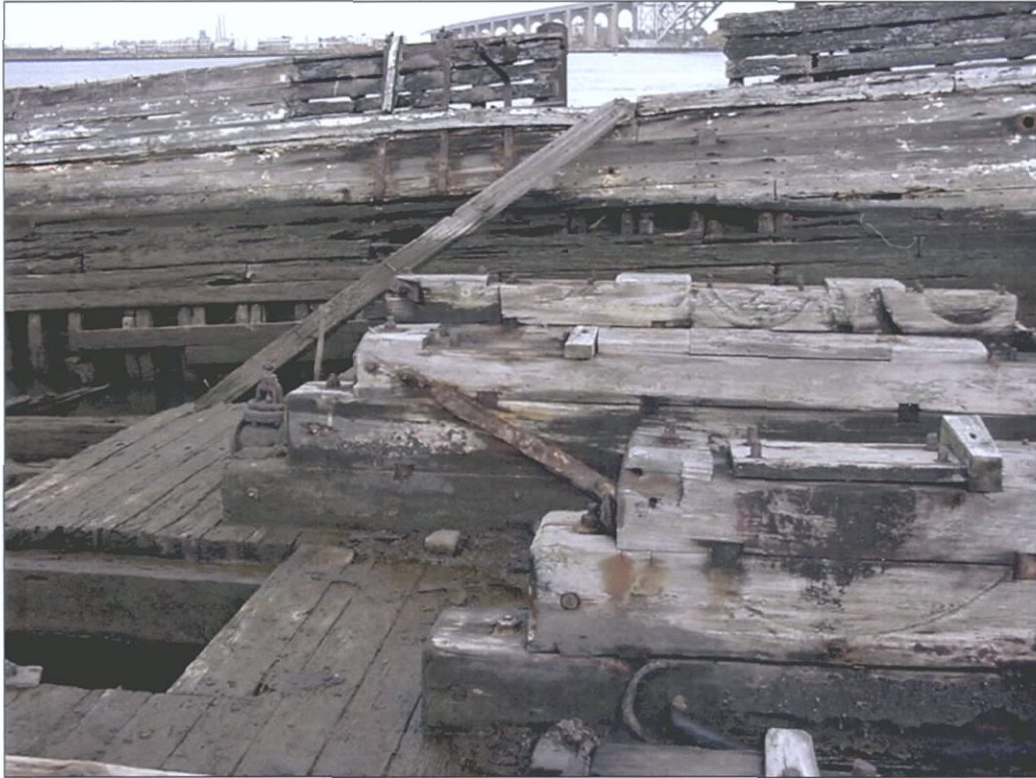
Figure 4-52. Main deck showing machinery mounts. View to the east (port).
