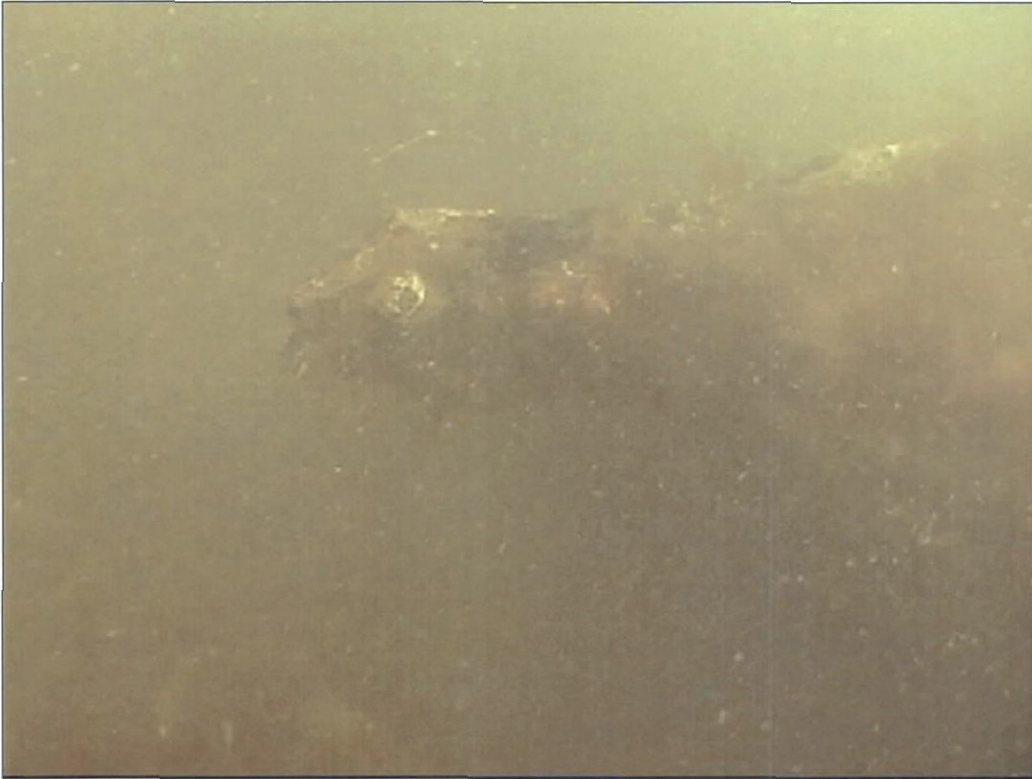
Figure 8-19. Video frame of deteriorated iron framing of SS16b.
