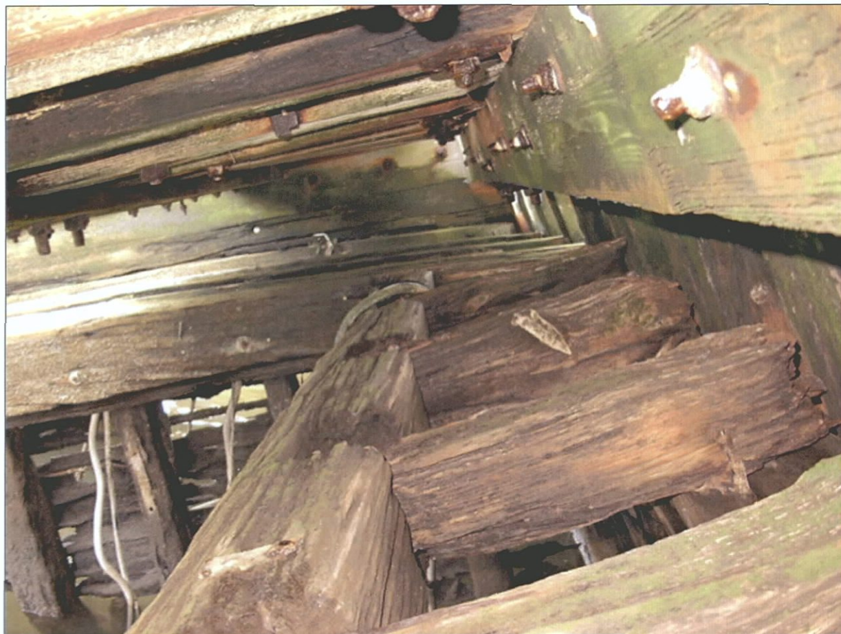
Figure 7-61. Longitudinal stringer in engine room compartment, looking forward (south).
