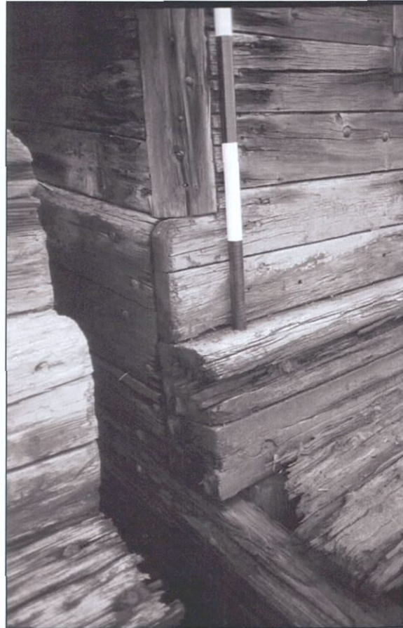
Figure 5-121. Port wing aft showing wing chine logs. View to the northwest (port).
