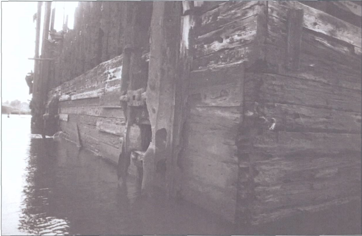
Figure 5-36. Sacrificial wooden planking added to hull of V2 below waterline.
