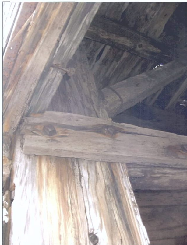
Figure 5-110. Port wing, inner wall truss joint. Note composite horizontal beam. View to the southwest (aft).
