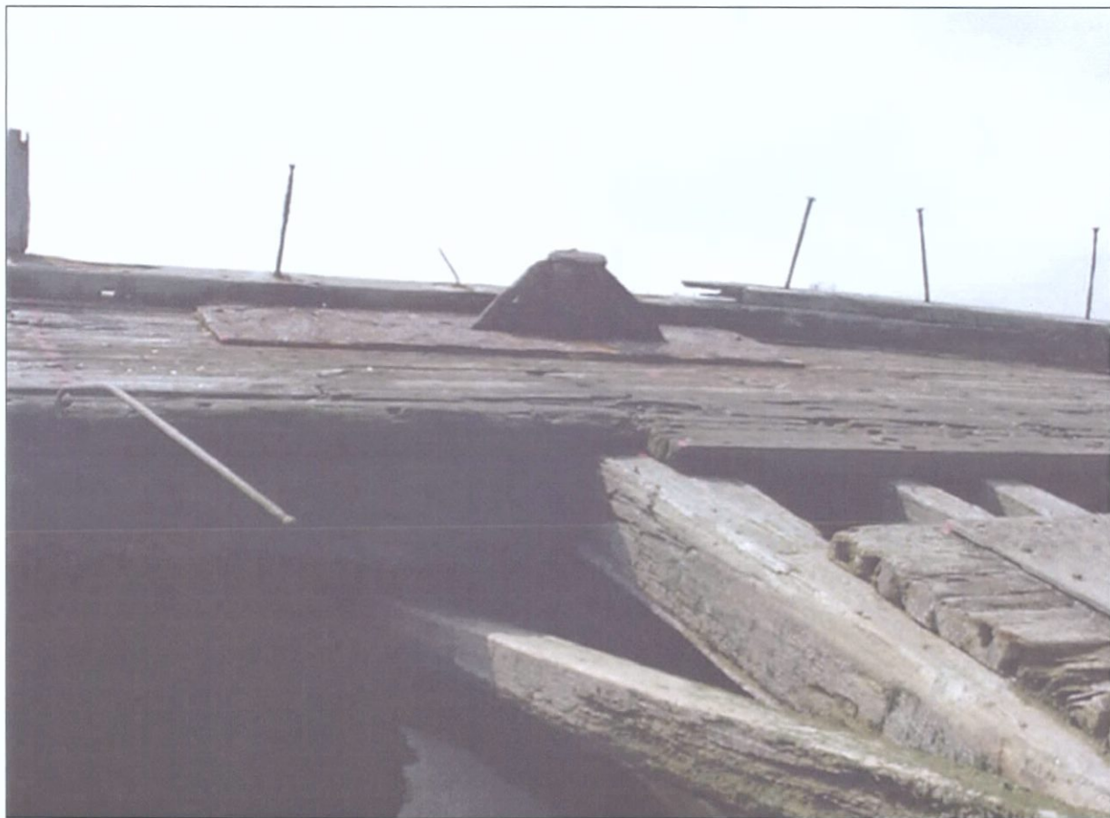
Figure 7-94. Aft davit, starboard side, looking northwest.
