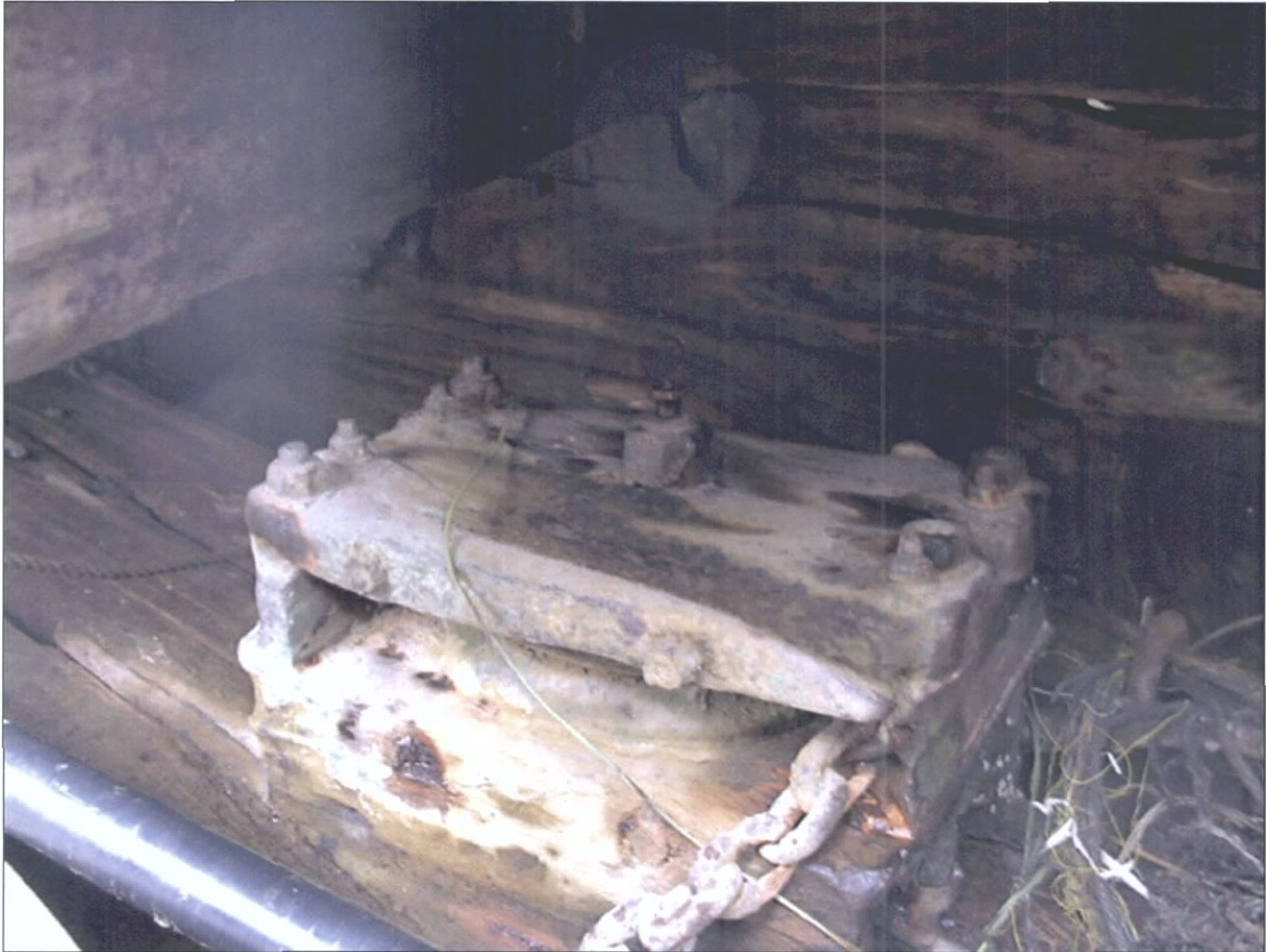
Figure 7-105. Starboard steering pulley, looking southwest.
