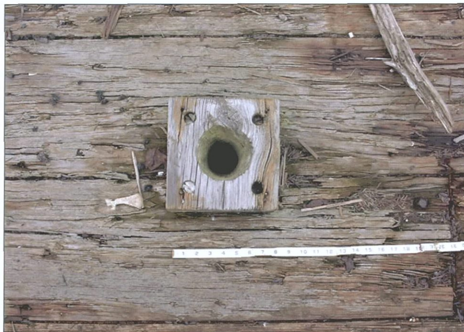
Figure 5-87. Deck fitting with tapered hole.
