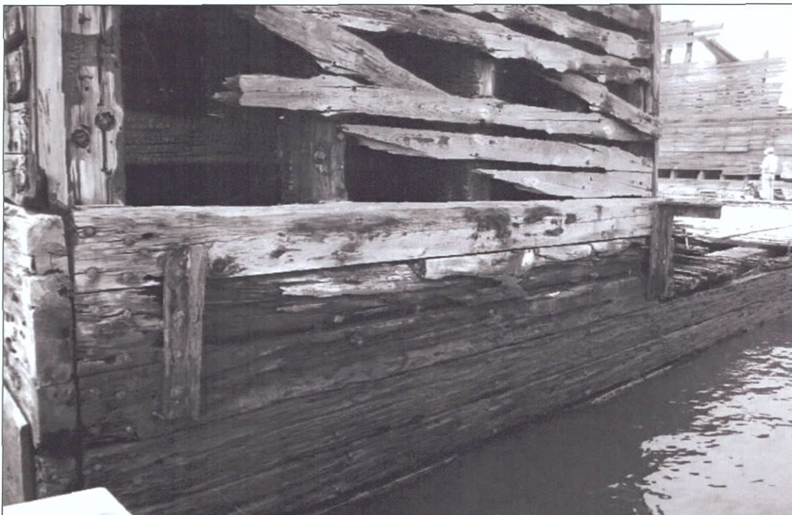
Figure 5-29. Starboard quarter forward, view to the southwest (aft), showing transition between hull planking and wing planking.
