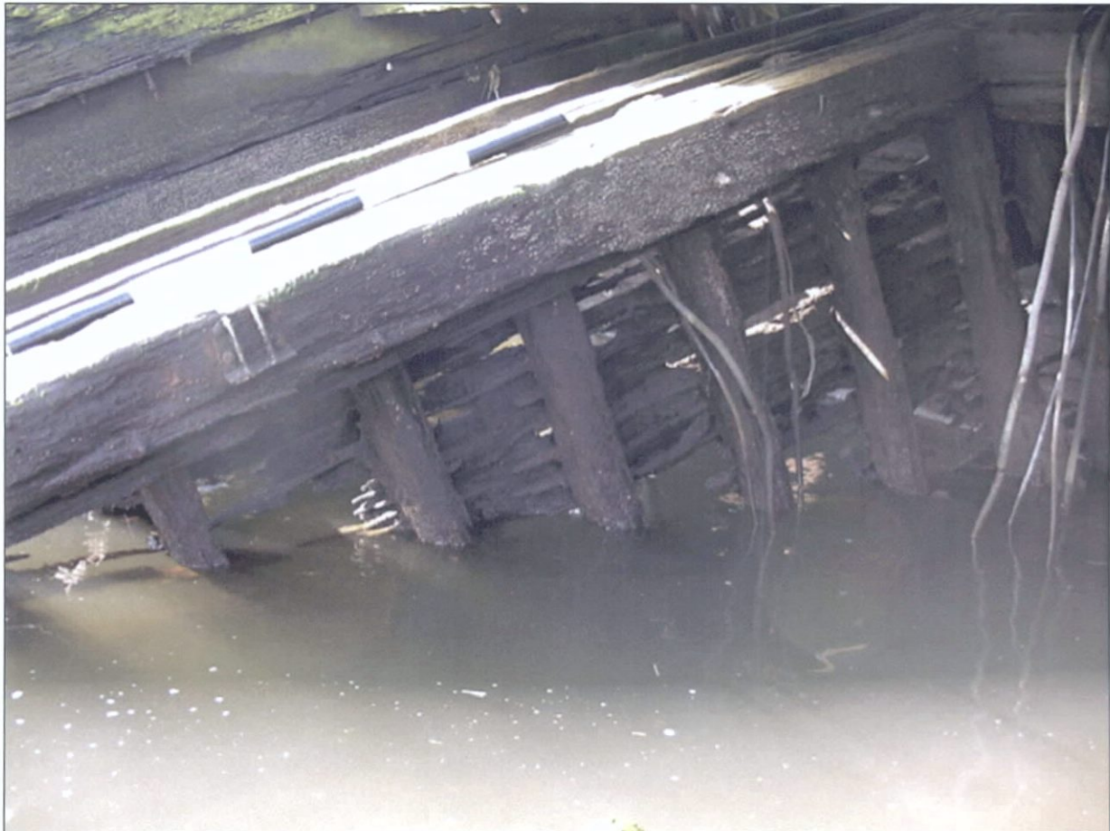
Figure 7-65. Detail of aft bulkhead showing stanchions and facing planks, starboard side, looking south (forward).
