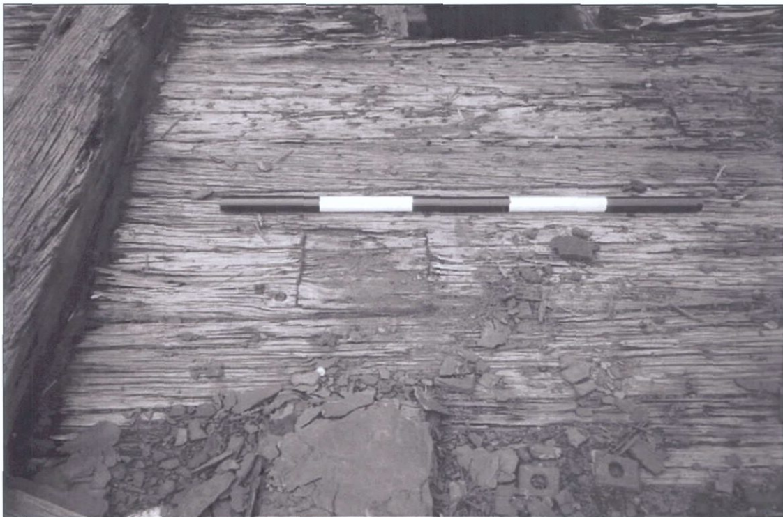
Figure 5-172. Small plug repair on main deck.
