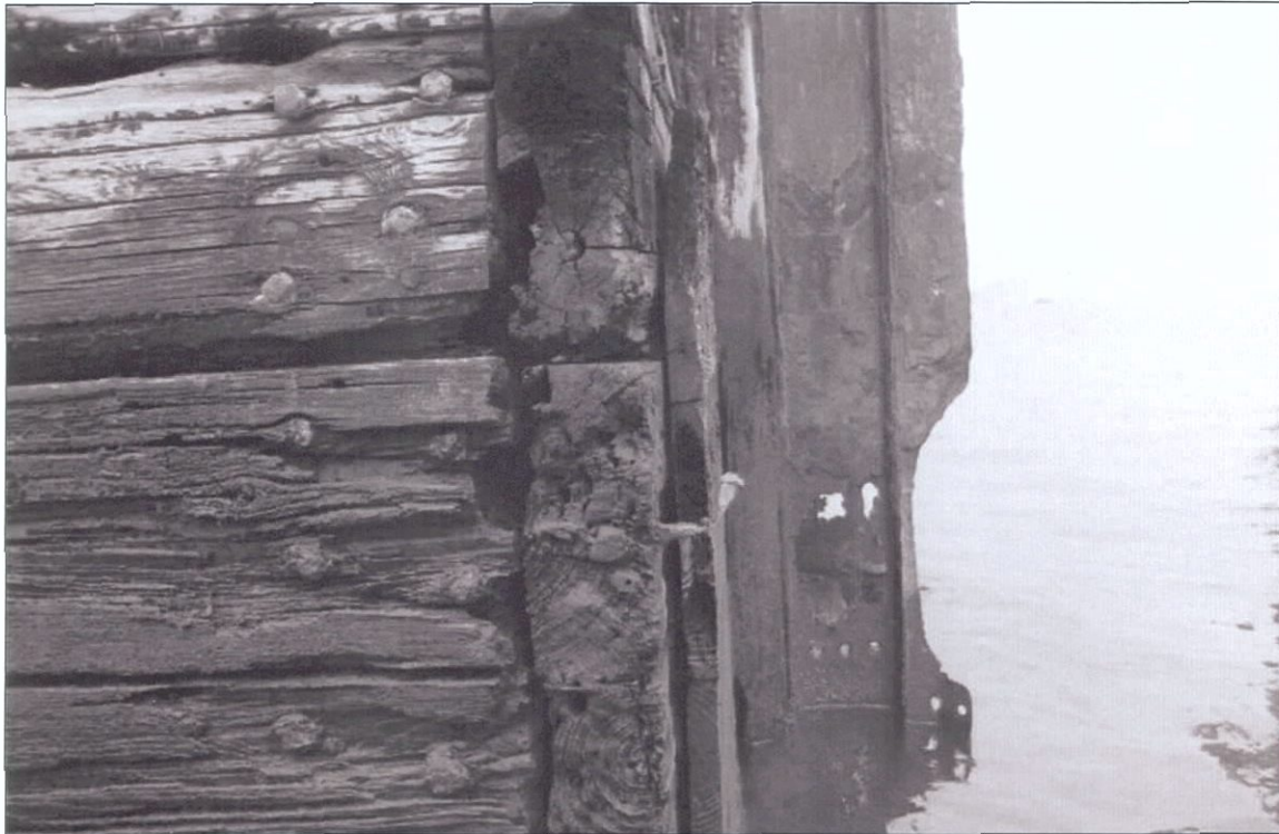
Figure 5-28. Outer planking of pontoon.
