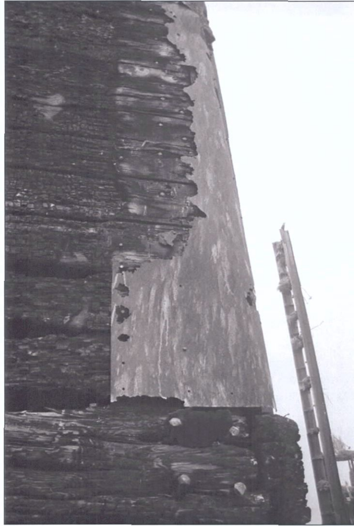
Figure 5-133. Starboard wing aft showing metal sheathing. View to the north (forward).
