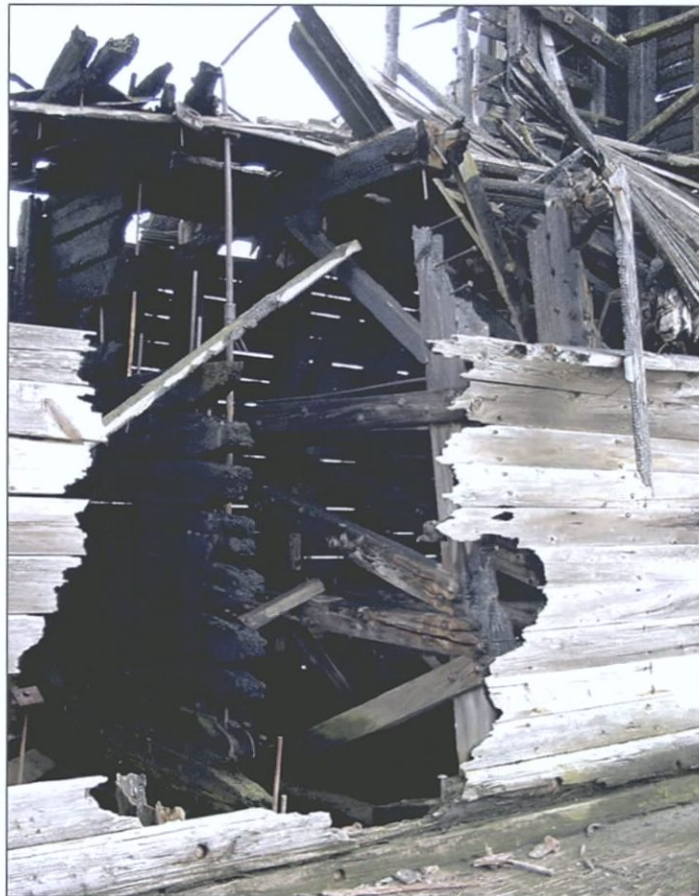
Figure 5-103. General view of wing truss. Starboard, view toward aft quarter of V1 (southeast).
