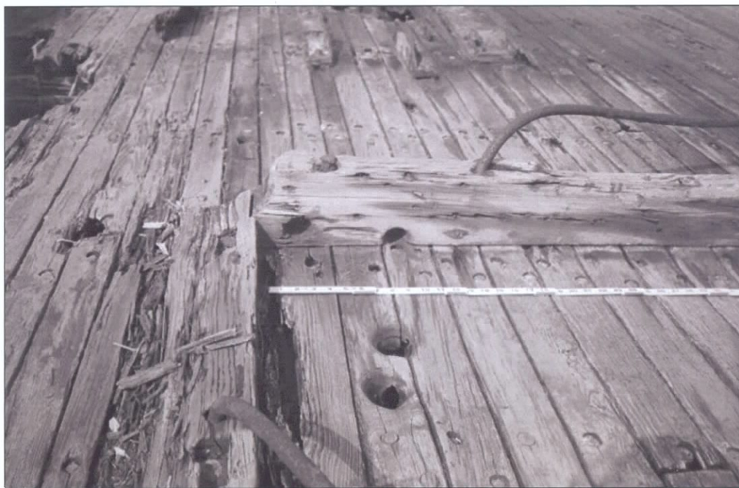
Figure 7-85. Aft pilothouse bulkhead remains showing steering cable passages. View to the north (aft).
