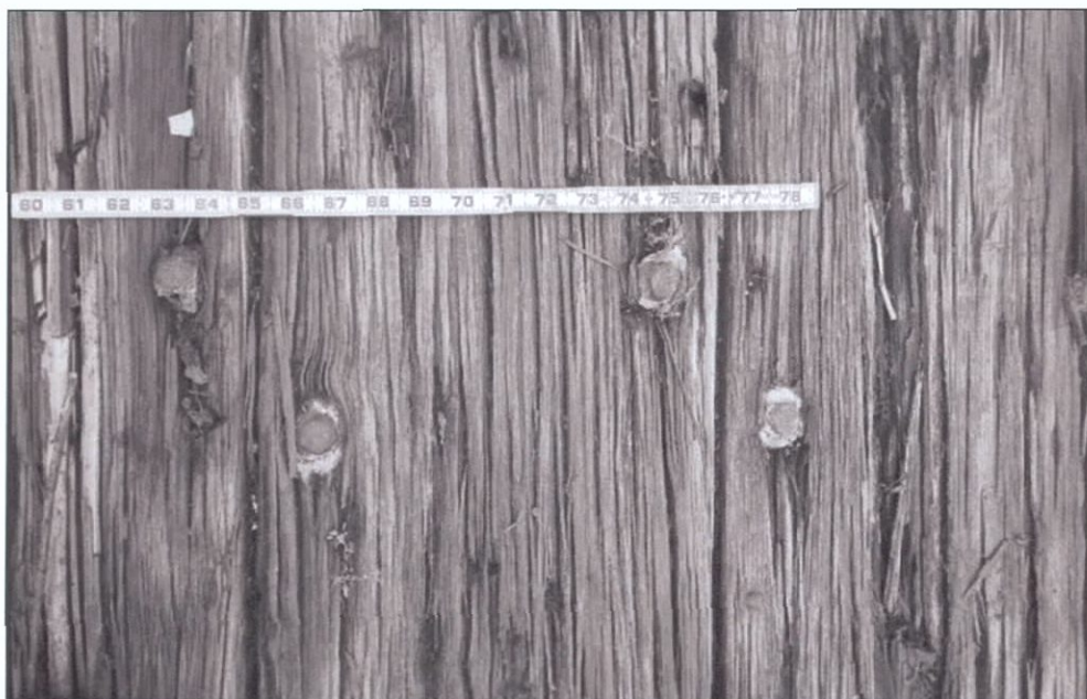
Figure 5-176. Deck plank detail showing staggered fasteners.
