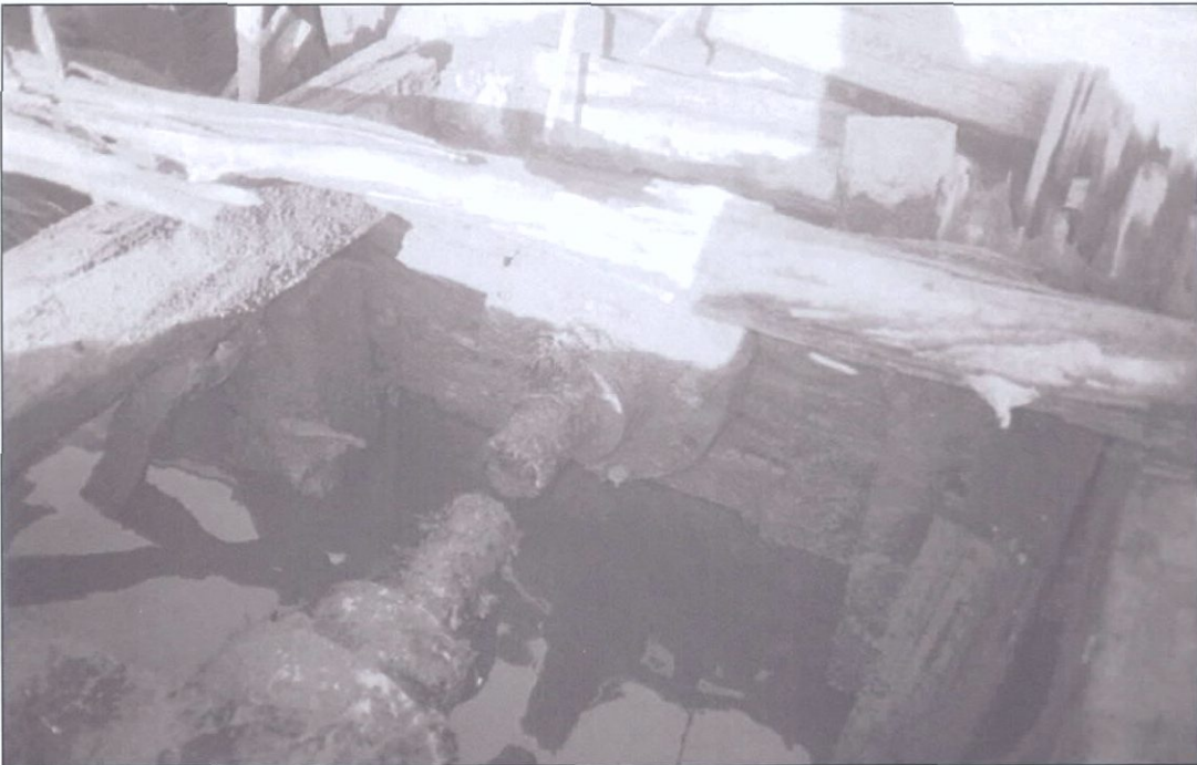
Figure 4-42. Remains of port pivot shaft. The shaft extends through the hull at center of photo. The companion shaft on the starboard side of the vessel terminates in the gear seen in Figures 4-40 and 4-45. View to the southwest (starboard).
