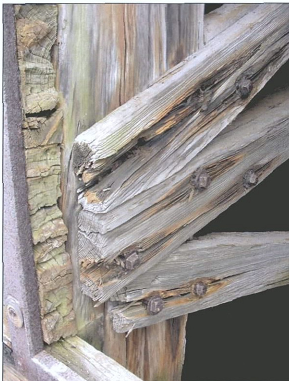
Figure 5-107. Inner wing wall frame with truss timbers fastened. Note lower timber is notched rather than composite. View of starboard wing, view to the south (aft).
