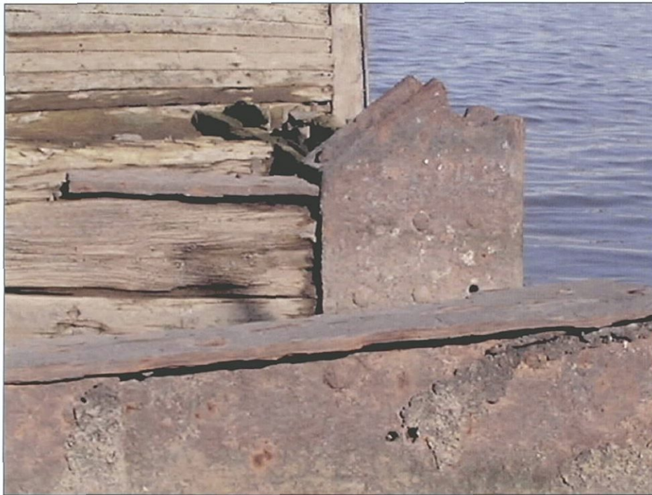
Figure 4-47. Profile view of port A-frame mount. View to the east (port).
