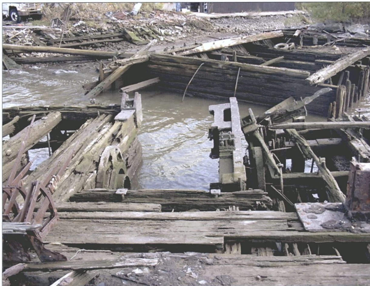
Figure 4-28. Ladder well in the bow of V36. Note remains of A-frame attachment. View to the south (forward).
