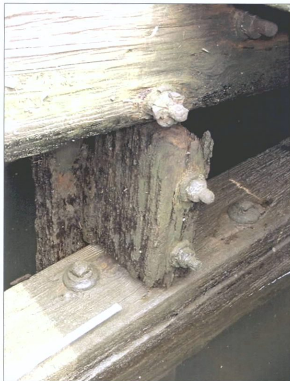
Figure 5-51. Example of chock between hull structural members.
