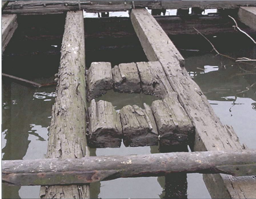
Figure 6-93. Detail of mainmast hole. View to the west.
