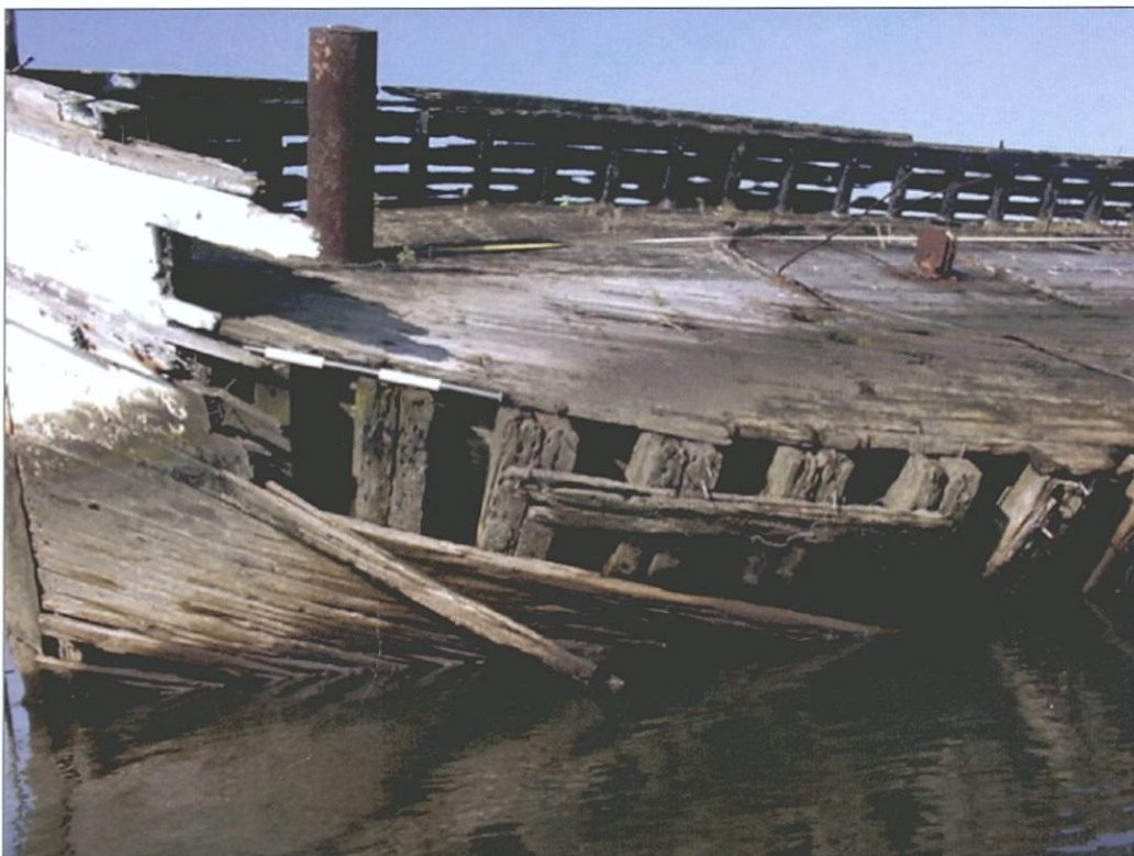
Figure 7-52. View of port bow showing exposed canted frames, looking west.
