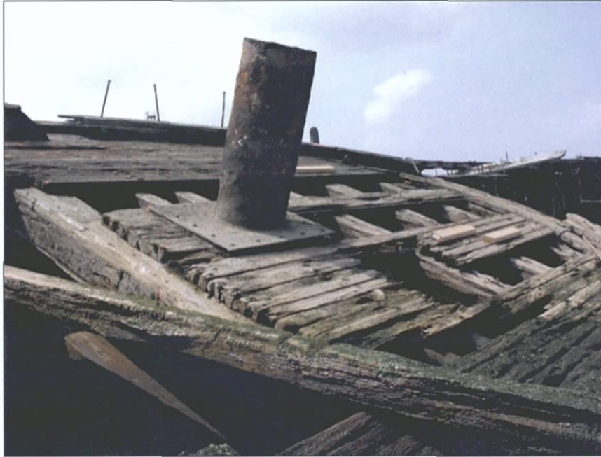
Figure 7-99. Aft ventilation stack.
