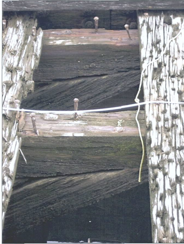
Figure 5-61. Truss 6 at main deck. Note end of triangular chock at left. View to the north (forward).
