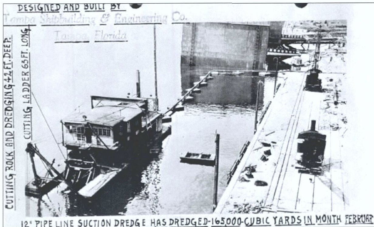
Figure 4-12. Small suction dredge at work in Tampa. Built by Tampa Shipbuilding and Engineering Company, this dredge had a 12-inch suction pipe with a 63-foot long cutting ladder (photo courtesy of the Florida Photographic Collection).
