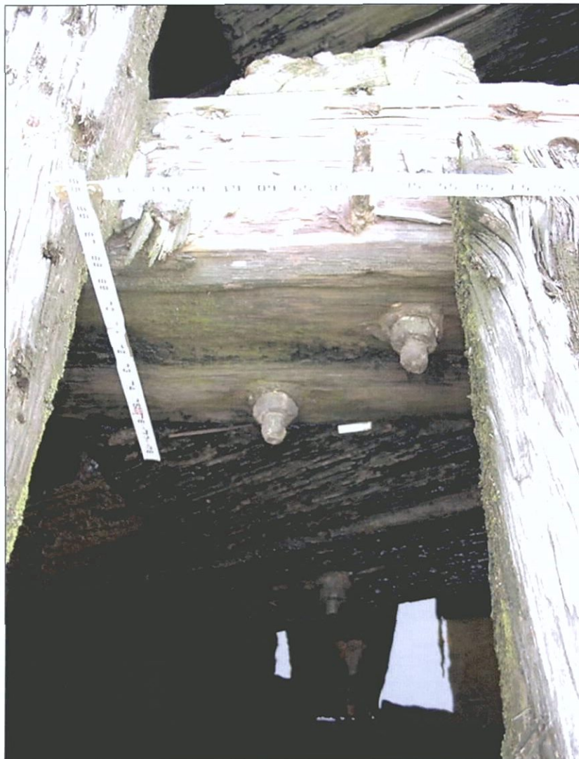
Figure 5-43. Reinforced butt joint on deck beam. View to the north (forward).
