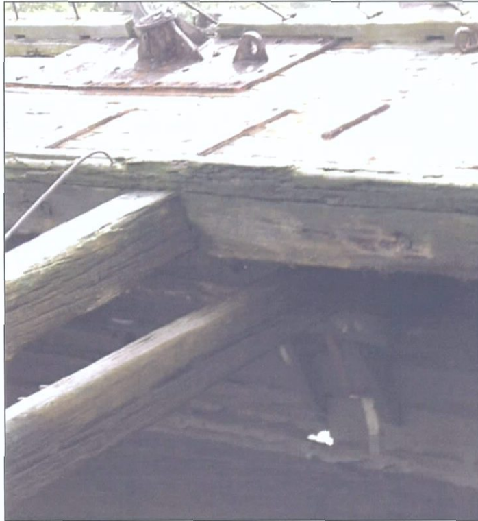
Figure 7-95. Forward davit, starboard side, looking west. Note supporting structure below deck.
