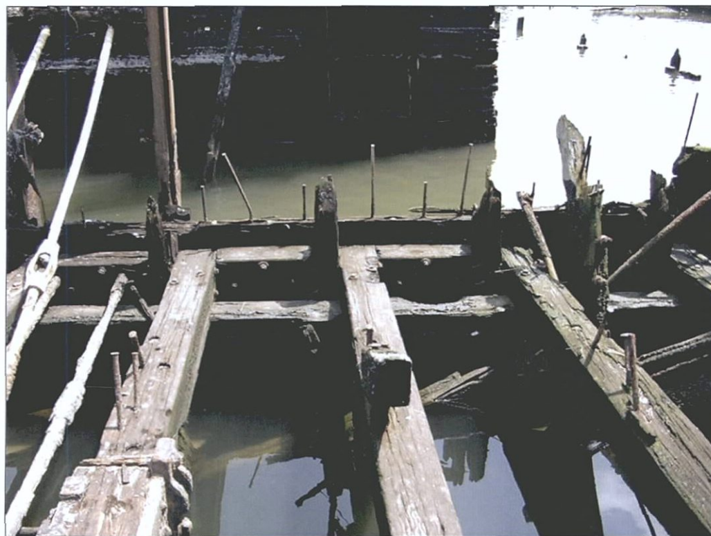
Figure 5-40. Deck beams at starboard side. View to the east.
