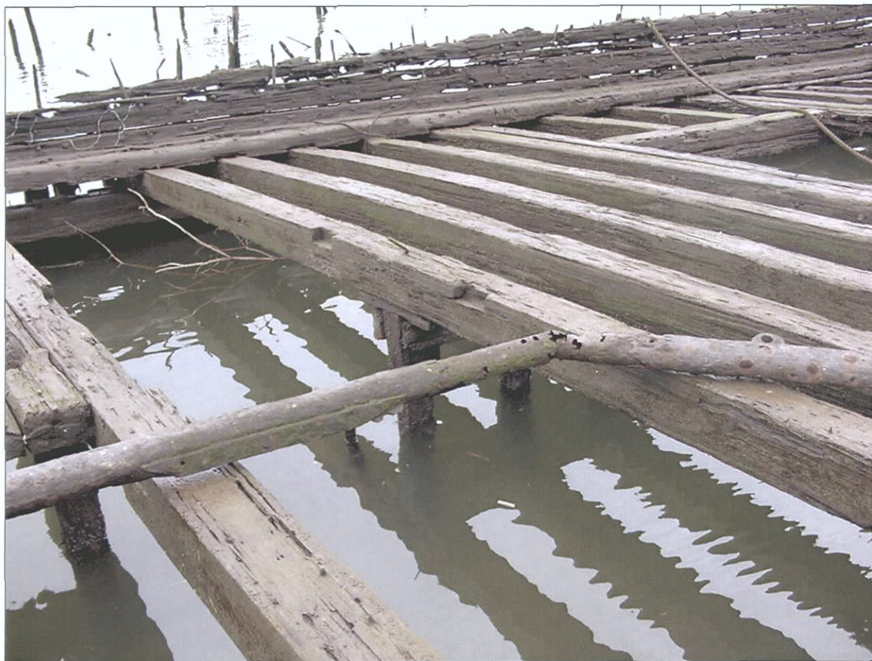
Figure 6-86. Cargo deck midships. View to the west.
