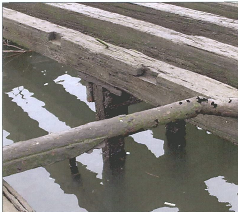
Figure 6-98. Stanchion detail on aft edge of forward cargo hatch. Note presence of stringers, cut just forward of the stanchion, the caps, and the absence of an iron reinforcing strap.
