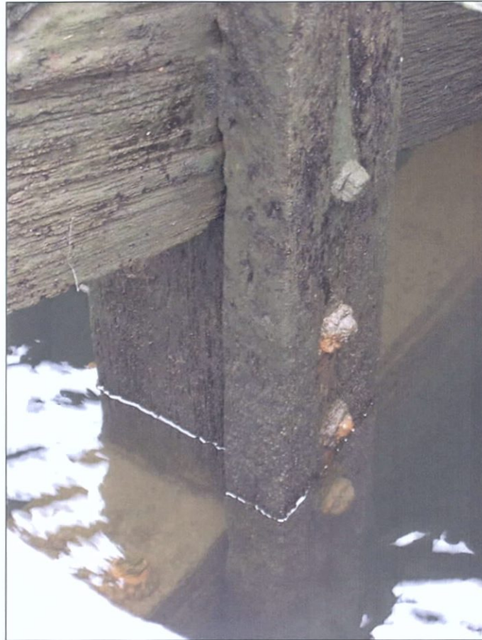
Figure 5-52. Opposite side view of chock between hull trusses.
