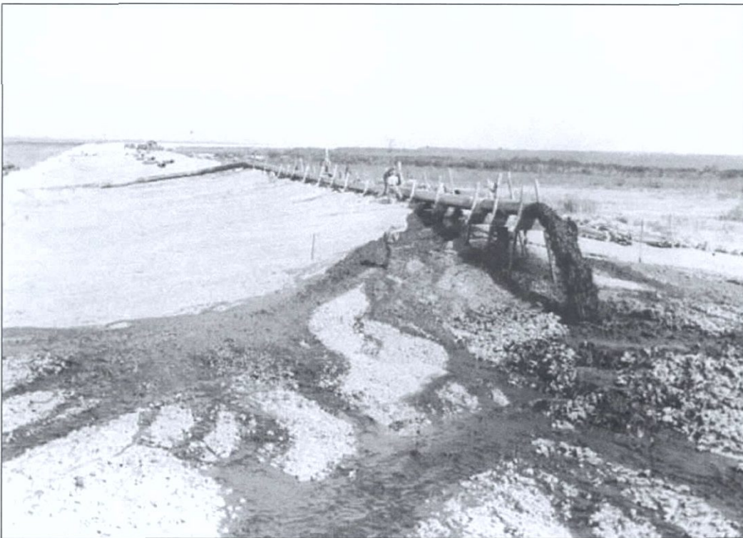
Figure 4-11. Discharge end of discharge pipe, Lake Okeechobee, Florida, circa 1935 (photo courtesy of Florida Photographic Collection).
