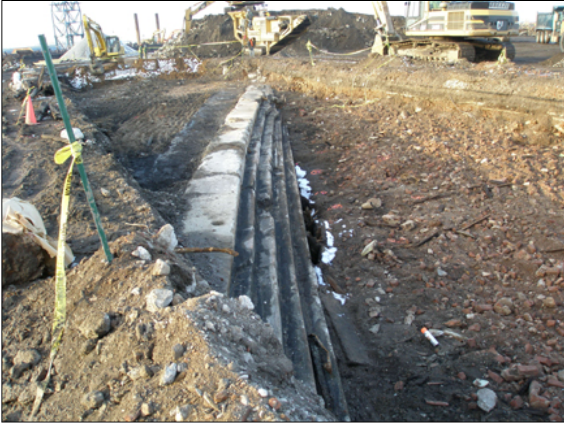
Photo 3.15. Trench 1 Looking North at the East Wall of Graving Dock No. 2. Interior/Eastern Face of East Wall of Graving Dock No. 2 was characterized by Stepped Altars. A circa 1940 electrical conduit runs parallel with the wall along the exterior side.
