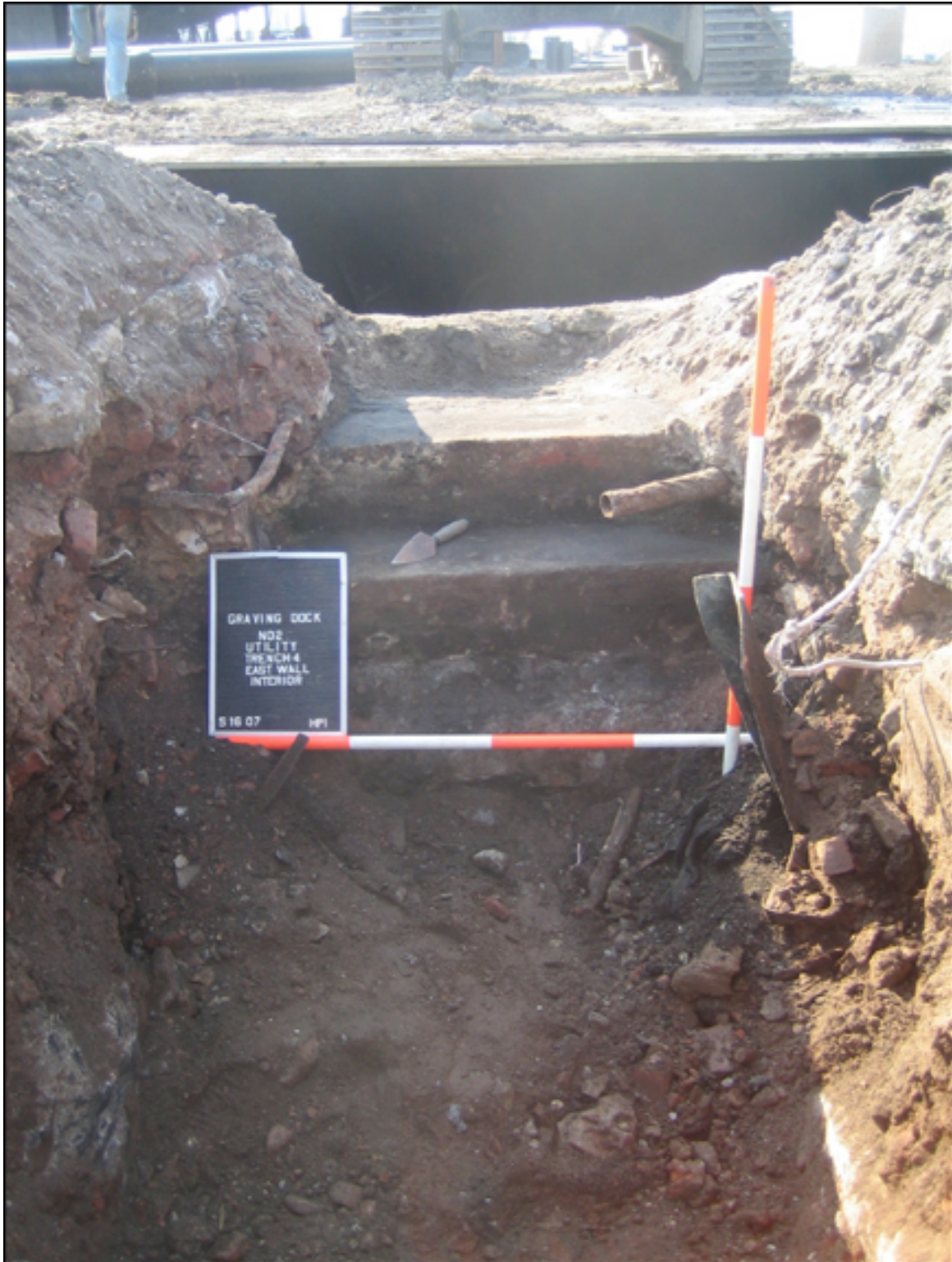
Photo 3.34. Looking southeast toward East Wall of Graving Dock No. 2 Interior (East Profile). Note: Pipe in foreground is within fill. Four stepped altars exposed.
