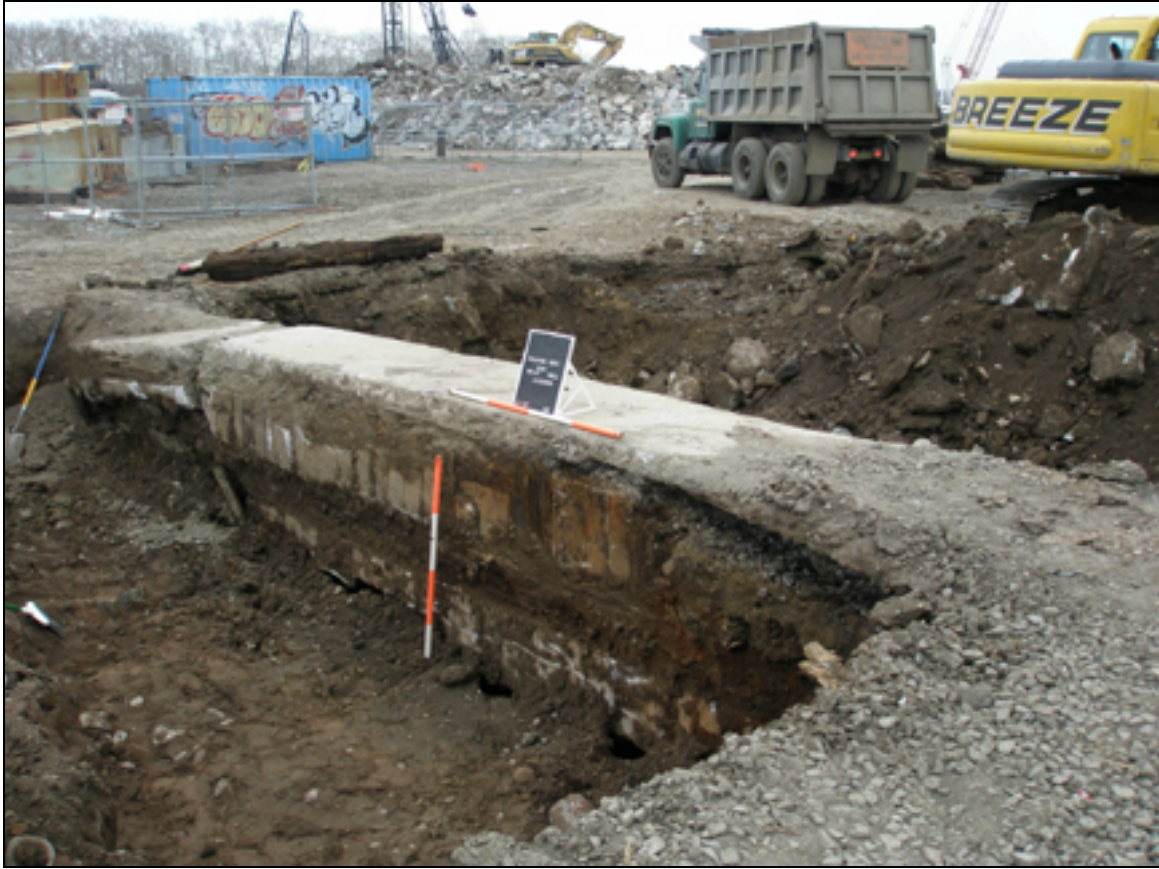
Photo 3.8. Exterior View/East Profile of West Wall of Graving Dock No.2 looking northeast. Wooden forms are visible on the exterior of the wall from the construction of the concrete cap.
