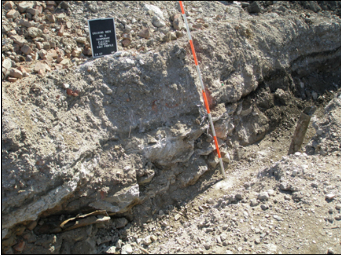
Photo 3.21. Temporary Utility Trench, east profile, after removal of Eastern Wall of Graving Dock No. 2. Note cross section of Eastern Wall of Graving Dock No. 2. The pipe in the foreground is likely located on one of the steps of the dock, as depicted on the 1969 map. The pipe is also seen in the right of the photo, turned upright. Once the wall was removed the trench depth was approximately 5-6 feet deep in this section.
