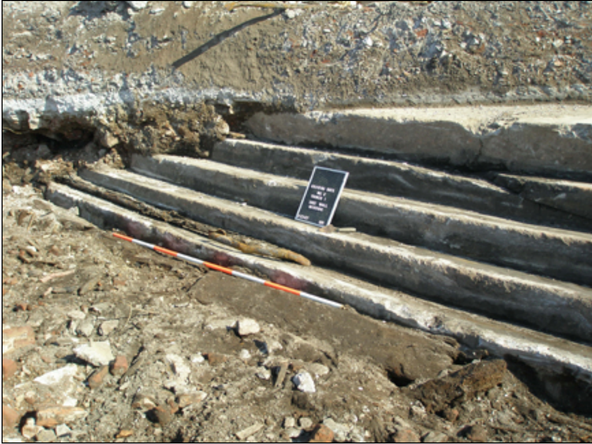
Photo 3.18. Trench 1 Looking Northeast towards East Wall of Graving Dock No. 2. Interior/Eastern Face of East Wall of Graving Dock No. 2 showing remnants of 4-inch pipe located atop Stepped Altar.
