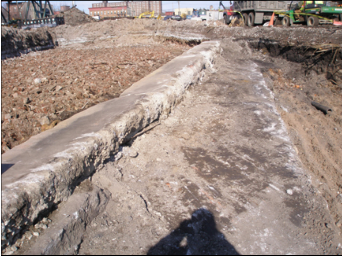
Photo 3.14. Trench 1, Looking North. Exterior/western face of East Wall of Graving Dock No. 2 exposed, though with little detail. A small pipe is visible in the middle ground running out of the wall. A Circa 1940 electrical conduit runs parallel with the wall along its exterior side, separated by a compact clay.
