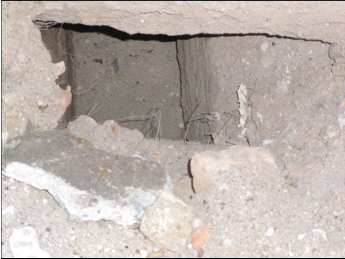
Photo 3.5. Void along eastern face of Eastern Wall of Graving Dock No. 2. Horizontal wooden elements are visible below the poured concrete cap.
