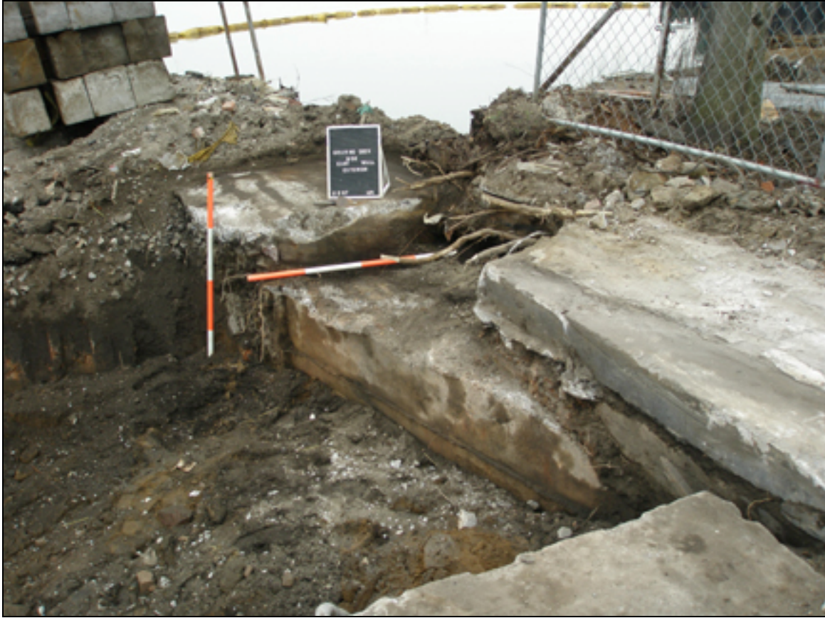
Photo 3.2. View of intact graving dock elements/Erie Basin looking southwest from Electrical Vault. East Wall of Graving Dock No. 2 is manifest as poured concrete. The Caisson Gate is just beyond the concrete on the right, out of view.
