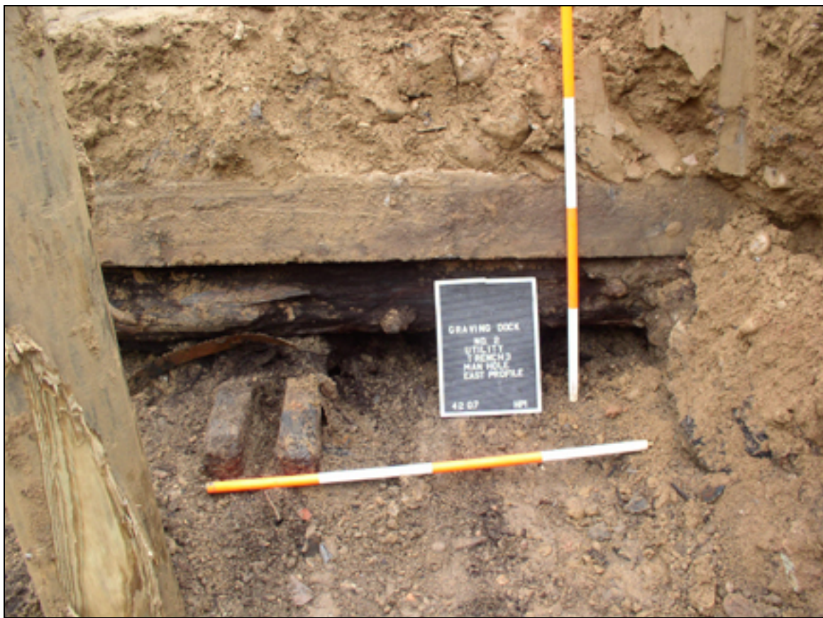
Photo 3.28. Close up of southernmost portion of Manhole Box, East Profile of Utility Trench 3, showing exposed wooden elements of East Wall of Graving Dock No. 2.
