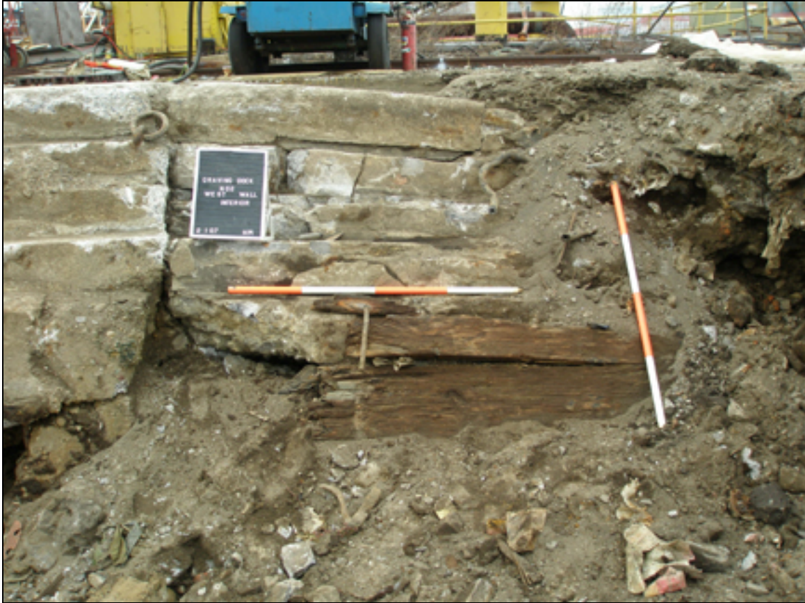
Photo 3.11. Interior View/West Profile of West Wall of Graving Dock No. 2 within Bulkhead Trench. Wooden sheeting connected to concrete cap by iron ties. The concrete cap is cracked and slumping towards the north. Iron ring located on second Stepped Altar on left side of photo.
