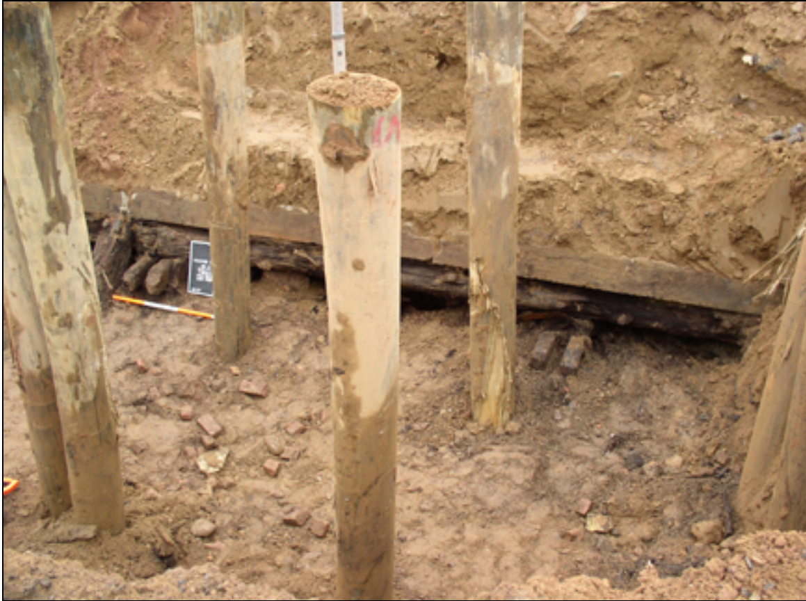
Photo 3.27. East Profile of Utility Trench 3, Manhole Box, showing exposed wooden elements of East Wall of Graving Dock No. 2.
