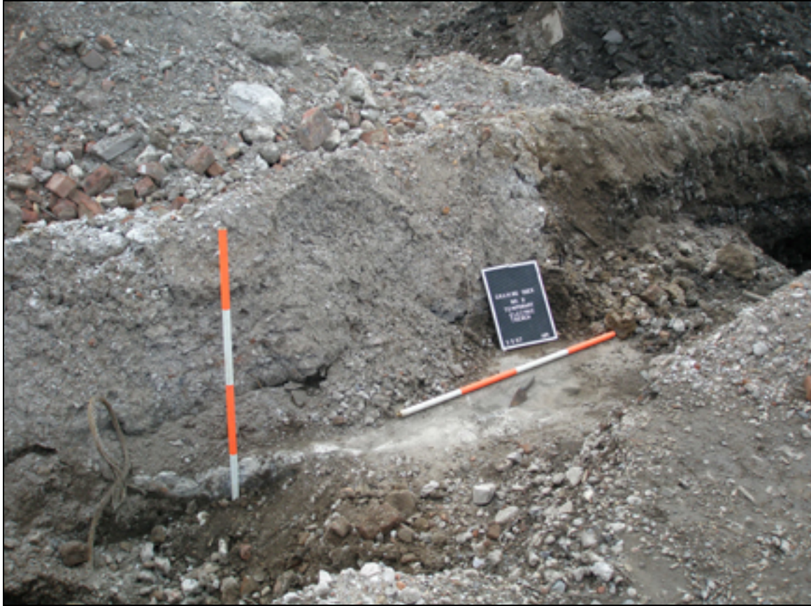
Photo 3.19. Temporary Utility Trench looking southeast. Note uncovered interior edge of Eastern Wall of Graving Dock No 2 (poured concrete). Top of dock was approximately 2.5 feet below grade.
