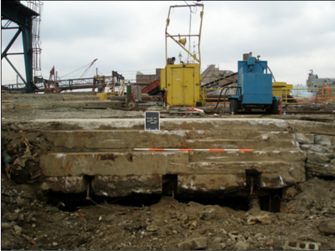
Photo 3.10. Interior View/West Profile of West Wall of Graving Dock No. 2 within Bulkhead Trench. West Wall of Graving Dock No. 2 is composed of poured concrete overlying and supported by wooden piles. The piles are connected to the concrete cap by iron ties. Much of the wood is rotting away. The concrete cap is slumping towards the north. Iron rings are located along the second altar on the dock, visible on the right hand side of the photo and to the right of the photo board.
