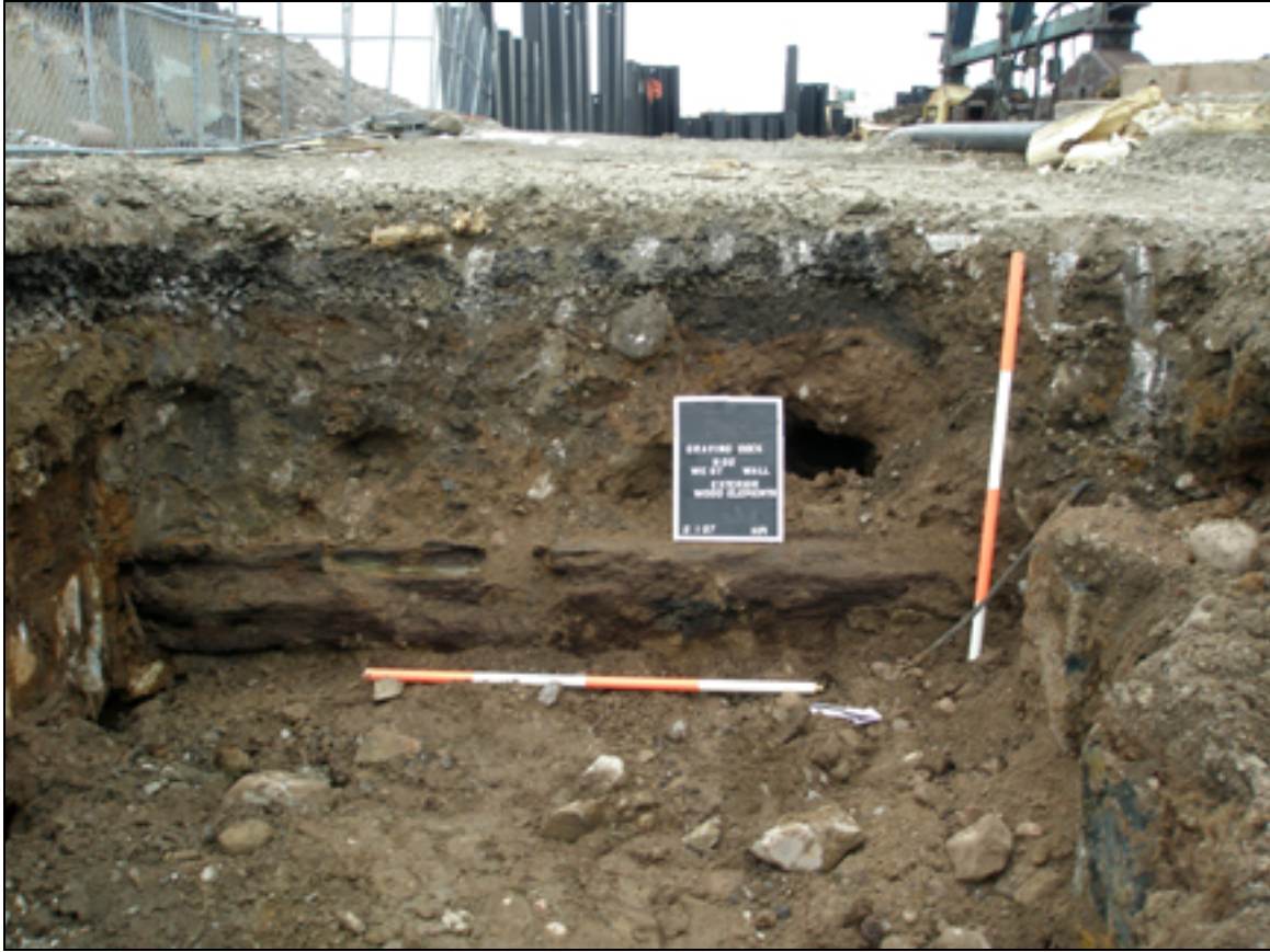
Photo 3.9. South profile of 15-Foot Apron along the western side of the West Wall of Graving Dock No. 2. Horizontal wooden element running from the graving dock (left of photo) northwest. A perpendicular wooden element was located above the visible horizontal wooden element within the void partially obscured by the photo board. The perpendicular wooden element was located within the fill episode overlying the visible wooden element.
