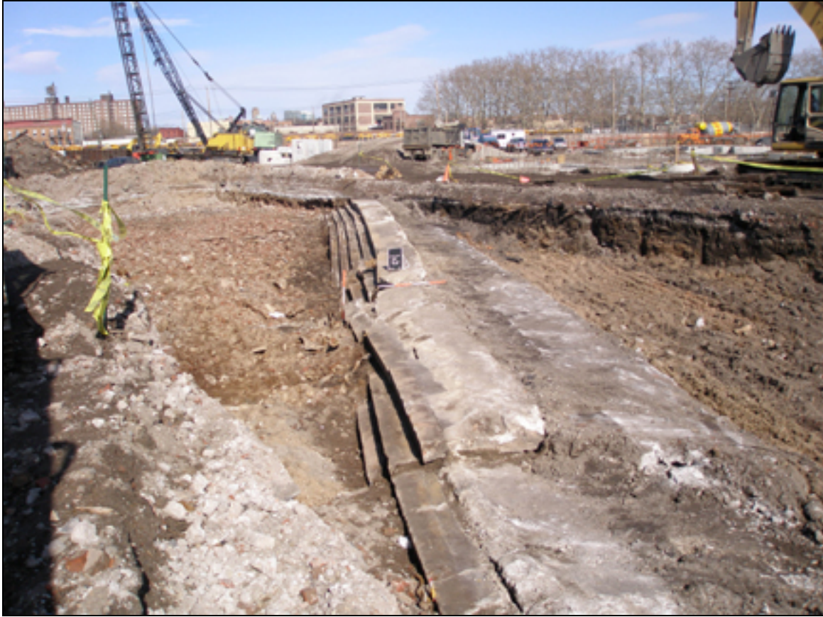
Photo 3.13. Trench 1 Looking Northeast towards East Wall of Graving Dock No. 2. Interior/Eastern Face of East Wall of Graving Dock No. 2 was characterized by Stepped Altars. A circa 1940 electrical conduit runs parallel with the wall along the exterior side.
