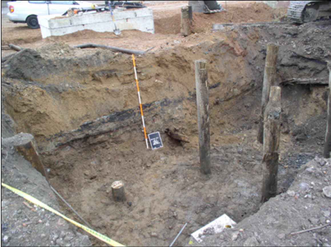
Photo 3.24. Western Profile of Manhole Box cut within Utility Trench 2 looking northwest. Note: Circa 1940s electric duct is located above wooden element. No visible cuts or associated features were identified with the wooden element. Vertical piles in the foreground were driven to support the manhole box.
