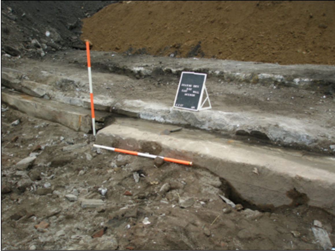
Photo 3.4. Looking Northeast toward Eastern wall of Graving Dock No. 2 within Bulkhead Trench/15-Foot Apron. Intact elements of the East Wall of Graving Dock No. 2 were composed of poured concrete. The steps of the wall are known as Stepped Altars. A void opened along the face (lower right hand corner of photograph) and wooden supports were identified (see Photo 3.5).
