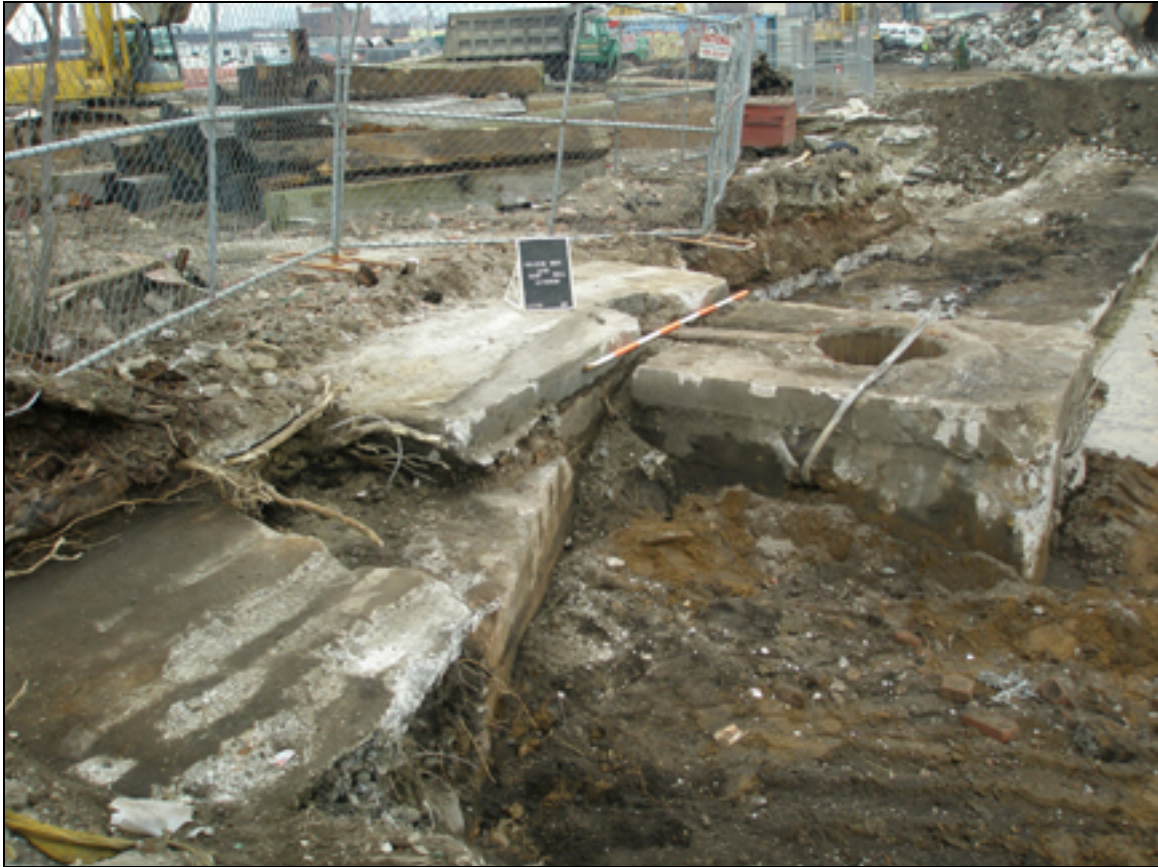
Photo 3.1. Bulkhead Trench/15-Foot Apron, Looking Northeast. Electrical vault and related conduit are located on the right hand side of the photo. The intact graving dock elements are manifest as poured concrete and appear on the left hand side, on or above grade. The electrical vault is connected to the graving dock by metal pipes.
