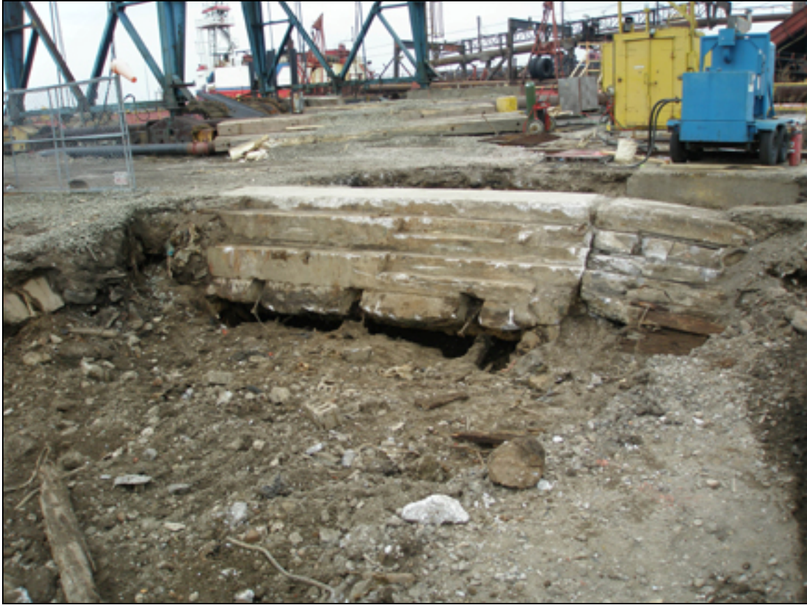
Photo 3.7. West Wall of Graving Dock No. 2 within Bulkhead Trench/15-Foot Apron looking southwest. The West Wall is composed of poured concrete Stepped Altars overlying and supported by wooden piles. Wooden sheeting is visible on the right hand side of the photo, attached to the concrete cap by iron ties. The wooden elements of the dock had largely been destroyed or were in the process of rotting away.
