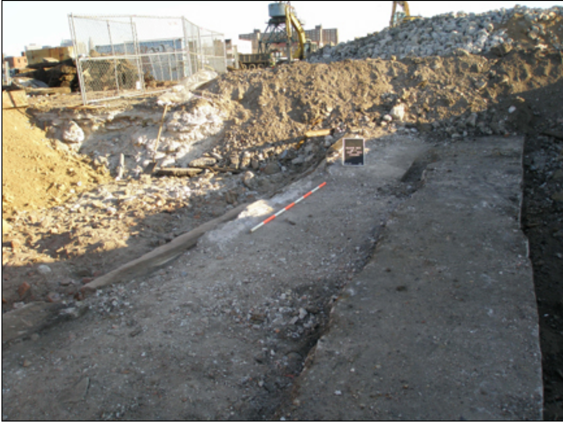
Photo 3.6. Looking northeast along the East Wall of Graving Dock No. 2 and electrical conduit within Bulkhead Trench/15-Foot Apron. The east wall was likely compromised during filling in the 1970s and further altered during monitoring/soil remediation. The electrical conduit is located on the right hand side of the photo and the East Wall on the left. Eight-inch pipe removed prior to photo.
