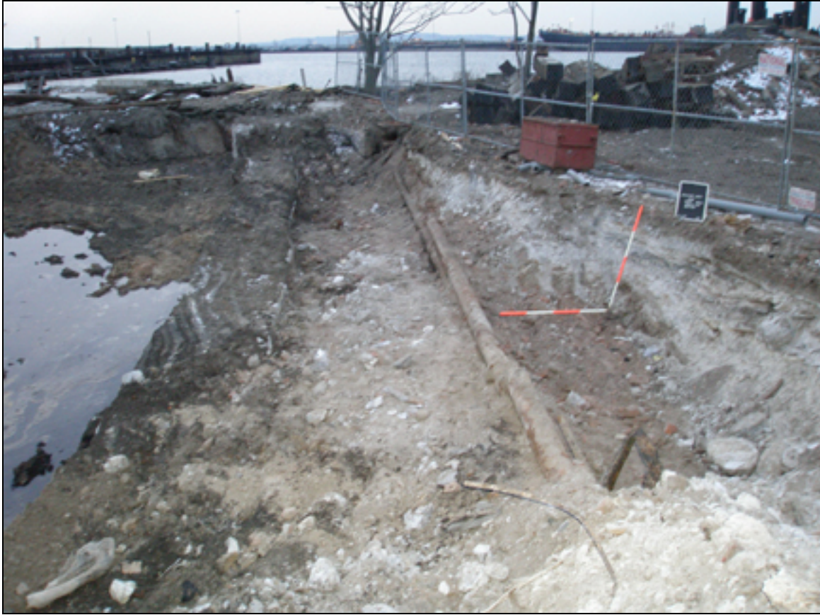
Photo 3.3. Southeast view of Bulkhead Trench/15-Foot Apron. Two eight-inch pipes run along the eastern wall of the graving dock (right hand of photo) parallel with an electrical conduit (left hand of photo). The pipes were laid on the Stepped Altars of the dock.
