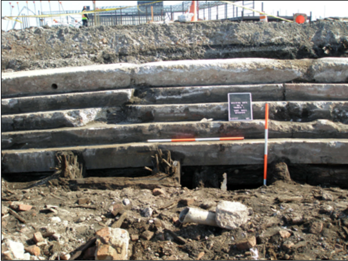
Photo 3.17. Trench 1 Looking Southeast towards East Wall of Graving Dock No. 2. Interior/Eastern Face of East Wall of Graving Dock No. 2 overlaid horizontal wooden elements with “pulled” iron ties. The horizontal wooden elements and concrete cap were attached to vertical wooden elements with additional “pulled” iron ties.
