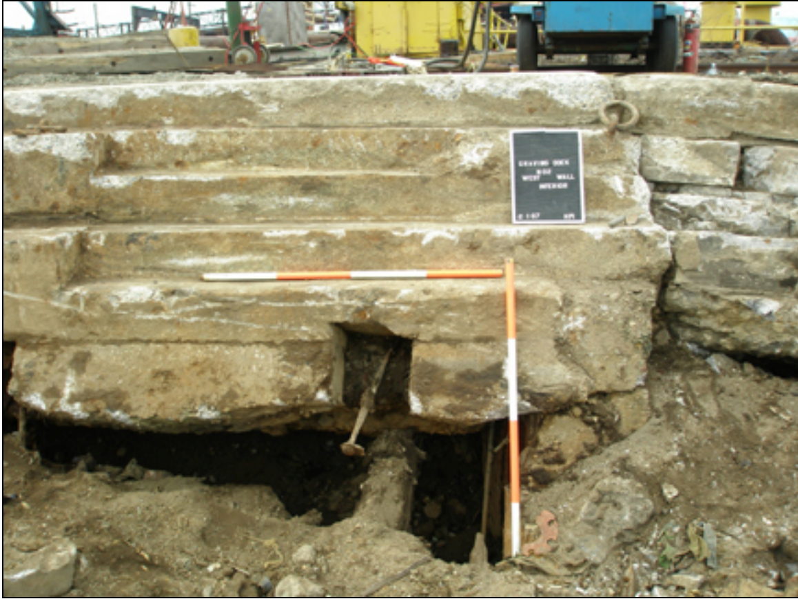
Photo 3.12. Interior View/West Profile of West Wall of Graving Dock No. 2 within Bulkhead Trench. Note iron tie protruding from the cut on the lower Stepped Altar of the concrete cap. The tie once intersected the rotting wooden pile behind. Metal sheeting is running into the fill and supporting the concrete cap just to the right of the pile, and left of the vertical range pole.
