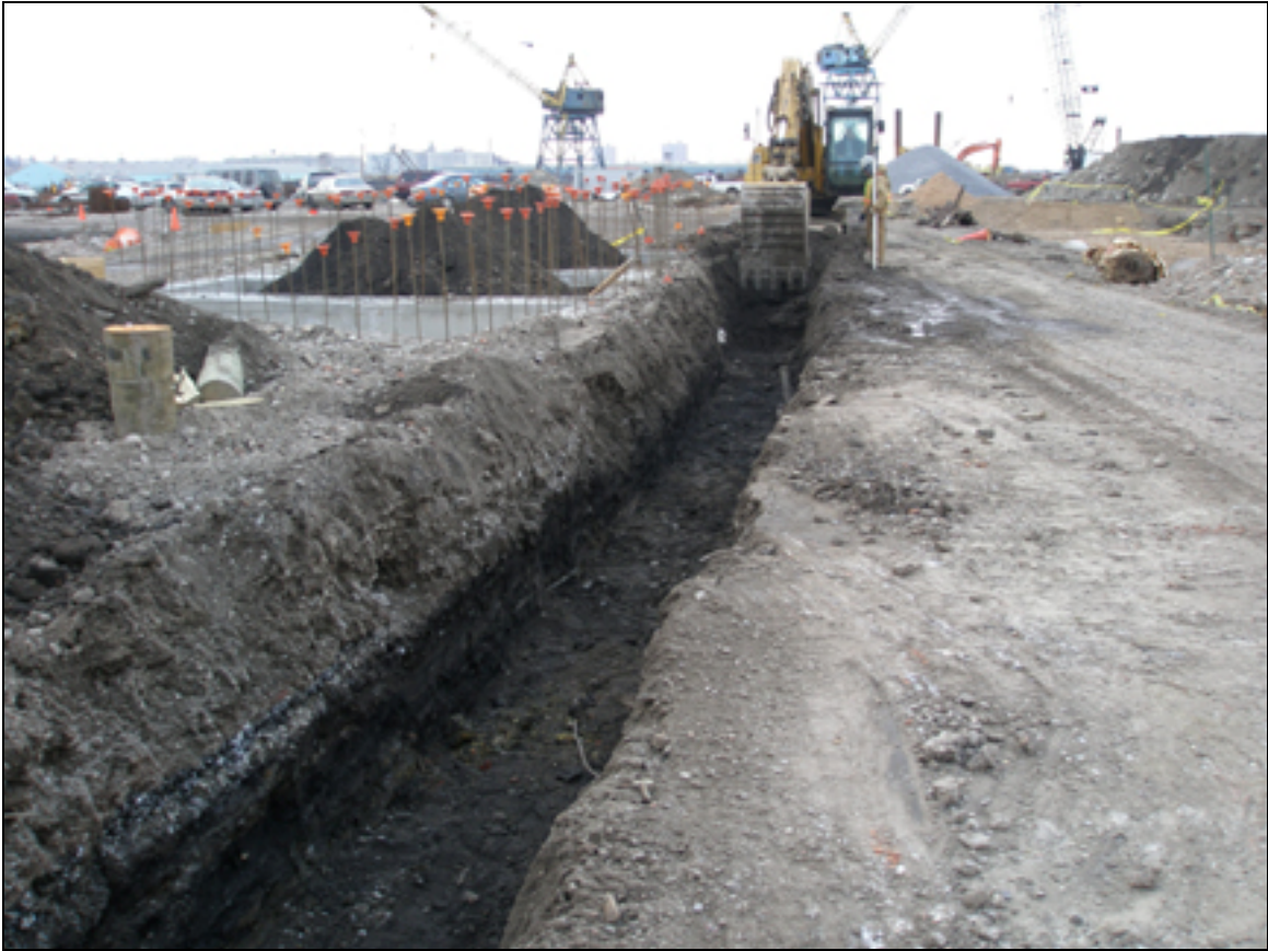
Photo 3.20. Temporary Utility Trench looking south from Eastern Wall of Graving Dock No. 2. Trench depth in this section was approximately 4 feet below grade, later taken to 5 feet below grade.
