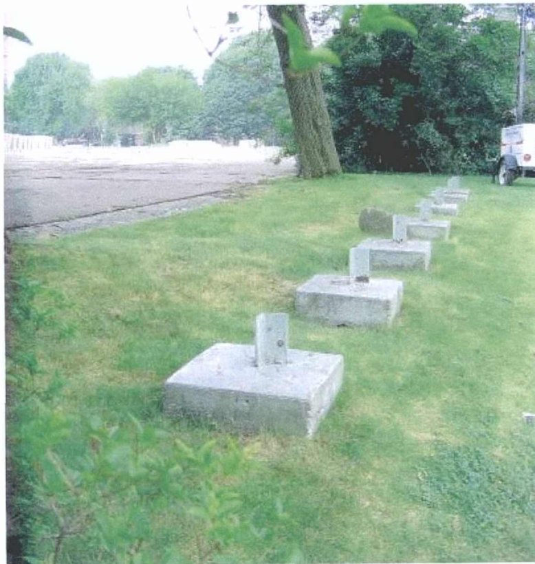
Photo 8 Concrete fence footings on the northern side of the tennis courts, facing southwest (July 7, 2008).
