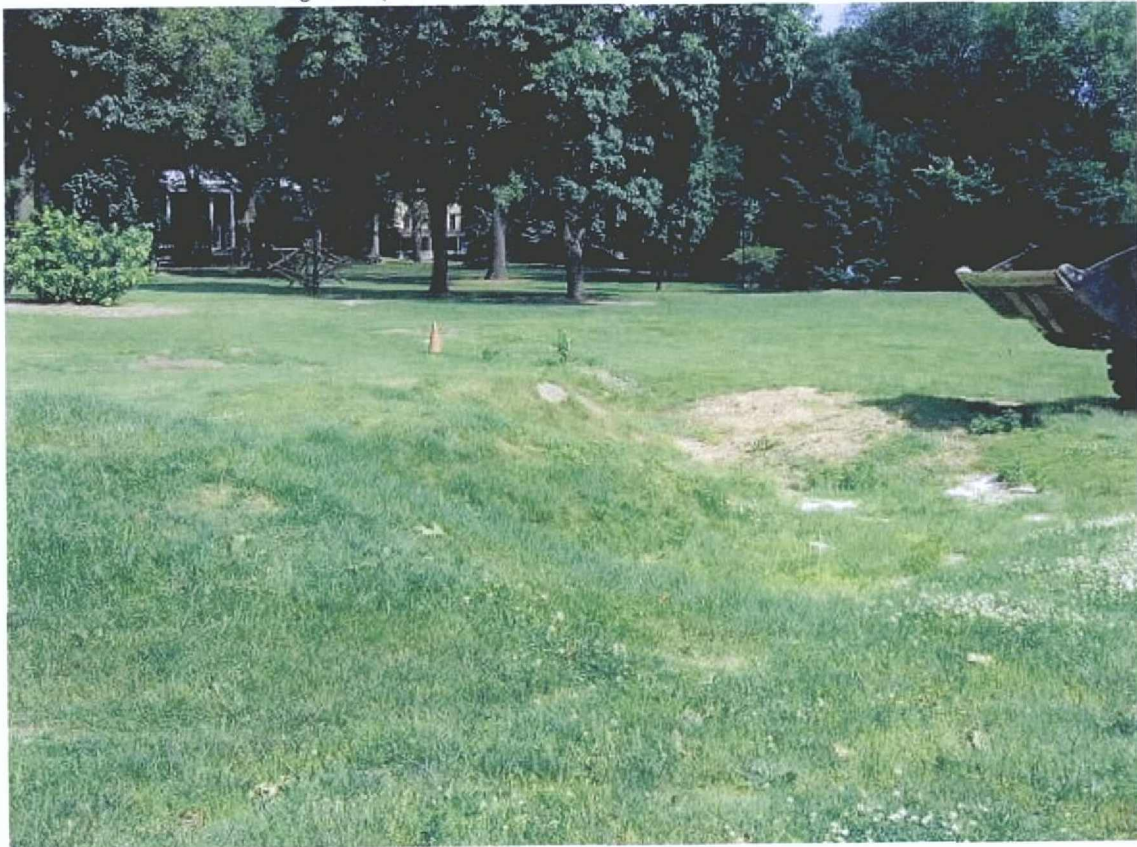
Photo 4 Grading Area 8 prior to excavation, facing southeast (June 11, 2008).
