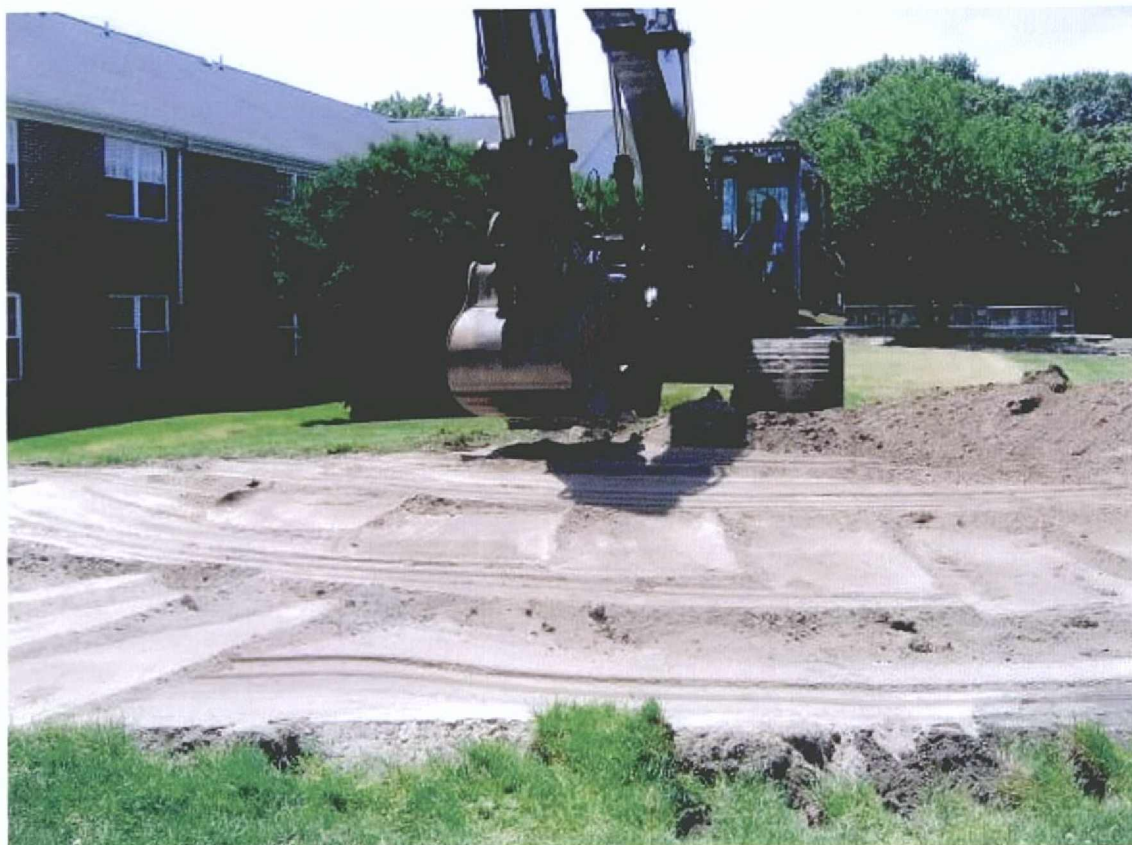
Photo 2 Grading Area 1 excavations nearly completed (June 11, 2008).
