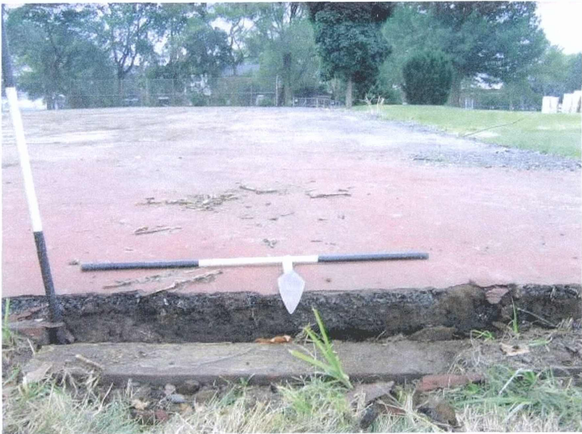
Photo 7 Layers of asphalt and concrete exposed above the ground surface prior to excavation, facing south (July 7, 2008).
