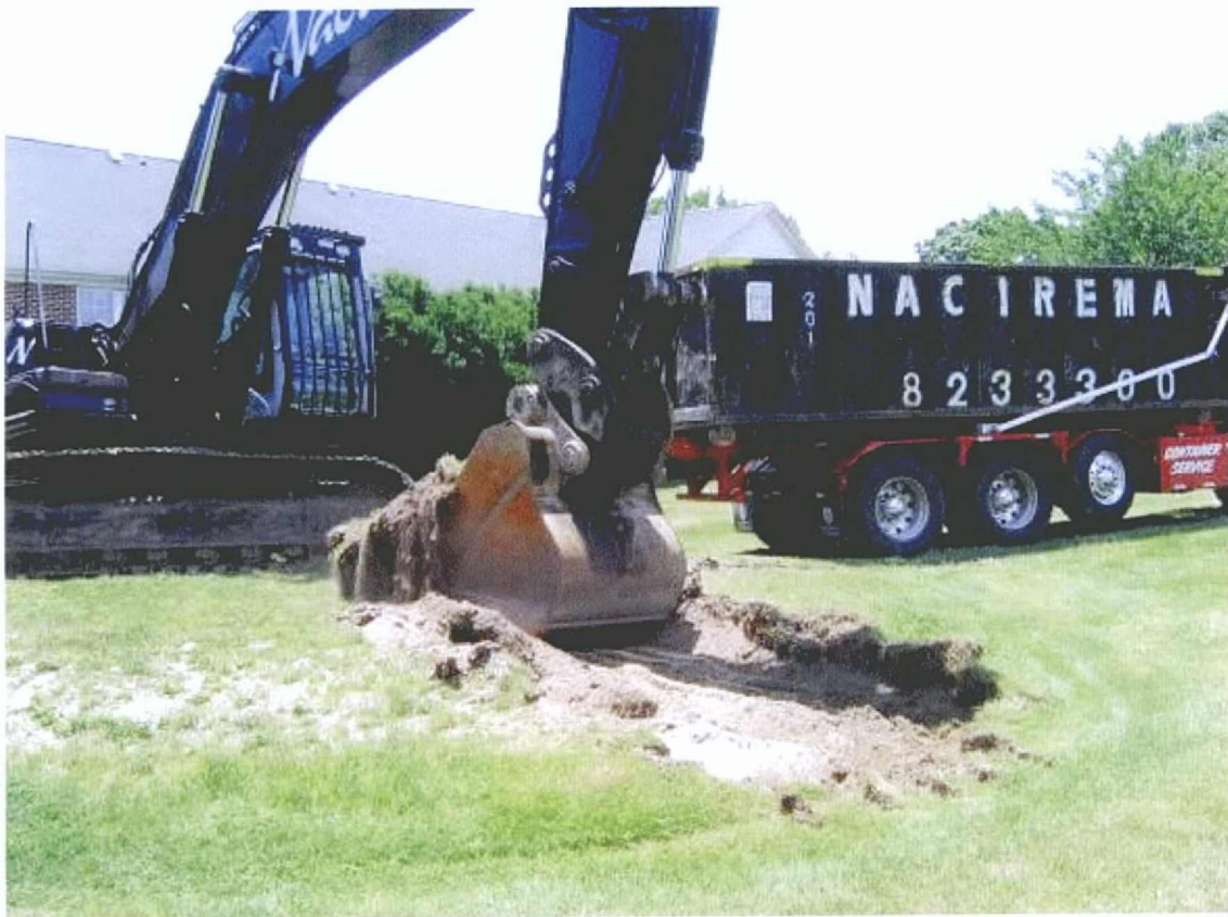
Photo 1 Excavation at Grading Area 1 underway (June 11, 2008).
