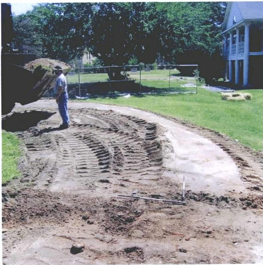
Photo 3 Grading Area 4 showing demolition debris with 3-foot scales, facing east (June 11, 2008).
