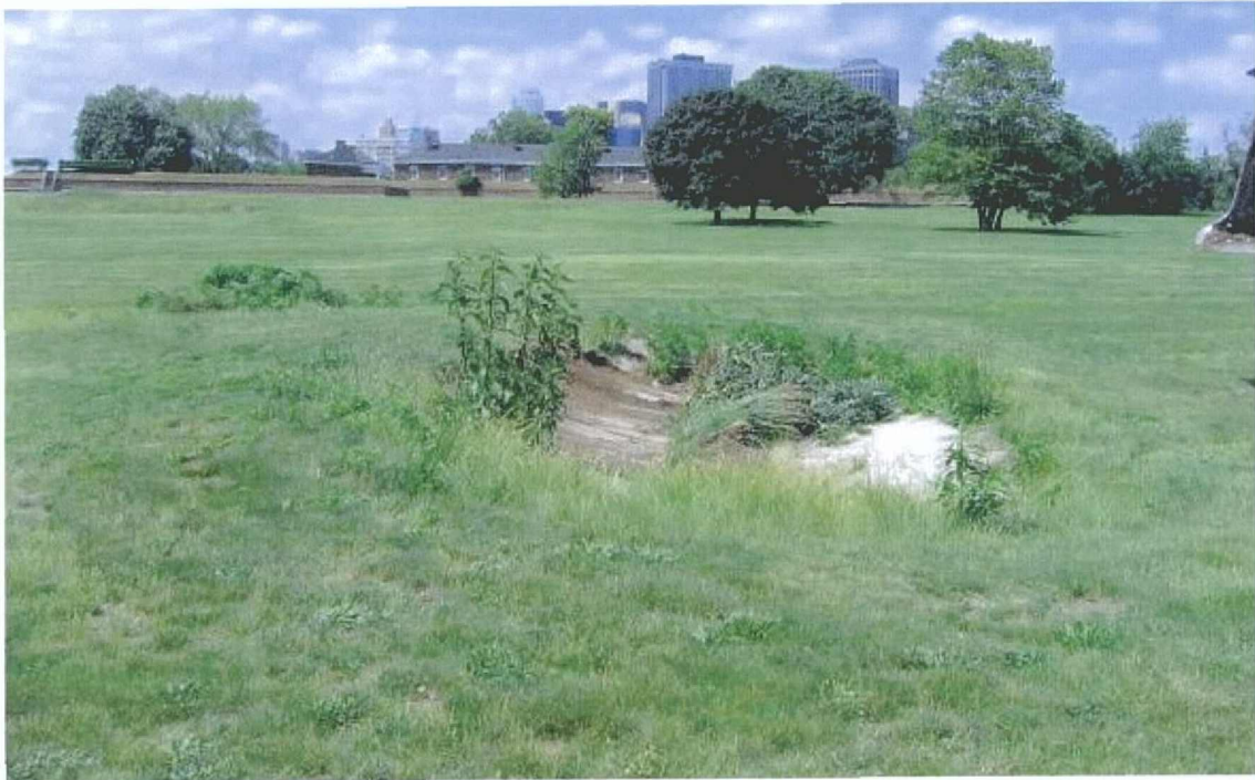
Photo 5 Grading Area 9 prior to excavation, facing northeast (June 11, 2008).
