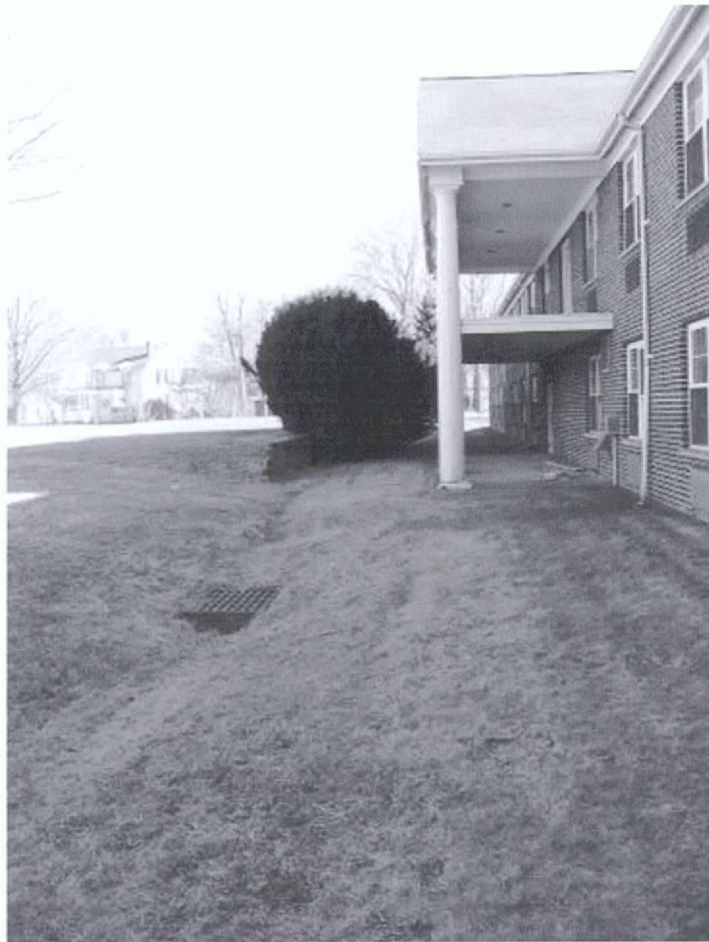
Photo 1 View behind Building #293 facing east showing a depression in the ground due to an existing drainage line which will be filled.
