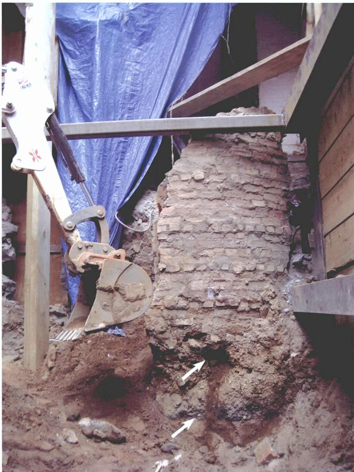
6 Cistern wall exposed in the southwest corner of the yard where a frame overhang is depicted on early maps (see Figure 2). The approximately 7.5-foot deep and 7-foot diameter cistern, constructed from the inside-out, displays a random pattern of header and footer bricks. A thick layer, possibly stones and tar, was located under the cistern (upper arrow) and a deeper layer (lower arrow), under rocky soil, was found throughout the yard. (Geismar 12/8/08)
