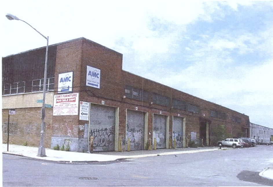
SITE 41 - BLOCK 2538 looking southwest along India Street (above) and looking south along West Street (below)
