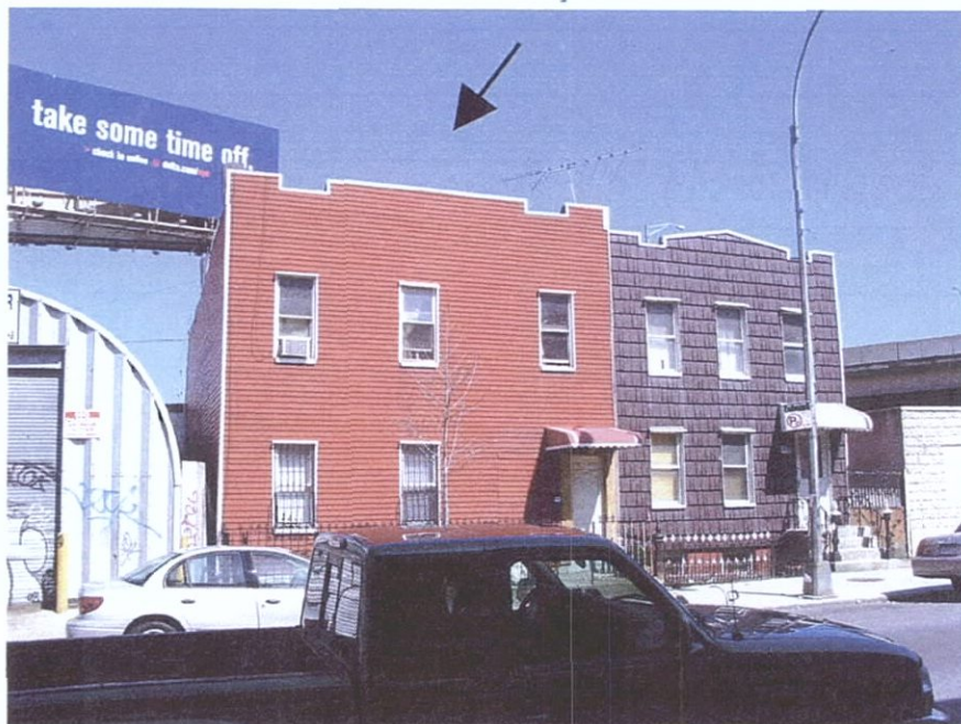
SITE 137 - BLOCK 2733 from Leonard Street (above), and from Meeker Avenue (below)
