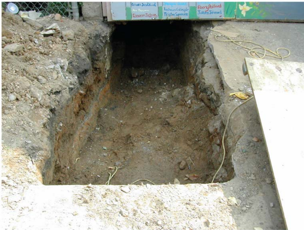
14 Test trench 11 (TT11) under and in front of the garage located east of 1698 Bergen Street. Trench was excavated to find evidence of old Hunterfly Road, but none was found. (Geismar 8/21/2003)
