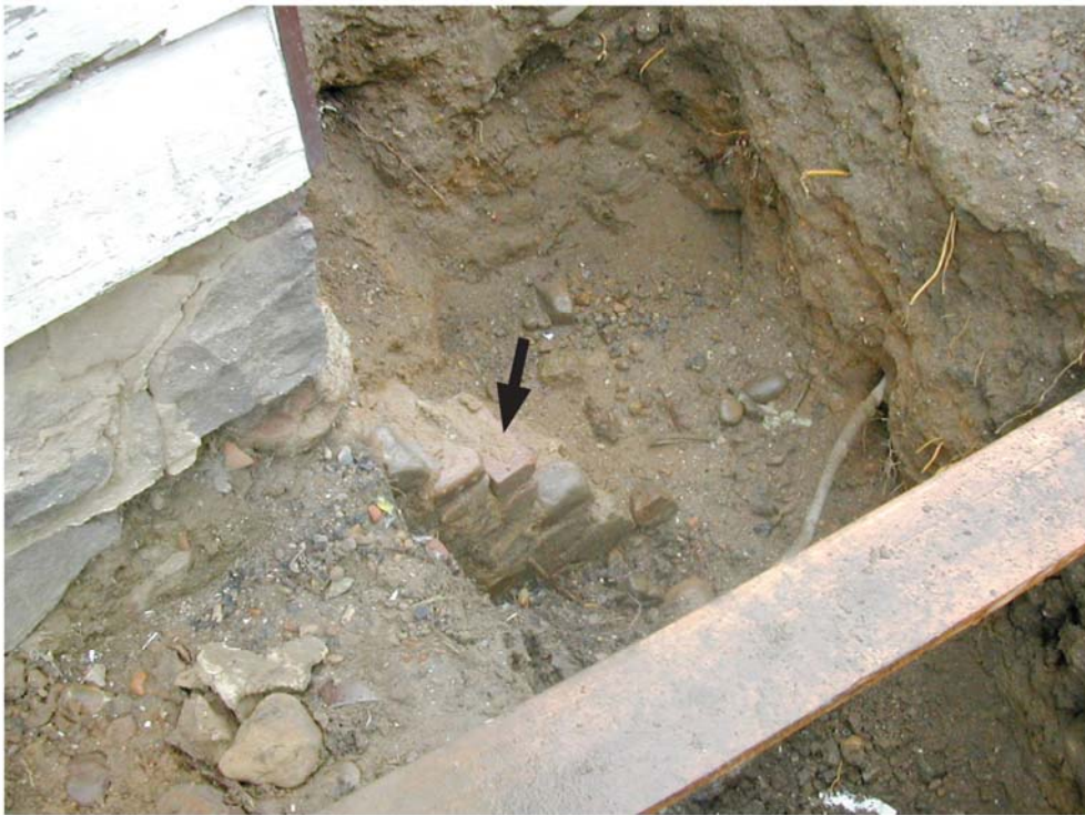
57 Northwest corner of 1700 Bergen Street with remnant of demolished outdoor toilet superstructure (arrow) exposed during reconstruction. (Geismar 2003)
