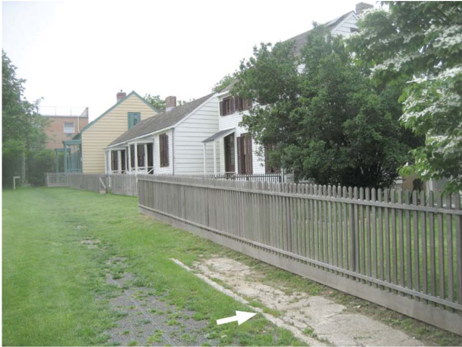
8 Three of the four Hunterfly Road houses after recent restoration (1698 Bergen Street, the fourth house in the cluster, is to the right beyond the trees). View is south. Note sidewalk and curb (arrow) of former Hunterfly Court exposed during restoration work. (Geismar 6/6/2008)
