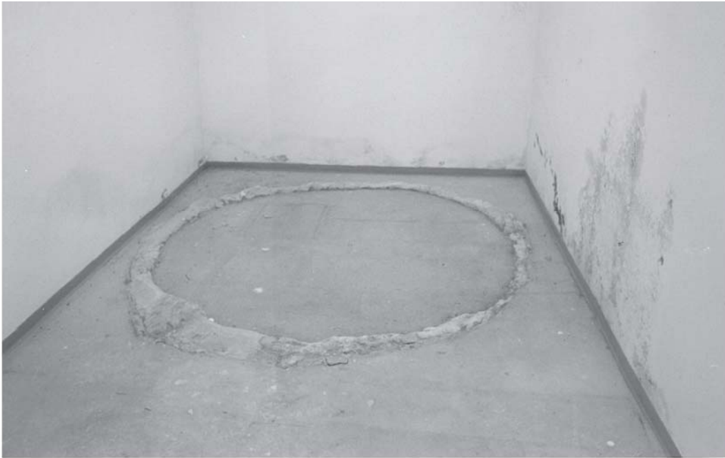
58 Mortared stone “ring” in the basement of 1706-1708 Bergen Street, the remnant of a former 5.5-ft. diameter water cistern removed when the basement was extended in 1980. (Geismar 2000)
