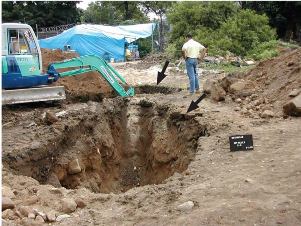
13 Two dry wells (arrows) under excavation east of the Hunterfly Road houses in 2003. (Geismar 8/11/2003)
