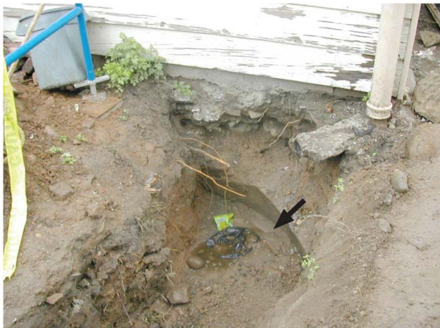
61 Northern edge of Feature C (FC), the large truncated cistern located between 1698 and 1700 Bergen Street (arrow). The back wall (southeast corner) of the 1698 Bergen Street extension is adjacent to the cistern. A lightwell was reintroduced above the cistern's edge in 2003. (Geismar 2002)
