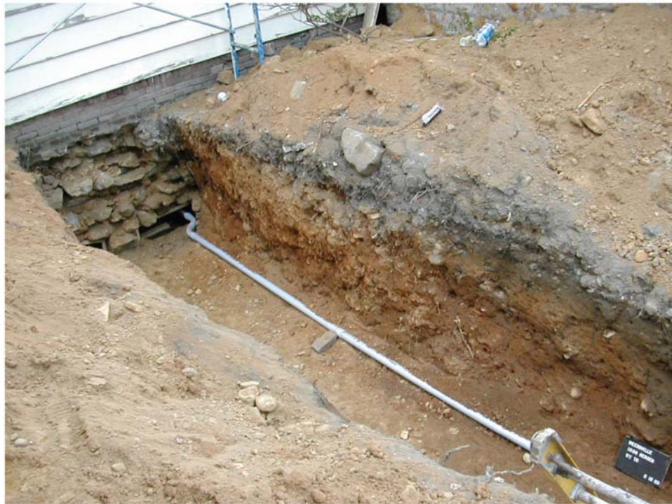
12b West end of east-west utility trench (UT) and exposed foundation of 1698 Bergen Street just north of rear extension. (Geismar 5/15/2003)
