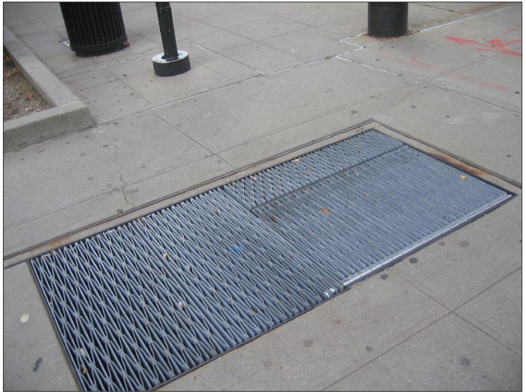
Transformer vault in sidewalk along western side of Rutgers Slip 1
