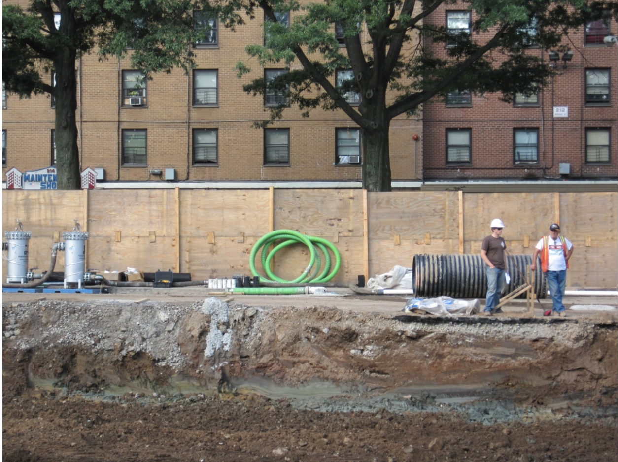
Image 21: Zone 2 note layer of greenish clay in the trench wall
