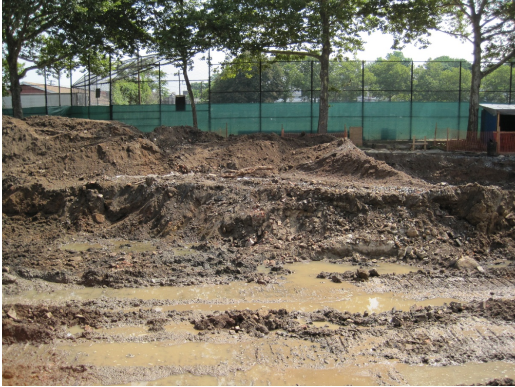
Image 30: groundwater seepage throughout the excavation trench
