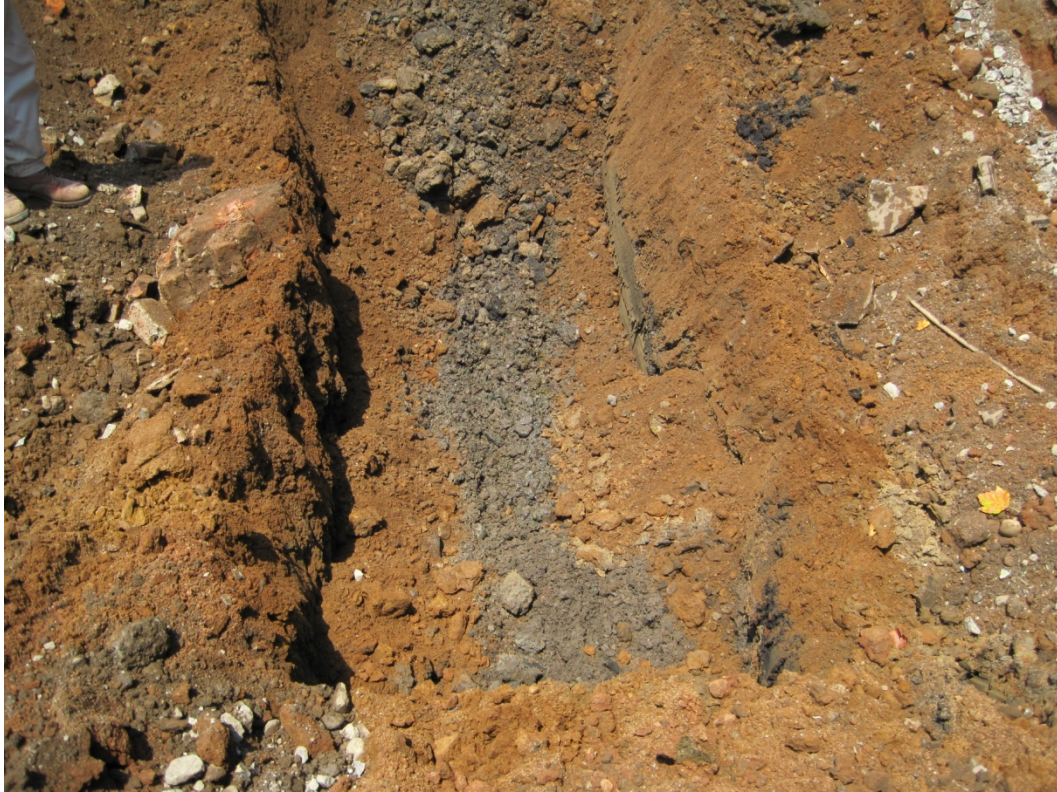
Image 26: construction rubble mixed throughout the excavation trench
