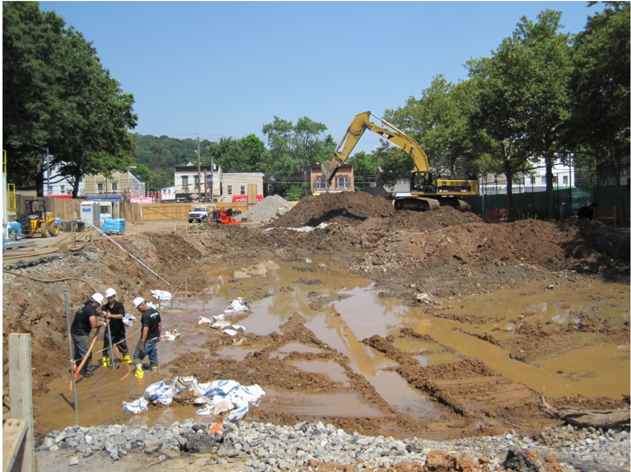
Image 06: Installation of the dewatering system
