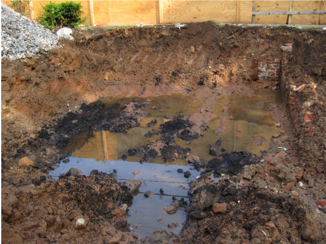
Image 33: groundwater seepage throughout the excavation trench
