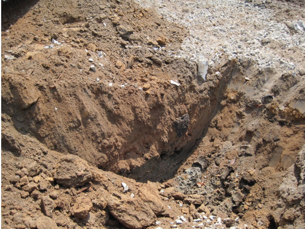
Image 24: construction rubble mixed throughout the excavation trench
