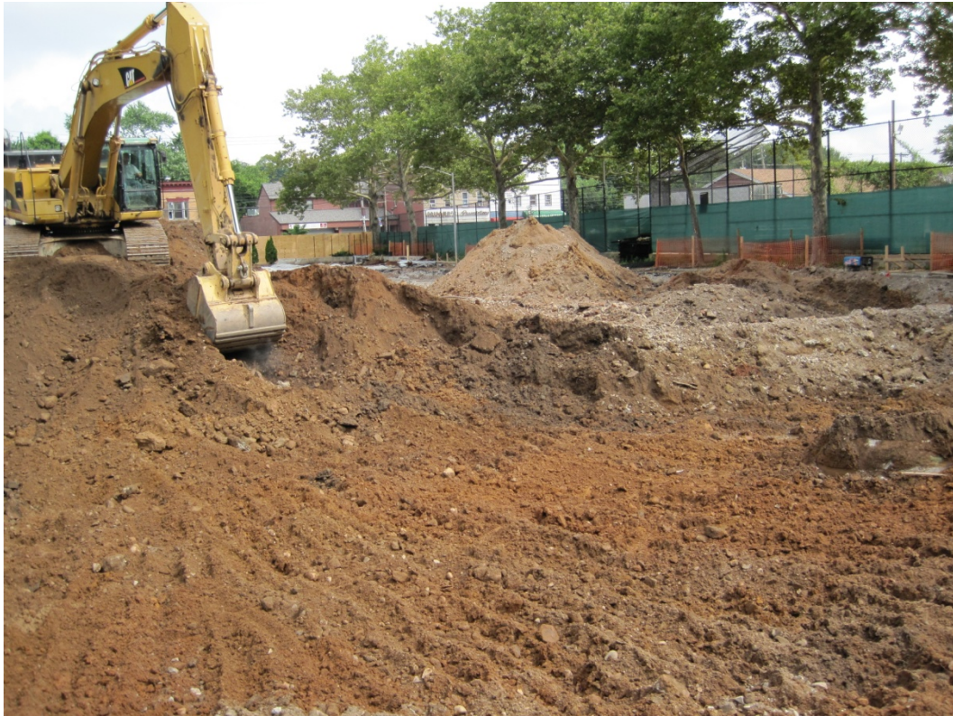
Image 28: construction rubble mixed throughout the excavation trench
