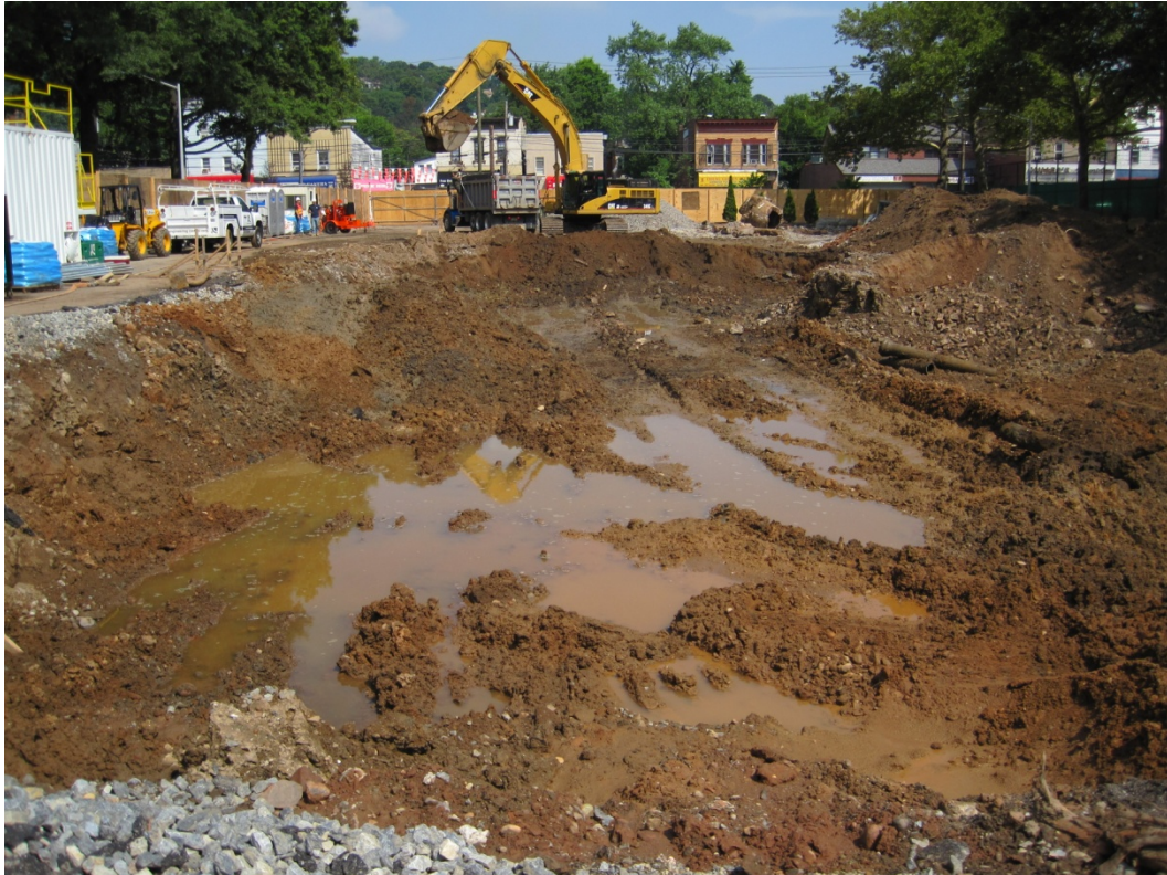
Image 31: groundwater seepage throughout the excavation trench
