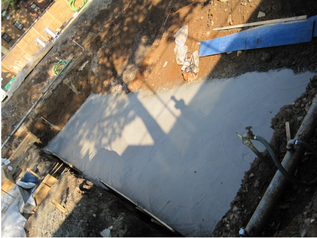
Image 36: concrete foundation floor installation
