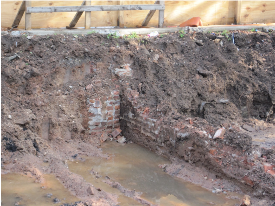
Image 32: groundwater seepage throughout the excavation trench
