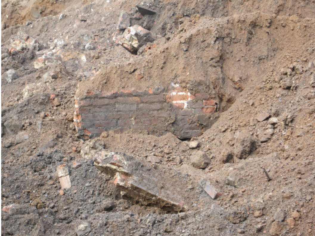
Image 16: Zones 1 to 2 broken portion of foundation wall
