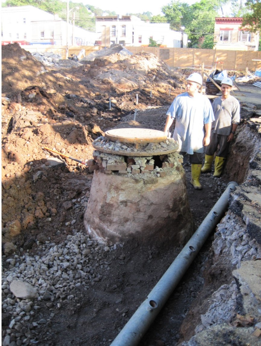
Image 13: Zone 4 non-functioning sewer
