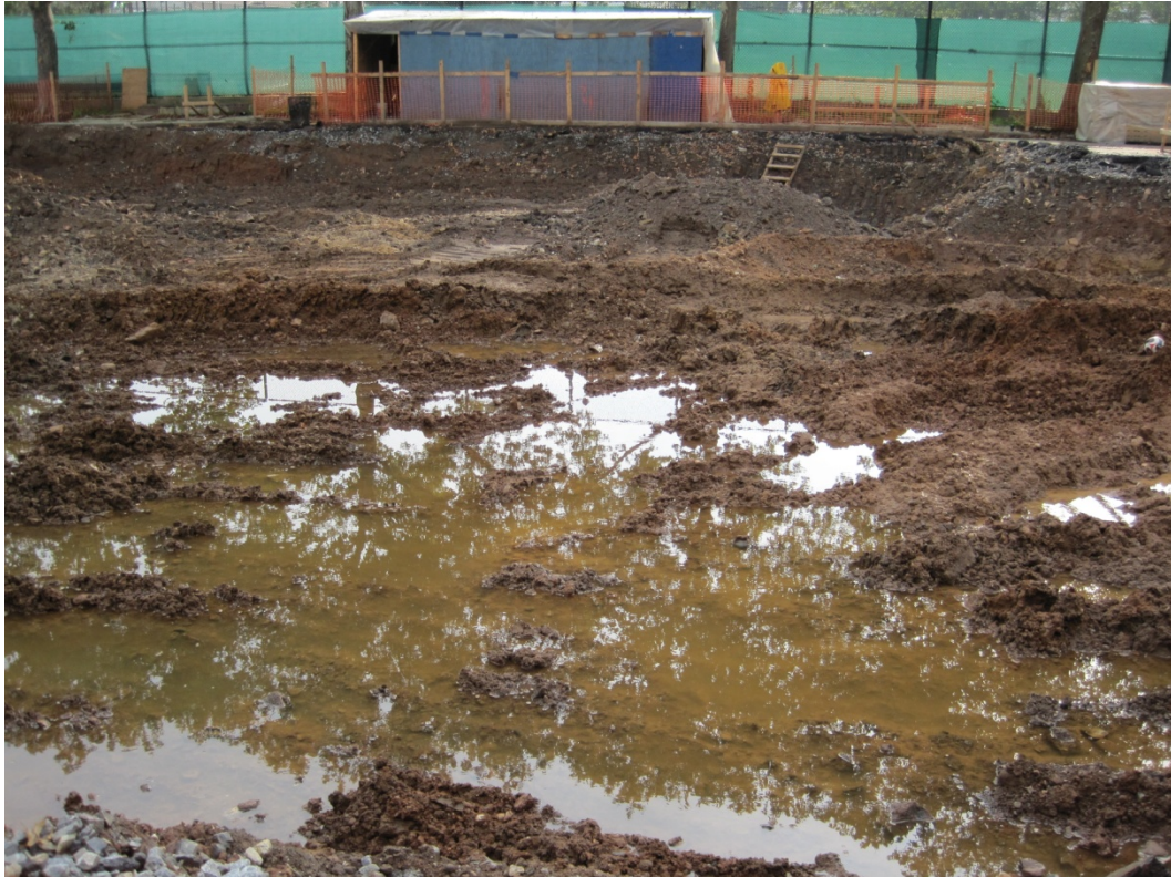
Image 29: groundwater seepage throughout the excavation trench
