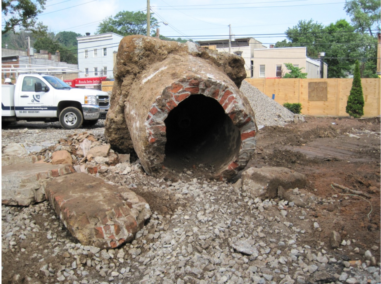
Image 14: Zone 4 non-functioning sewer shaft removed
