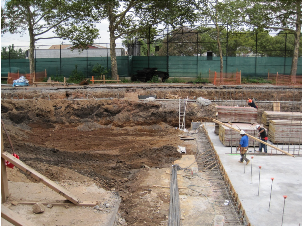
Image 37: concrete foundation floor installation
