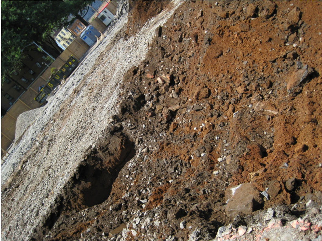
Image 25: construction rubble mixed throughout the excavation trench
