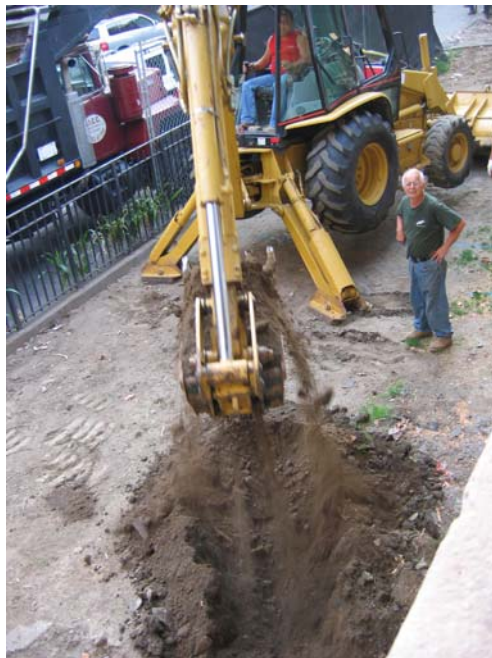
Photograph 10: Excavation of soil in the area east of the stairway
