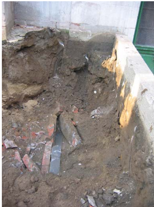
Photograph 14: Uncovering of brick foundation wall
