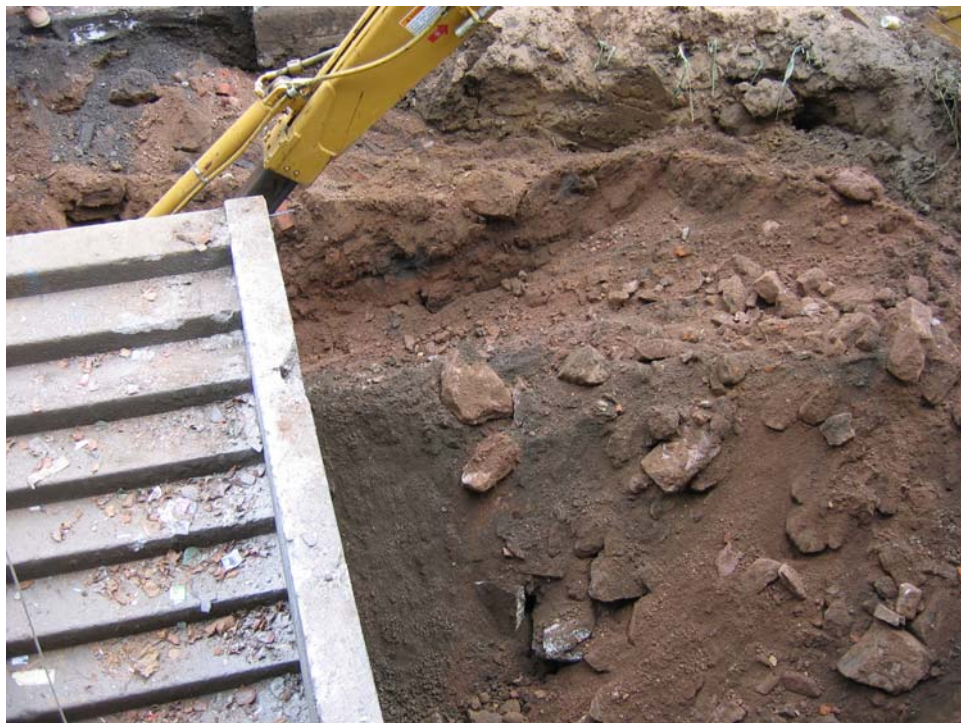
Photograph 36: Columbus Park Pavilion - Brick Foundation Wall Removal
