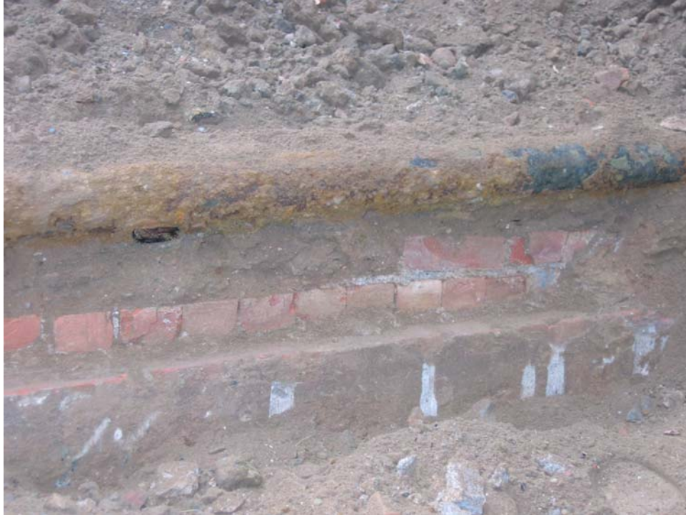
Photograph 31: Columbus Park Pavilion - Brick Foundation Wall
