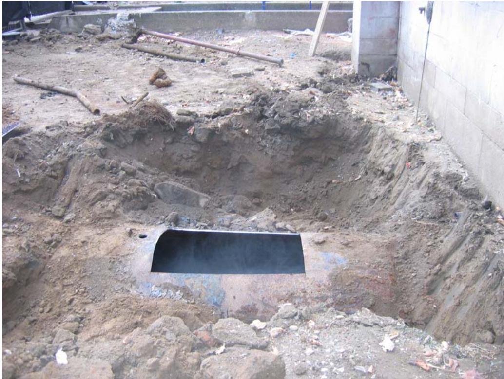
Photograph 03: Oil Tank location - just below ground surface - stairway in the top of picture
