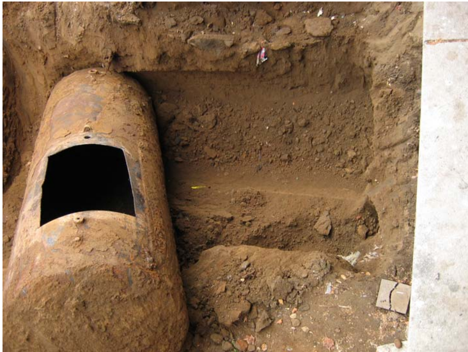
Photograph 06: Oil tank removed - note lack of stratigraphy
