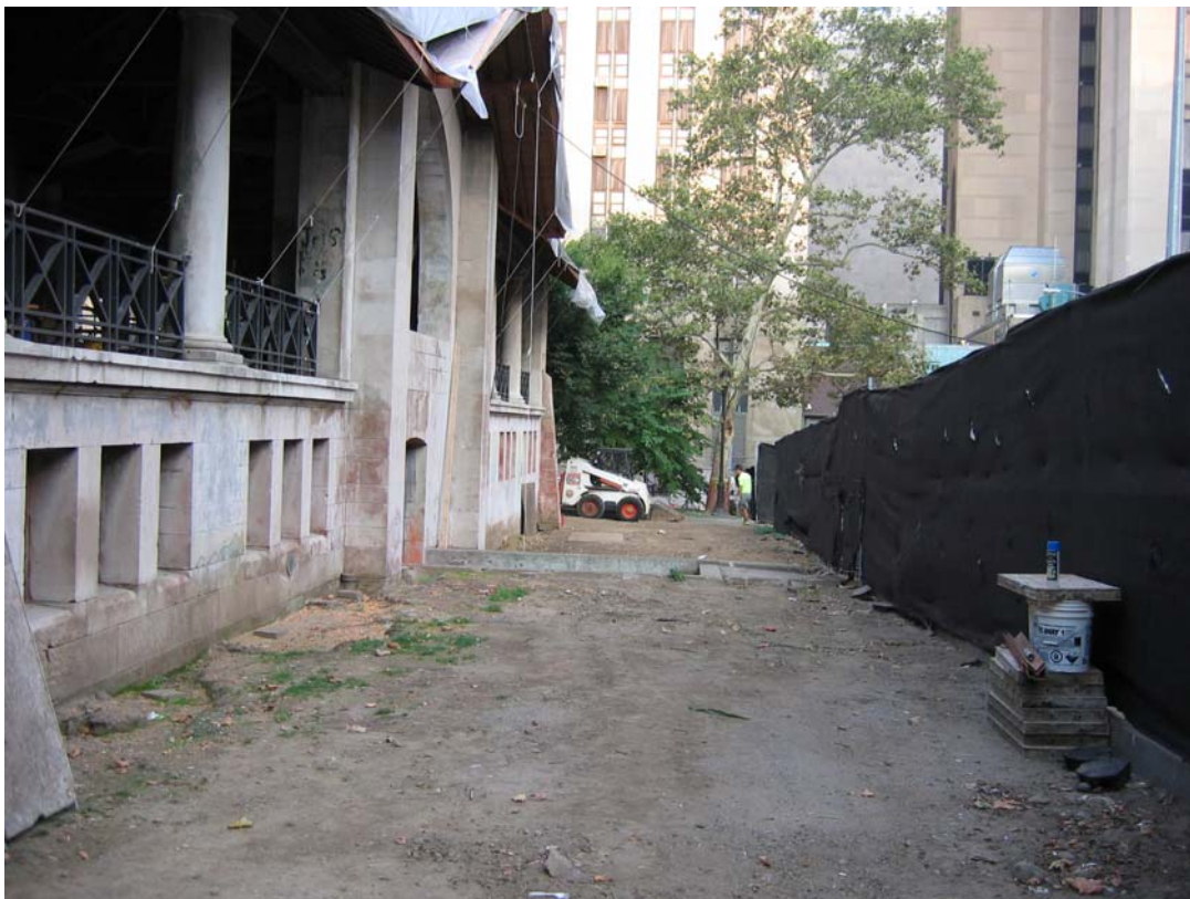
Photograph 08: Handicapped access ramp excavation area - note the stairway in the mid section of the image - excavation for the oil tank was to the north of the stairway and was completed approximately one week prior to this work - the area was backfilled upon completion.
