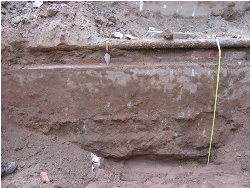
Photograph 32: Columbus Park Pavilion - Brick Foundation Wall
