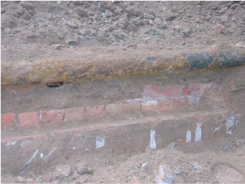
Photograph 17: Electrical line incorporated into existing brick wall - used as support
