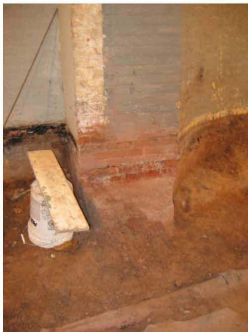
Photograph 16: Basement of Pavilion showing incorporation of previous brick wall into the current structure
