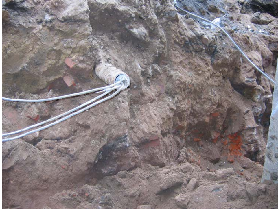
Photograph 13: Electrical line uncovered - note the other electrical line in the upper right portion of photograph
