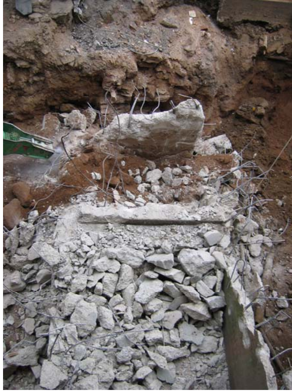
Photograph 21: Removal of stairway completed
