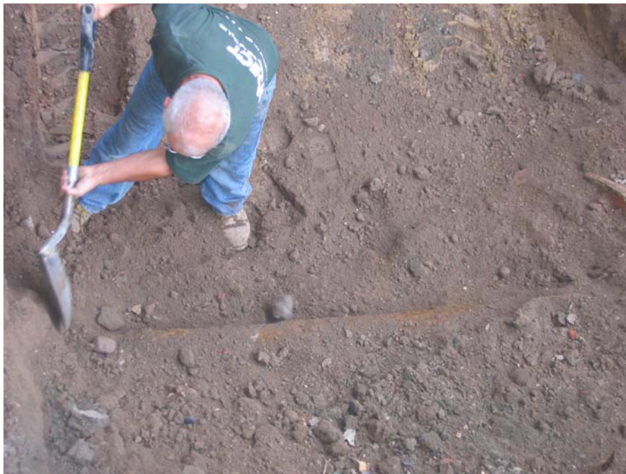
Photograph 12: Red, sandy dry soil - note the beginning of an iron water pipe being uncovered
