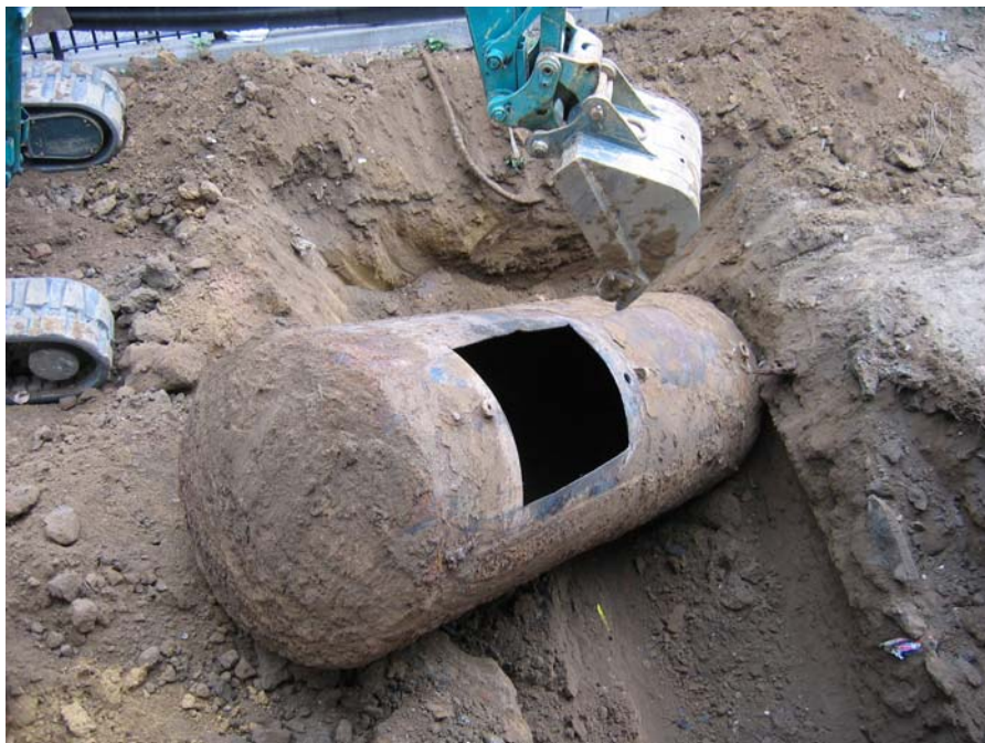
Photograph 05: Oil tank removed
