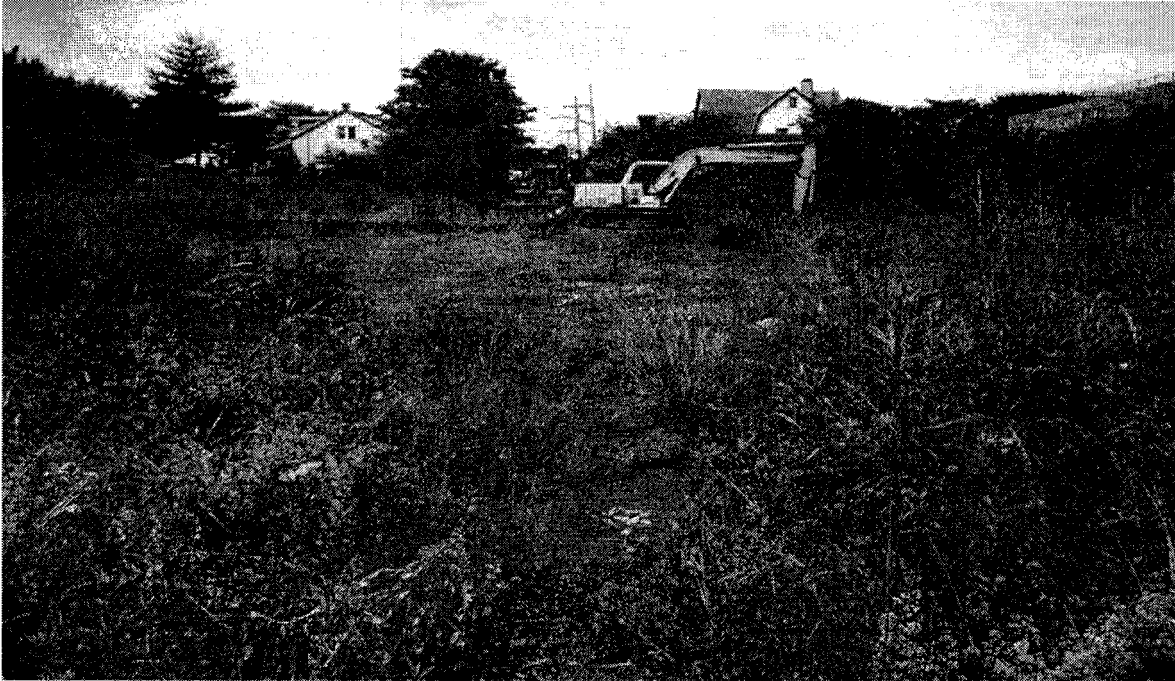
Photo 1. Project site looking west from top-of-bank on eastern end of site. Houses in center background are located on either side of Marine Street west of the project limit. The multi-story structure in the right background is located on Pilot Street north of the project site. (Geismar 6-17-09)
