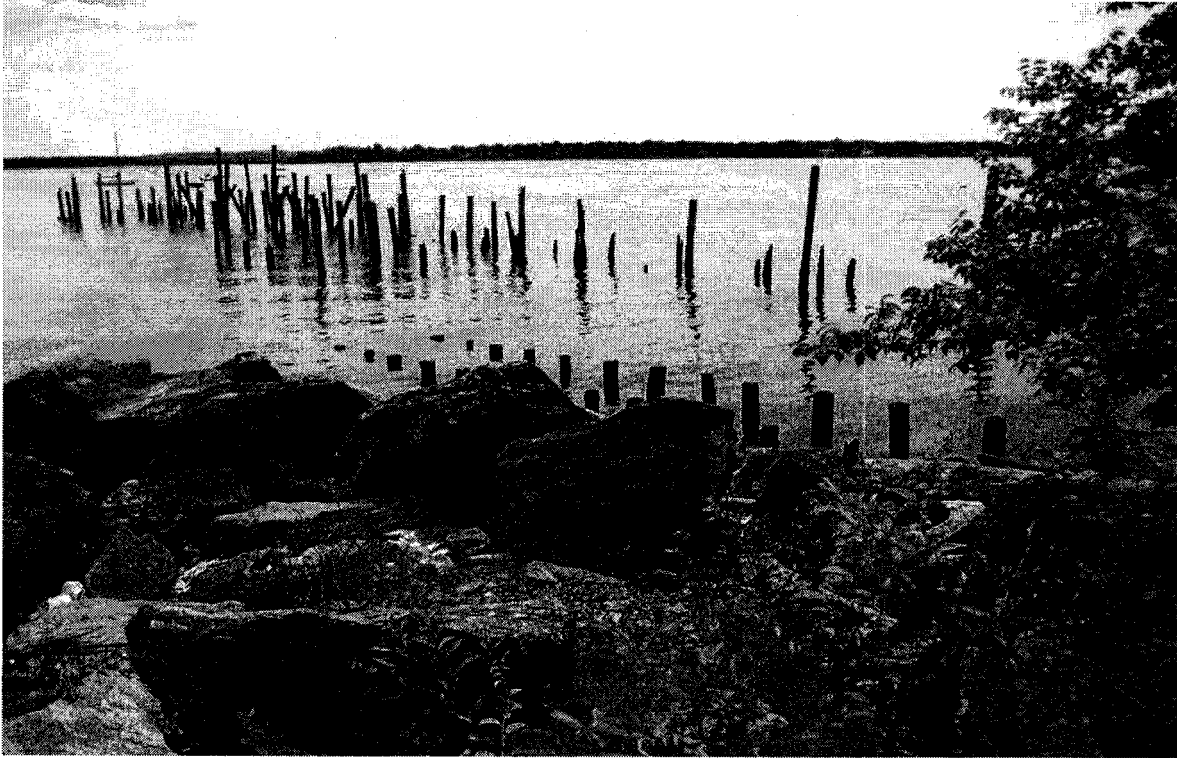
Photo 5. View east across Long Island Sound from the top of the bank. Note boulders that are part of the bank fill and remnants of timber piers. (Geismar 6-17-09)
