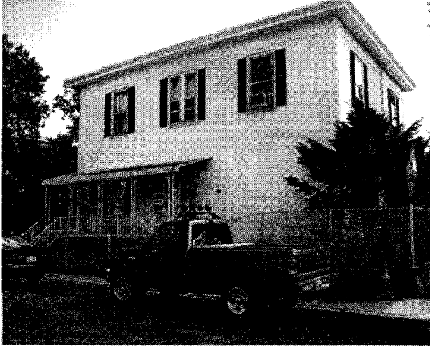
1. 88 City Island Avenue (entrance on south side of Marine Street).
