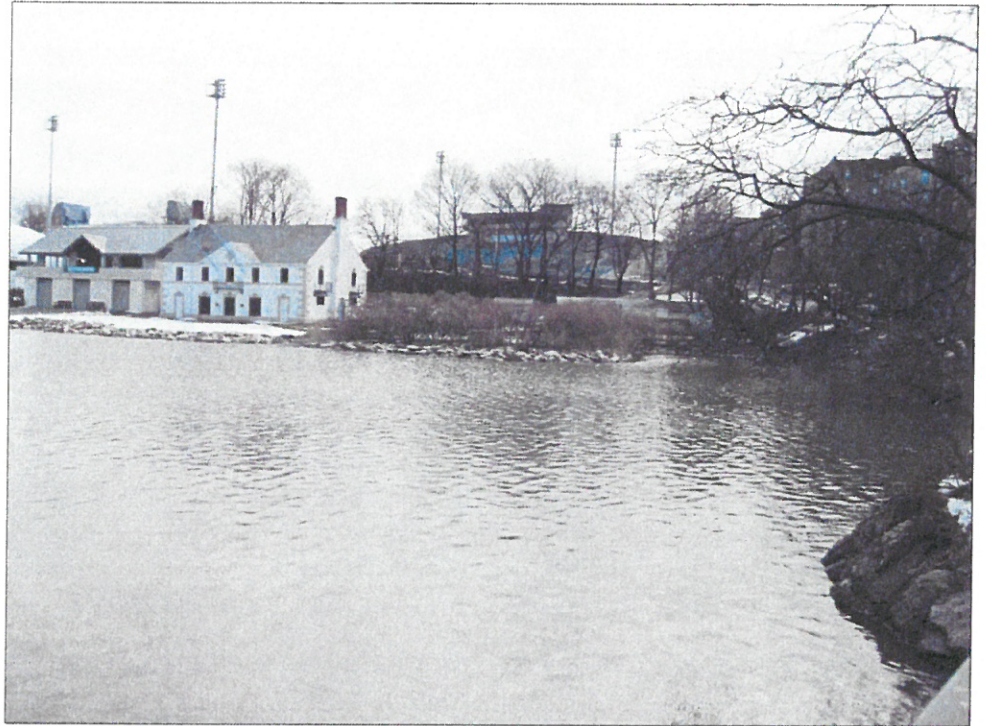
Looking east at the waterfront and cove 11
