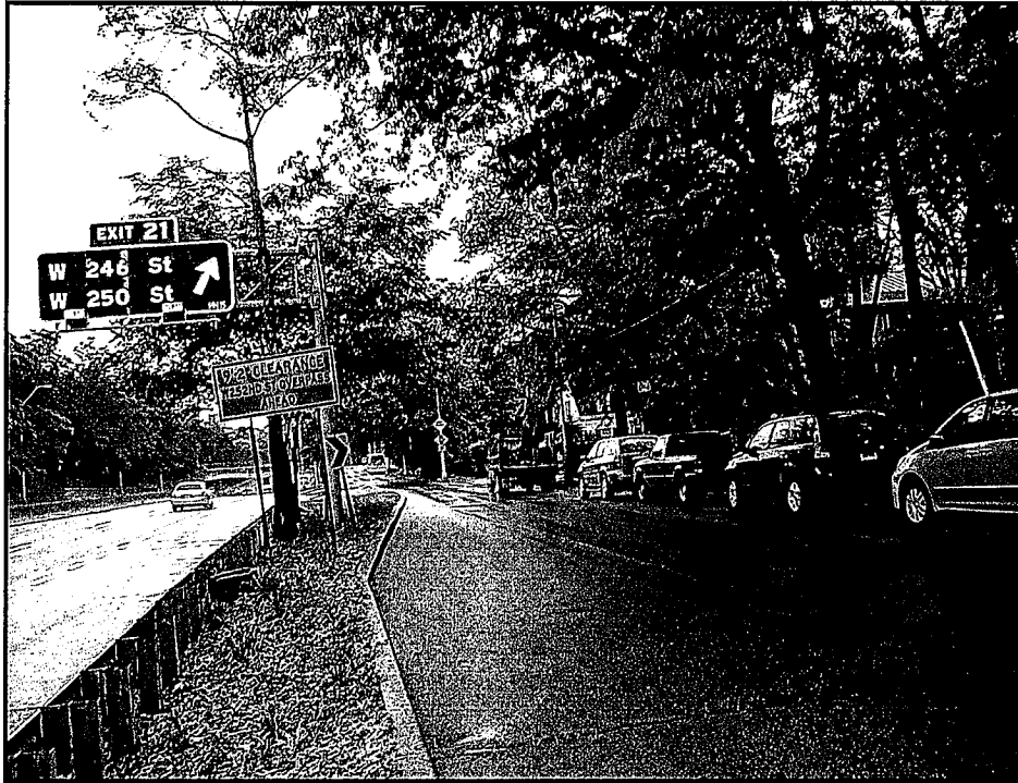
Photograph 8: Riverdale Avenue adjacent to the Henry Hudson Parkway in the Bronx. (facing north)
