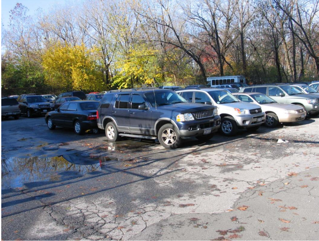
Photograph 1: Project site showing existing parking lot on southwestern side of property. Note cracked asphalt and water pooling on left. View looking west.
