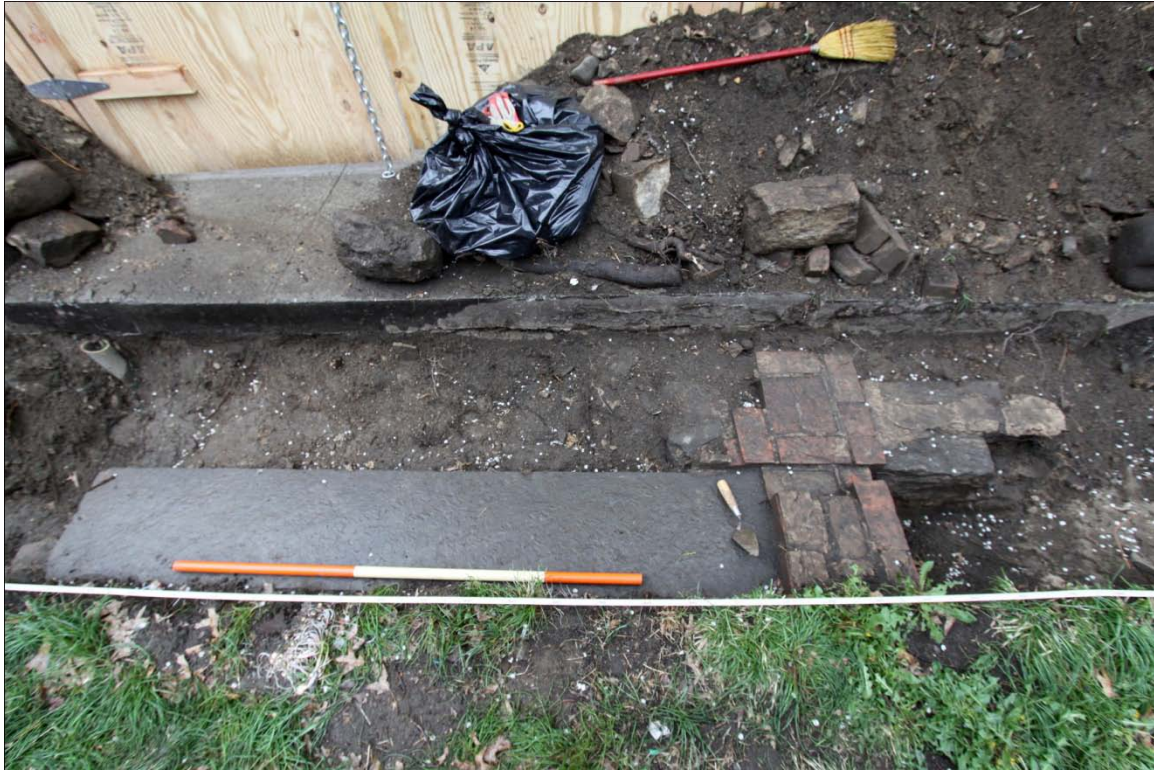
Image 10: Brick wall, bluestone cap and fieldstone wall abutment
