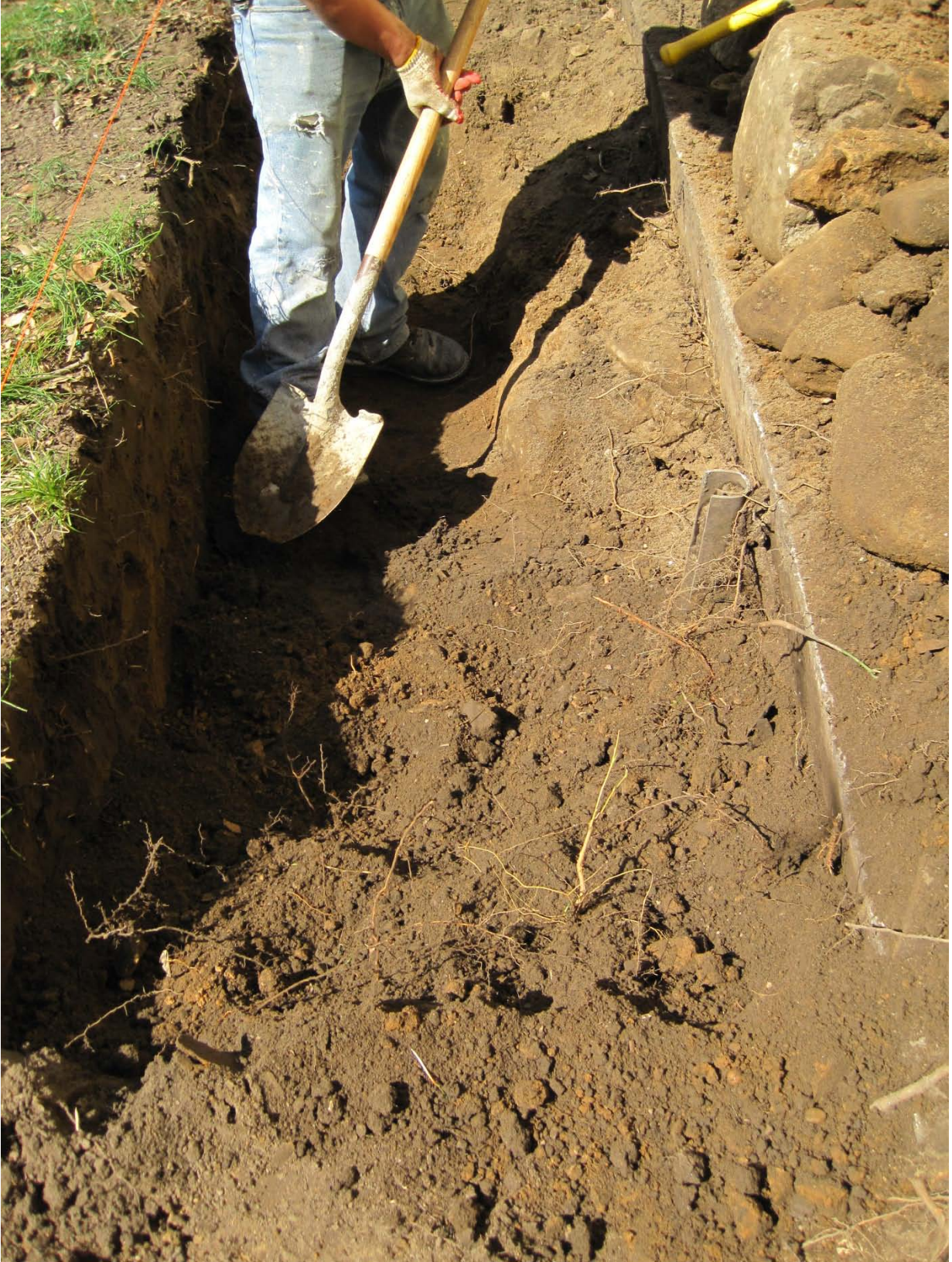
Image 22: Excavation for the foundation trench
