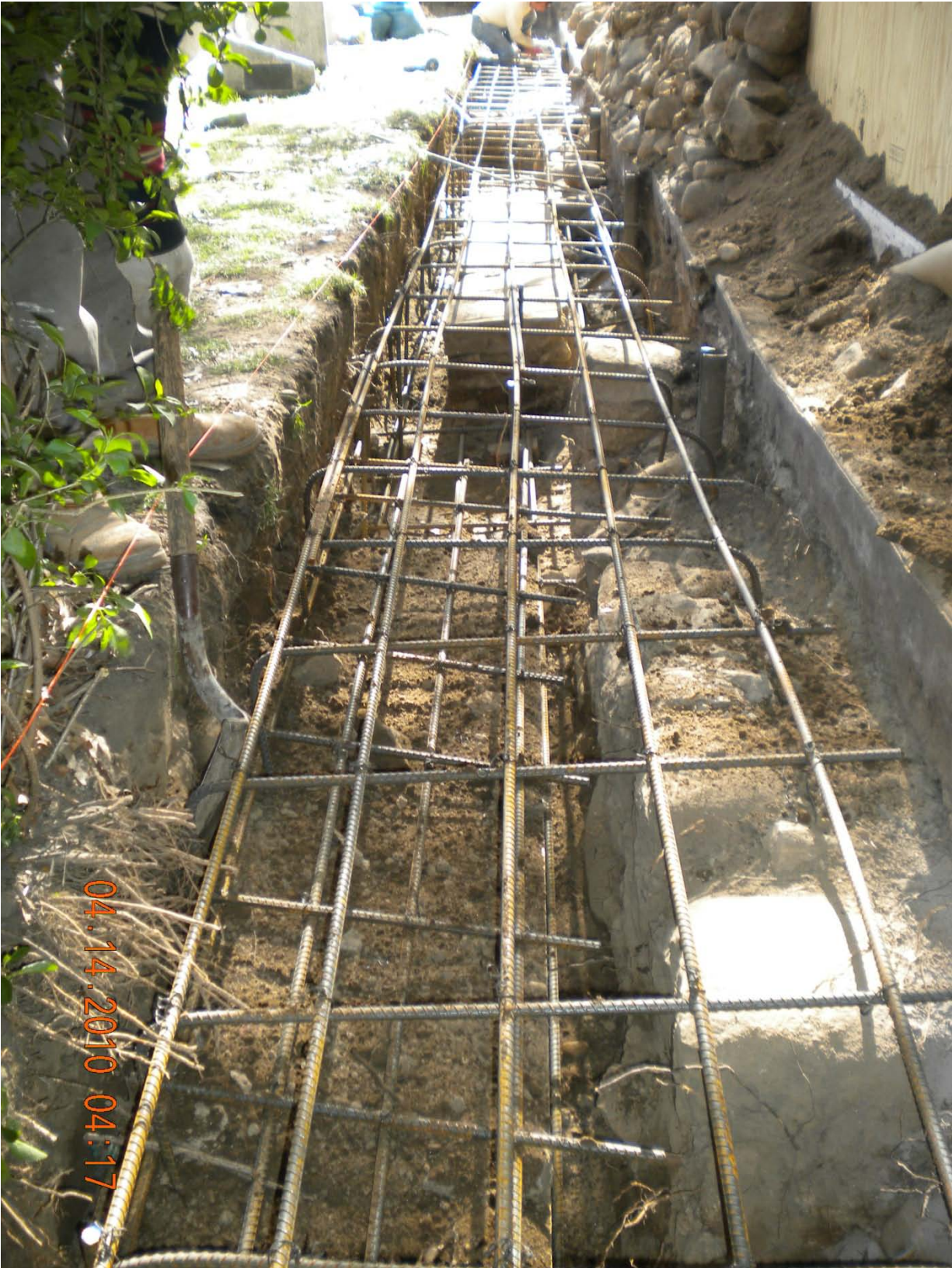
Image 30: Preparing the trench for concrete
