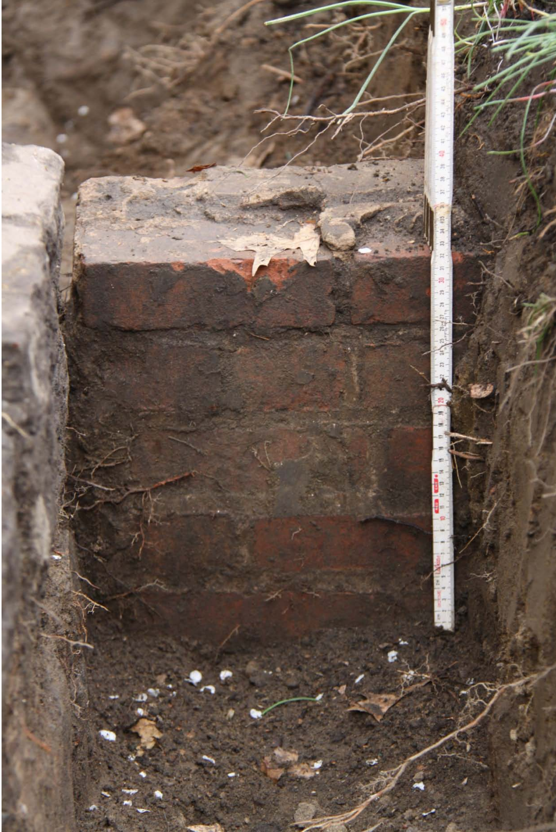
Image 26: Brick foundation wall
