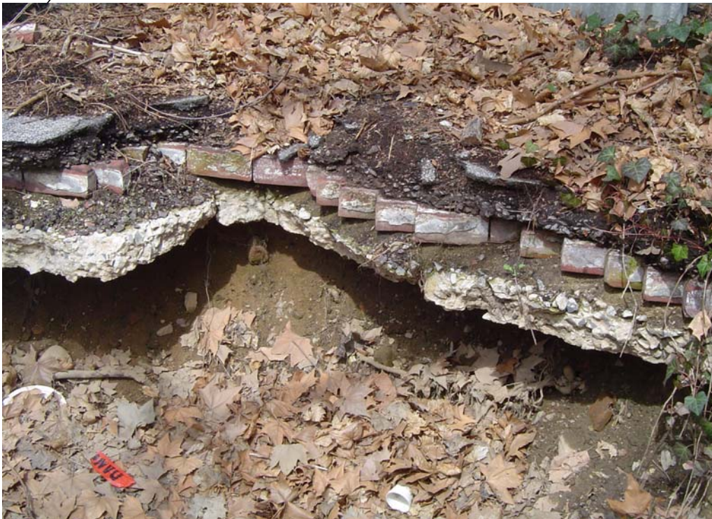
Figure 4.20. A sinkhole at the north end of Park Avenue exposing part of a former brick pavement, facing north. Brooklyn Navy Yard, Kings County, New York (PCI 2008).
