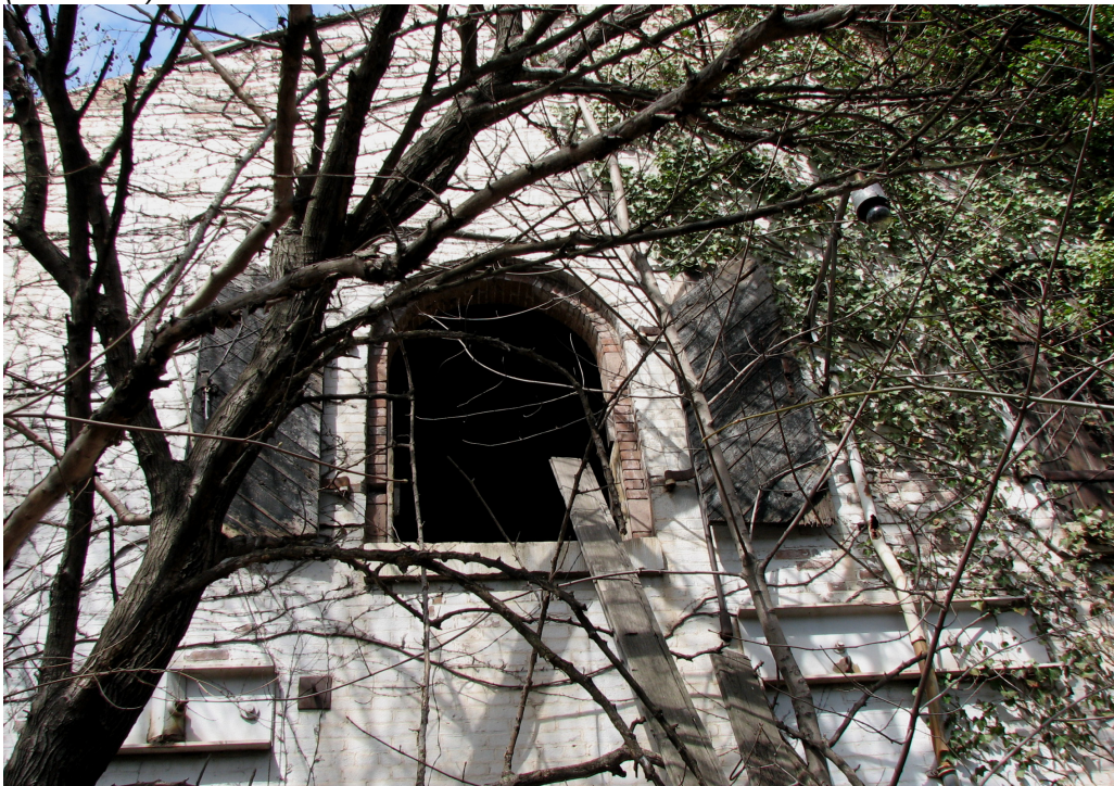
Figure 6.39. Detail of round-arch window opening, with intact wooden shutters and hardware, south elevation of Timber Shed, facing north. Brooklyn Navy Yard, Kings County, New York (PCI 2008).
