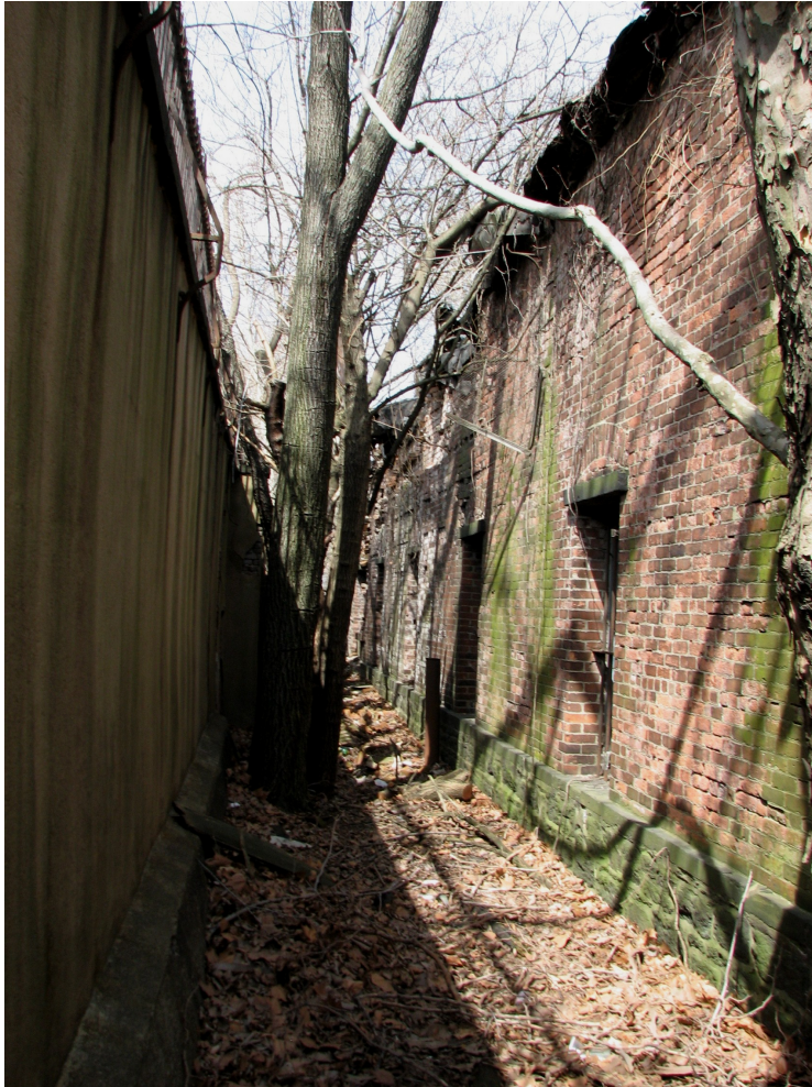
Figure 6.41. West elevation of Timber Shed at right and interior of brick fence at left, facing north. Note raised stone foundation and stone beltcourse. Brooklyn Navy Yard, Kings County, New York (PCI 2008).
