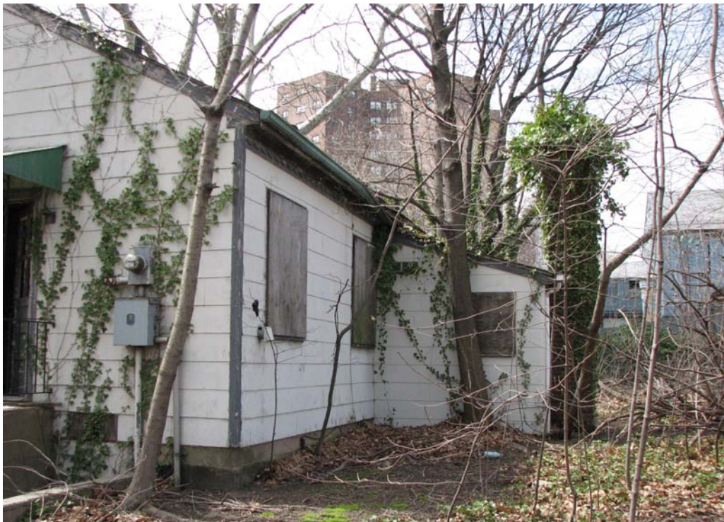
Figure 9.5. Quarters J, rear elevation with shed roof addition and exterior chimney, facing west. Brooklyn Navy Yard, Kings County, New York (PCI 2008).
