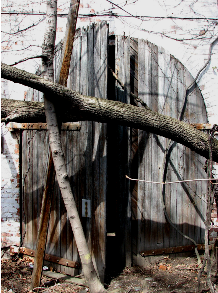
Figure 6.40. West entry bay with double-leaf doors, south elevation of Timber Shed, facing north. Note original hardware. Brooklyn Navy Yard, Kings County, New York (PCI 2008).
