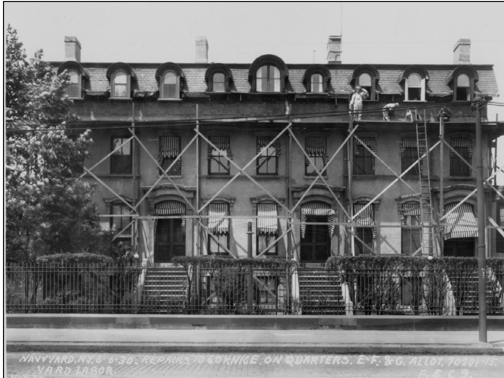
Figure 7.54. “Repairs to Cornice on Quarters E-F & G.” June 6, 1930. (New York Navy Yard: 1900-1945; Record Group 181-B; NARA—Northeast Region (NYC). Photograph No. FE C9. Reproduced courtesy of BNYDC Archives.)
