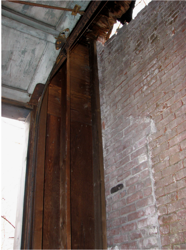
Figure 6.29. Detail of interior of northeast corner of Timber Shed, at right facing north. Note bricked window opening at right. Brooklyn Navy Yard, Kings County, New York (PCI 2008).
