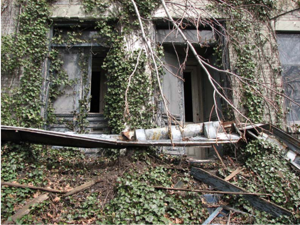
Figure 7.3. Quarters K-L, entrance detail, facing north. Note collapsed cornice. Brooklyn Navy Yard, Kings County, New York (PCI 2008).
