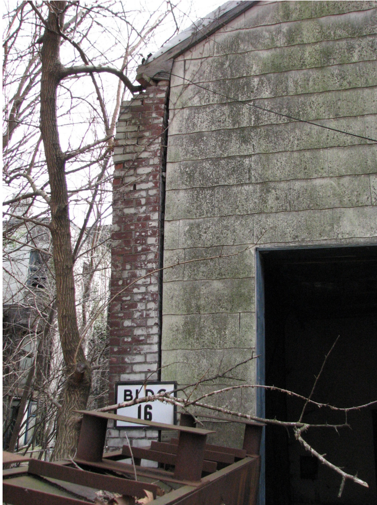
Figure 6.28. Detail of northeast corner of Timber Shed, at left, facing south-southeast. Note juncture of original brick masonry wall and later asbestos-covered frame wall.
