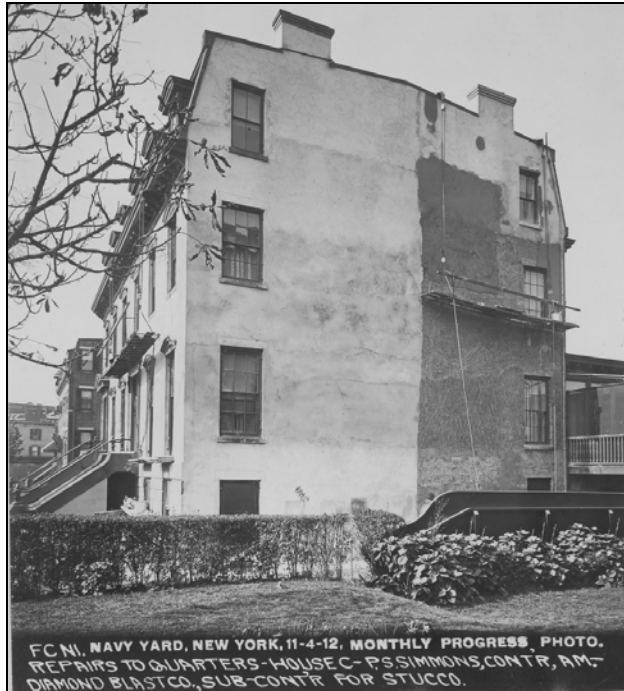
Figure 7.17. “Repairs to Quarters – House C,” November 4, 1912. Note brownstone stylistic accents prior to application of stucco. Brooklyn Navy Yard, Kings County, New York ( New York Navy Yard: 1900-1945; Record Group 181-B; NARA—Northeast Region (NYC). Photograph FC N1. )
