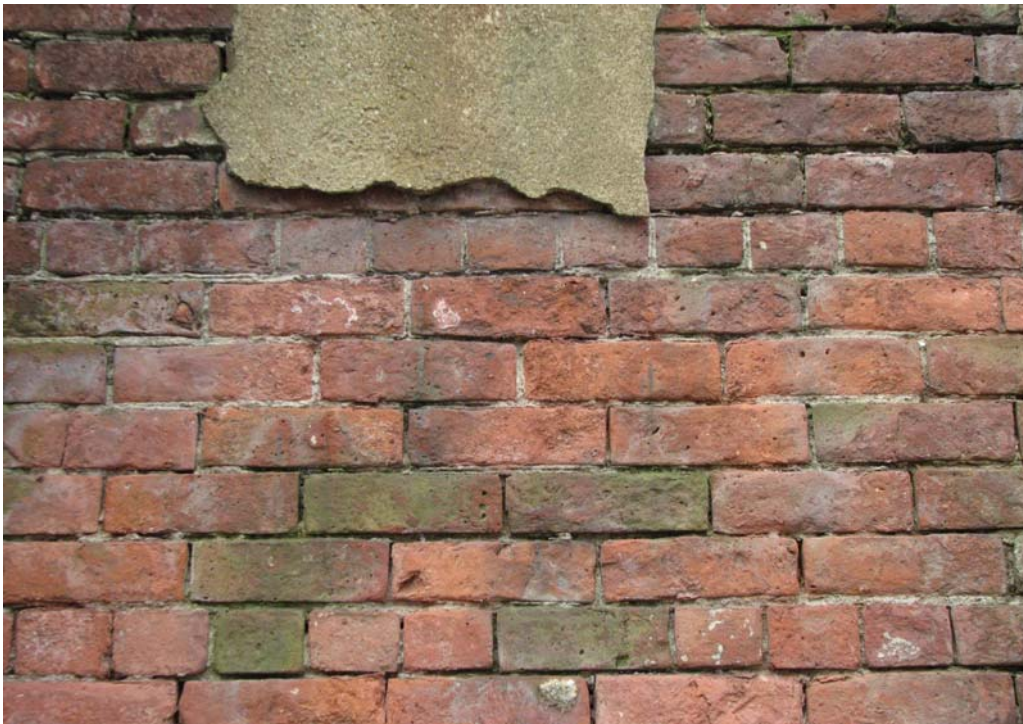
Figure 10.2. Detail of brick masonry of wall showing common bond construction. Note stucco above. Brooklyn Navy Yard, Kings County, New York (PCI 2008).
