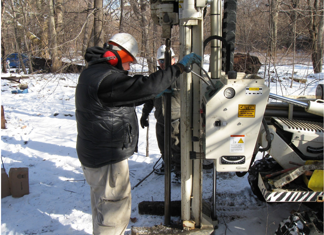
Figure 6. Acquiring a core sample with the Geoprobe machine during the geomorphological investigation. Brooklyn Navy Yard, Kings County, New York (PCI 2009).
