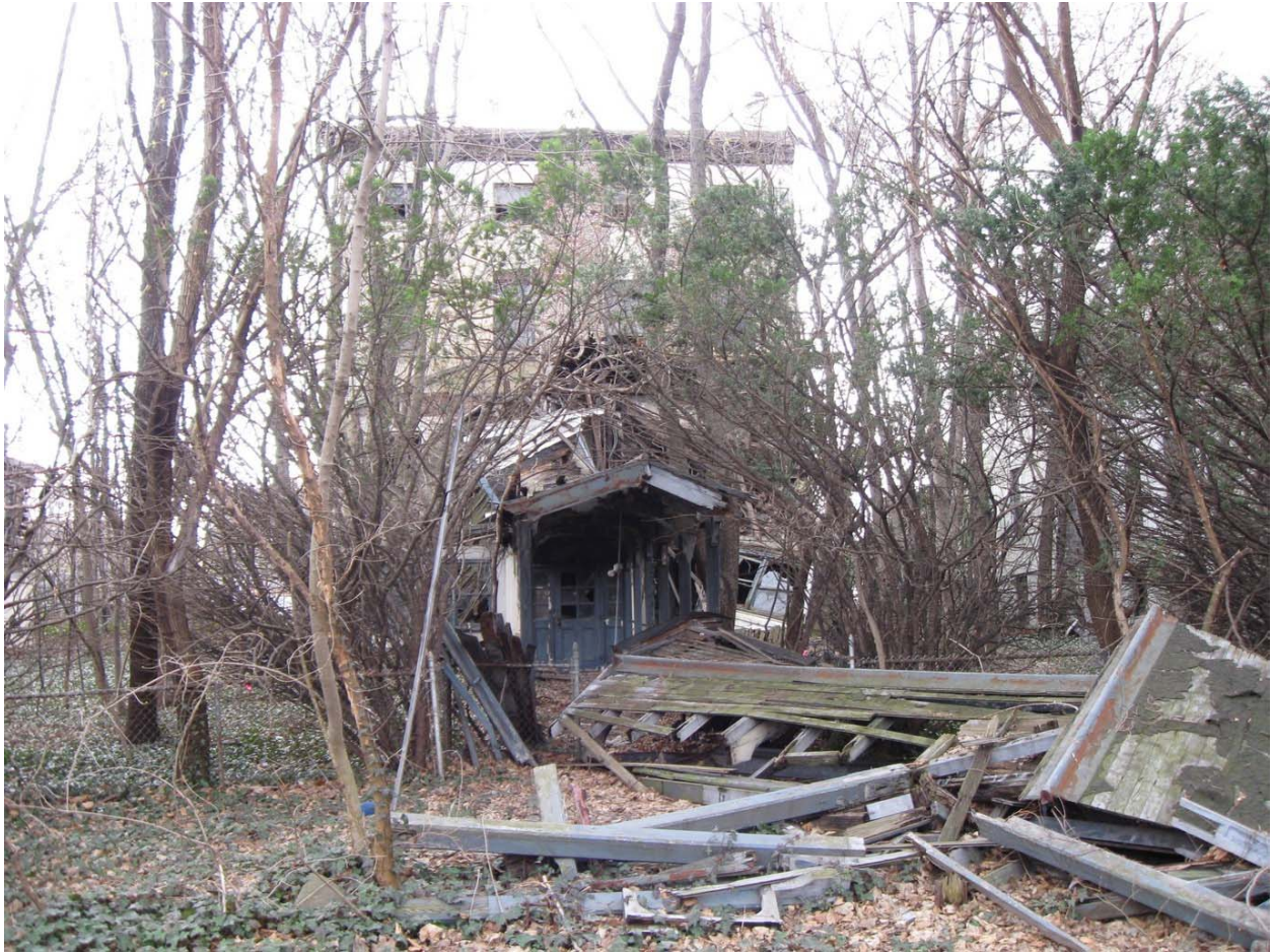
Figure 28. Collapsed portion of the superstructure for the roofed walkway that extends north from Quarters B, facing south from Park Street. Brooklyn Navy Yard, Kings County, New York (PCI 2009).
