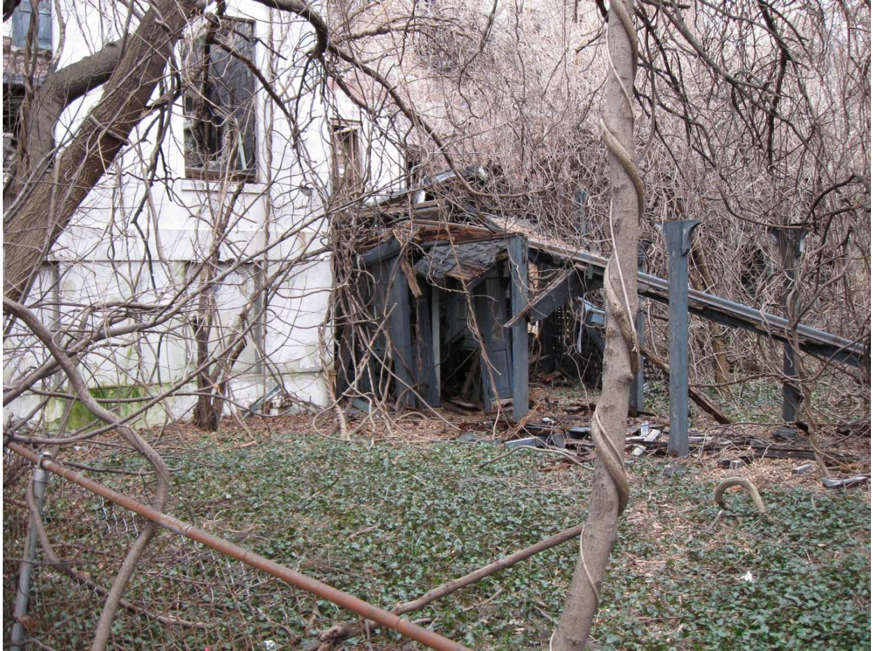
Figure 29. Collapsed portion of the superstructure for the roofed walkway that extends north from Quarters C, facing southwest. Brooklyn Navy Yard, Kings County, New York (PCI 2009).
