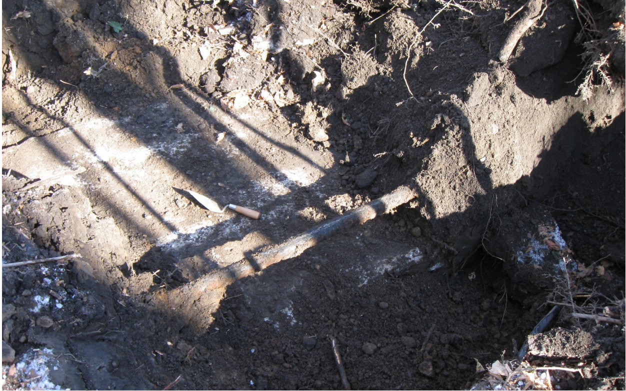
Figure 18. Concrete utility casing in Trench 5 after the trench was widened to the north. Brooklyn Navy Yard, Kings County, New York (PCI 2009).
