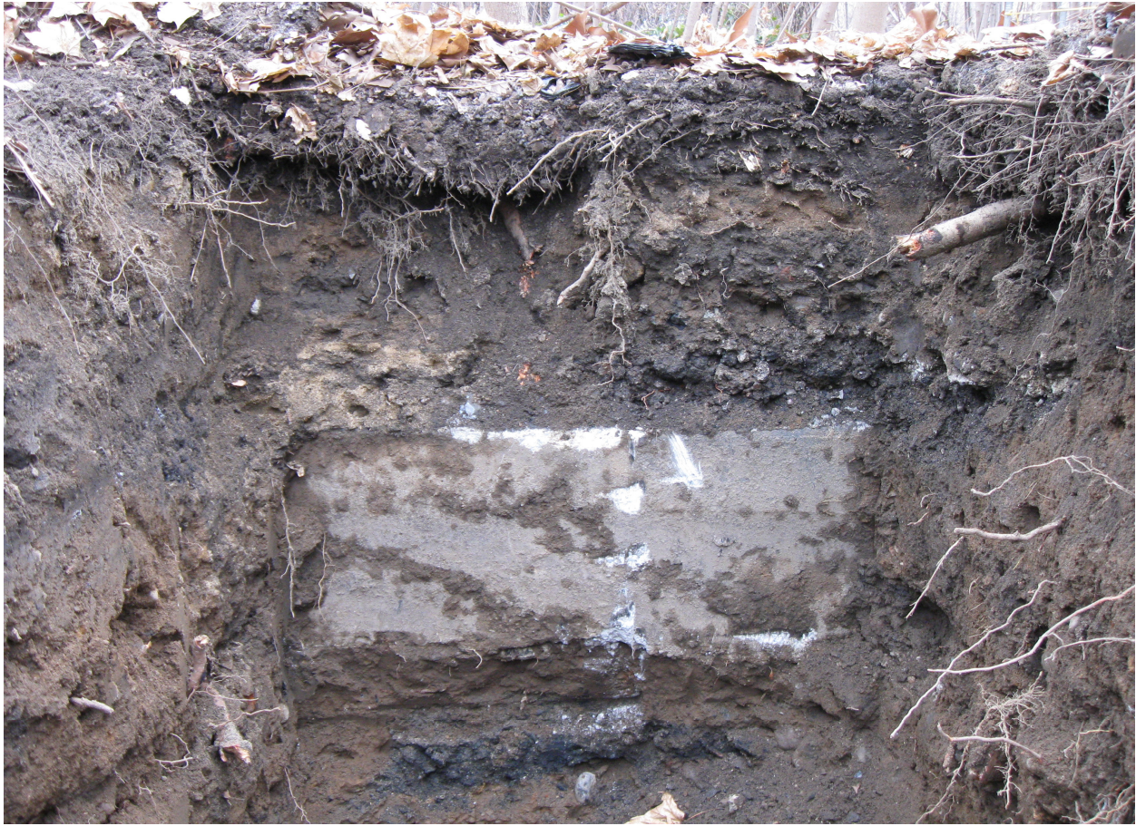
Figure 11. Poured-concrete utility casing exposed in the west end of Trench 1. Brooklyn Navy Yard, Kings County, New York (PCI 2009).
