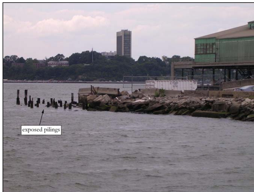
Photograph 5-2. Riprap portion of the Hudson River Bulkhead along the Project pipeline route
