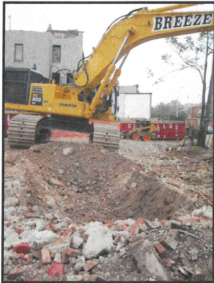
Photograph 3.5 Block 1127, Lots 48 and 50, Test Trench A2.
