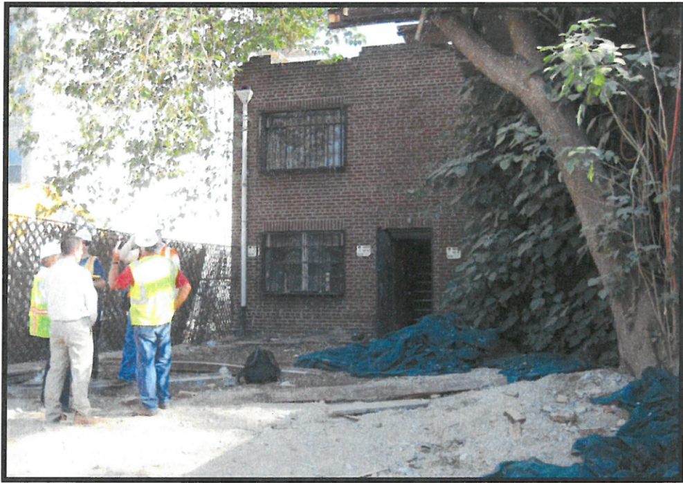
Photograph 1.1 Block 1127, Lot 50 prior to demolition.
