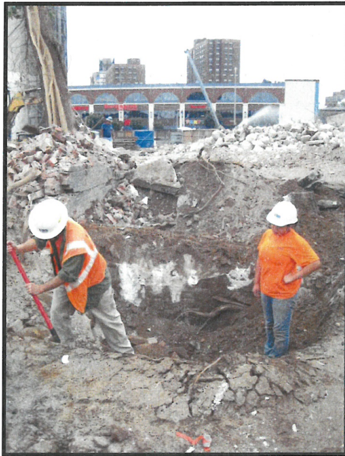
Photograph 3.7 Block 1127, Lot 48, concrete foundation wall.
