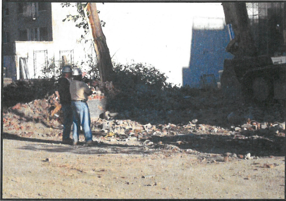
Photograph 3.1 Block 1127, Lots 48 and 50 post-demolition.
