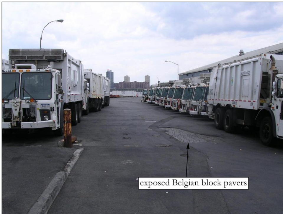
Photograph 5-1. Belgian block pavers visible under asphalt surface of Gansevoort Street at the NY Sanitation Pier/Gansevoort Destructor Plant, view looking west.
