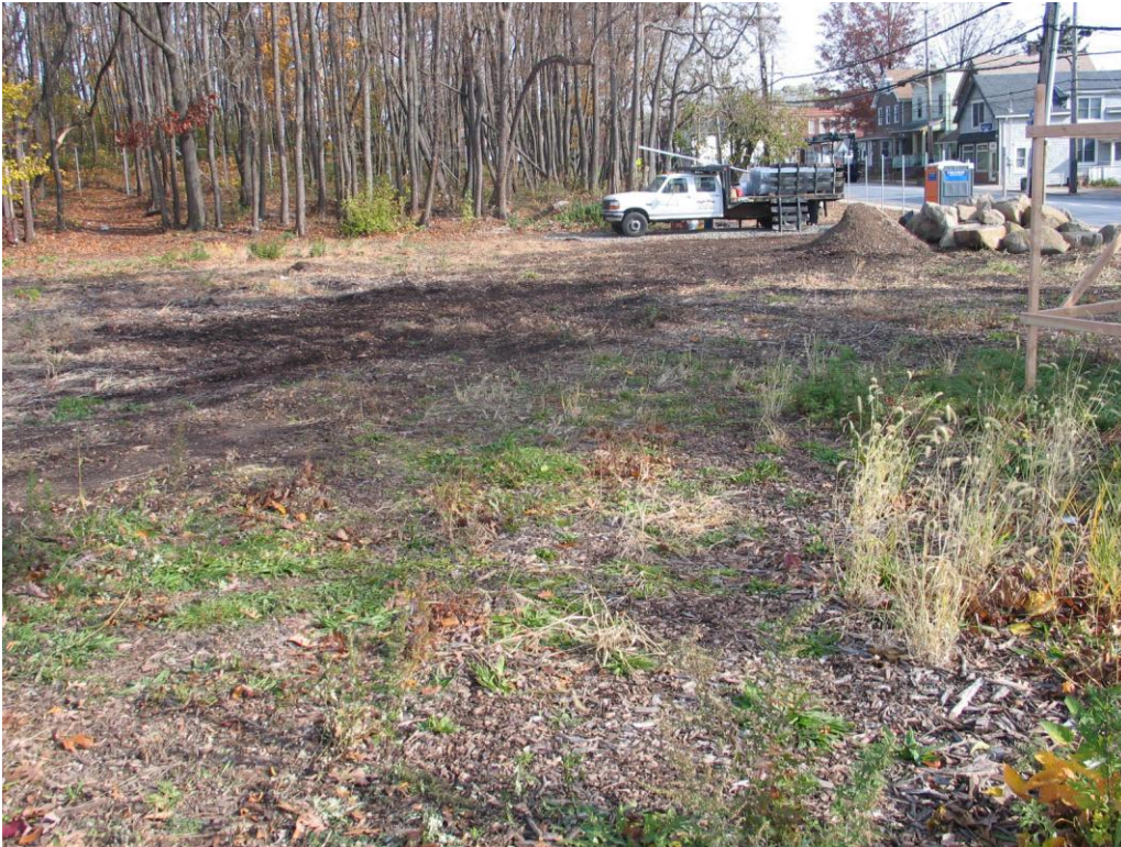
Photograph 21: Lot 22 showing its current use as a DPR construction staging area. View looking east from Glen Street.
