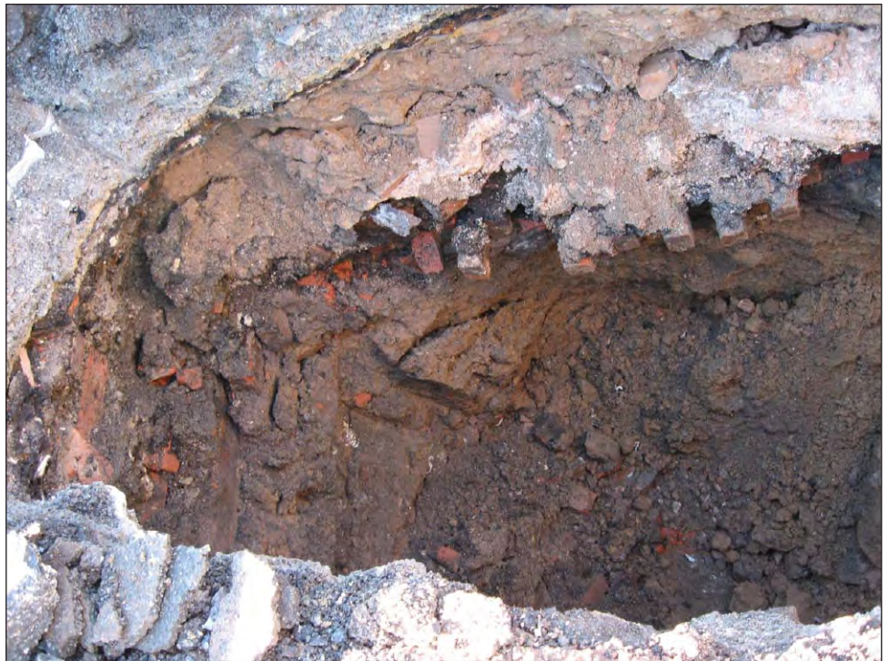
Test Pit 4 showing loose construction debris and bricks to a depth of ten feet below pavement
