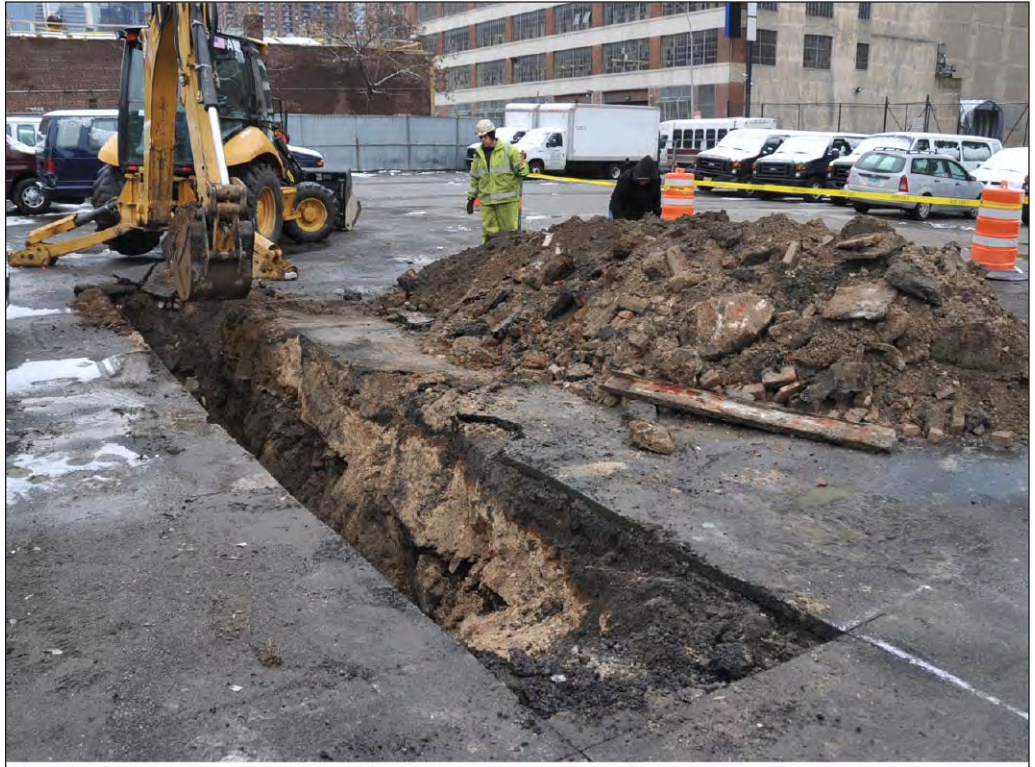
Trench 2 in Area 3, facing southeast showing removal of loose demolition debris 13
