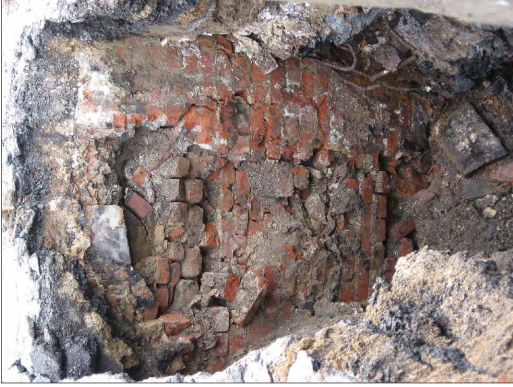
Test Pit 1 showing brick foundation wall on east wall of pit. A concrete slab was observed at the base of this wall 6
