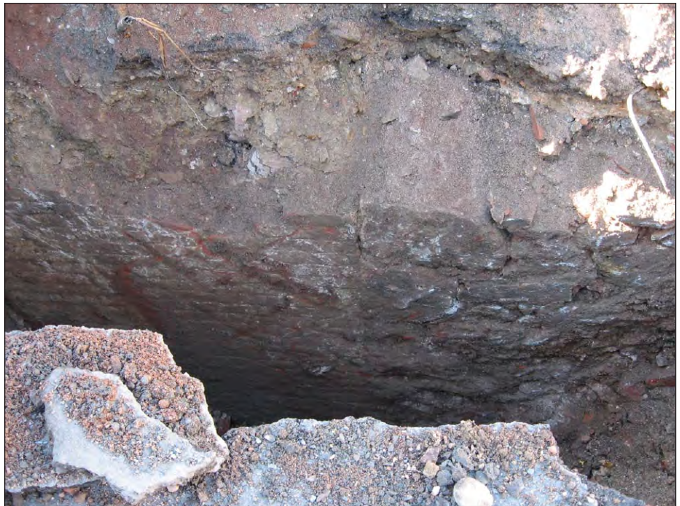
Test Pit 5 showing south wall of pit where two foundation walls meet, one brick and one, on right, larger cut stone
