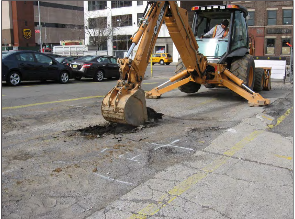
Facing northwest from center of parking lot toward intersection of W45th Street and 11th Avenue
