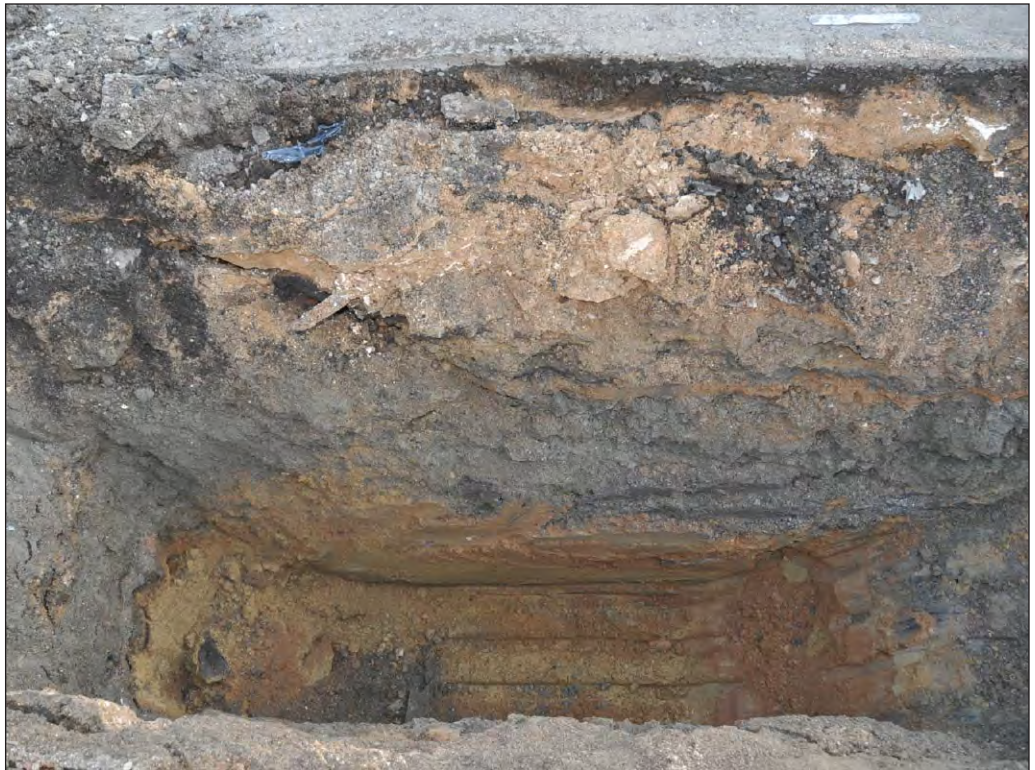
Trench 2 in Area 3, showing sterile light brown sandy subsoil 14 beneath four feet of loose historic fill and demolition debris
