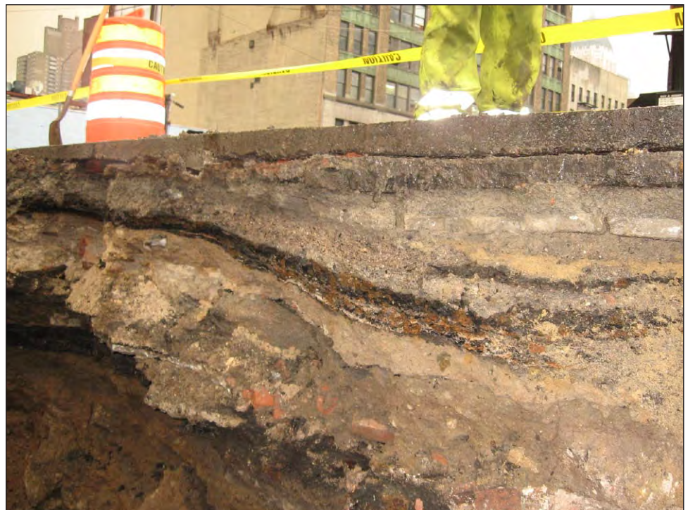
Trench 1 in Area 2 showing layers of fill and demolition debris on east side of trench 12
