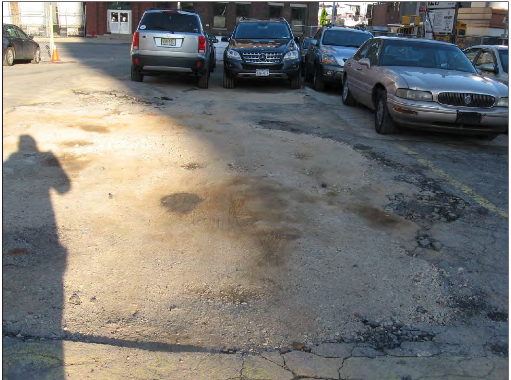
Facing north across Area 1 toward 45th Street
