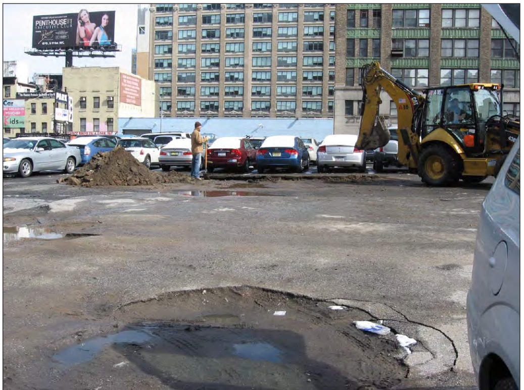
Facing north from south side of parking lot near W44th Street showing testing of Area 3 4
