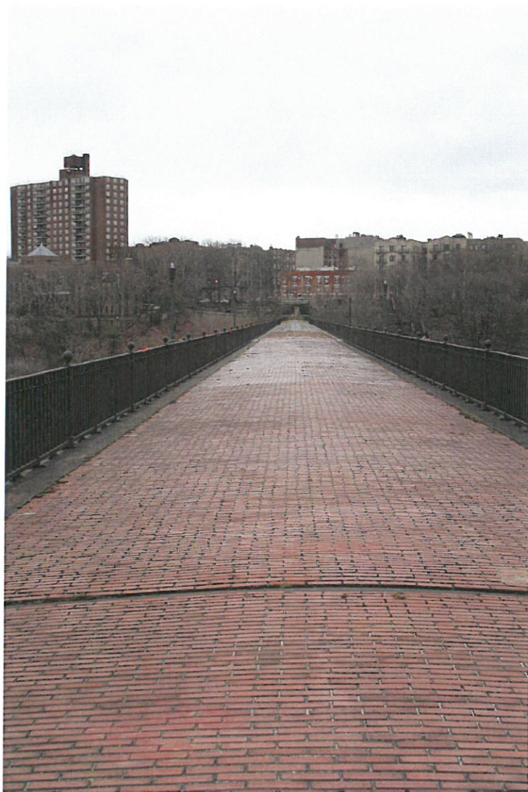
Photograph 9: High Bridge with Bronx APE in background. View looking east from bridge.
