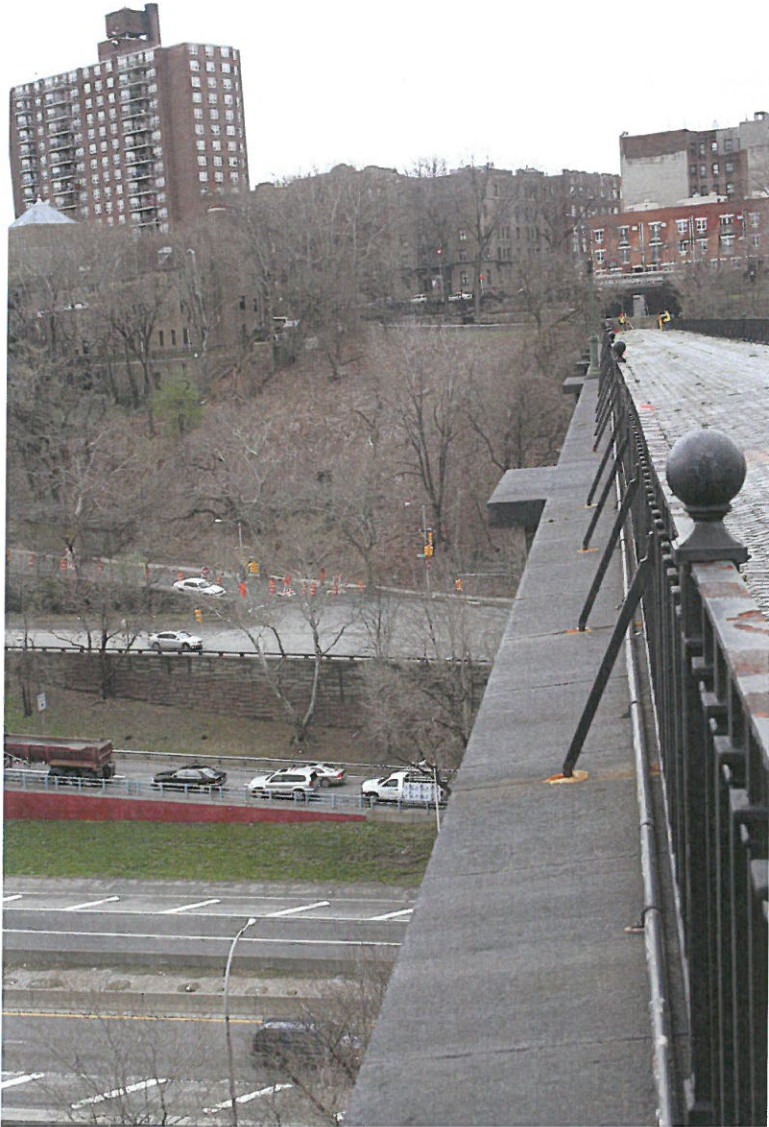
Photograph 12: Bronx terminus showing wooded and brushy slope on north side of APE in background. View looking east from bridge.
