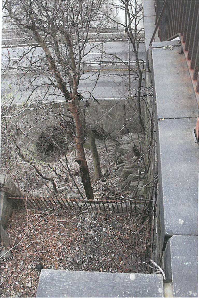
Photograph 2: Manhattan terminus of High Bridge, with Harlem River Drive and Harlem River at base of slope. View looking east from north side of APE.
