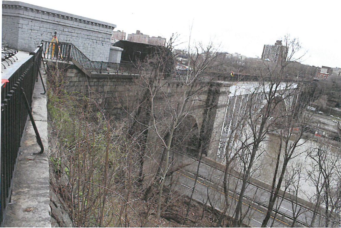
Photograph 1: Manhattan terminus of High Bridge, with Harlem River Drive and Harlem River at base of slope. View looking northeast from south side of APE.
