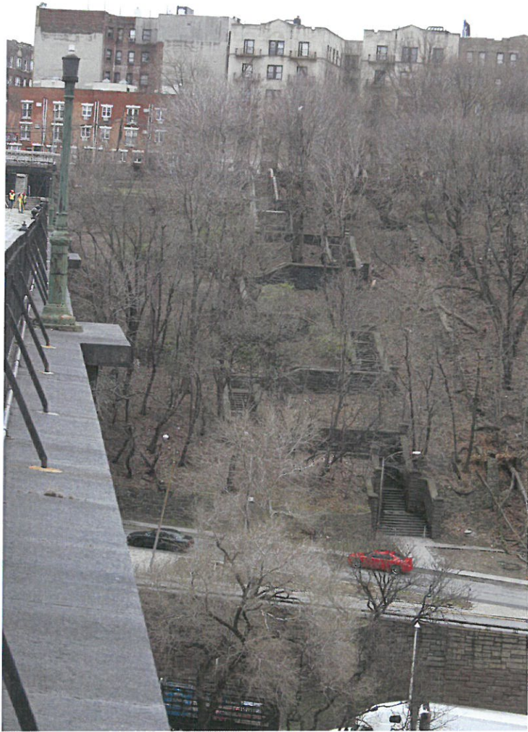
Photograph 10: Bronx terminus showing ashlar block stairway immediately to the south of the bridge touchdown. View looking southeast from bridge.
