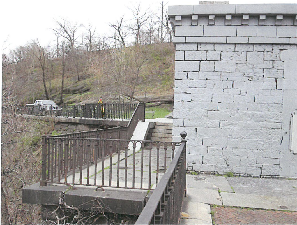
Photograph 6: Manhattan terminus showing gate house and approach to bridge. View looking west from bridge.
