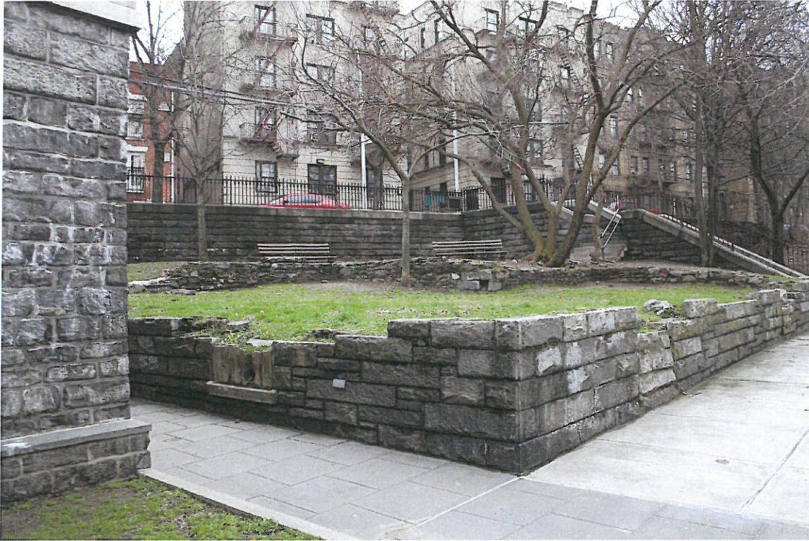
Photograph 15: Bronx APE showing detail of park on south side of bridge. The foundation represents remains of the former office building that was once in this location. View looking southeast.
