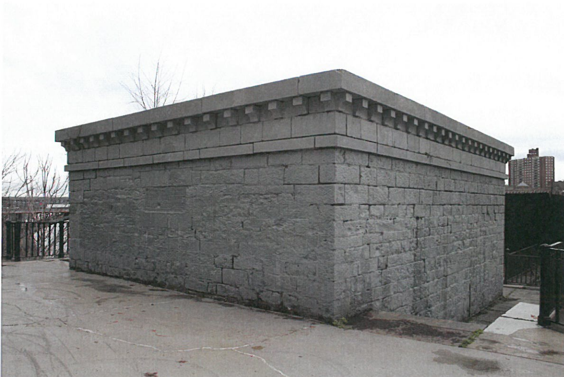
Photograph 7: Manhattan terminus showing detail of gate house. View looking northeast from bridge approach.
