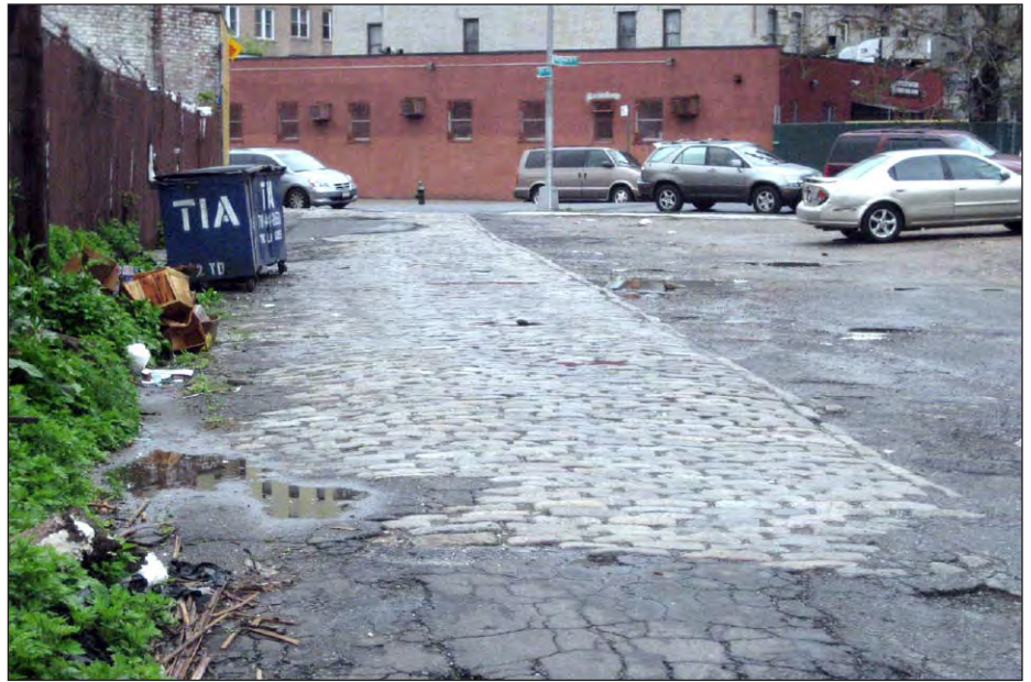
A view of Clove Road prior to commencement of the Phase 1B investigation, looking north towards the intersection of Montgomery Street. Note that only the western portion of Clove Road is paved with Belgian Block
