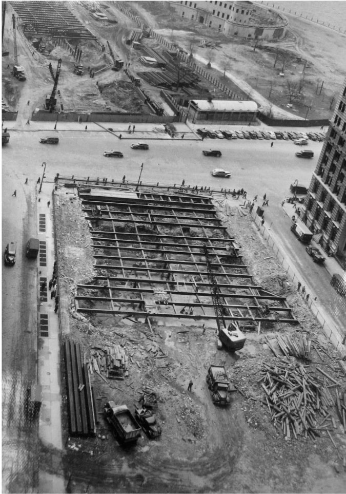
Photo 2. Cut-and-cover-construction activities in 1947 at the site of the "Blower Building" for the Brooklyn/Battery Tunnel located north of Battery Place between Greenwich and Washington Streets. (courtesy of MTA Bridges & Tunnels, Contract 6, Photo No. 2205-April 24, 1947)
