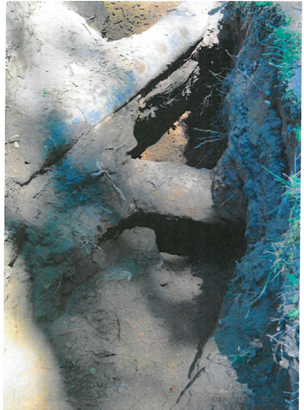
Photo 2. Detail of a utility pipe network found in TP1. (Geismar 6-27-11)
