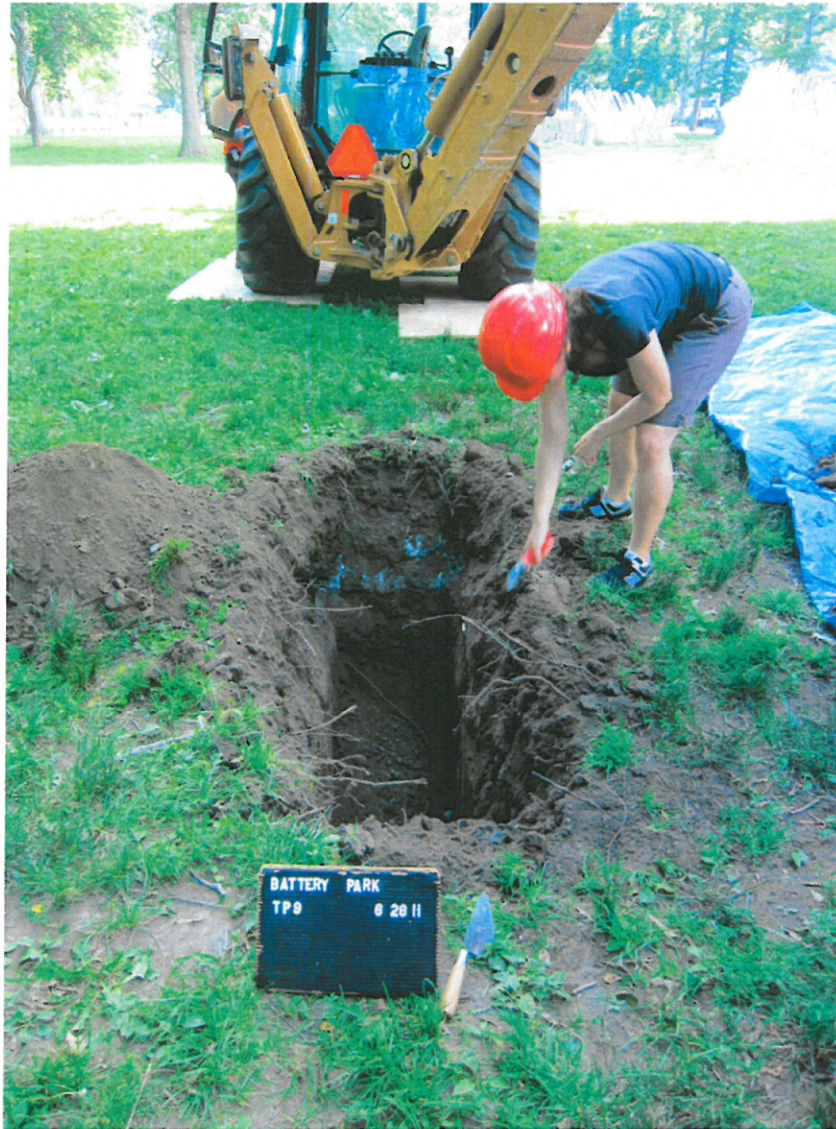
Photo 11. Test Pit 9 (TP9) looking north. Because tree roots were a concern in this test pit, the first 1.5 feet were hand excavated. (Laura Wooley, an arborist, is trimming exposed roots but none were considered significant). Here, as elsewhere throughout the tested area, the fill was a hard-packed soil with some small, redeposited artifacts mixed with modern debris. (Geismar 6-28-11)
