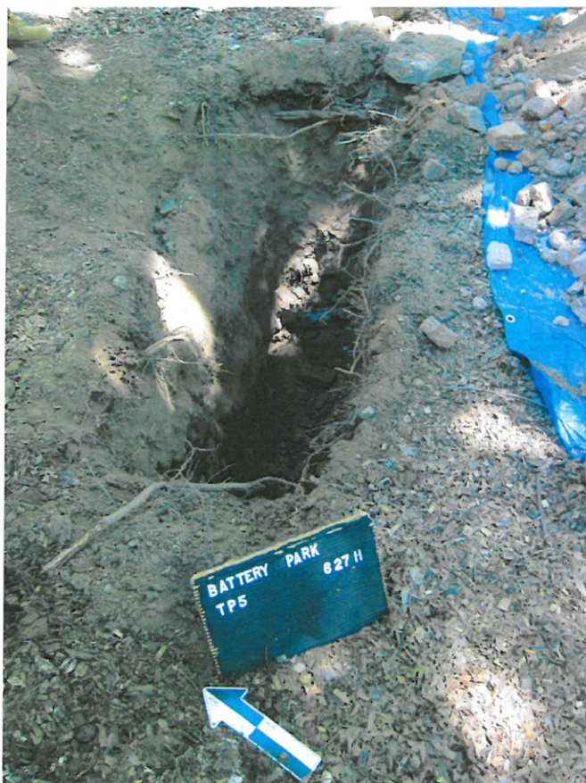
Photo 7. Test Pit 5 (TP5) looking northeast. Initial excavation was by hand because of concern about a potential gas line. The arborist in attendance trimmed the exposed tree roots. (Geismar 6-28-11)
