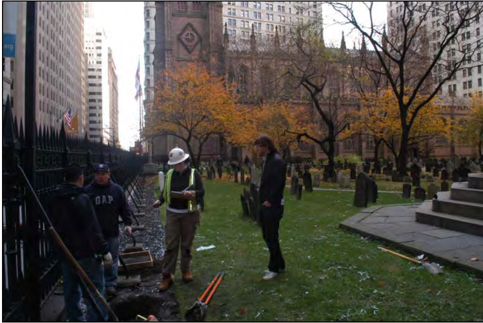
Photo 4 - View South of Test #2 for Trinity Church, Opposite Pine Street.
