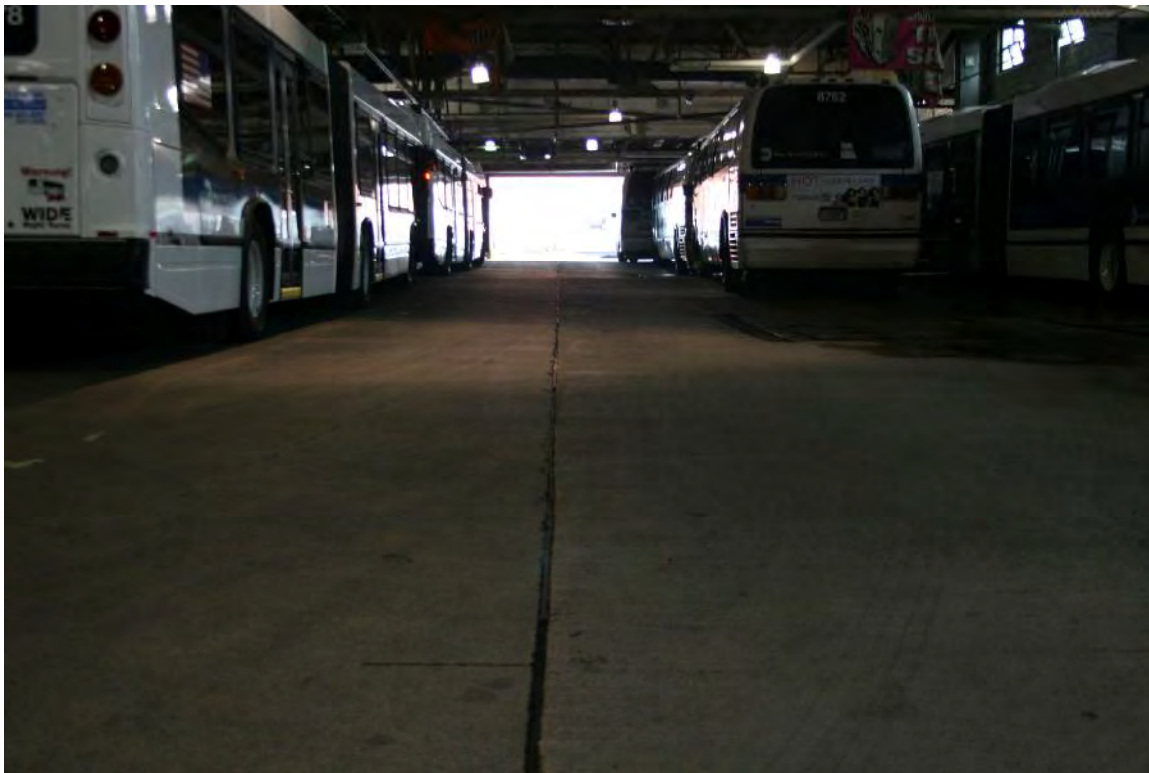
Photograph X: West end of Bus Wash where cement was piped below-grade ca. 2000 to raise the flooring which was sinking.
