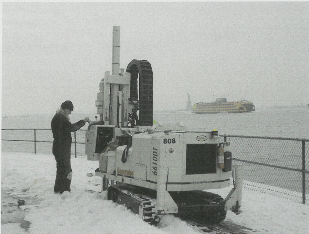
Work in progress at SB-1, facing southwest (January 25, 2011).
