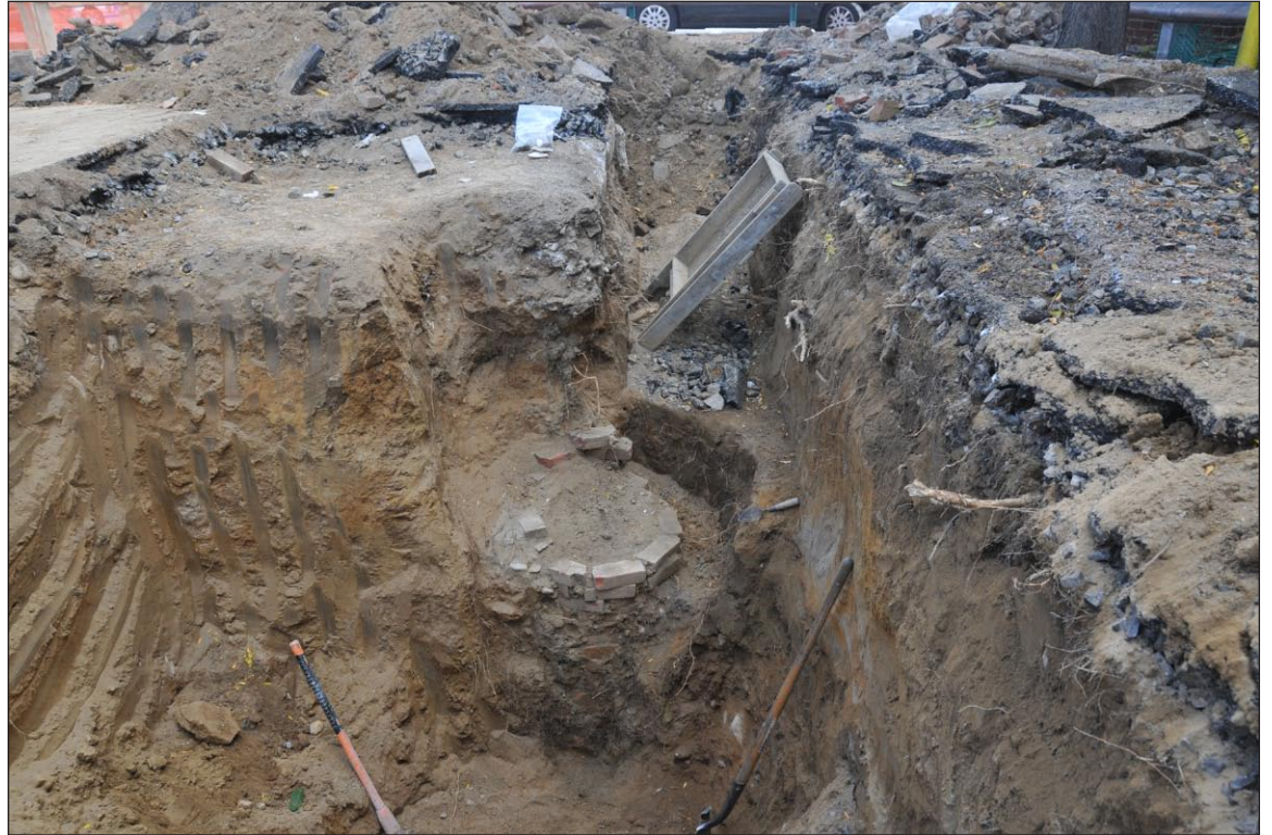
Trench 1 expansion exposes more of the privy and the buffer zone 5
