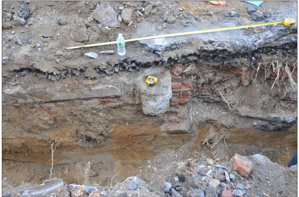
Concrete and brick foundation in the north wall of Trench 1, located approximately 14'-9" west of the fence at Union Street 2A
