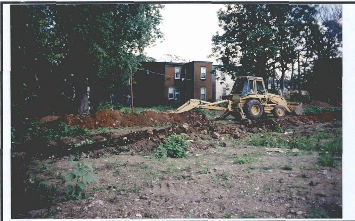
Photo 3: A trench was excavated along rear property lines in attempt to locate privy features. Large trees made excavation difficult. No privy features were revealed.
