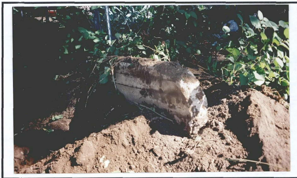
Photo 10: Brick debris and a substantial concrete foundation wall were revealed. These are interpreted as part of an outbuilding appearing on Sanborn maps of the site.
