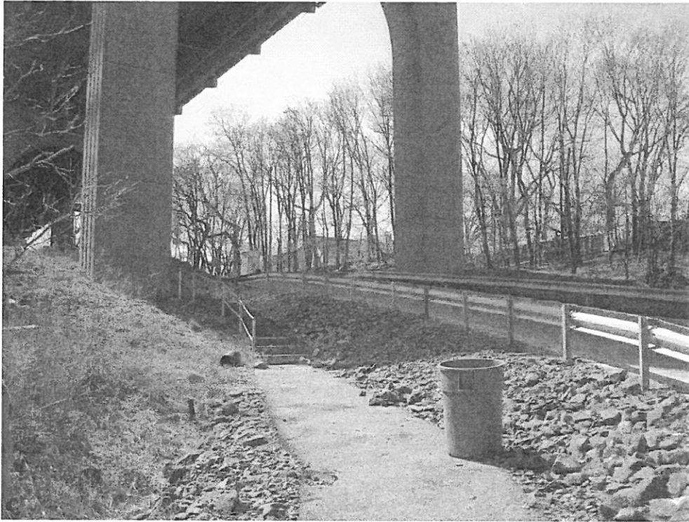
Photo 1. View south from south end of project showing existing path and roadway leading to the Queens anchorage located behind the photographer. A new access road is proposed in this area seen in the left of photo. Pier 1Q will be located near the beginning of the steps in the center of the photo.
