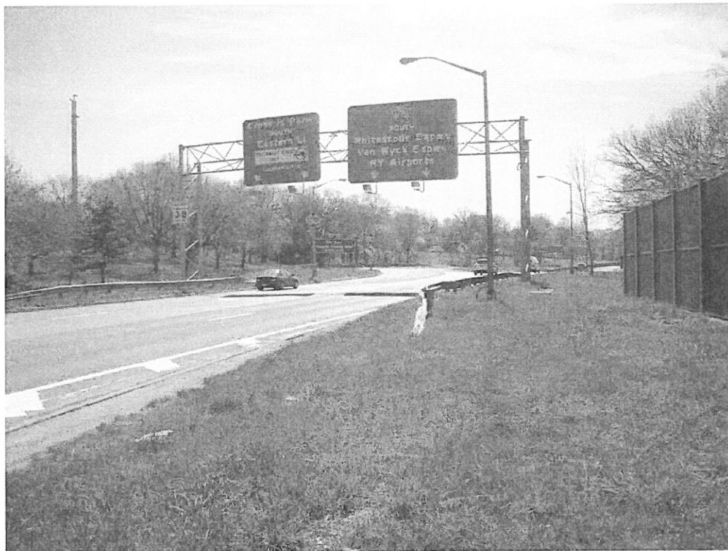
Photo 15. View southeast from southbound 14 th Avenue Exit (Parsons Road exit). The roadways in the APE from this point south simply will be repaved.
