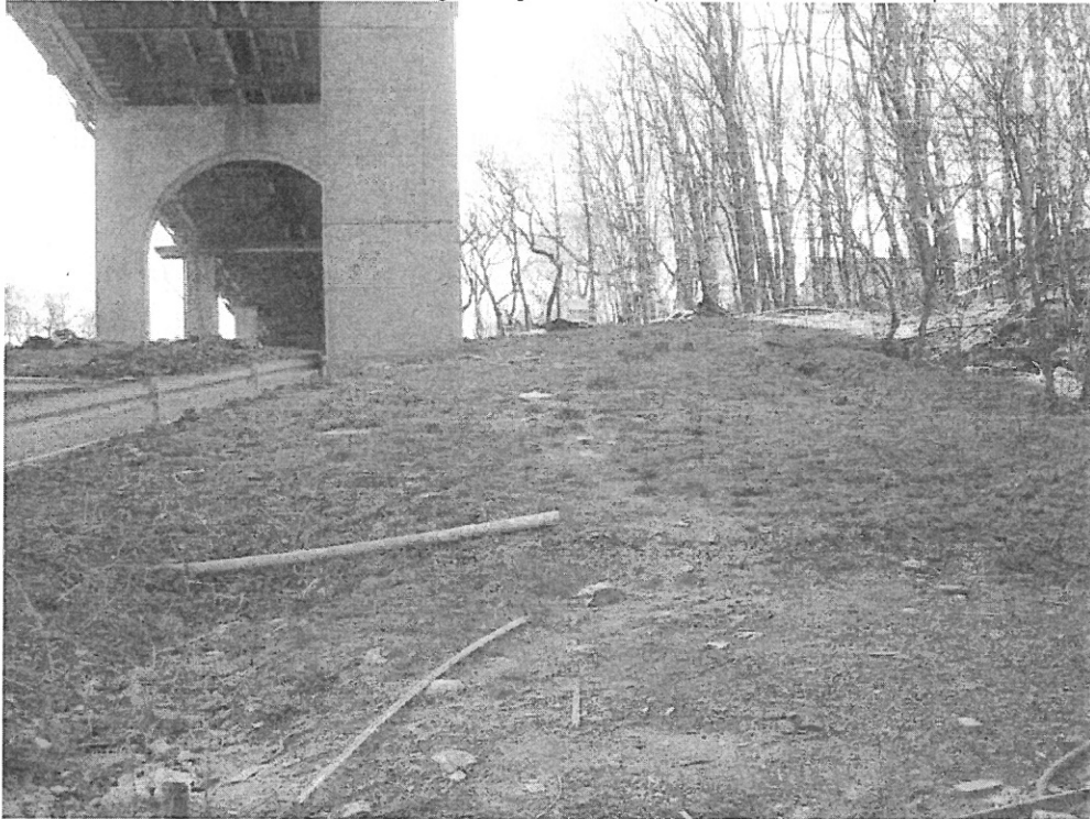
Photo 2. View southeast along the west side of the project area in vicinity of Pier 1Q and proposed outfall.
