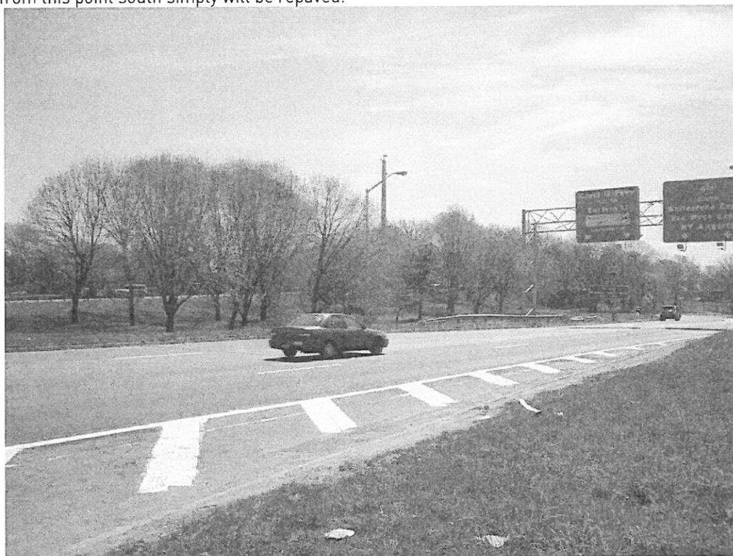
Photo 16. View east from same vantage point as Photo 15 across southbound Whitestone Expressway lanes. The staging area is seen in the center of the photograph.
