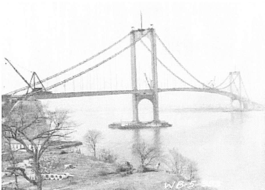
Photo 21. This photograph shows a view from Queens of the bridge during construction. Note the structure in the lower left of the photograph in what is now Francis Lewis Park. It appears the area was also used for staging. (Photographer and date unknown; from MTA From the Archive 2002:5)
