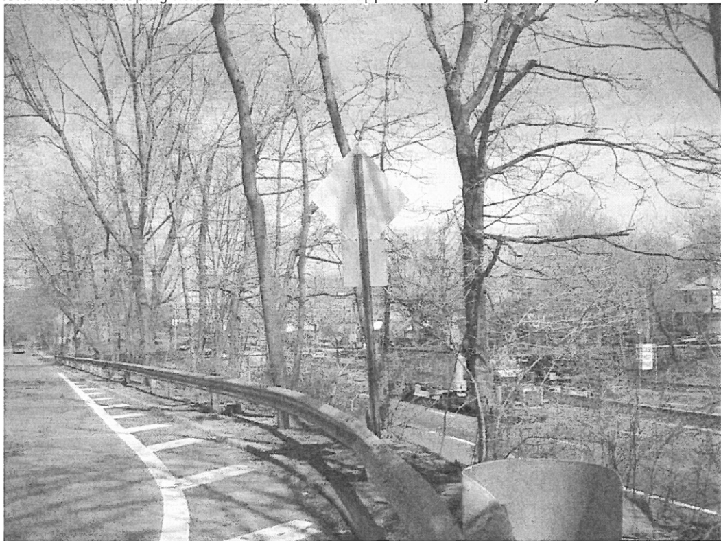
Photo 14. View north from the west side of the project looking across Whitestone Expressway. Note slope down to existing roadway.
