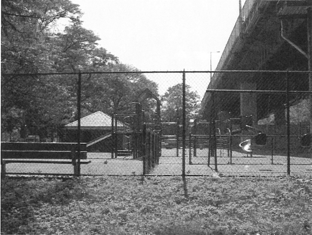
Photo 5. View south toward existing Francis Lewis Park playground with bridge approach to the west.
