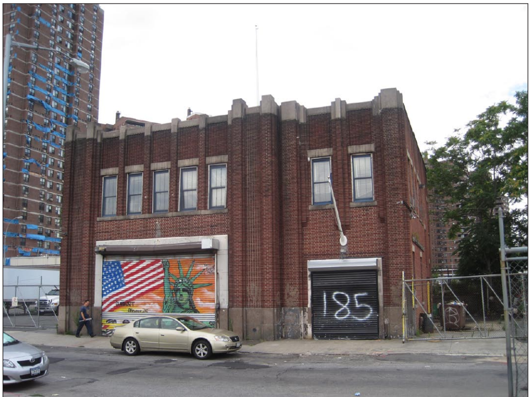
The existing structure along the northern side of Site 5
