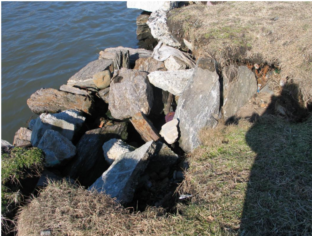
Photograph 10: Project site showing typical rubble fill behind deteriorating seawall. View looking north.
