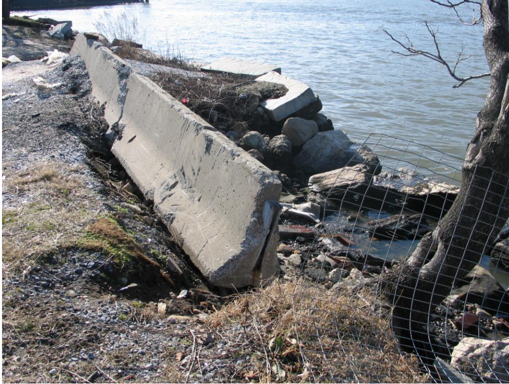
Photograph 11: Project site showing concrete jersey barrier along breach of seawall. View looking southwest.
