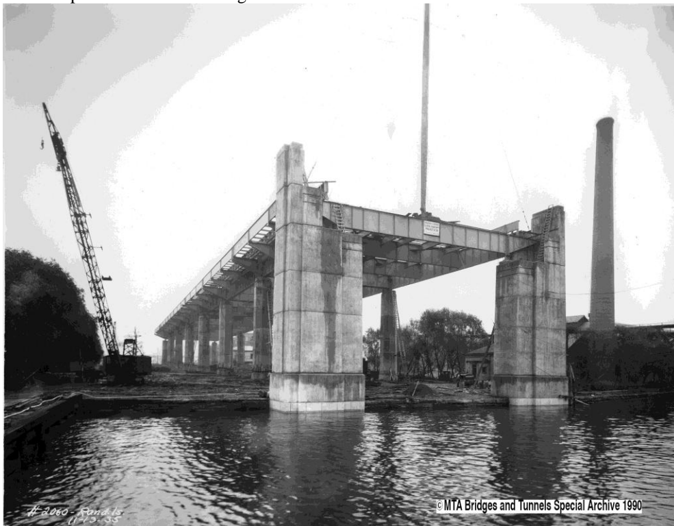
Photograph 20: “Randall’s Is./Roadway steel in place from pier 16 eastward. View east from point on “Police Dock Landing.” Image 2060, contract 31-A, courtesy MTA Bridges and Tunnels Special Archive. 11-13-35. Waiting room and store building and smoke stack for power house are visible on right.
