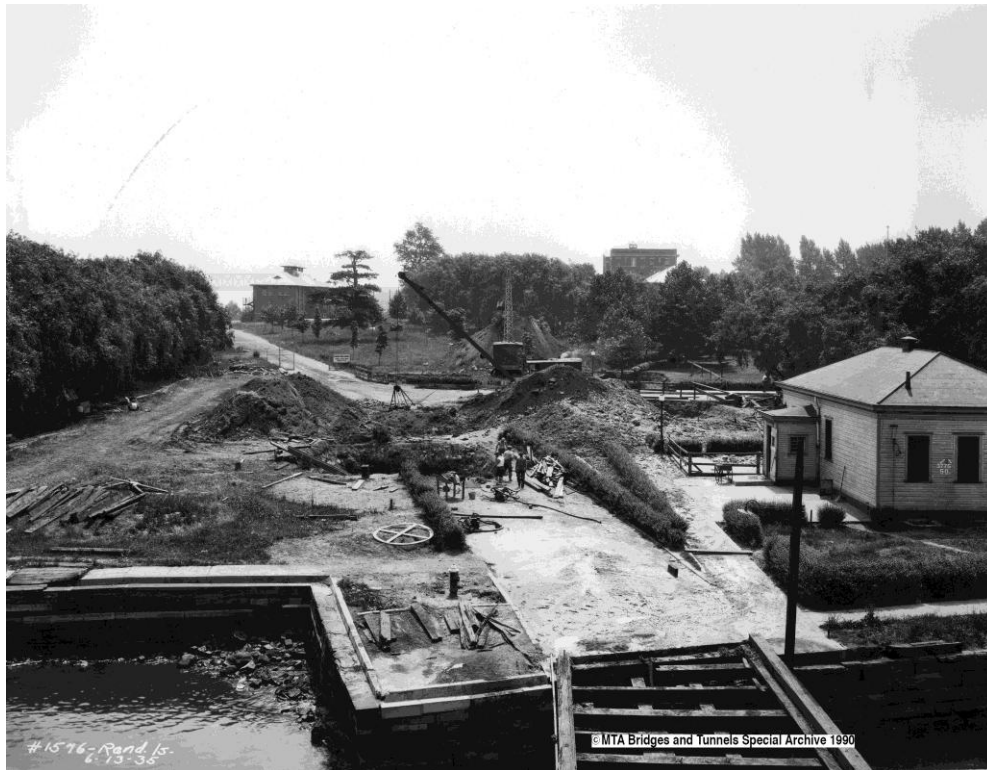
Photograph 17: "Randall's Is, general view of operations for pier footings. View east from top of Randall's Is. ferrybridge hoist." Image 1576, contract 31-A, courtesy MTA Bridges and Tunnels Special Archive. 6-13-35. Waiting room and store building is on right.
