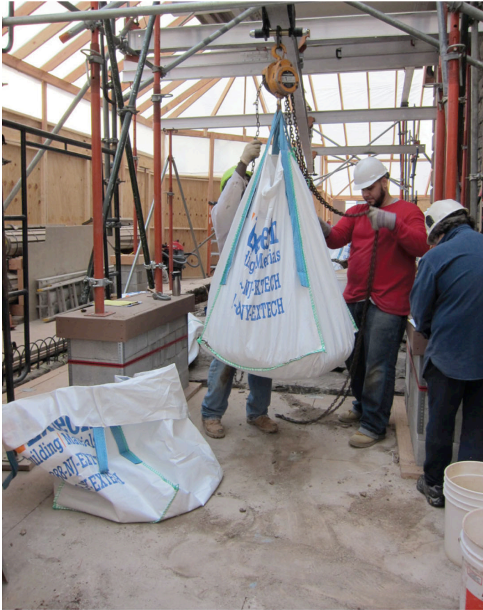
Photo 10. ICC crew moving a soil-filled Tyvek bag to the screening area out of view to the right. (3/19/12)
