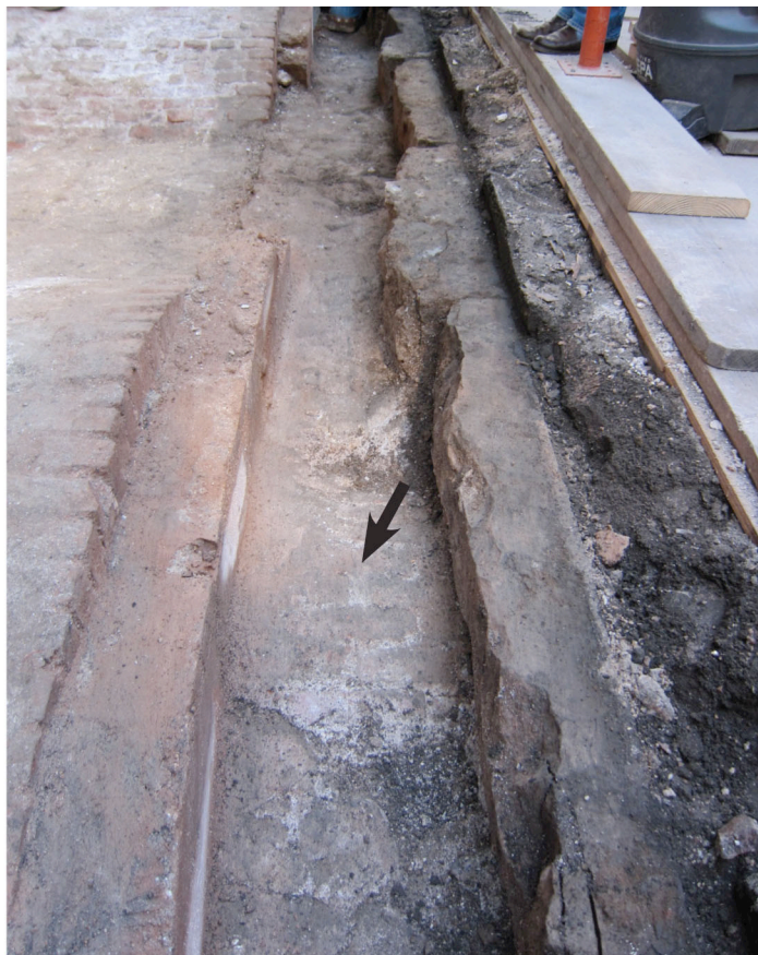
Photo 13. Further excavation along the western edge of the vaults partially exposed the brick "tunnel" (arrow) enclosing underground steps to the Waddington vault. The west retaining wall (right) is to be replaced. (3/27/12)
