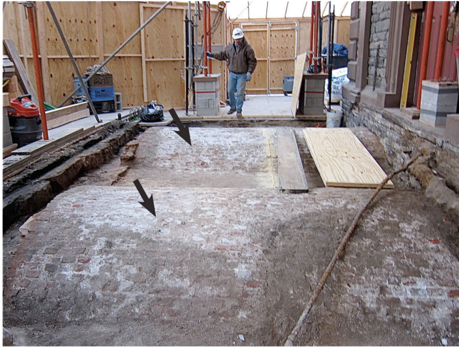
Photo 12. The top of the arched brick Waddington (upper arrow) and Ogden (lower arrow) vaults fully exposed. The view is north. (3/27/12)
