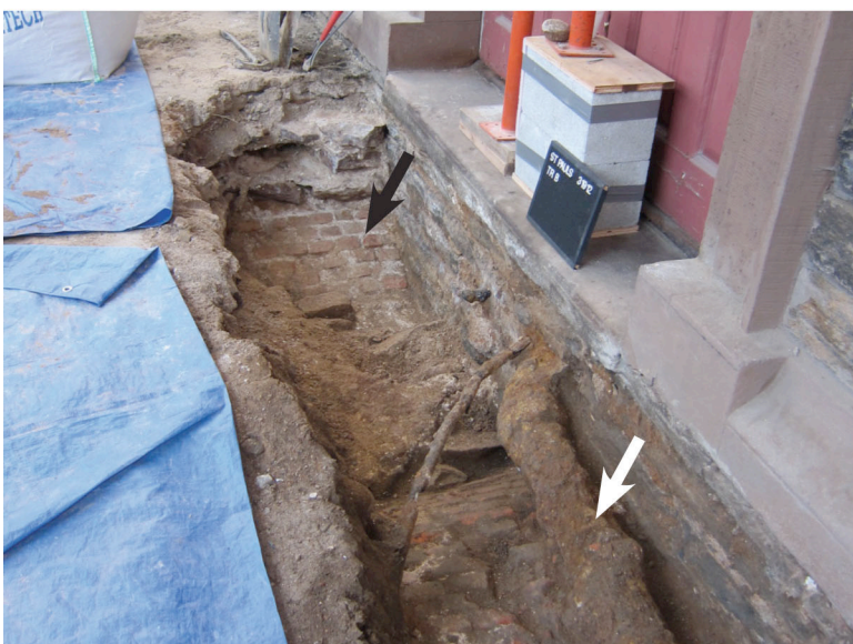
Photo 9. Excavation of Trench B (TR B) revealed that both vaults about the rear chapel wall. Waddington's vault (upper arrow) is intact but Ogden's has been compromised but not breached by a sanitary drain (white arrow) that runs along the back wall. (3/19/12)
