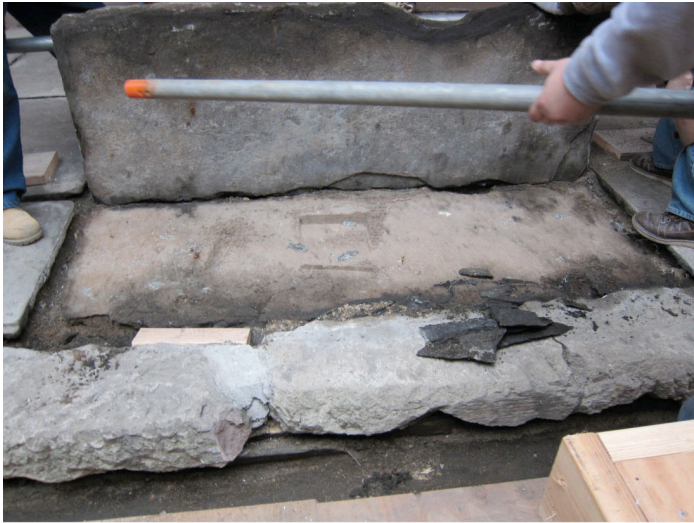
Photo 1. An ICC crew person is lifting a paving stone in the northwest corner of the portico to expose the sand and stone beneath it. The west retaining wall and the construction shelter's flooring are in the foreground. (2/24/12)
