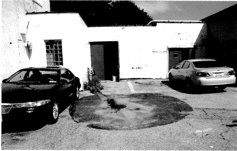
Fig. 5. View of one of the drywells at the western end of the parking lot on the project site.
