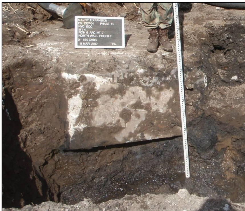
Photograph 5-1. Concrete footing with rebar located along north wall of MT-4, view north.
