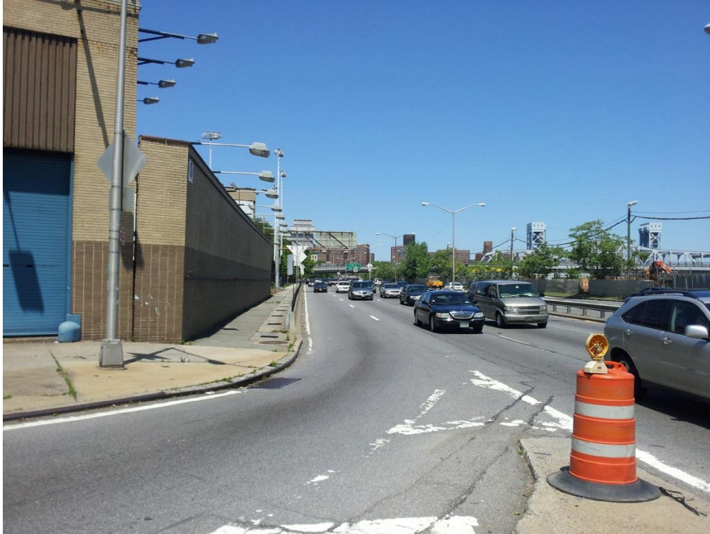
Photograph 1: Southbound Harlem River Drive at Second Avenue exit towards the north northwest. Third Avenue Bridge in the background.
