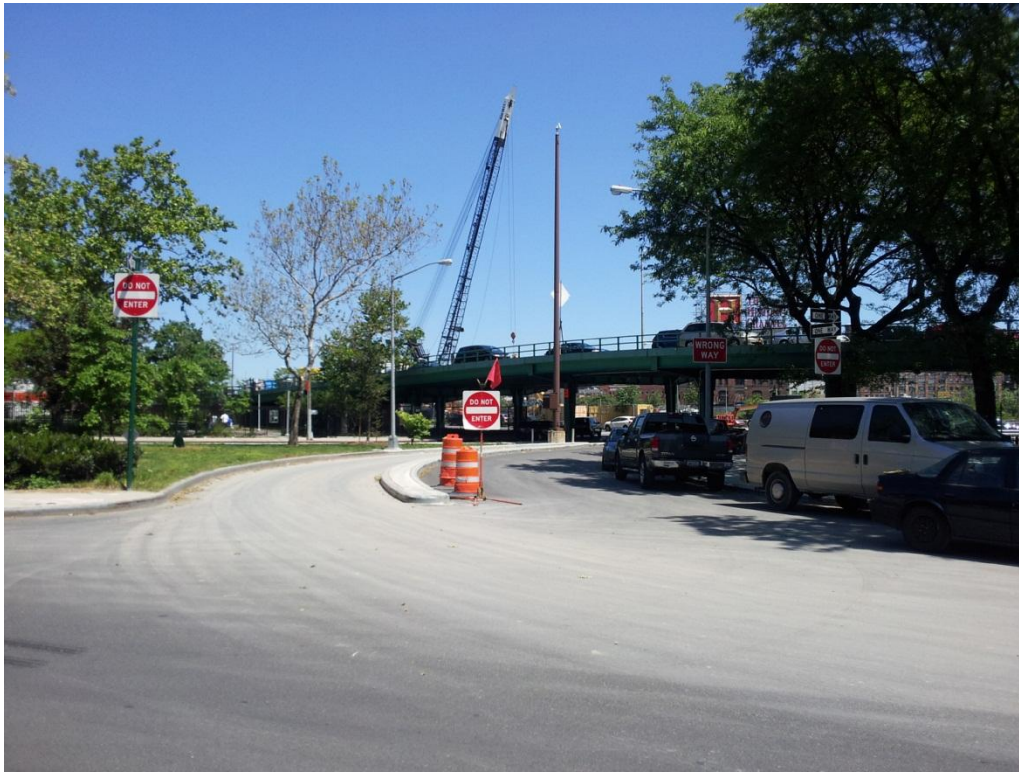
Photograph 9: Ramp B toward the northwest from East 127 th Street.
