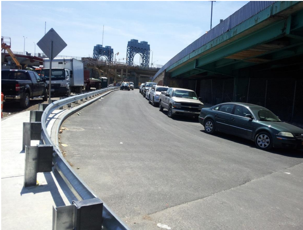
Photograph 11: Exit off northbound Harlem River Drive before it crosses under the highway to Ramp B, towards the southeast with the RFK Bridge in the background.
