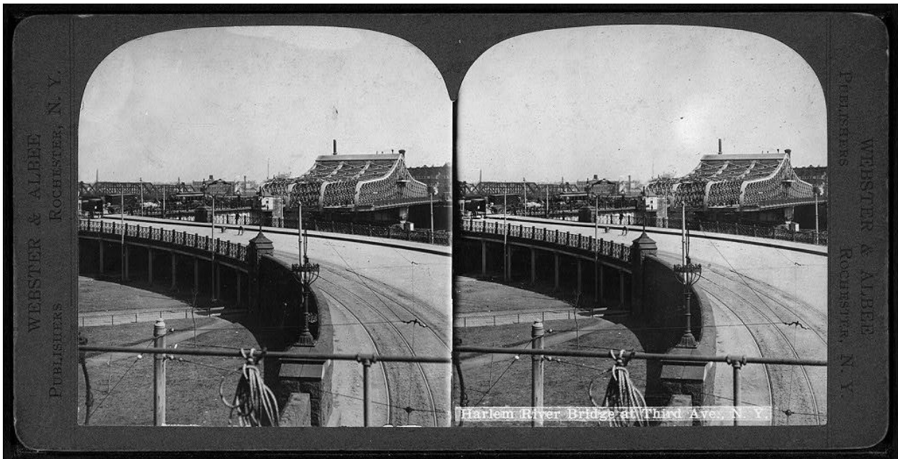
FIGURE 13b: Harlem River Bridge at Third Avenue, New York. (The Extant Bridge) Robert Dennis Collection of Stereoscopic Views. No date. Note the extensive system of piles supporting the entrance ramp.
