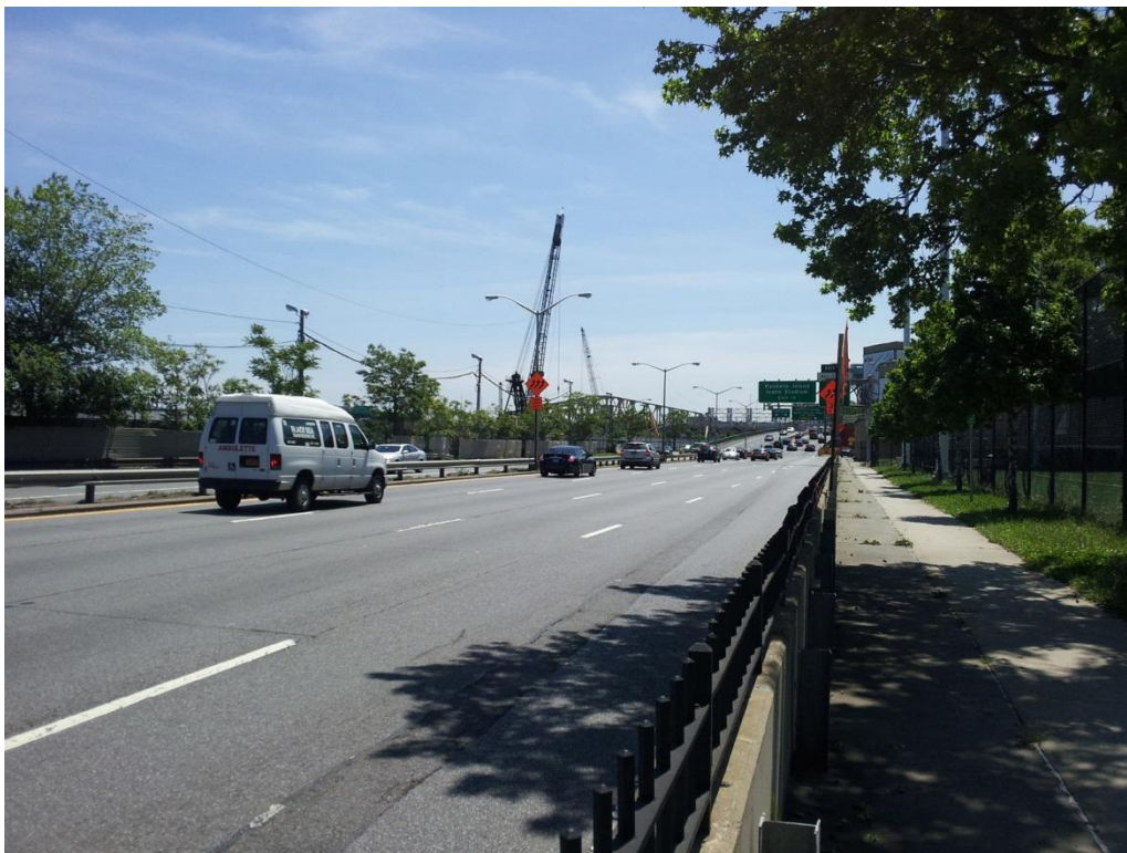
Photograph 2: Southbound Harlem River Drive towards the south southeast. Willis Avenue Bridge in the far background.
