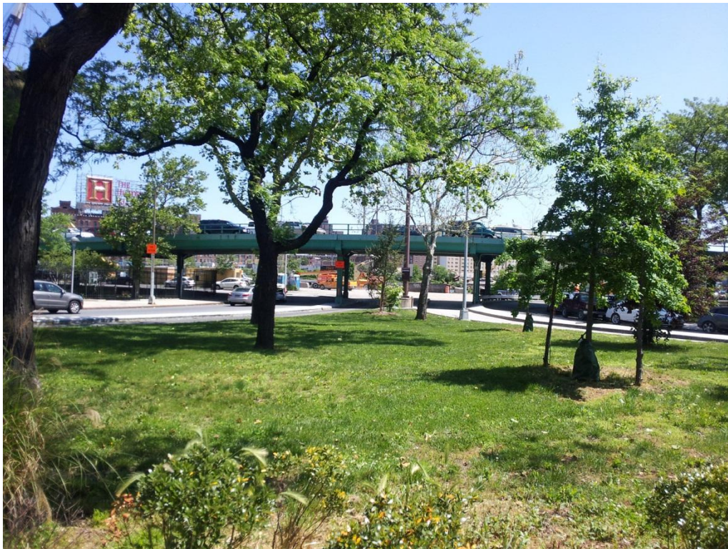
Photograph 8: Ramp C on the left and Ramp B on the right, toward the northeast, with Harlem River Drive in the background.
