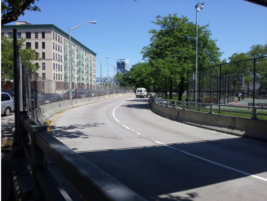
Photograph 3: Ramp A to Southbound Harlem River Drive towards the northeast.
